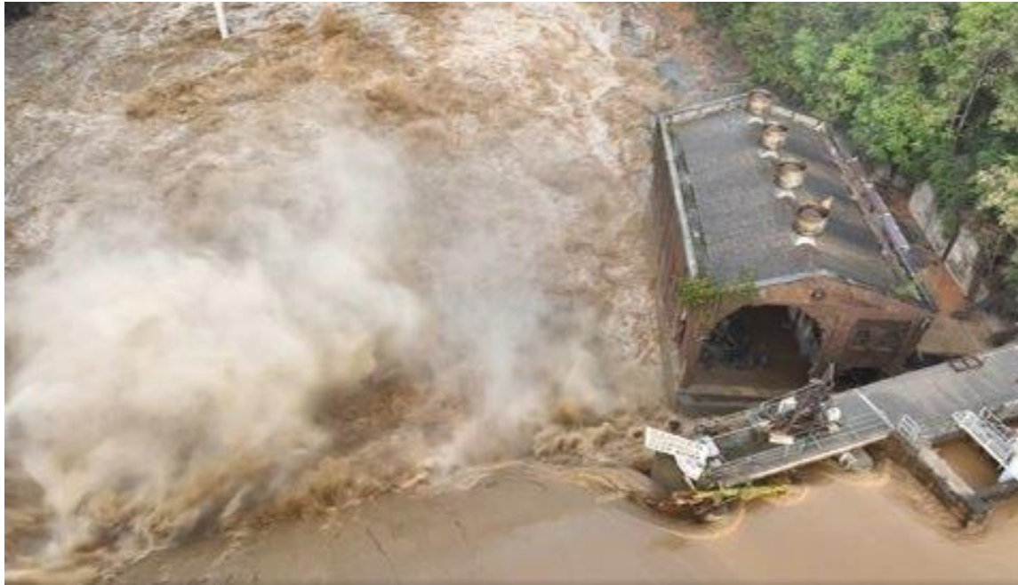
Nolichucky Dam and Powerhouse September 2024
