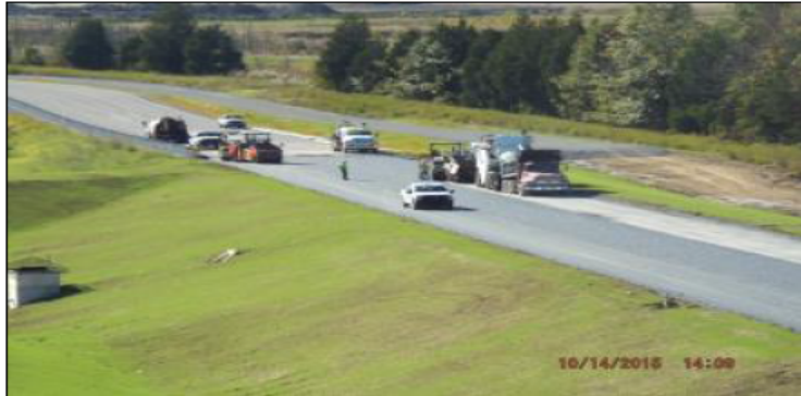
Haul Road paving
