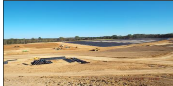
50% of Liner installed
