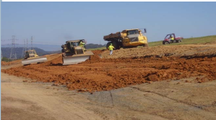
Construction of Improvements at Bull Run
