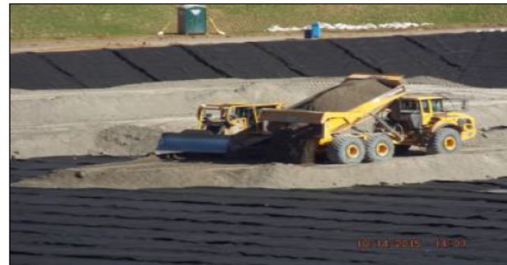
Placing Protective Cover
