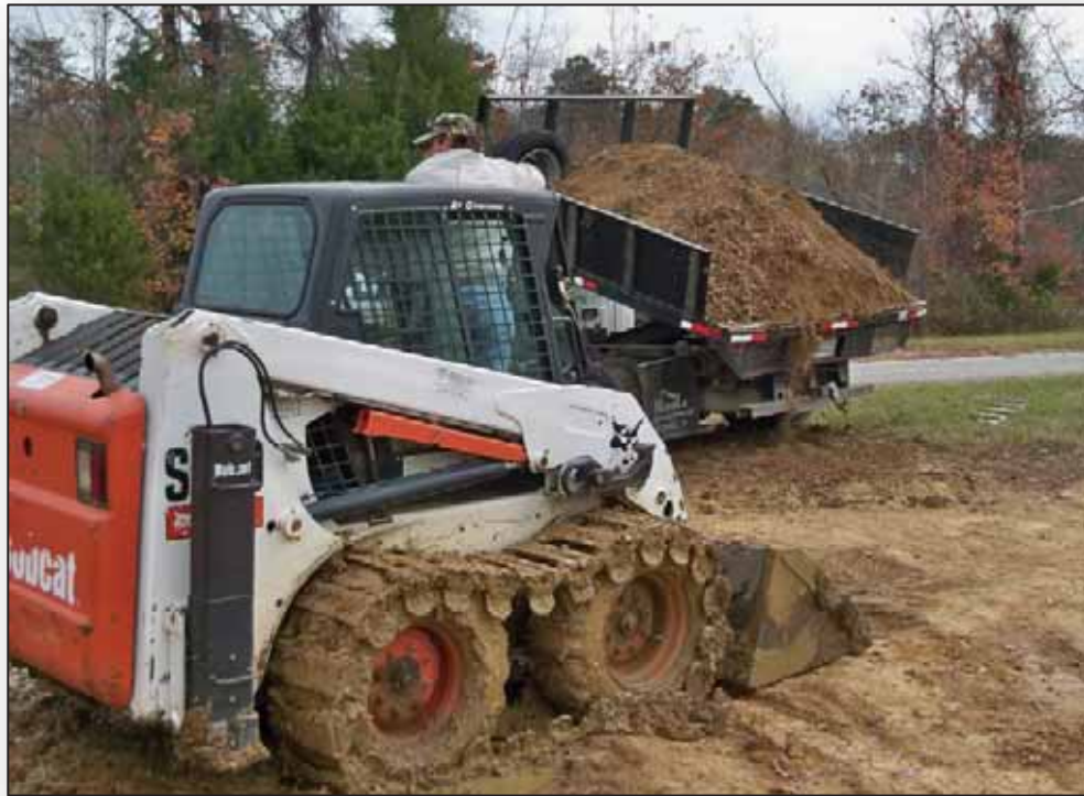
In Progress: Filling holes
