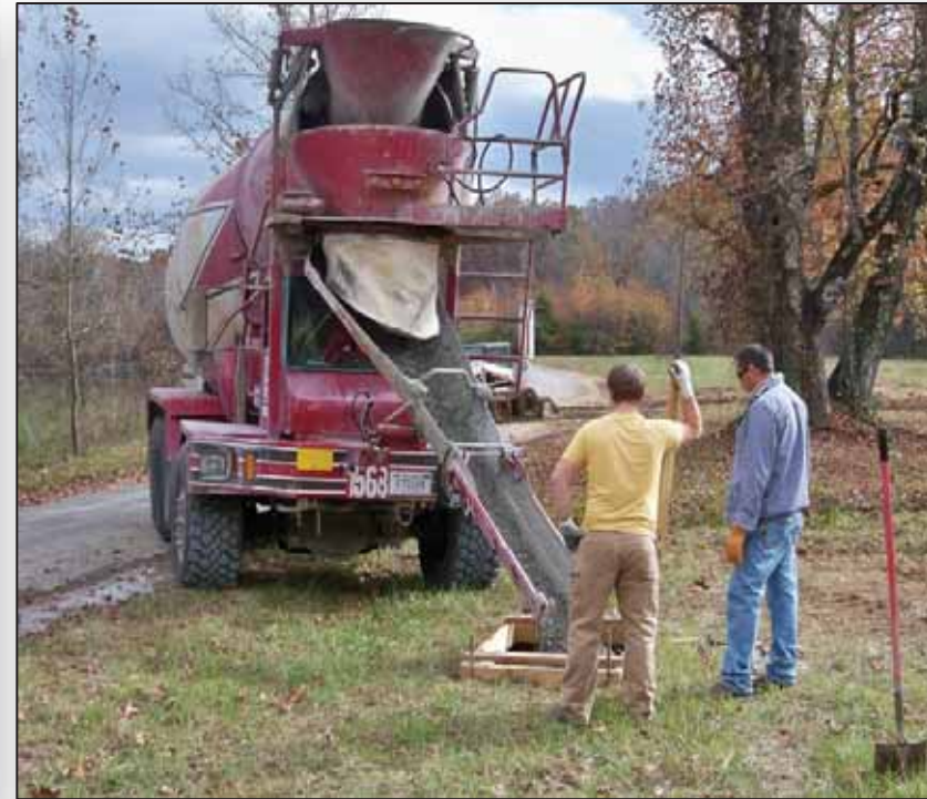
Concrete pads for Trash Cans
