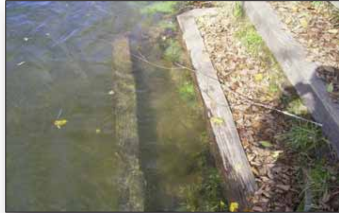
Fannin County – Curtis Switch Stream Access Below Blue Ridge Dam
