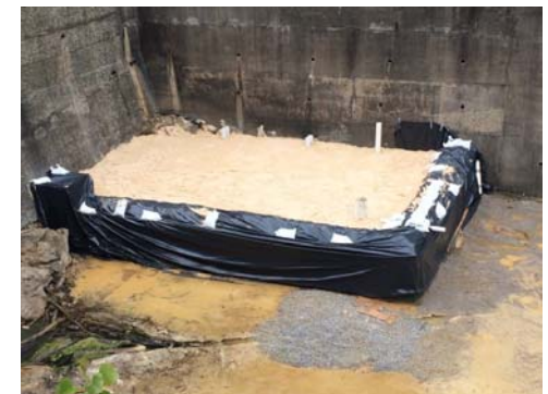
Sand filter completed 05/12/17
