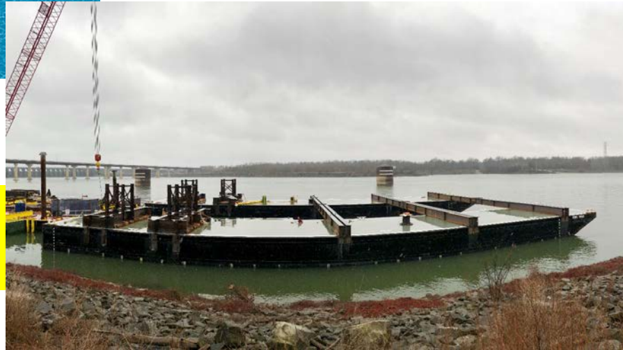
2 Feb 2018 – Gantry barge system being assembled
