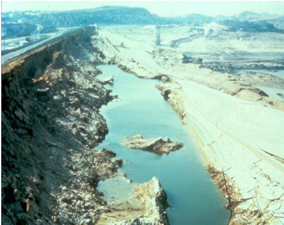
LOWER SAN FERNANDO DAM - CALIFORNIA
