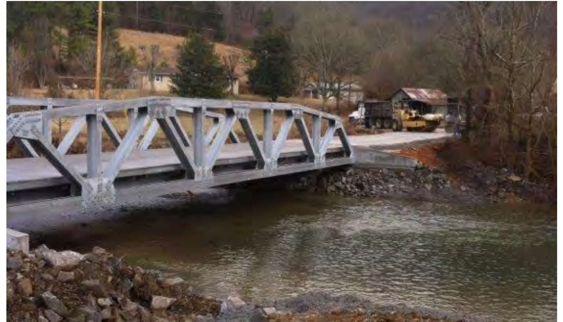
Estill Fork Bridge (After)
