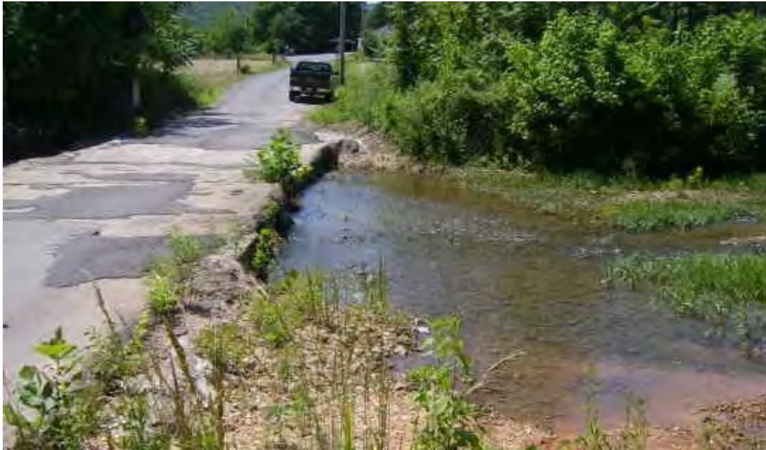
Estill Fork Bridge (Before)
