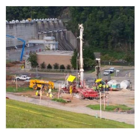
An average of 90 workers are on site daily drilling and testing different grouting formulas for use during the full-scare repair project scheduled to begin soon.
