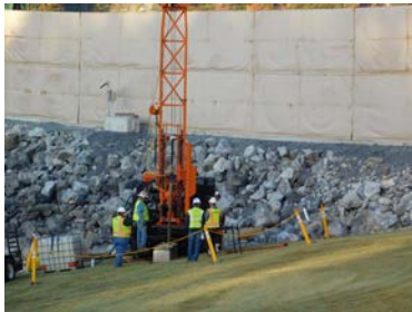
Drilling can be seen on the right rim of the earthen embankment.
