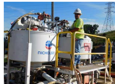
Satellite tanks store pre-mixed grout before it is pumped into boreholes
