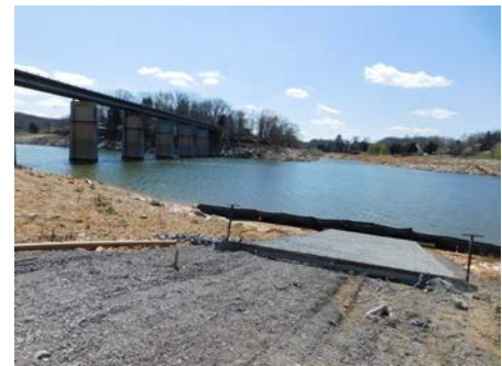
Concrete slab for new boat ramp at Devault Bridge
