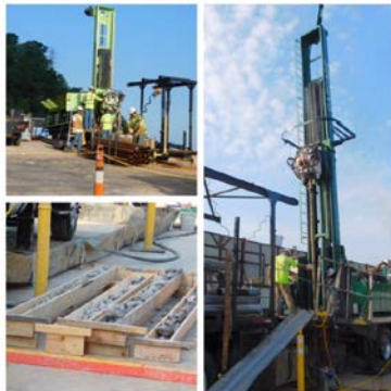
Above: Two sonic drill rigs and core samples pulled from the dam's earthen embankment. Below: TVA Vice President David Bowling provides an update for area officials and representatives about the project. Project Manager Sam Vinson speaks with local media.
