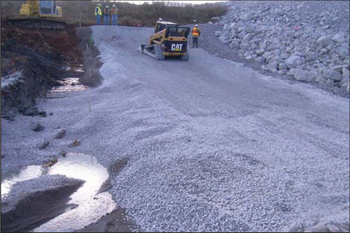
Placing layer of gravel on top of sand material in panel. December 27, 2009.
