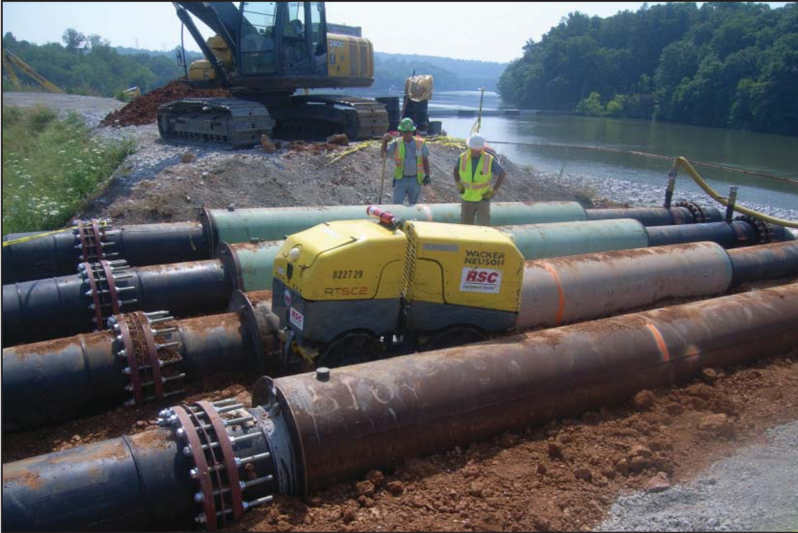
New siphon installation. June 7, 2011.
