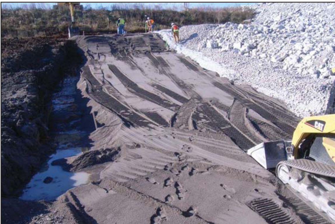
Placing layer of sand on top of dike material in panel. December 29, 2009.
