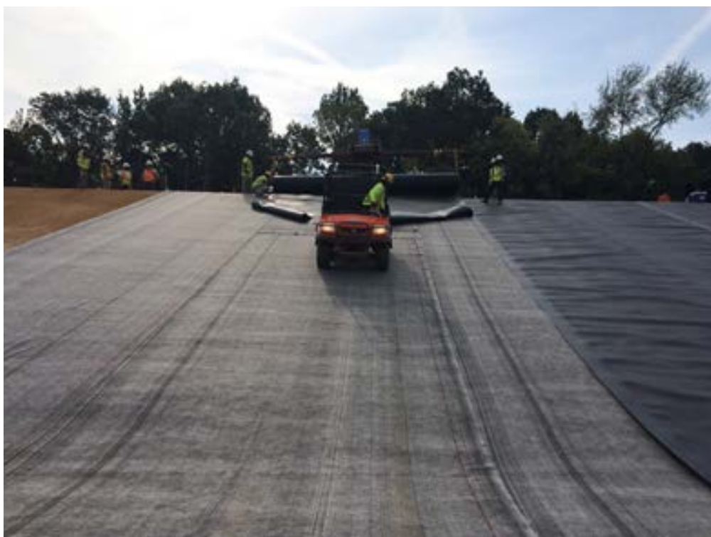
Install geomembrane over geosynthetic clay liner
