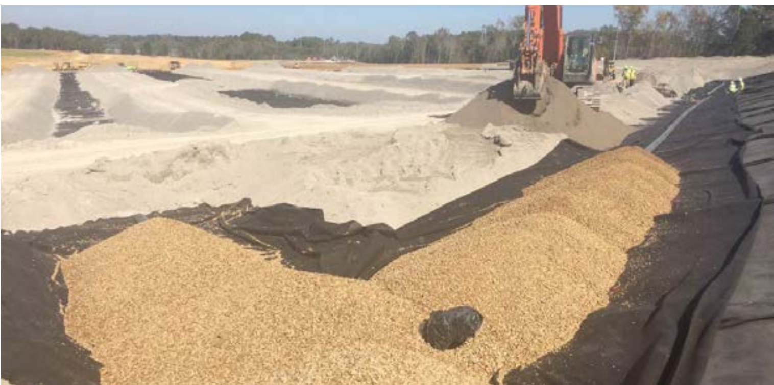
Install protective ash cover layer and perforated leachate collection pipe
