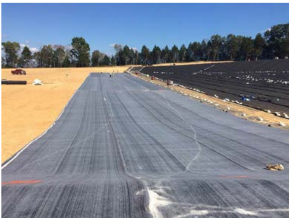
Place geosynthetic clay liner over compacted clay liner
