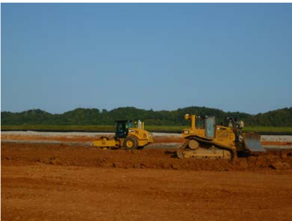
Place geologic buffer and compacted clay liner
