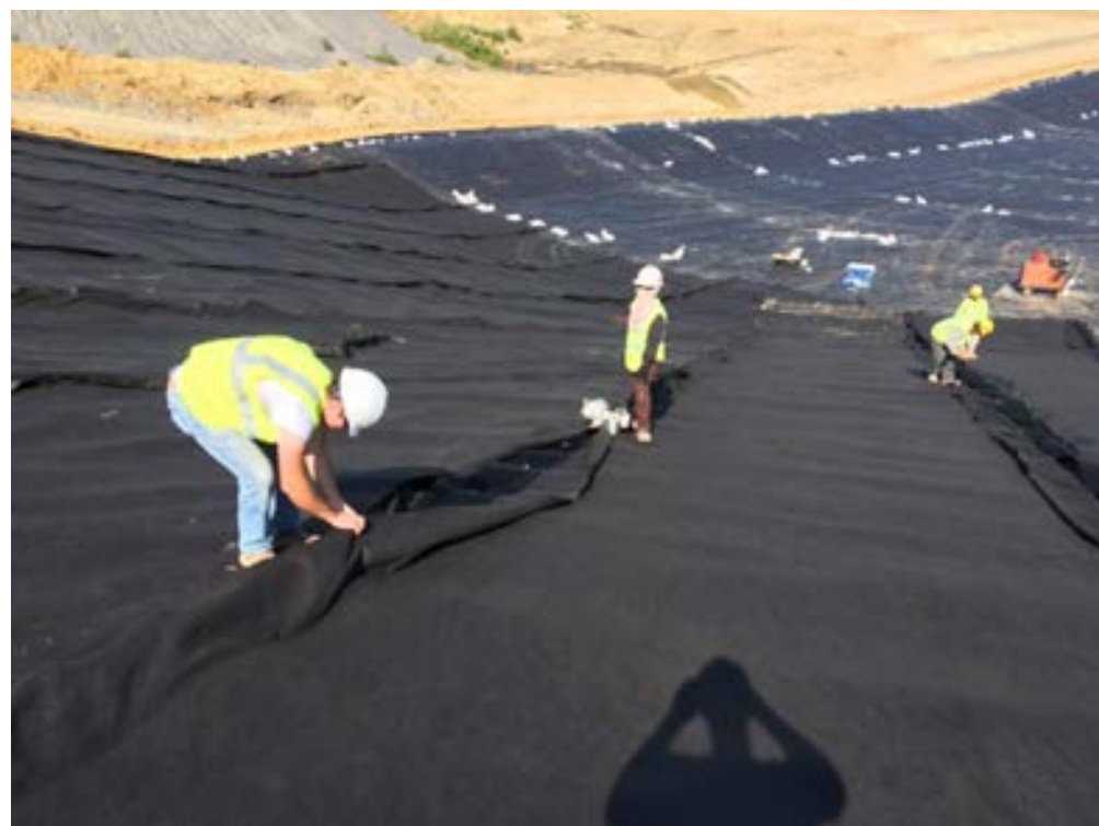
Install geocomposite drainage layer over geomembrane
