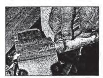
Figure 4.28. Score a line from top of liner to base of liner drive head using a utility knife.
