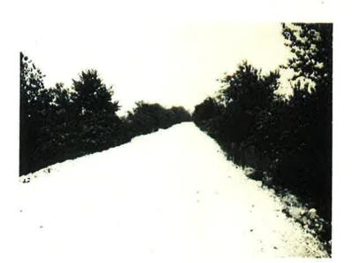
Area 2 East dike after being raised 1-foot to elevation 378±. Note chert surfacing and vegetation.
