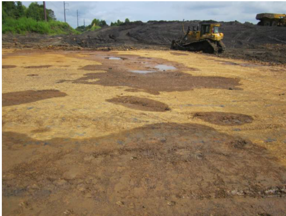
Figure 1. Excavation and Consolidation of CCR during Pond Closure (CDM Smith 2015)
