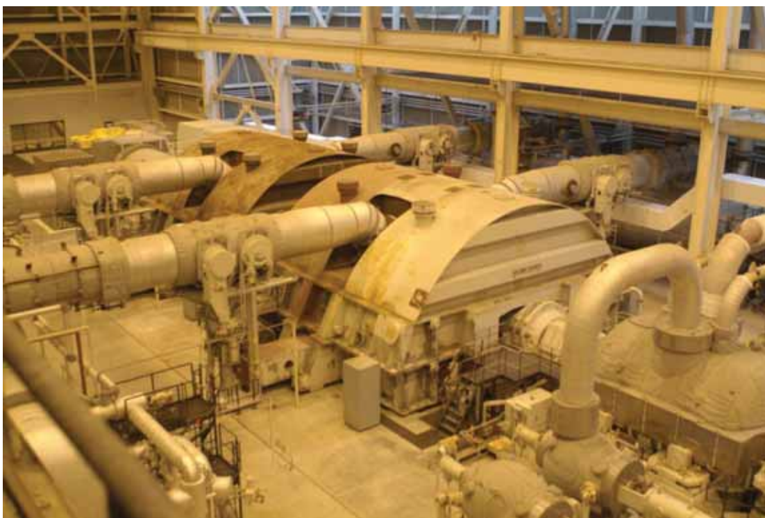
Figure 2-7. Unit 1 Turbine Generator
