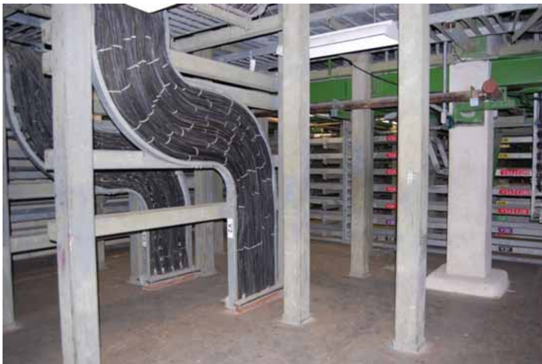
Figure 2-9. Cable Spreading Room
