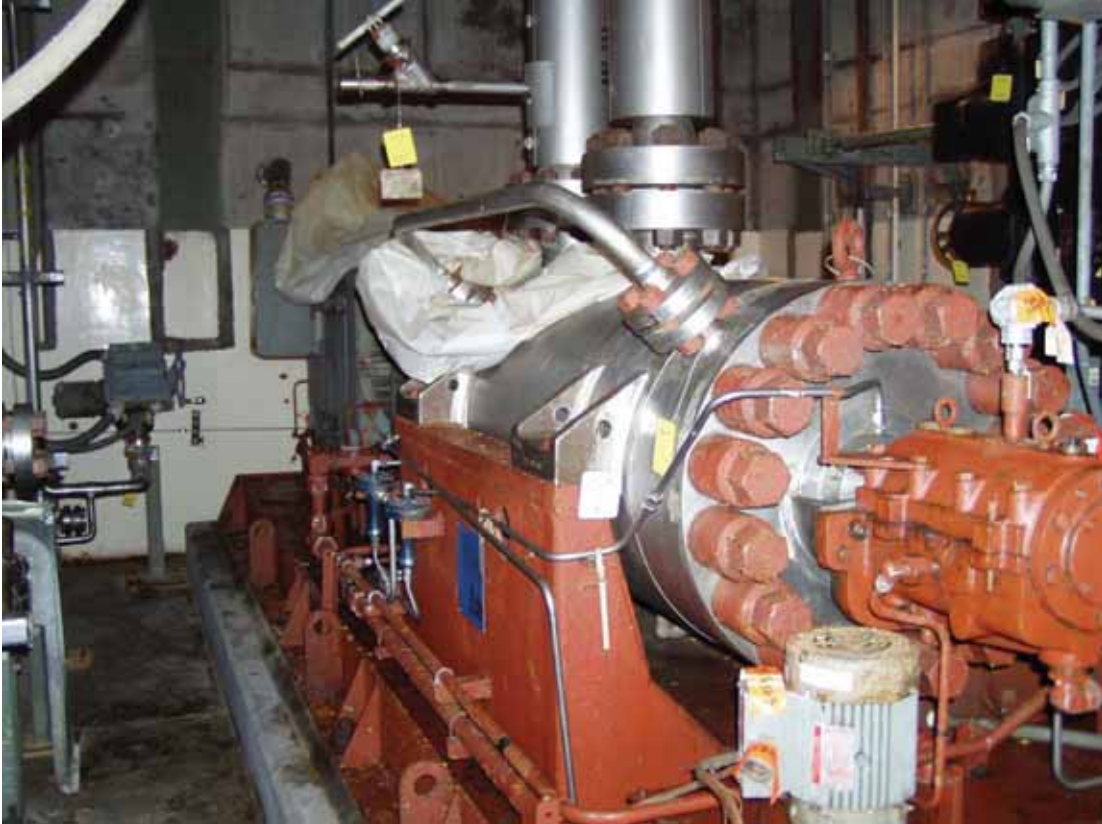
Figure 2-10. Unit 1 Makeup High-Pressure Injection Pump
