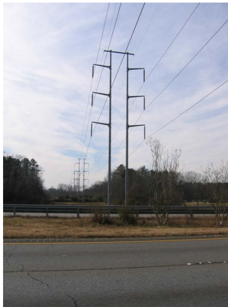
Figure 2-1. Typical Double Steel-Pole Structures, Double-Circuit Transmission Line
