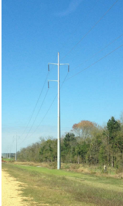
Figure 2-2. Typical Single Steel-Pole Structure
