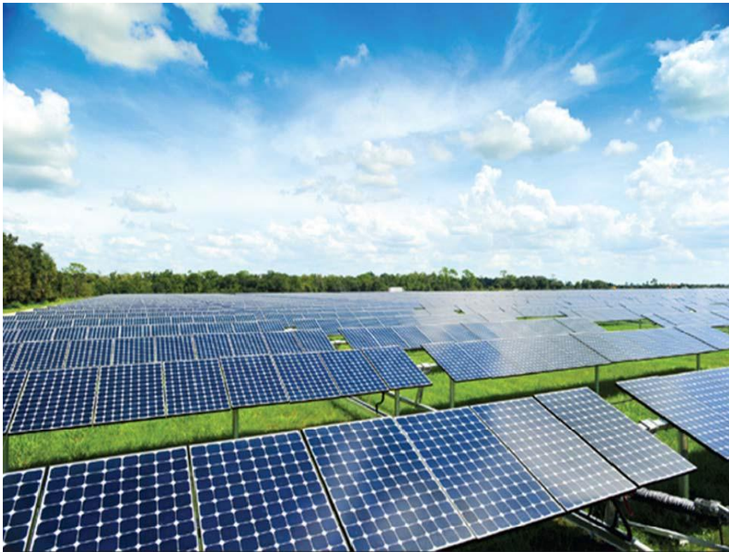
Photograph 3.5-5. Single-axis, tracking photovoltaic system with panels close to maximum tilt as viewed from the east or west.
