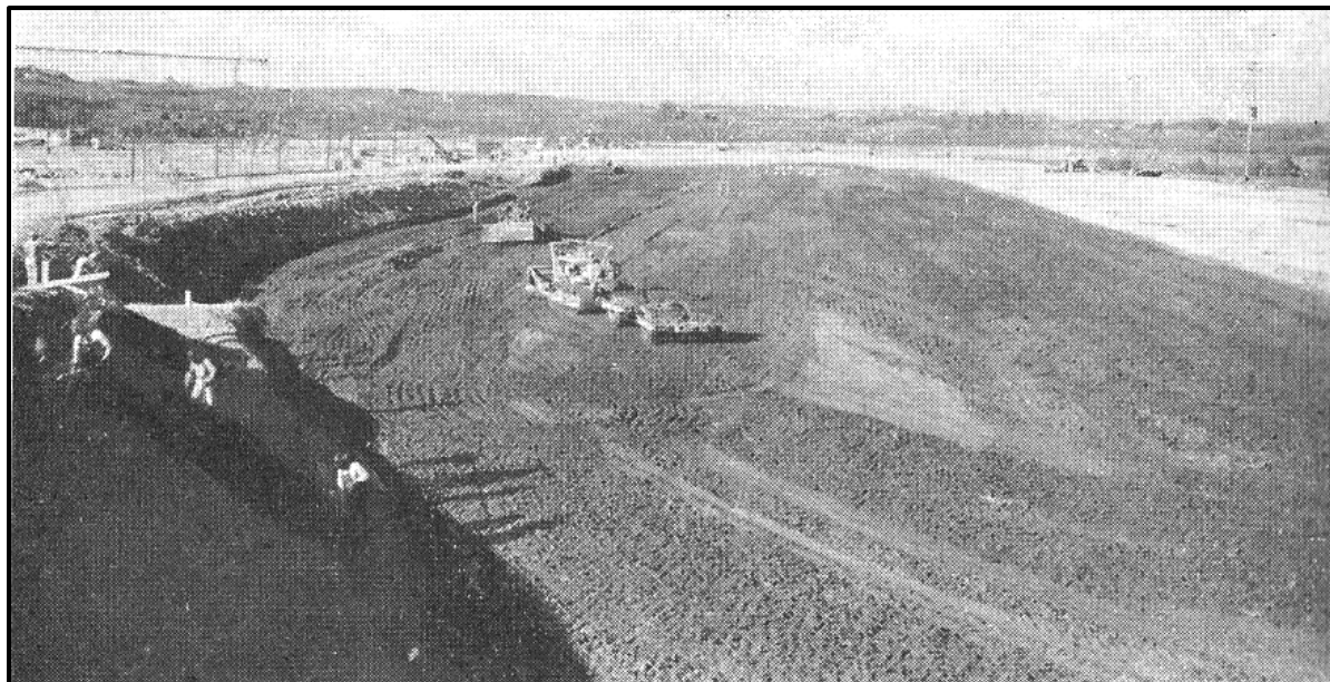
Figure 4. Photograph of the construction of the South Embankment at the Fort Loudoun Dam (downstream side) showing the degree of disturbance. View to the south. (TVA archives).
