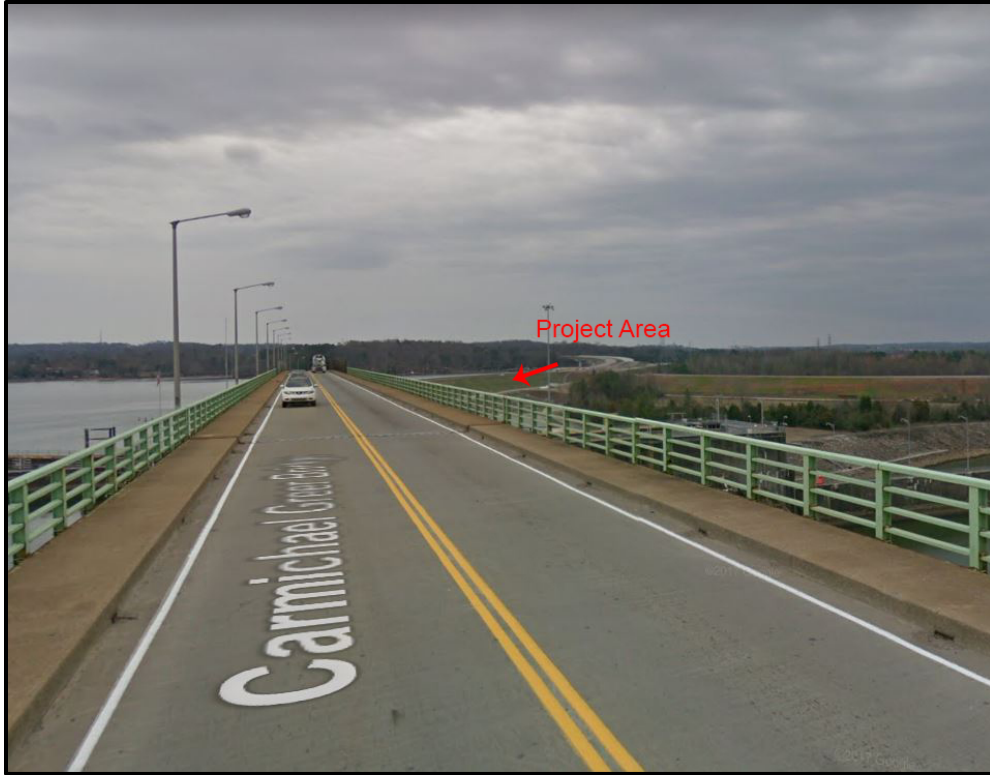
Figure 6. View of project area from Fort Loudoun Dam. View to the south.
