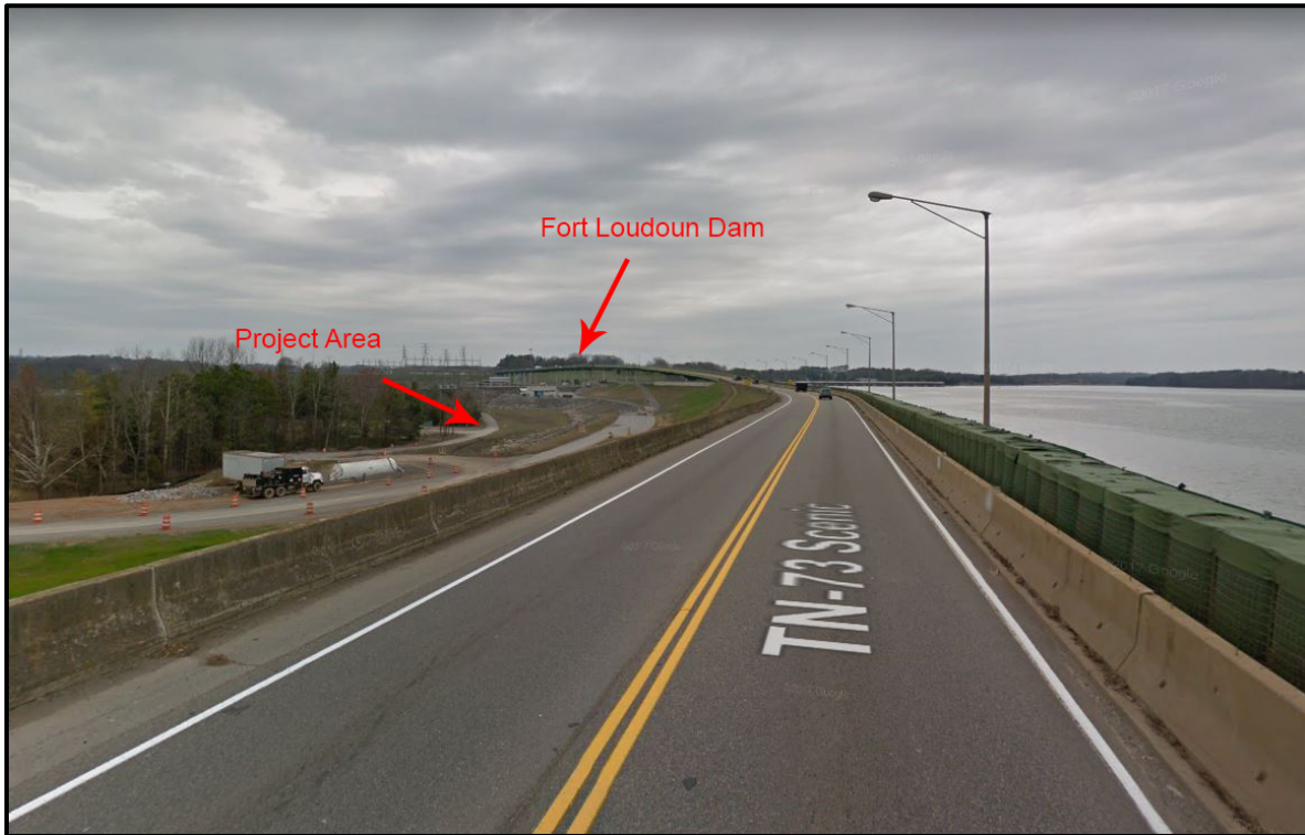
Figure 7. View of Fort Loudoun Dam from the project area. View to the north.
