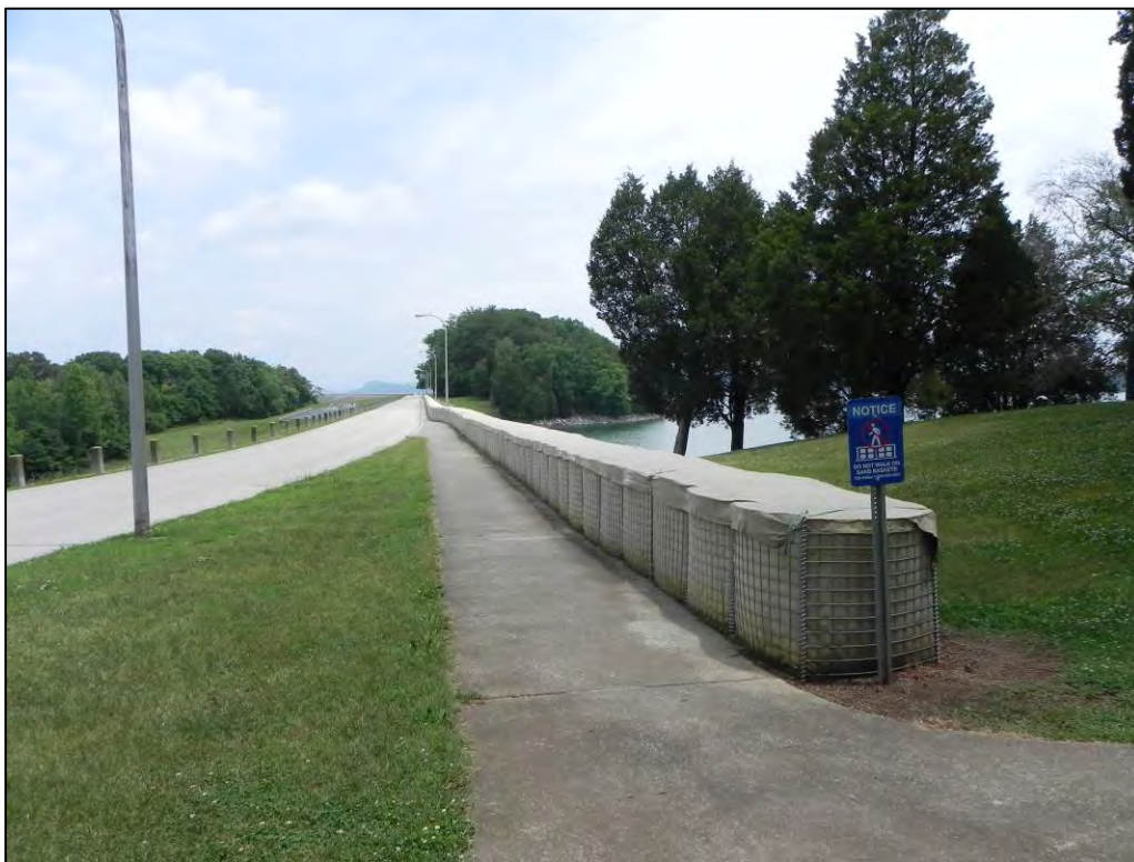
Photo 3.3-4a. View of Temporary Measures at Cherokee Segment C-3 (Facing Northeast)
