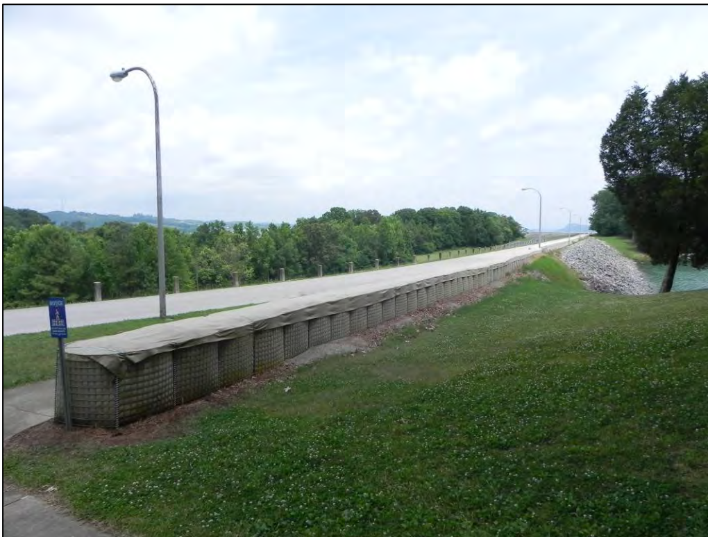
Photo 3.3-5a. View of Temporary Measures at Cherokee Segment C-3 (Facing North-Northeast)
