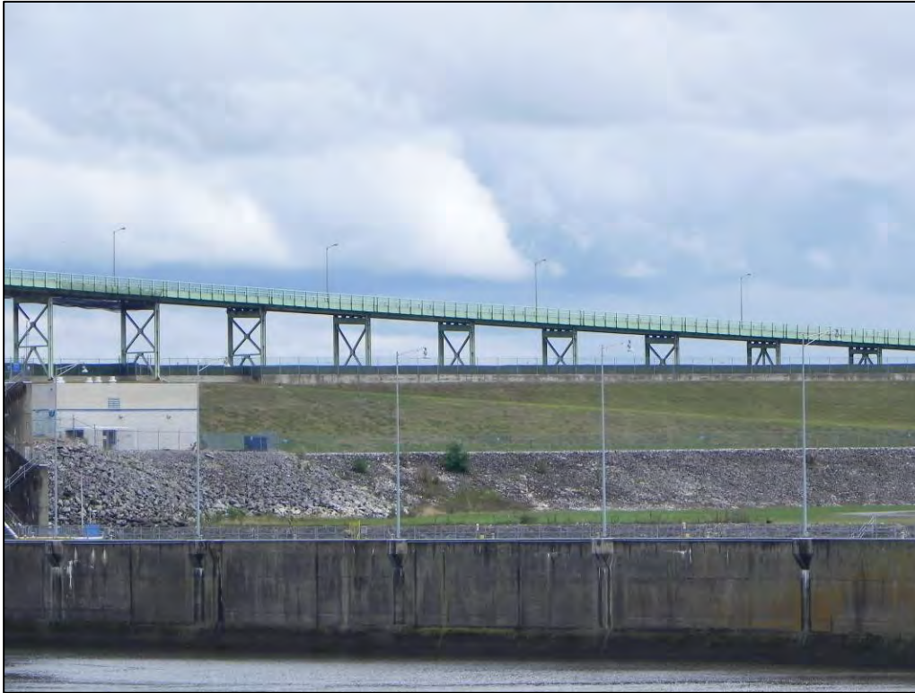
Photo 3.3-7a. Photo of Existing Temporary Measures at Segment FTL-2 (Under Bridge)
