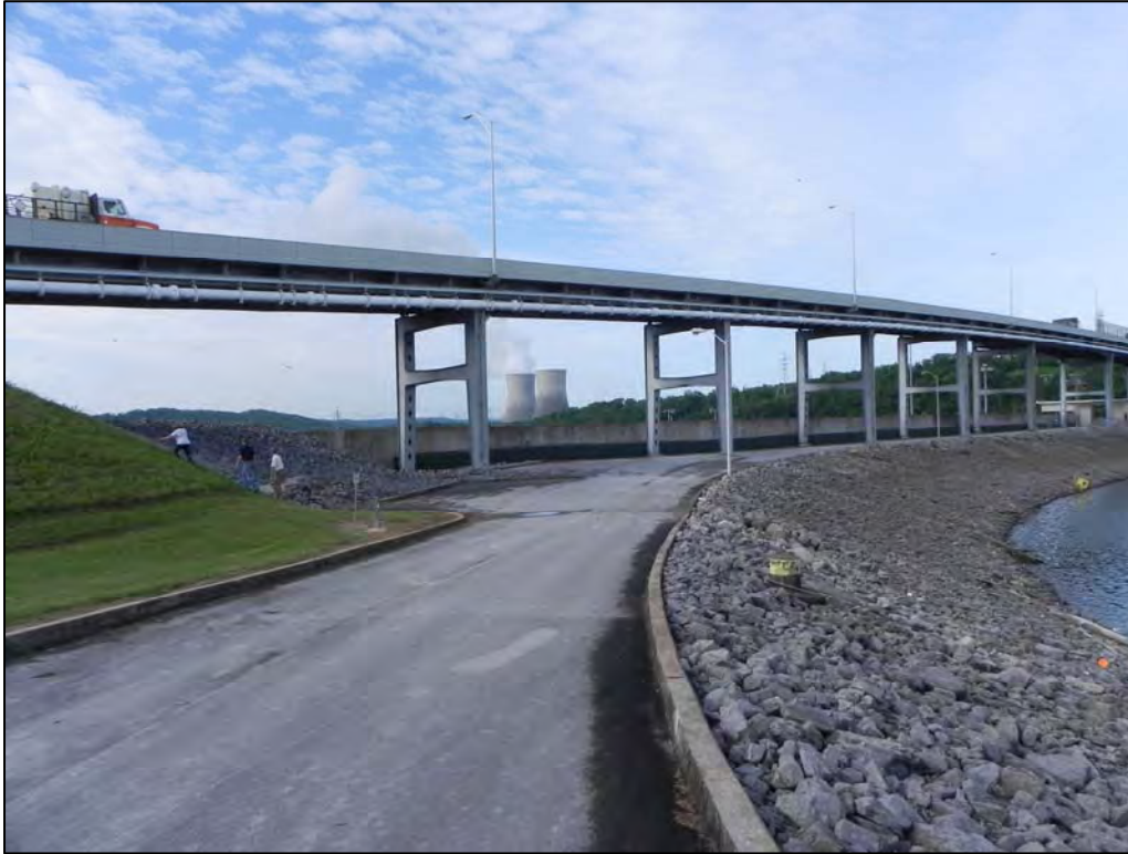
Photo 3.3-9a. Existing View of Segment WB-3 Floodwall and HESCO Barriers
