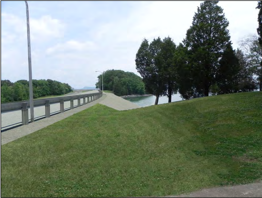
Photo 3.3-4b. Rendering of RCC (6.6-foot-tall) atop Segment C-3 showing optional guardrail under Revised Alternative B
