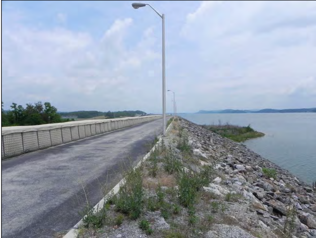
Photo 3.3-2a. Cherokee South Main Embankment with Temporary Measures
