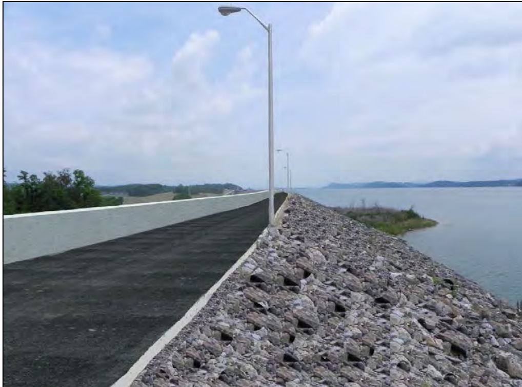
Photo 3.3-2b. Visual Rendering of Segment C-2 under Alternative B (6.6-foot-tall floodwall on the downstream side with a 3-foot-tall raised walkway)
