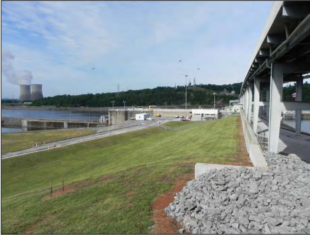
Photo 53. Approximate 2-acre Area of Watts Bar Dam Reinforced by Concrete Armoring during Temporary Measures (Facing Southwest)
