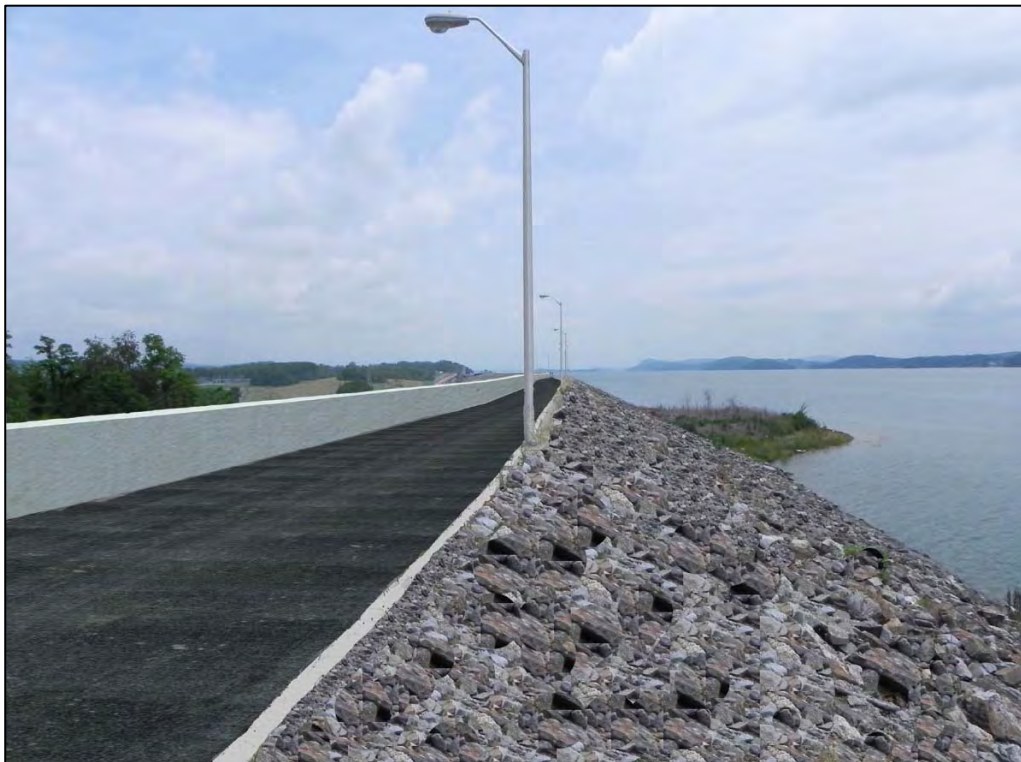
Photo 3.14-2b. Visual Rendering of a 6.6-foot-tall floodwall on the downstream side of Segment C-2 with a 3-foot-tall raised walkway at Cherokee Dam
