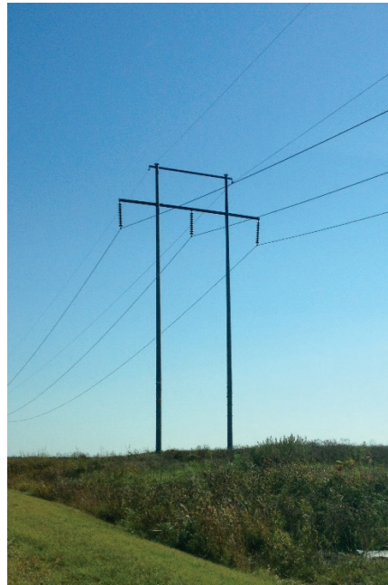
Photo 2.2-2. Proposed steel H-frame pole structure
