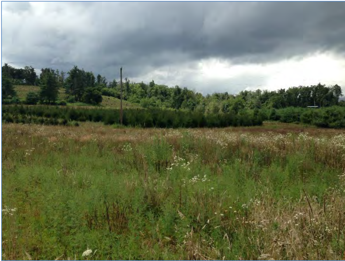
Photo 5. 1 MW Solar Farm (Avery Co.) - General view of the site from southeastern boundary looking northwest.
