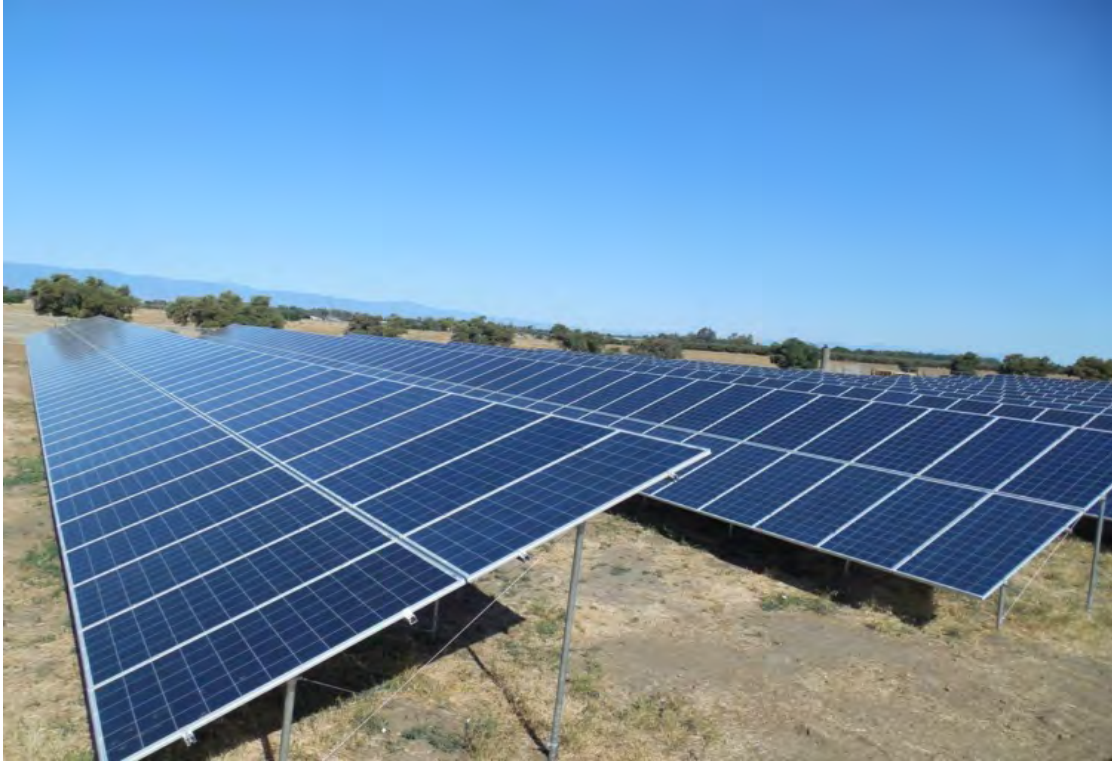
Figure 2-4. Example of fixed tilt photovoltaic array.
