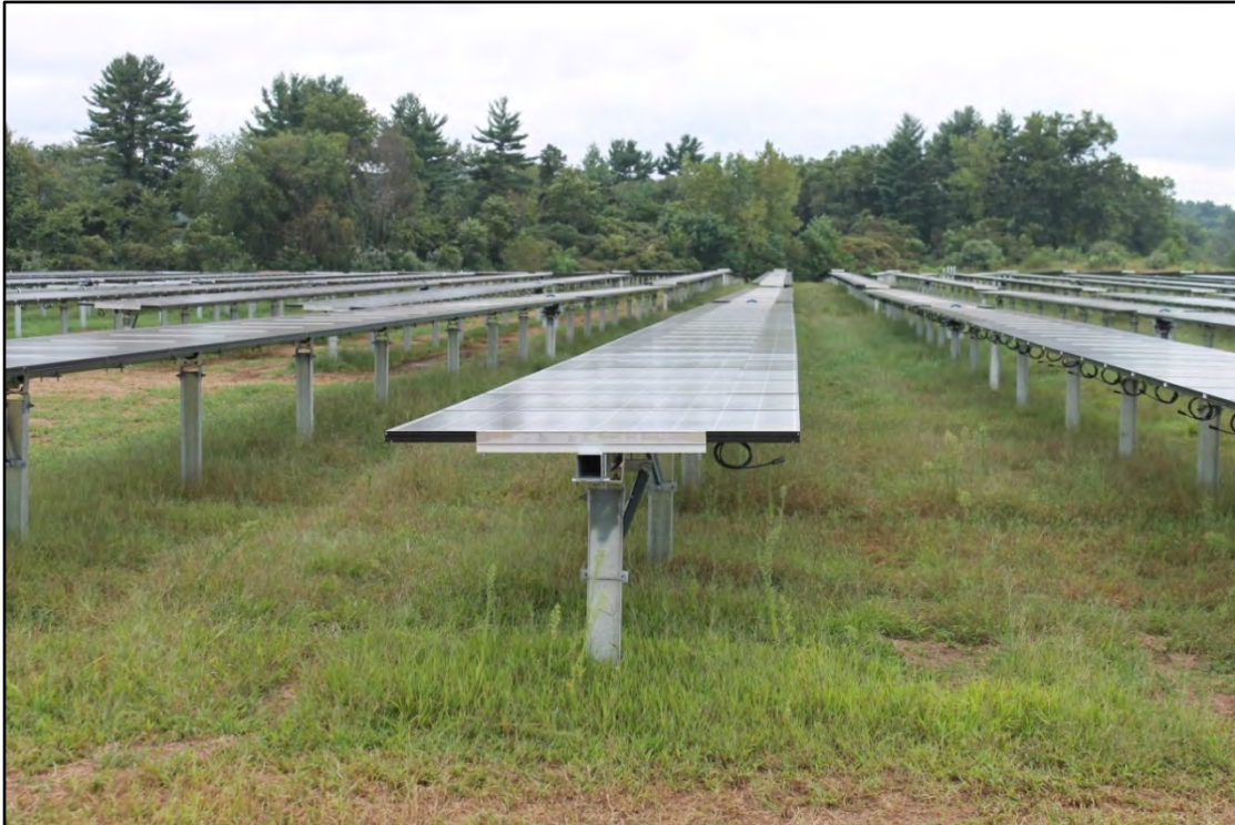
Figure 2-3. Example of single-axis tracking photovoltaic array.
