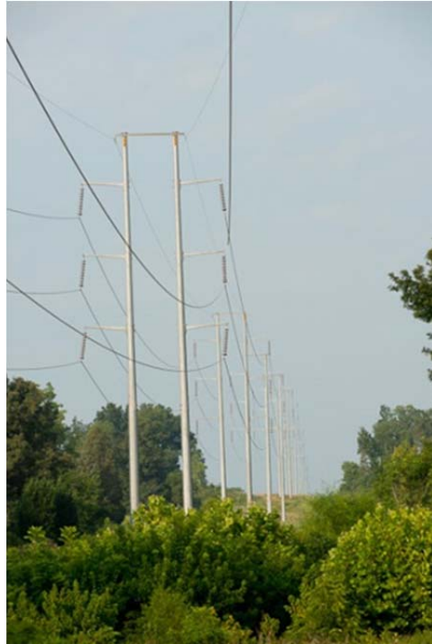
Figure 2-1. Typical Steel-Pole, Double-Circuit 161-kV Transmission Line
