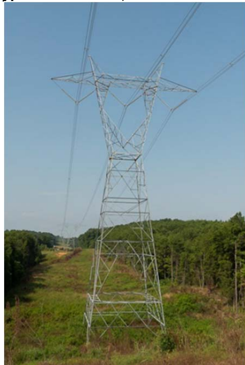
Figure 2-2. Typical 500-kV Laced-Steel Transmission Tower
