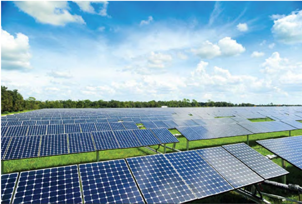
Photograph 3.5-5. Single-axis, tracking photovoltaic system with panels close to maximum tilt as viewed from the east or west.
