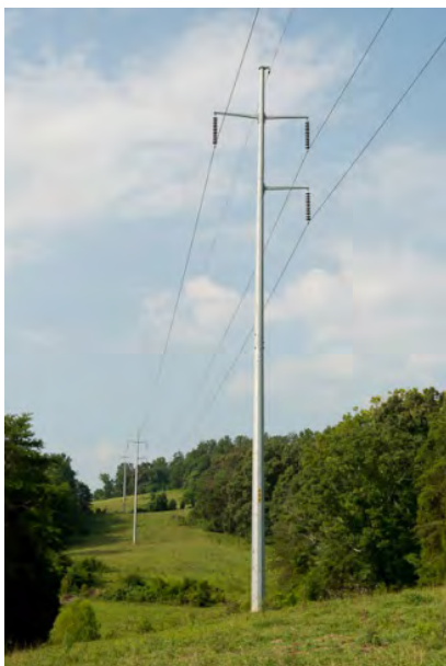
Photo 1. Typical single pole structure
