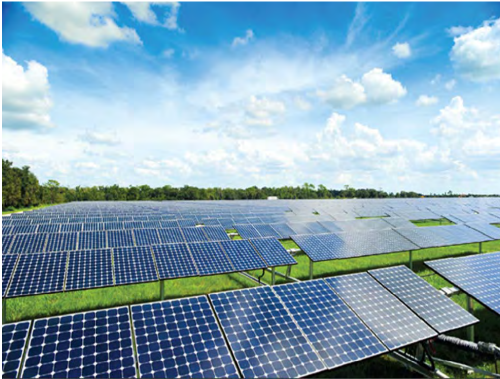
Photo 10. Single-axis, tracking photovoltaic system with panels close to maximum tilt as viewed from the east or west.
