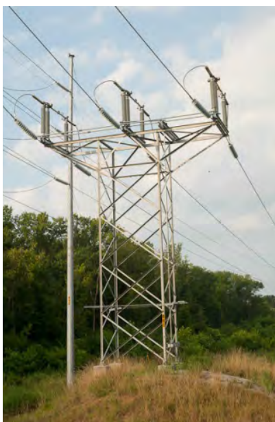
Photo 2. Example of switch structure
