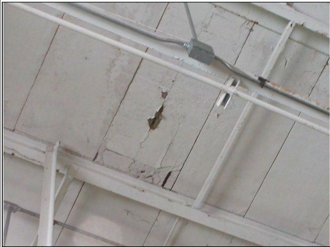
Photograph #: 12 Structurally defective concrete roof deck panel
