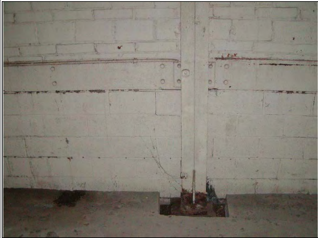
Photograph #: 9 Box-out in topping slab at column
