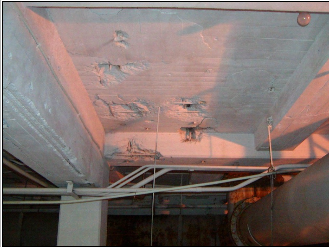
Photograph #: 20 Spalled concrete soffit at basement ceiling
