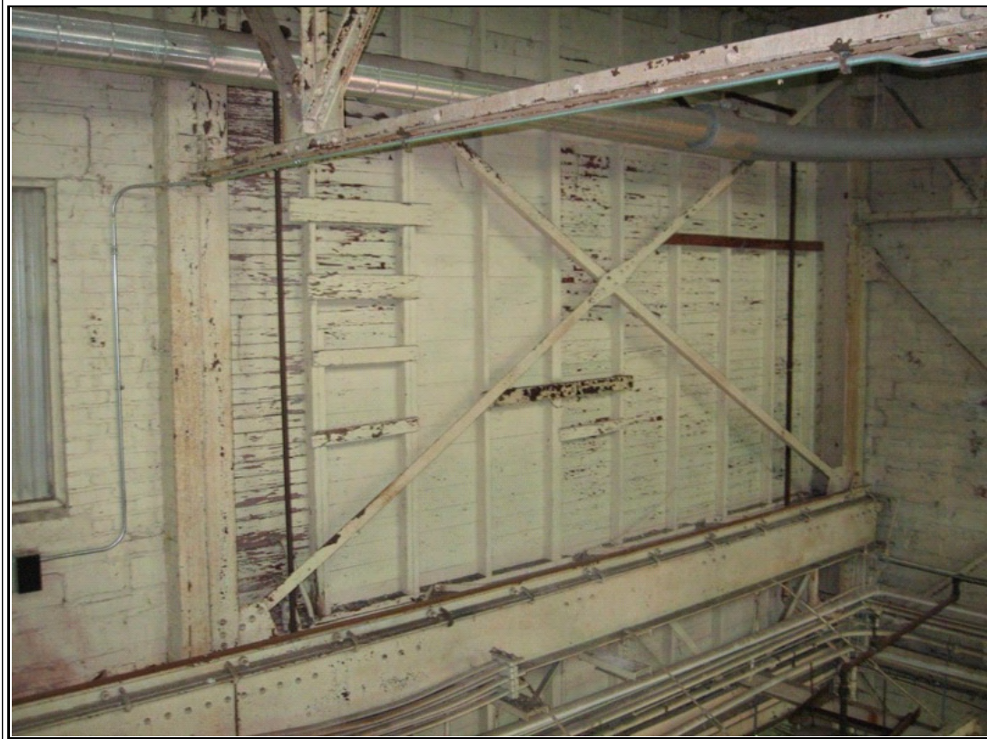
Photograph #: 18 Wood frame interior wall at second floor
