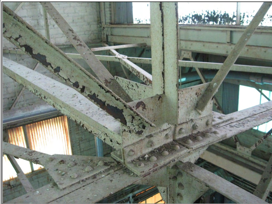
Photograph #: 19 Flaking paint at corroded steel roof framing
