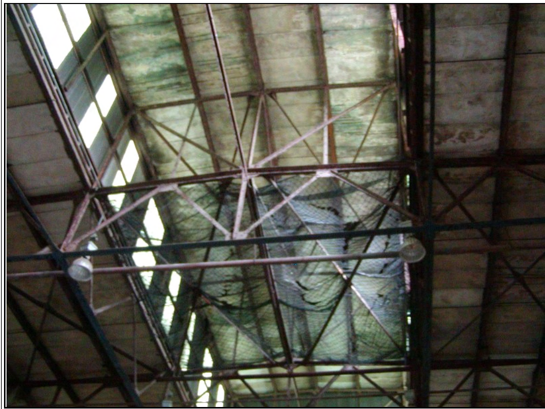
Photograph #: 4 Deteriorated concrete plank roof deck
