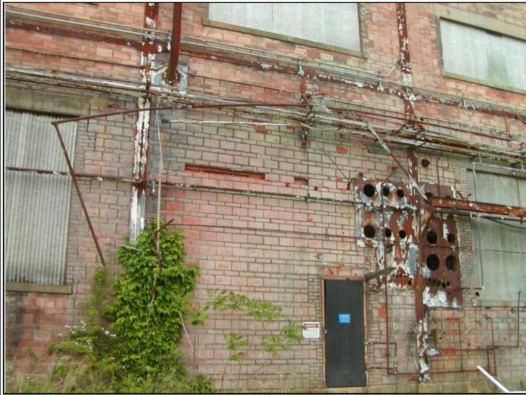
Photograph #: 4 Deteriorated steel and masonry at exterior building - east side
