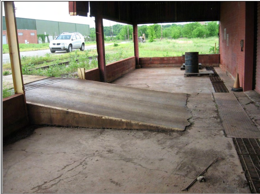
Photograph #: 5 Floor of track shed - note vertical steel framing partially removed adjacent to ramp
