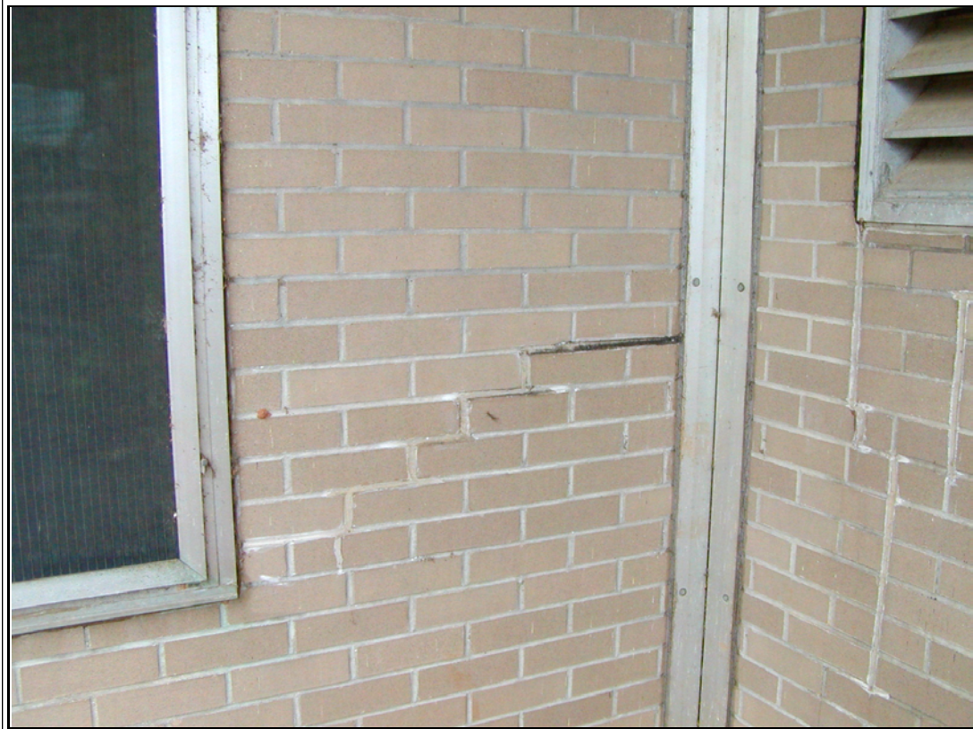
Photograph #: 8 ERC Building - crack in wall near building entrance
