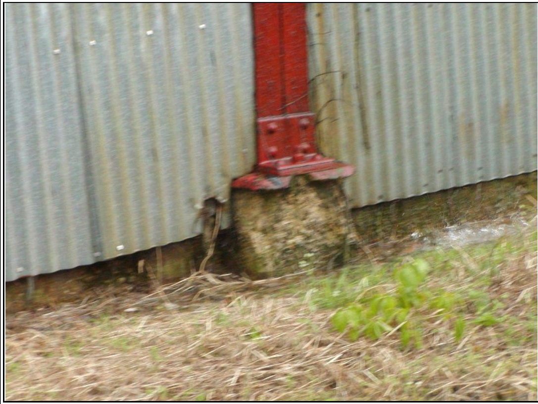
Photograph #: 6 Deteriorated concrete pier at column
