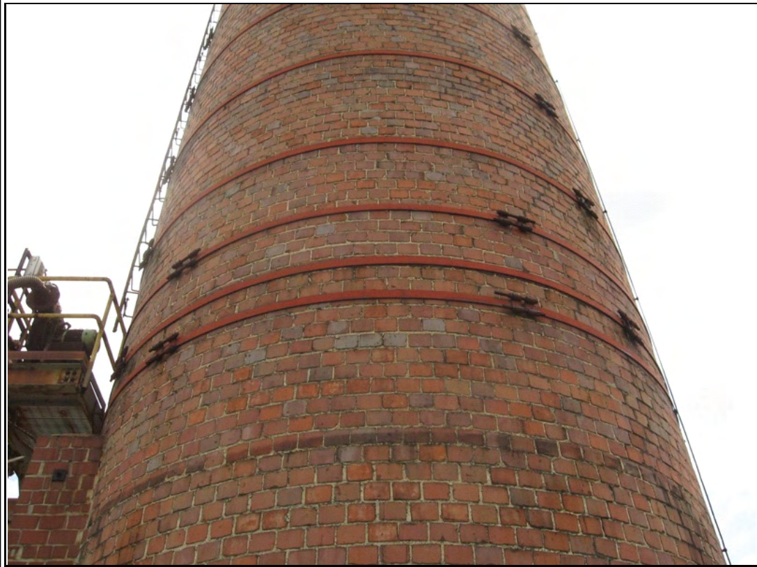
Photograph #: 17 Steel banding at smokestack
