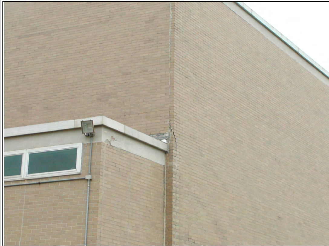
Photograph #: 7 ERC Building - crack at corner of auditorium wall
