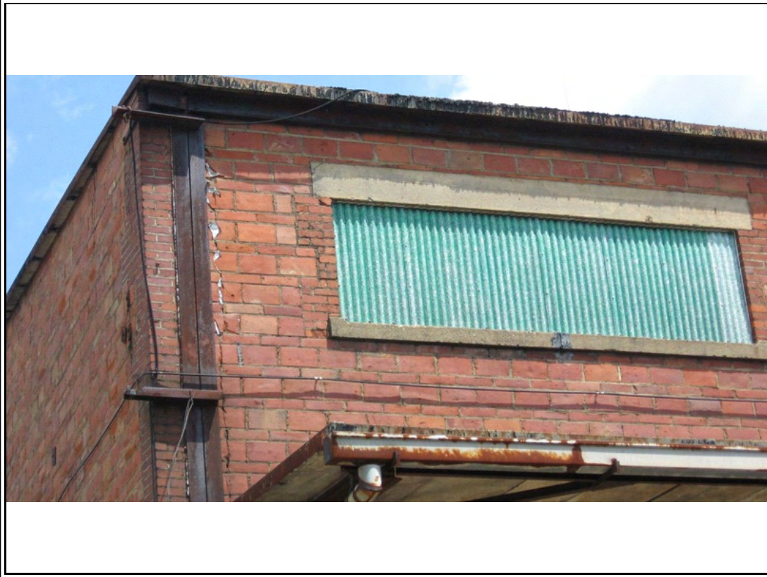
Photograph #: 14 Crack in exterior masonry on south side southwest corner.
