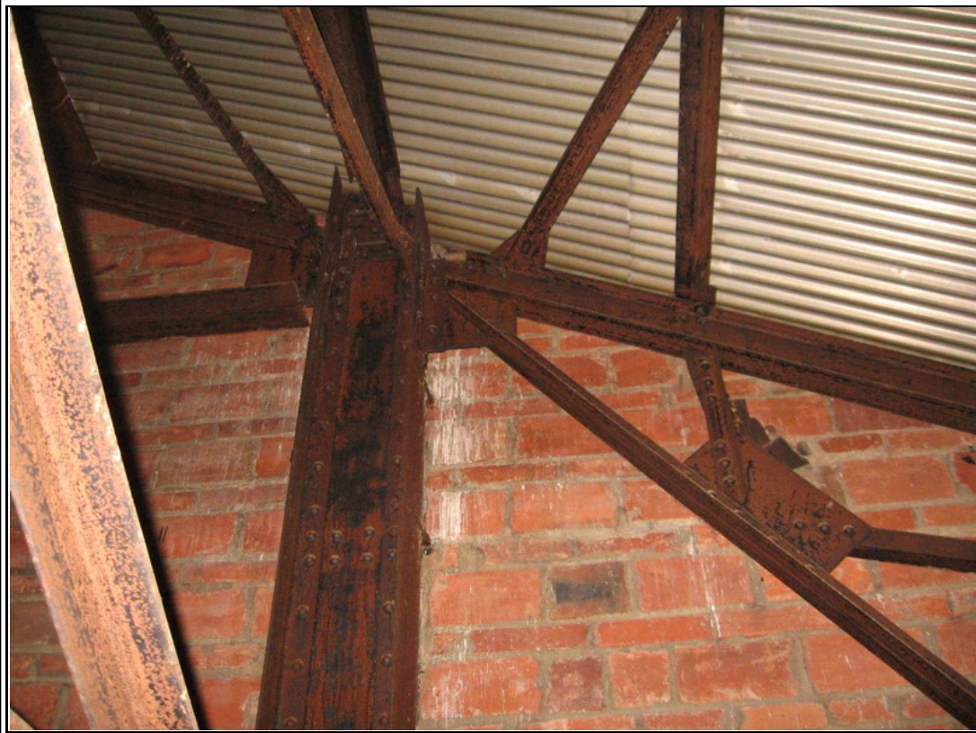
Photograph #: 16 Unpainted corroded steel framing under new metal roof deck
