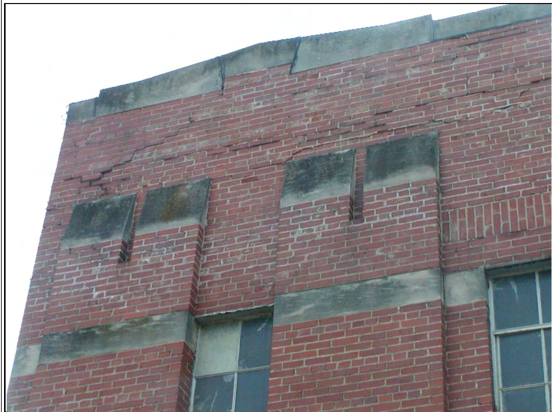
Photograph #: 5 Horizontal and diagonal cracks in masonry west side
