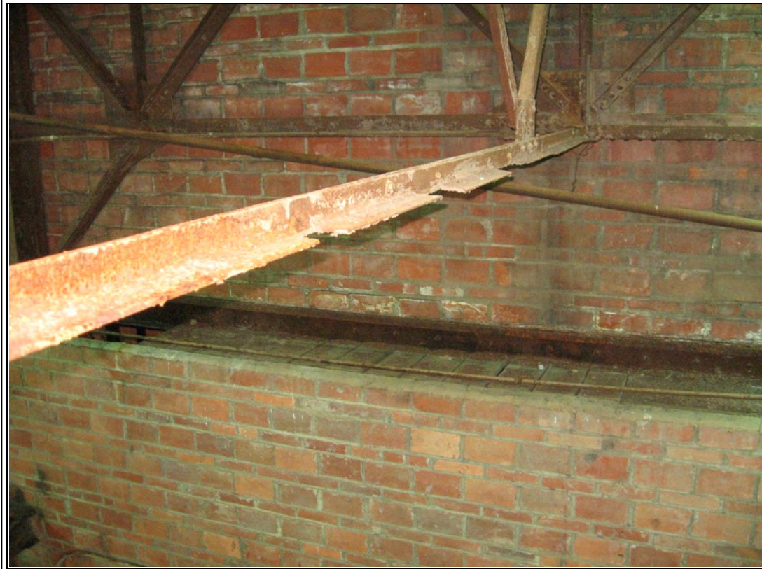
Photograph #: 6 Severely deteriorated steel framing
