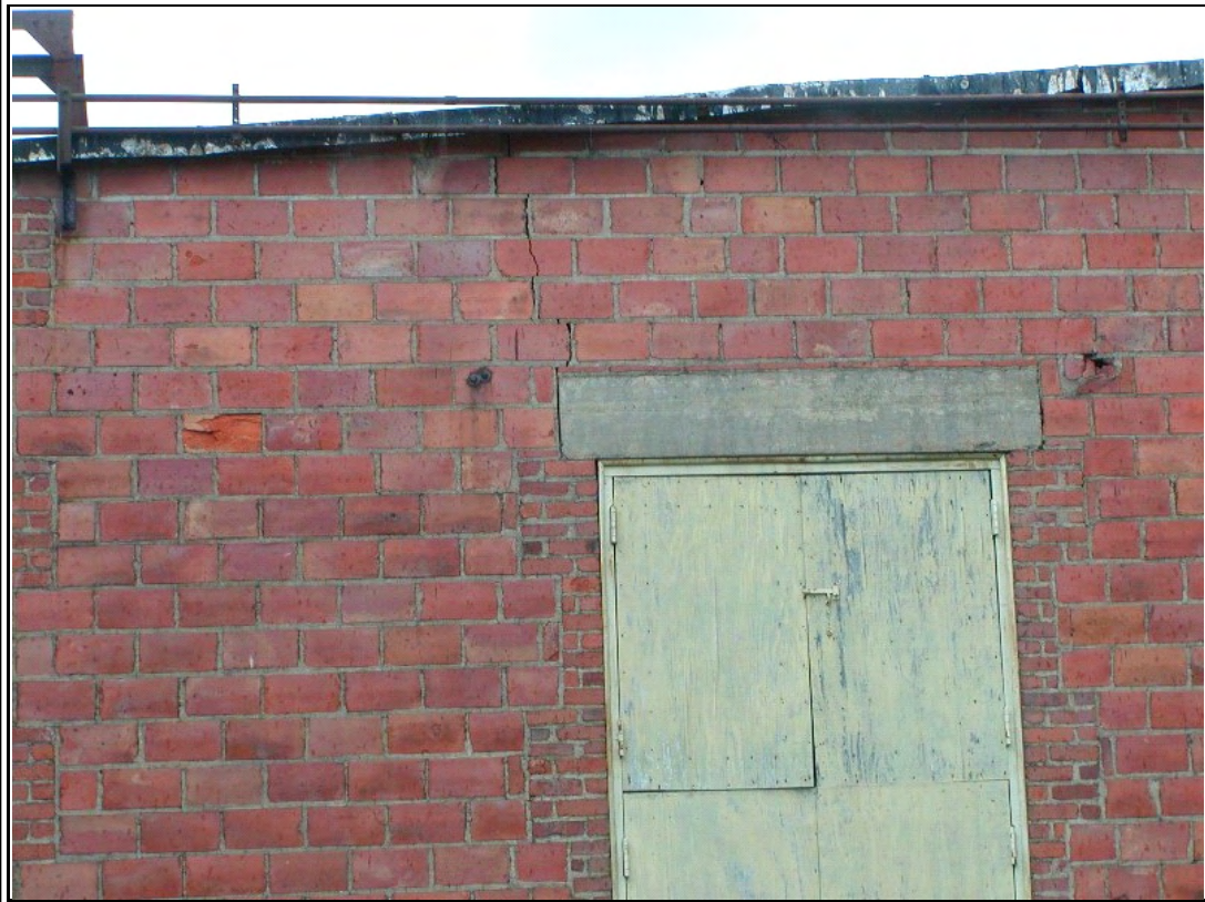
Photograph #: 3 Cracked and spalled masonry at substation
