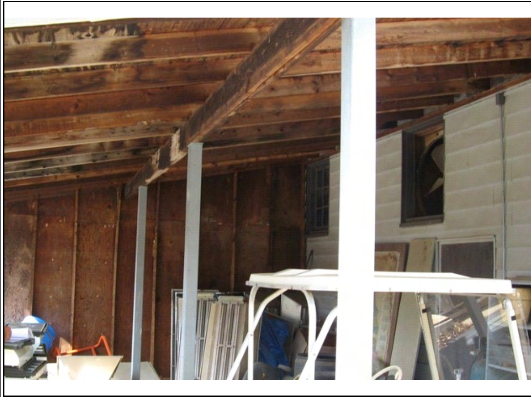
Photograph #: 7 Deteriorated wood canopy at north courtyard.
