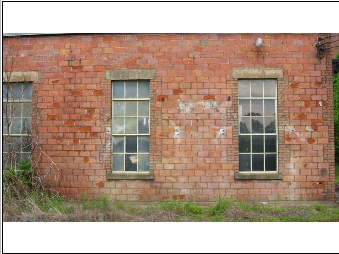
Photograph #: 2 Multiple surface spalls in exterior masonry - east side.
