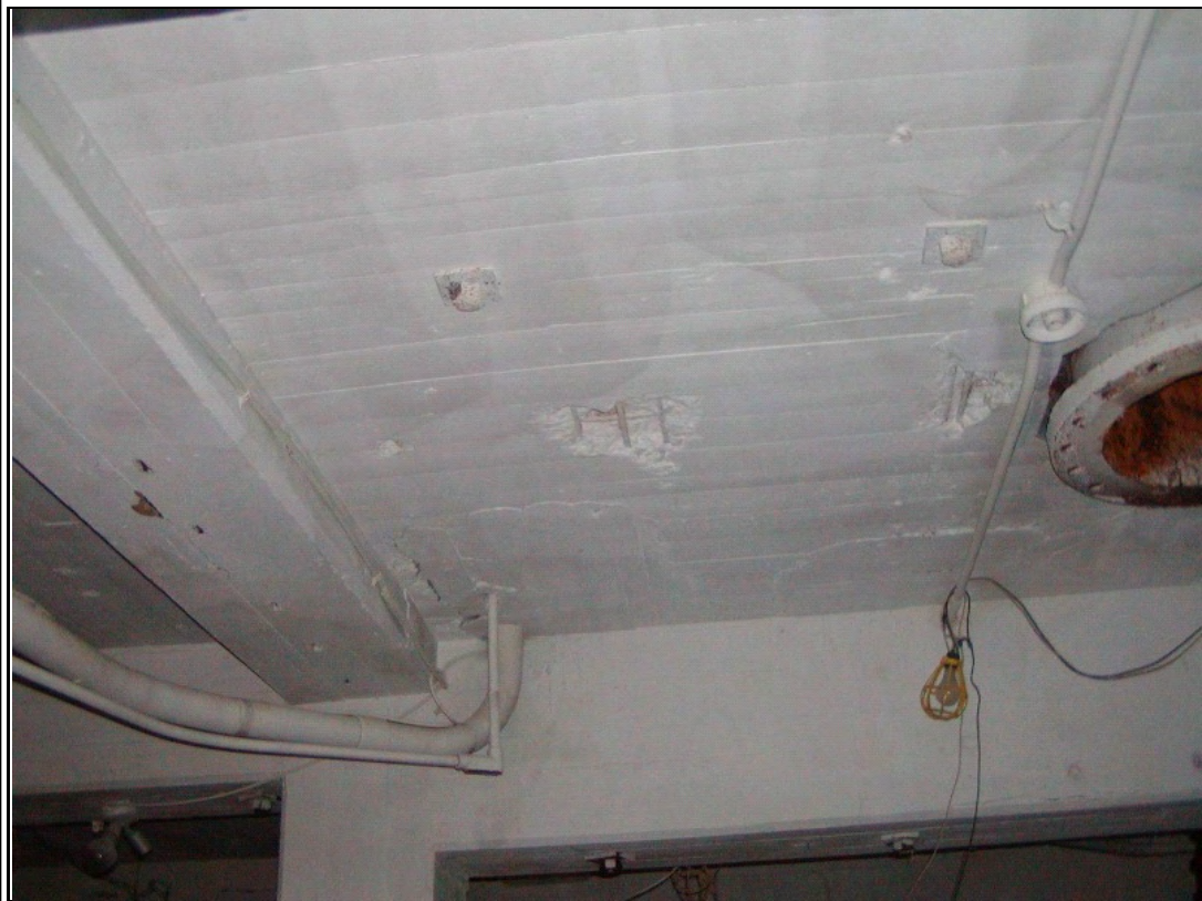
Photograph #: 19 Spalled concrete soffit at basement ceiling
