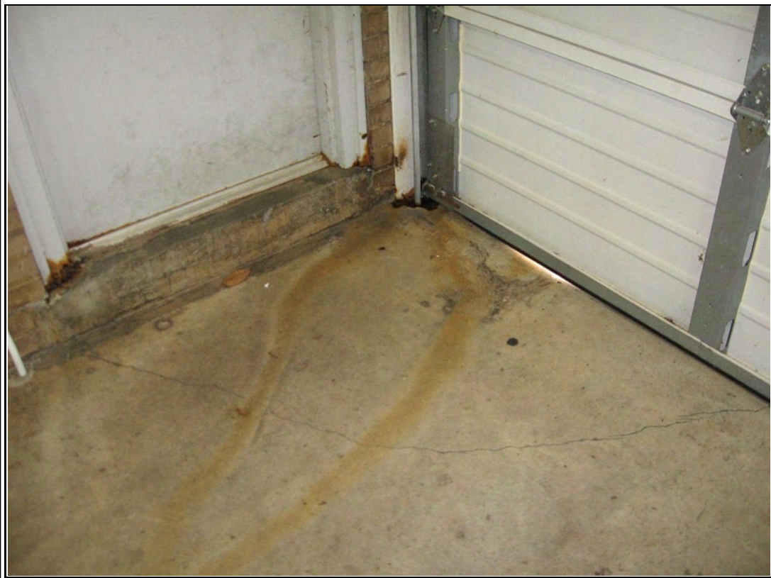
Photograph #: 20 Service Building - crack in slab at vehicle storage area
