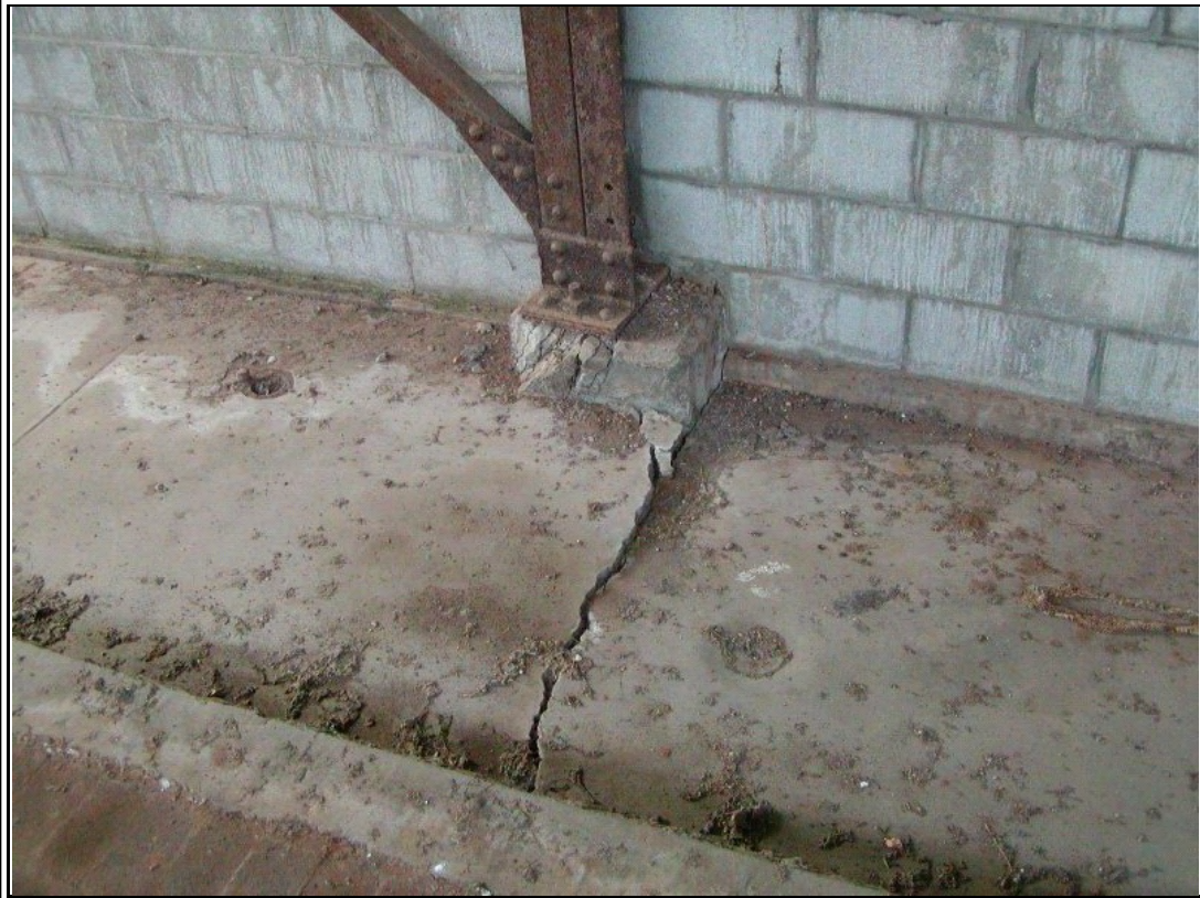
Photograph #: 7 Deteriorated concrete pier and slab at column
