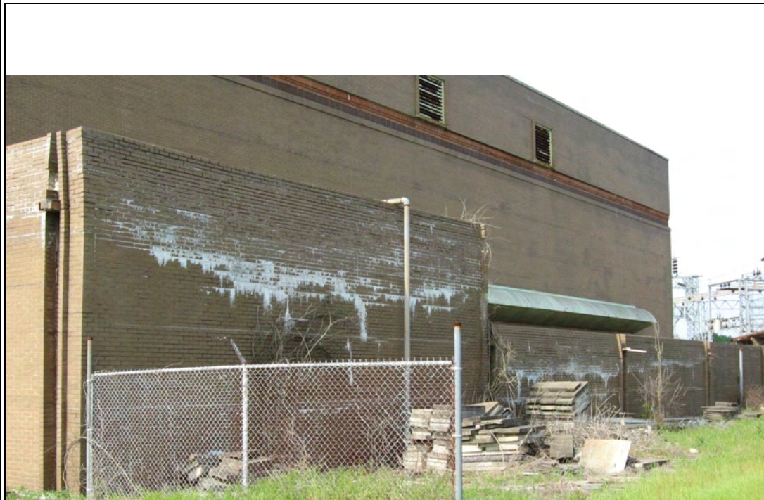
Photograph #: 5 Structurally unstable masonry parapet at north extension.
