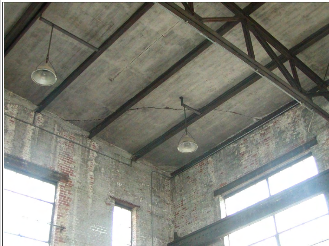
Photograph #: 13 Crack in concrete roof deck at northeast corner
