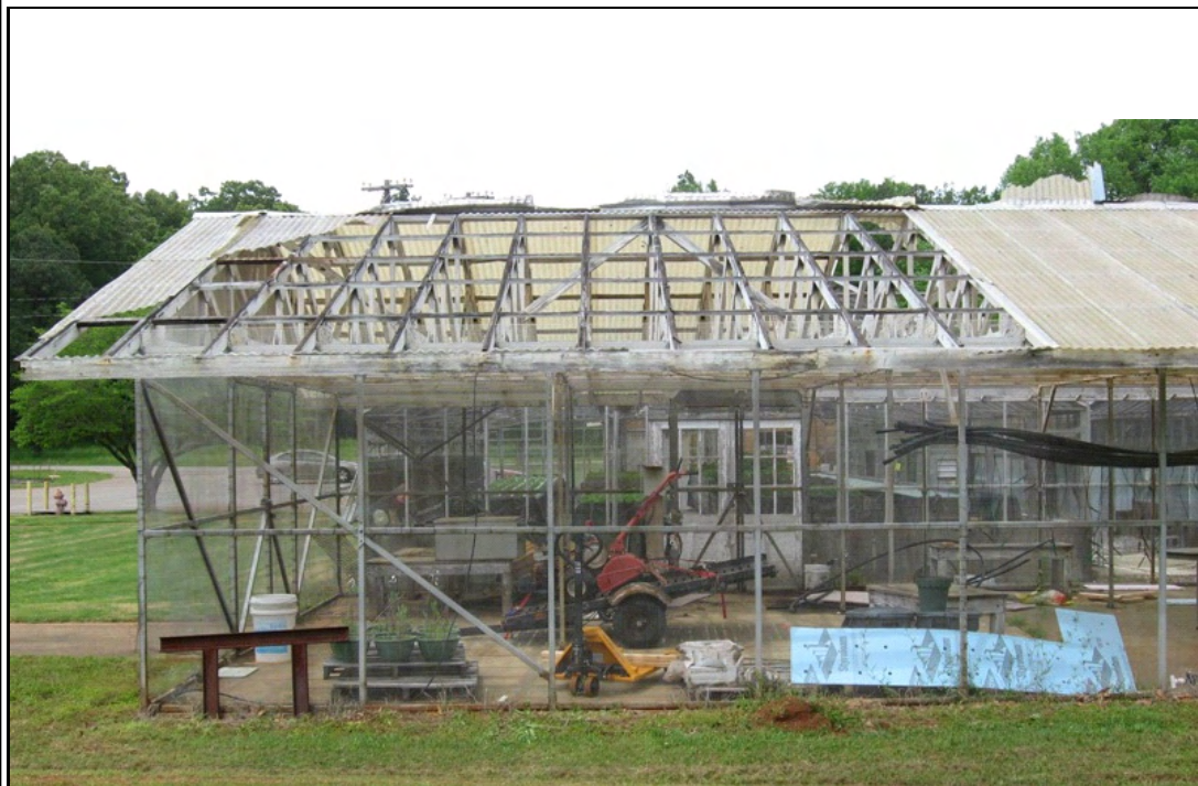
Photograph #: 18 Damaged roof covering at screened porch
