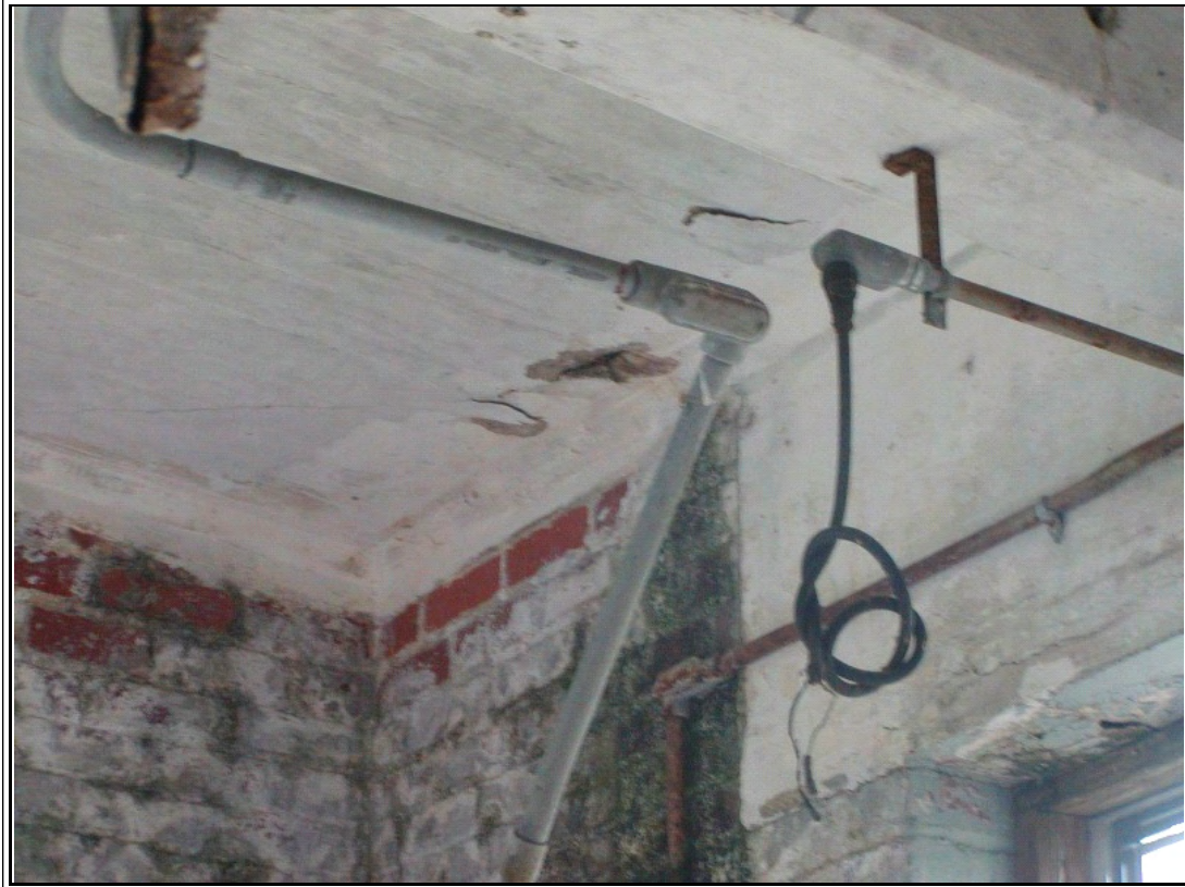
Photograph #: 14 Spalls in concrete at underside of upper floor
