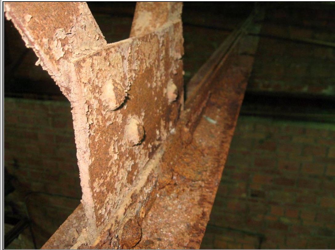
Photograph #: 5 Severely corroded steel framing
