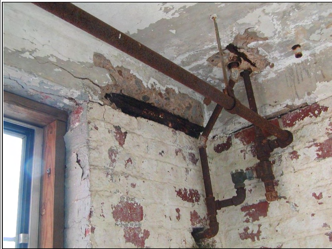
Photograph #: 12 Spalled concrete at underside of upper floor
