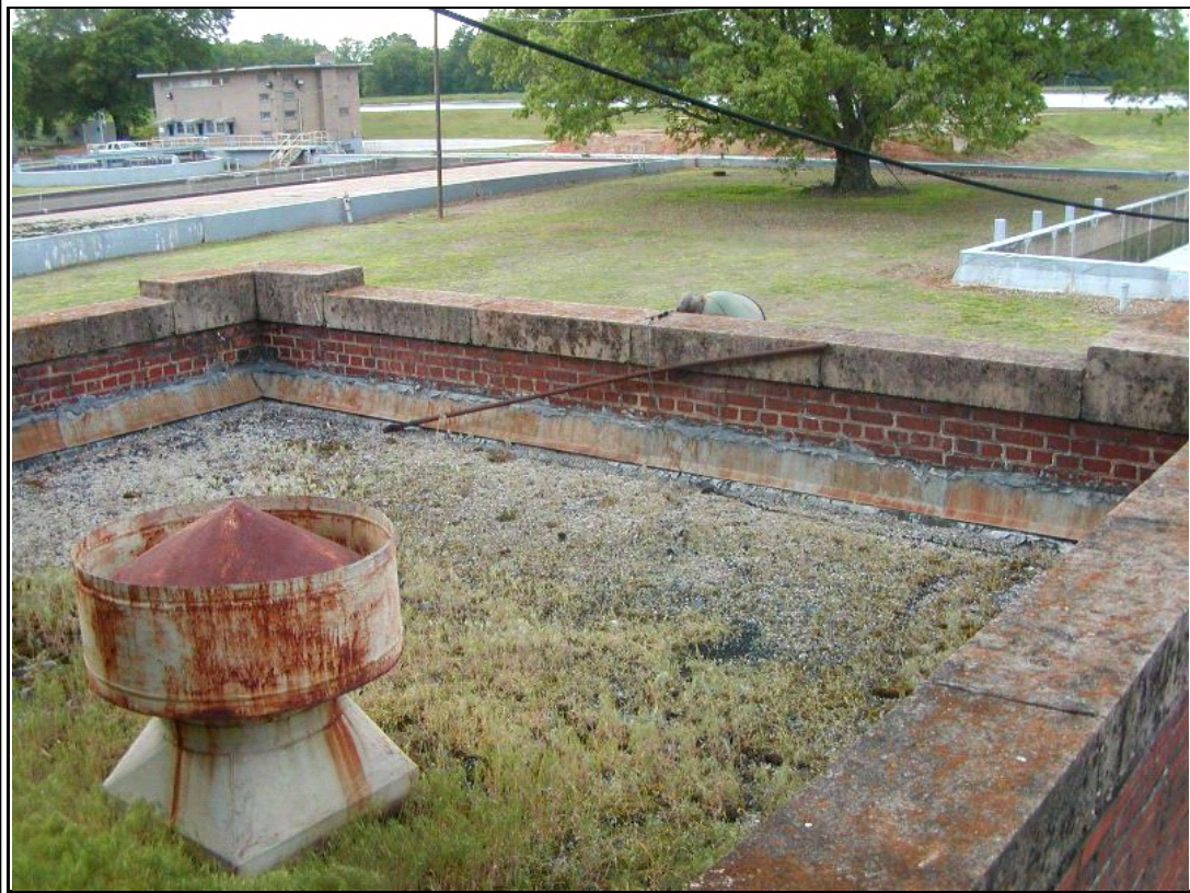
Photograph #: 7 Poor drainage at low roof
