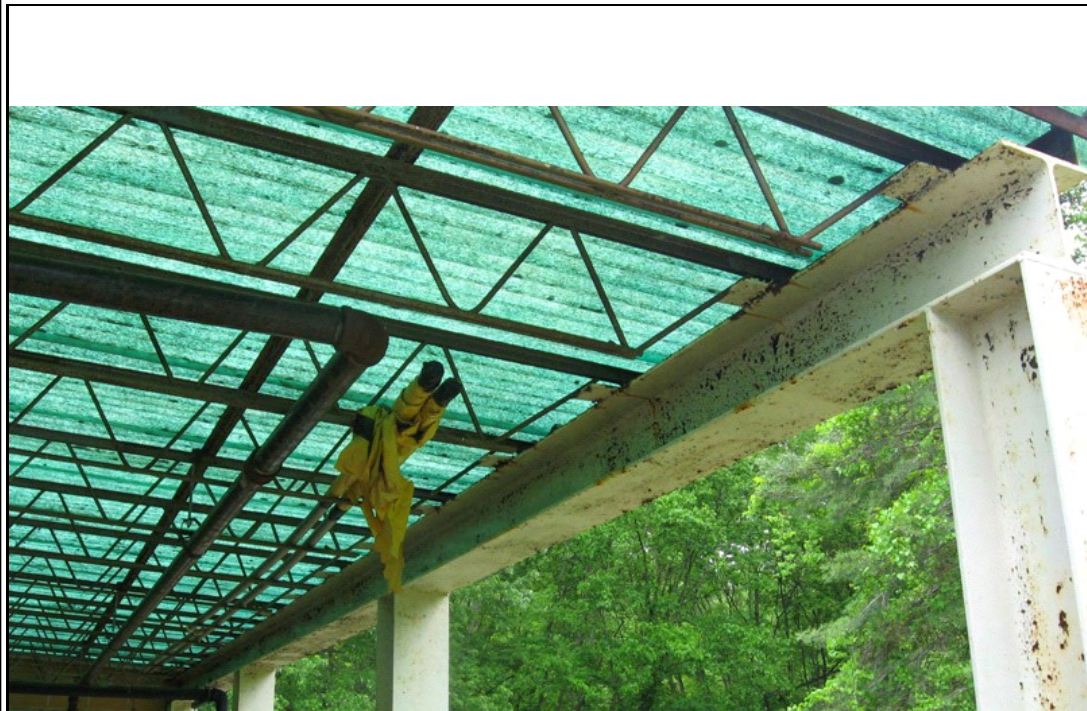
Photograph #: 4 Mildly to moderately corroded steel at open covered storage area
