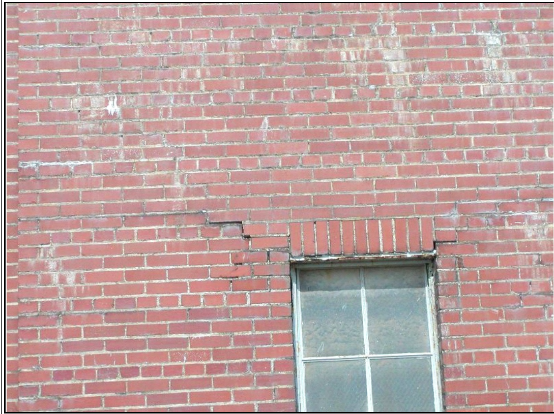
Photograph #: 6 Cracked masonry partially dislodged at lintel
