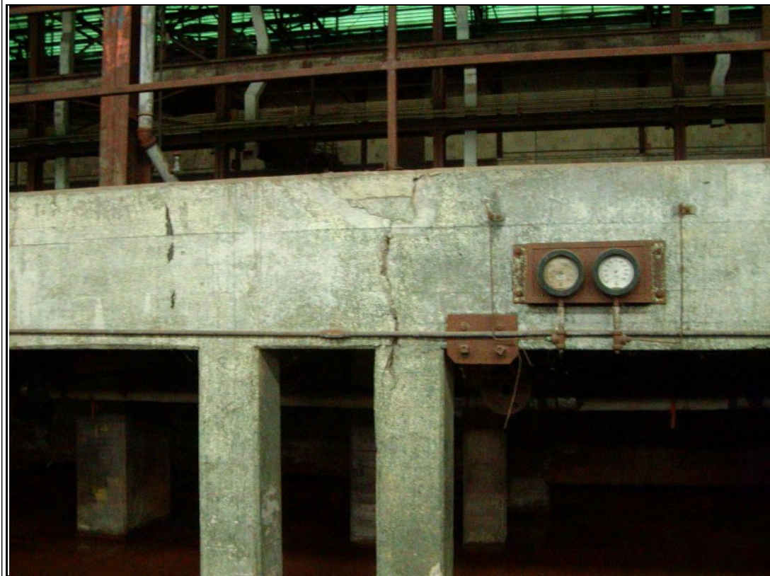
Photograph #: 17 Cracks at edge of elevated slab above basement
