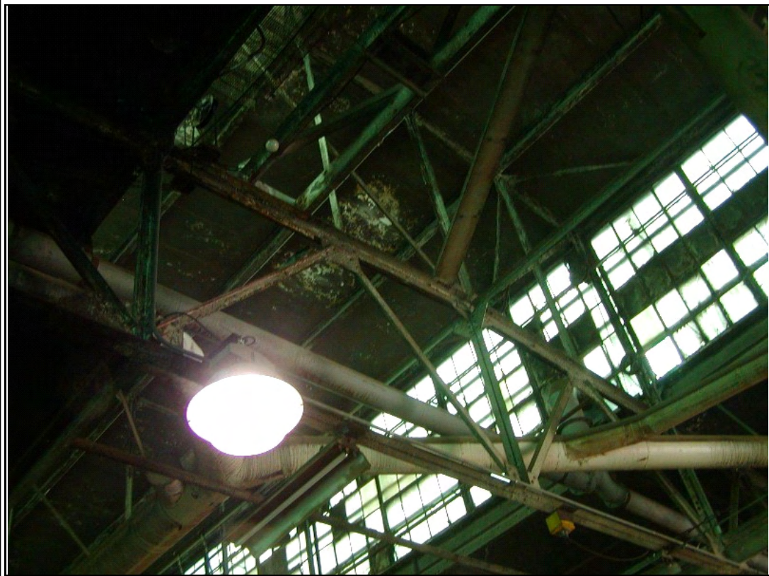
Photograph #: 20 Deteriorated concrete plank roof deck at monitor
