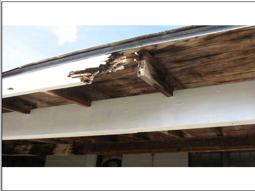
Photograph #: 6 Deteriorated wood canopy at north courtyard.
