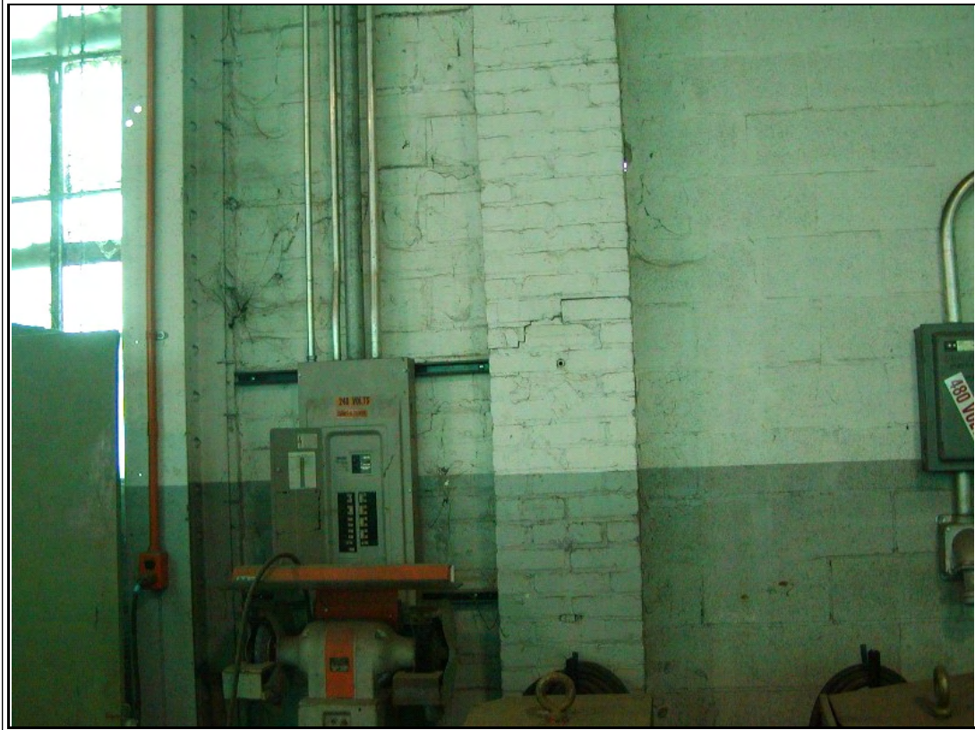
Photograph #: 10 Horizontal crack in brick pier
