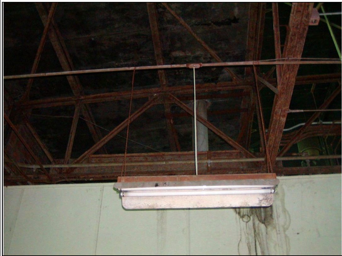
Photograph #: 10 Corroded steel framing and deteriorated roof deck
