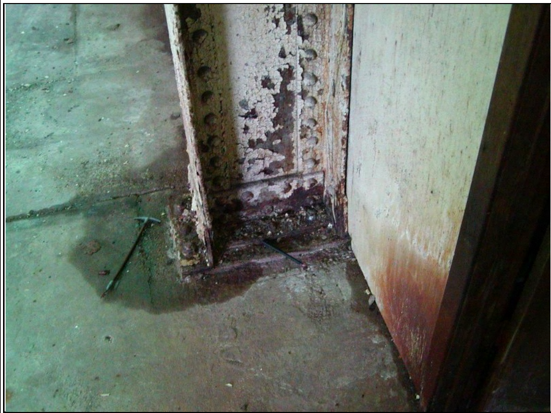
Photograph #: 13 Corroded steel column north side of main building
