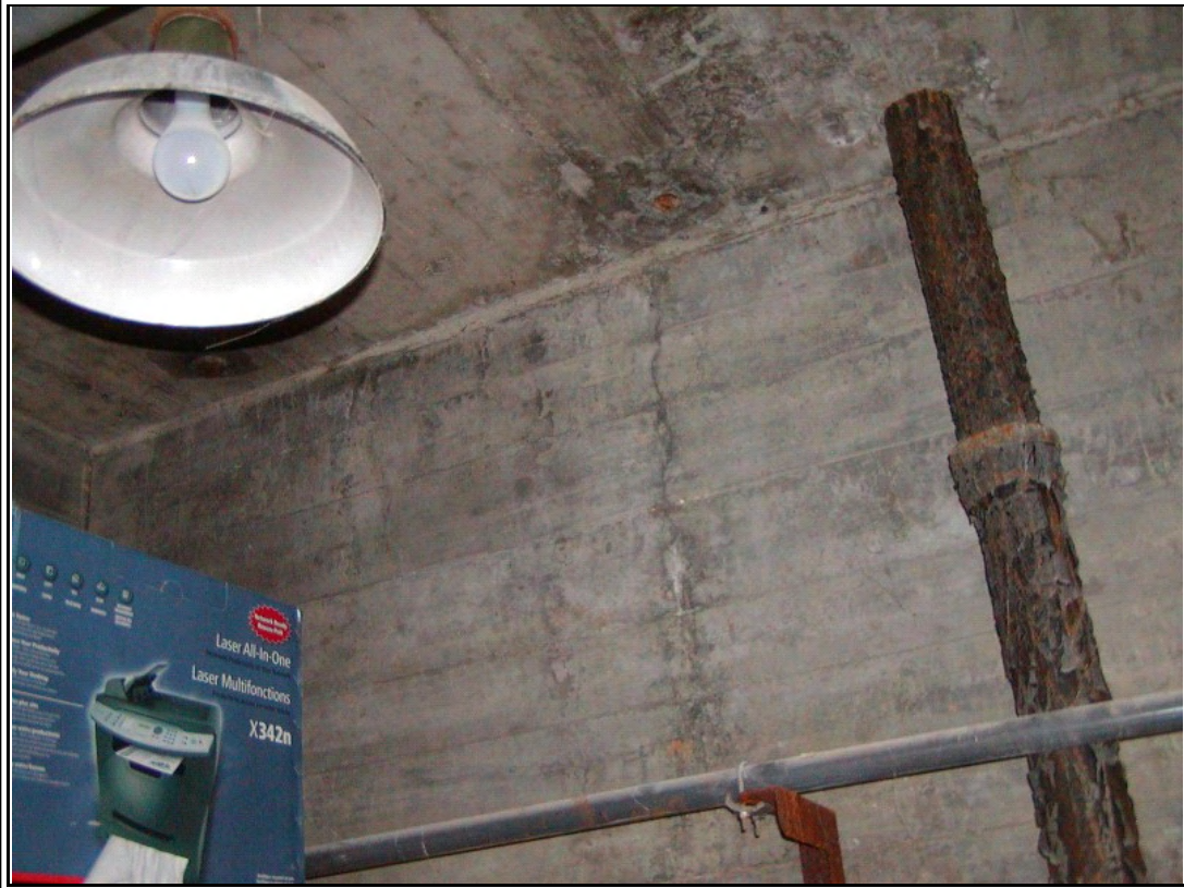
Photograph #: 8 Evidence of water intrusion at basement wall and ceiling
