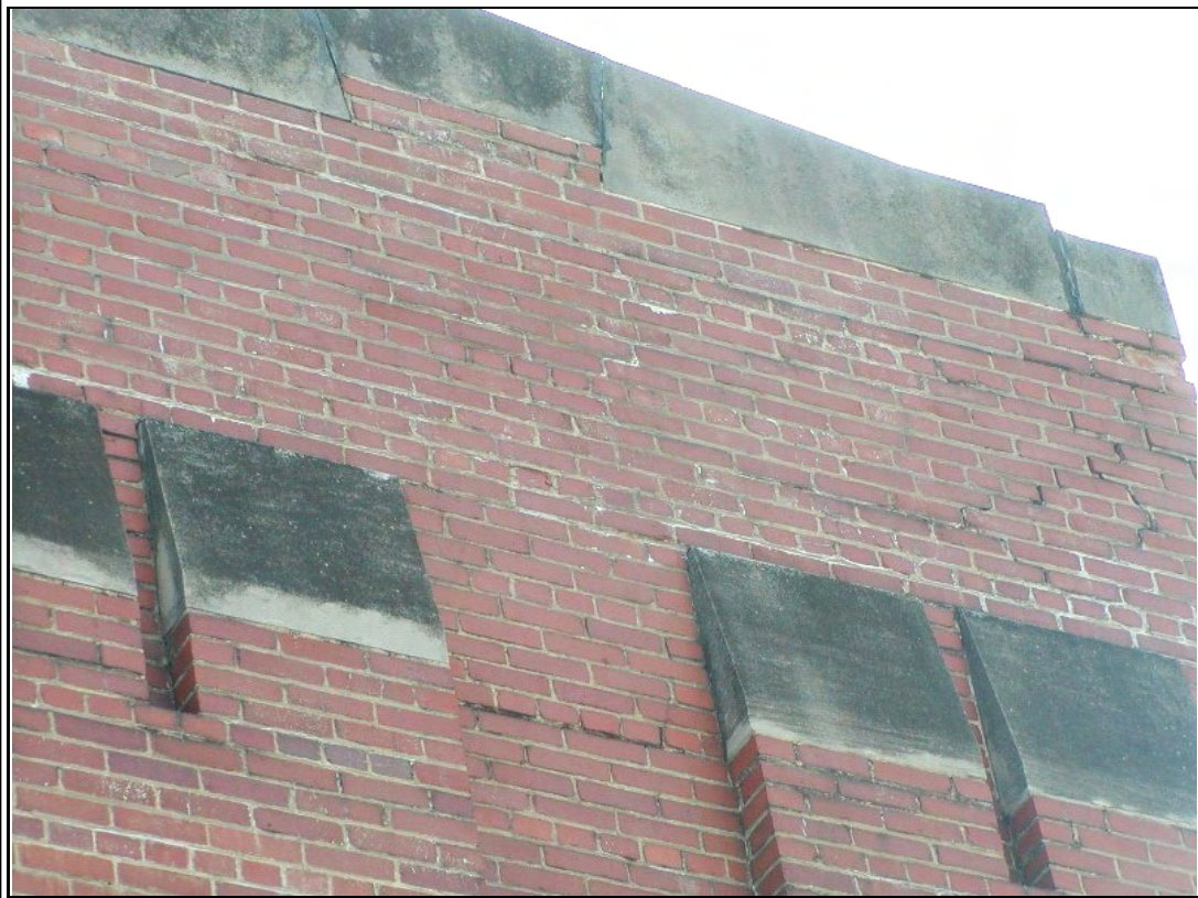
Photograph #: 8 Cracks in masonry at south end of west wall
