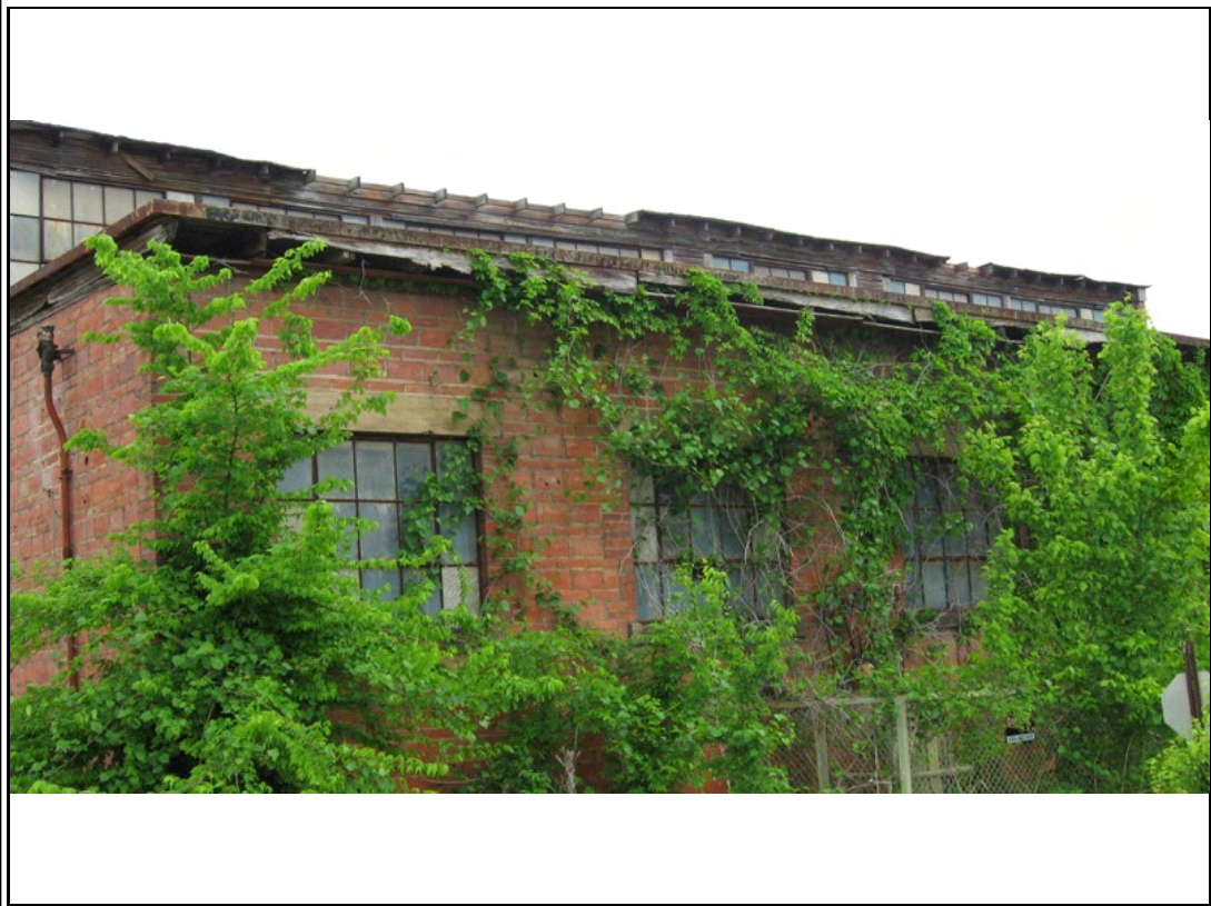
Photograph #: 4 View of decayed wood roof structure on south side.
