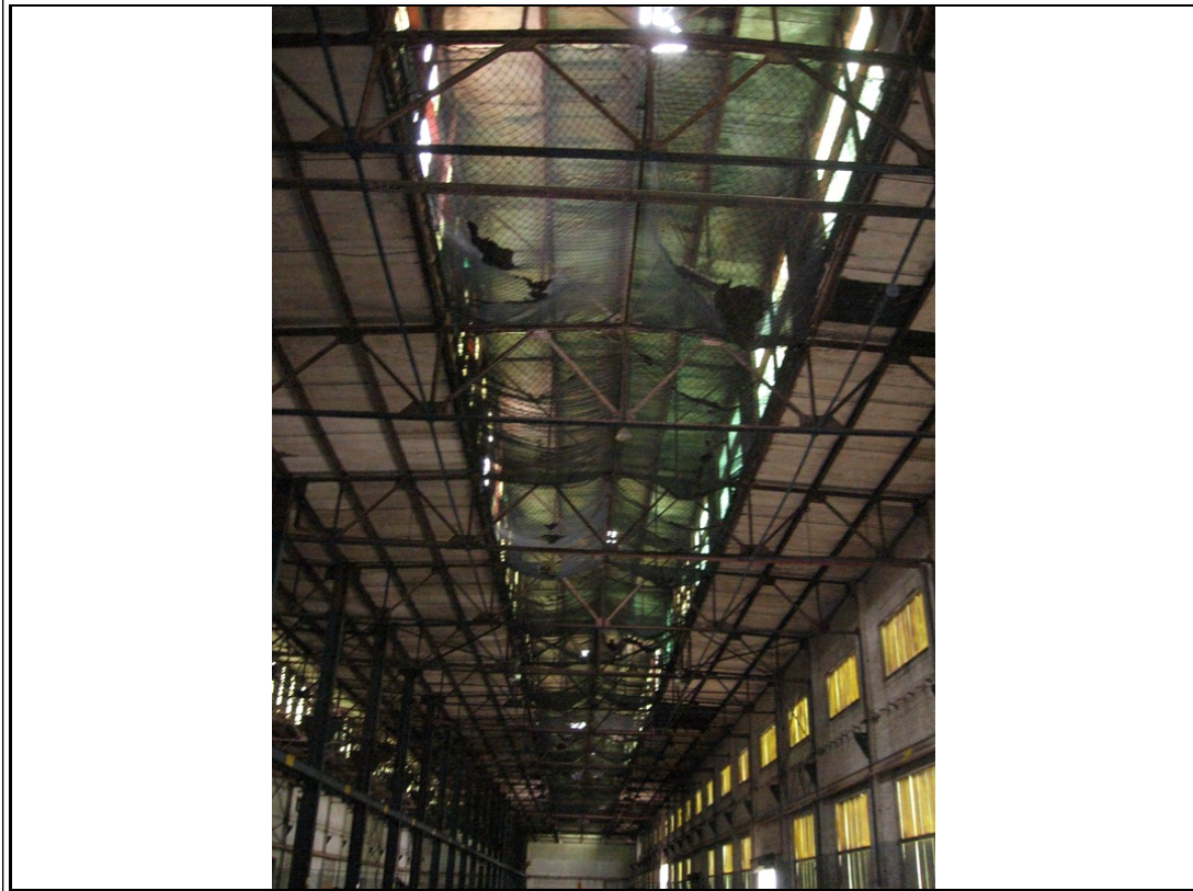
Photograph #: 12 Holes in deteriorated concrete plank roof deck
