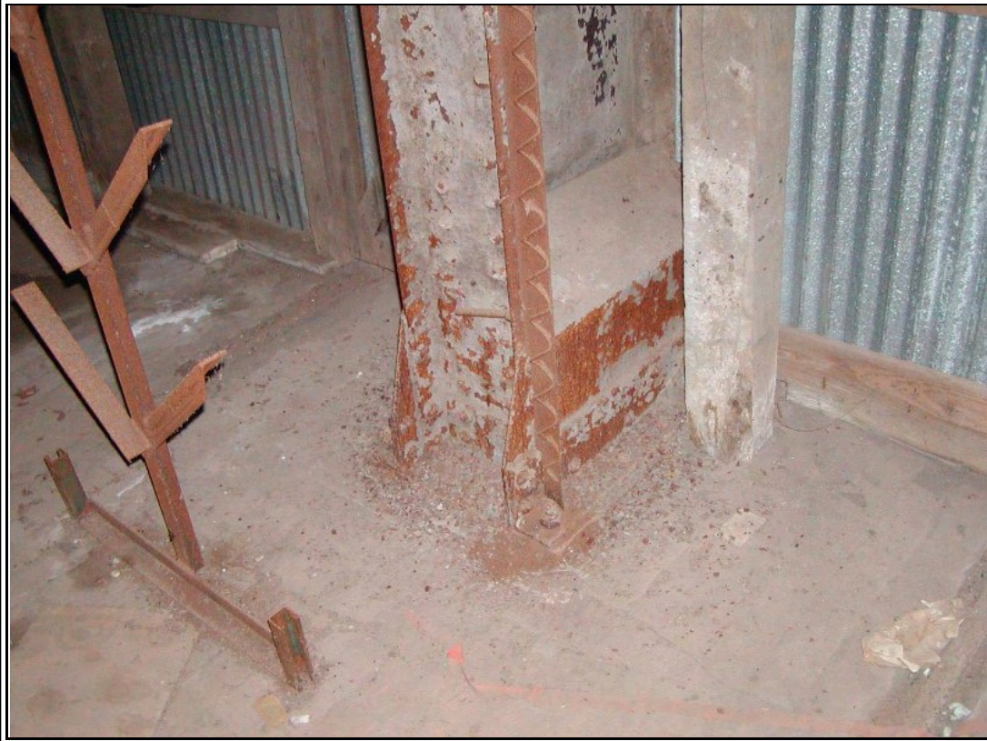
Photograph #: 10 Severely corroded steel column
