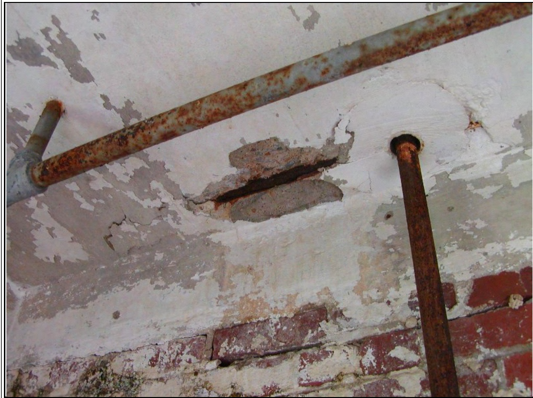
Photograph #: 13 Spall in concrete at underside of upper floor
