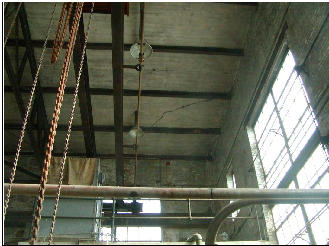
Photograph #: 15 Crack in concrete roof deck at southeast corner
