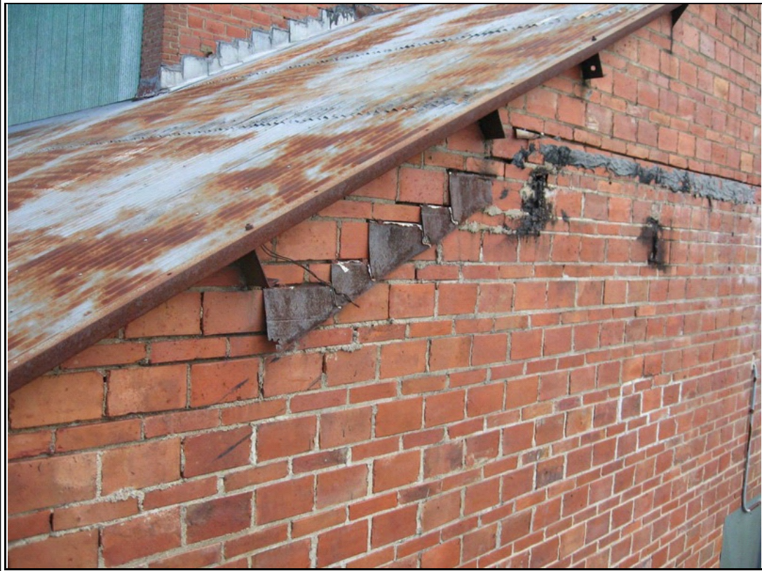
Photograph #: 6 Detail view of where track shed roof was attached to building
