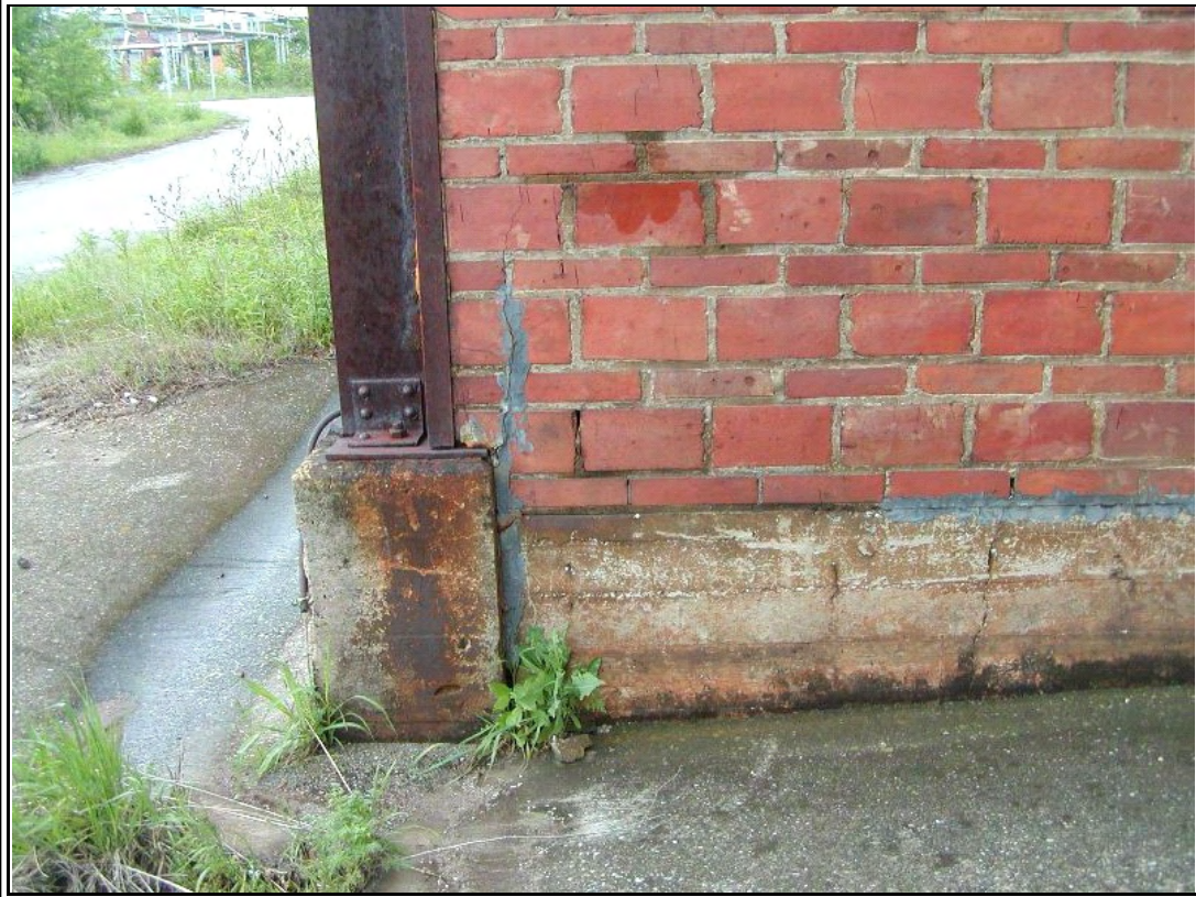
Photograph #: 14 Cracks in masonry and foundation wall at southwest corner
