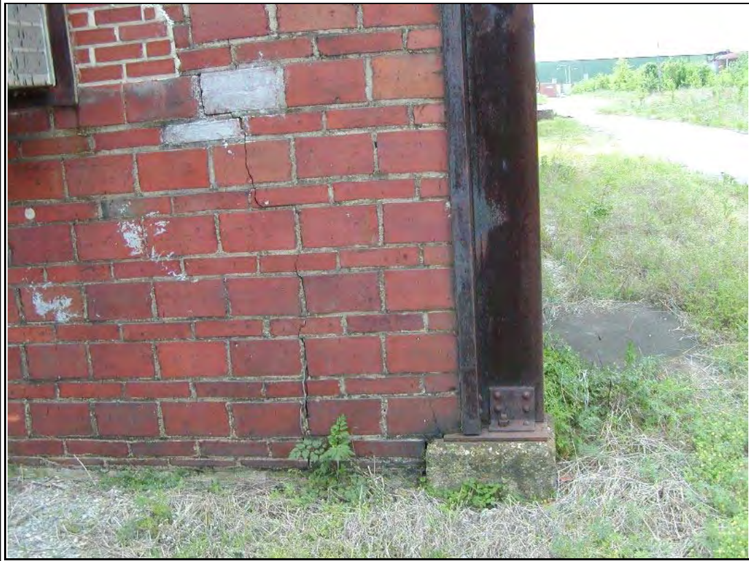
Photograph #: 4 Crack in wall at northwest corner
