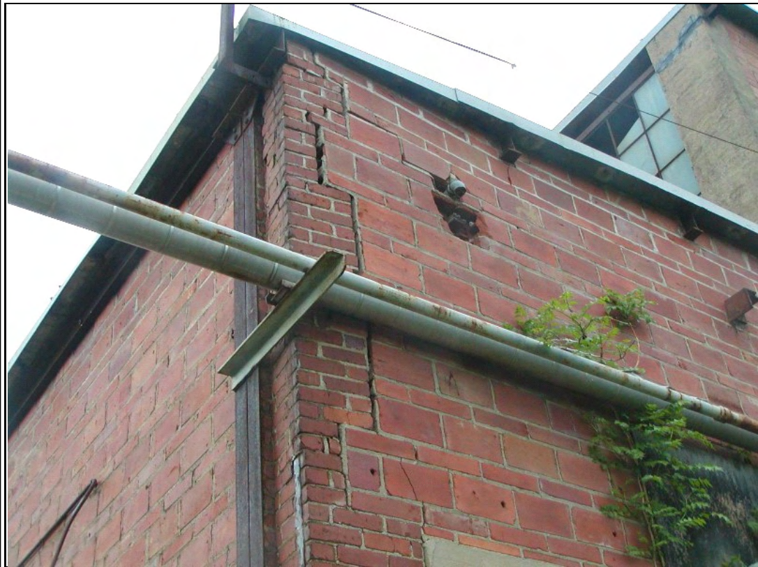
Photograph #: 3 Cracked and partially dislodged masonry at southeast corner
