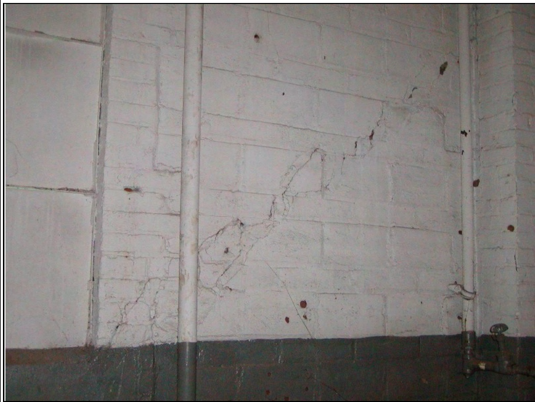
Photograph #: 22 Diagonal crack in masonry at west wall
