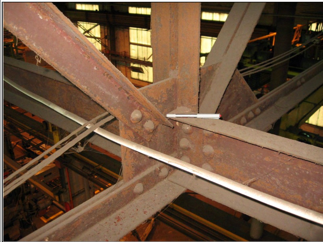
Photograph #: 17 Moderately corroded roof framing
