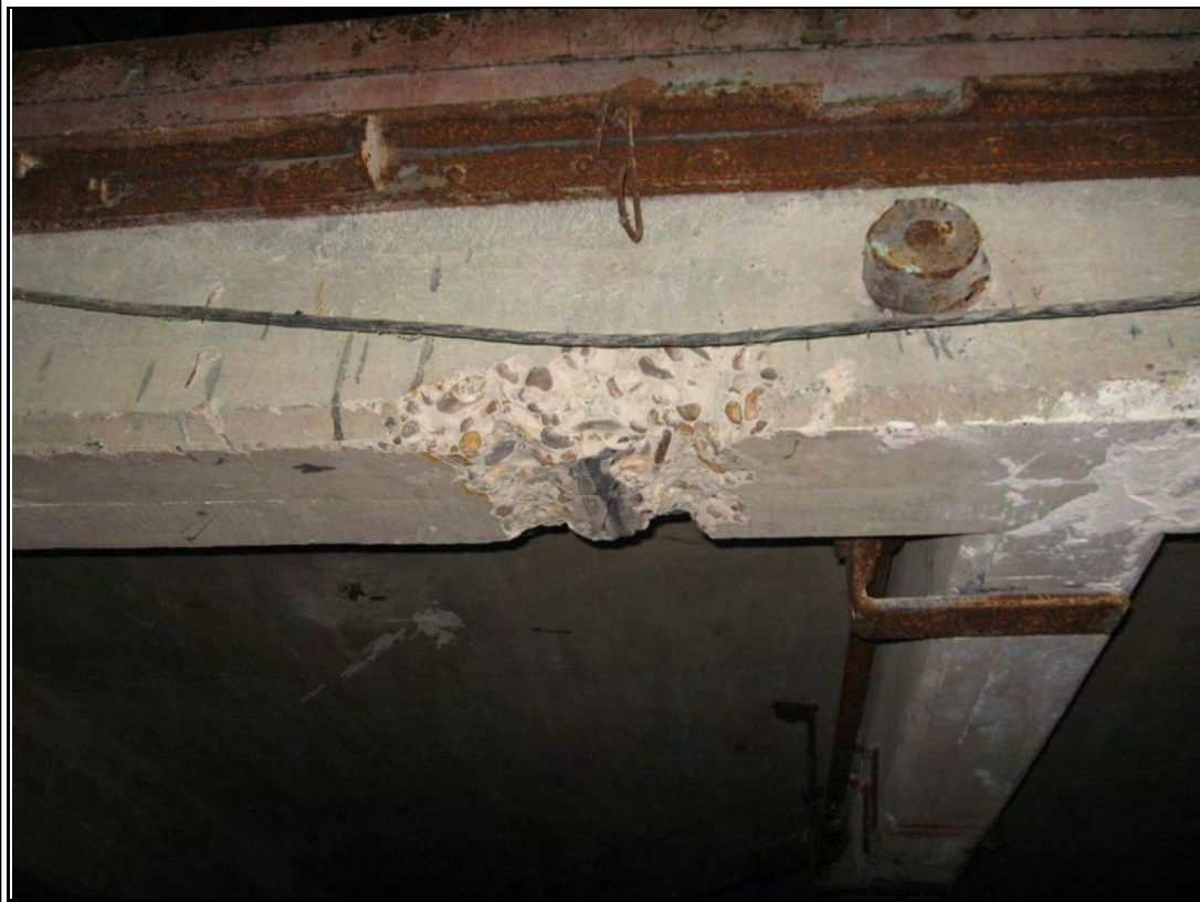
Photograph #: 25 Damaged mezzanine concrete beam
