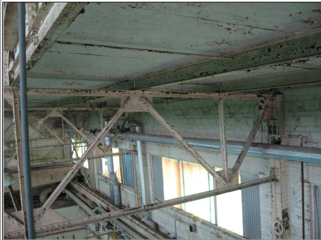
Photograph #: 17 View of main roof framing and roof deck
