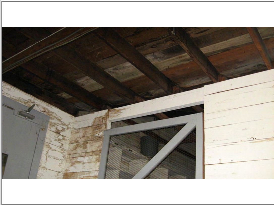
Photograph #: 8 Deteriorated wood framing and planking at central structure near east wing
