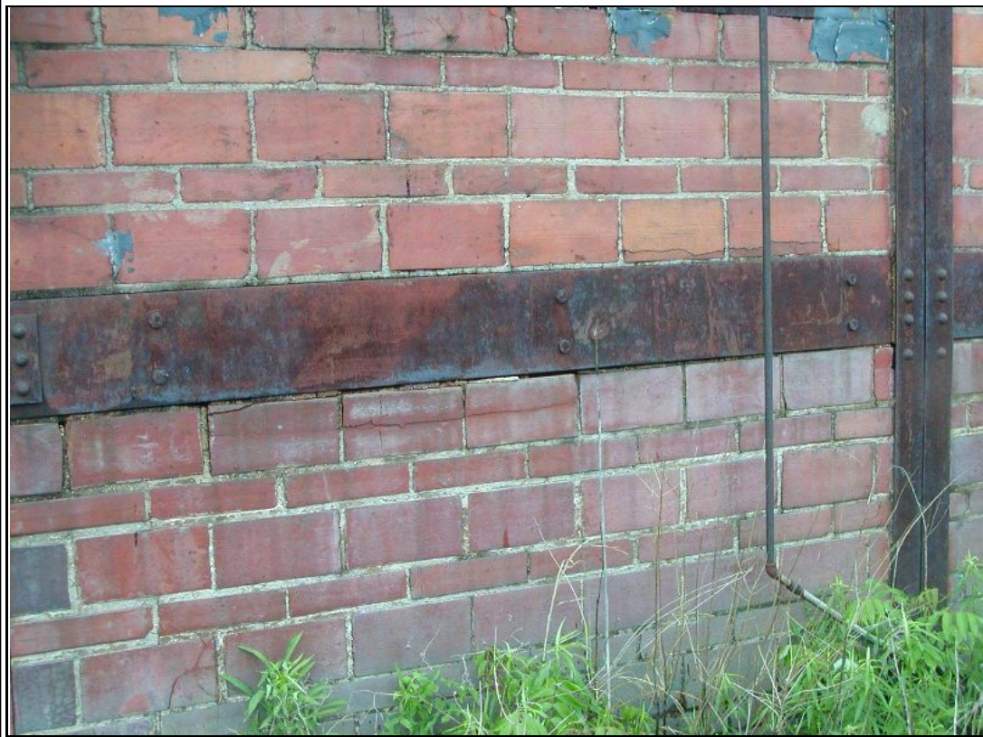
Photograph #: 4 Corroded exterior steel framing at south wall
