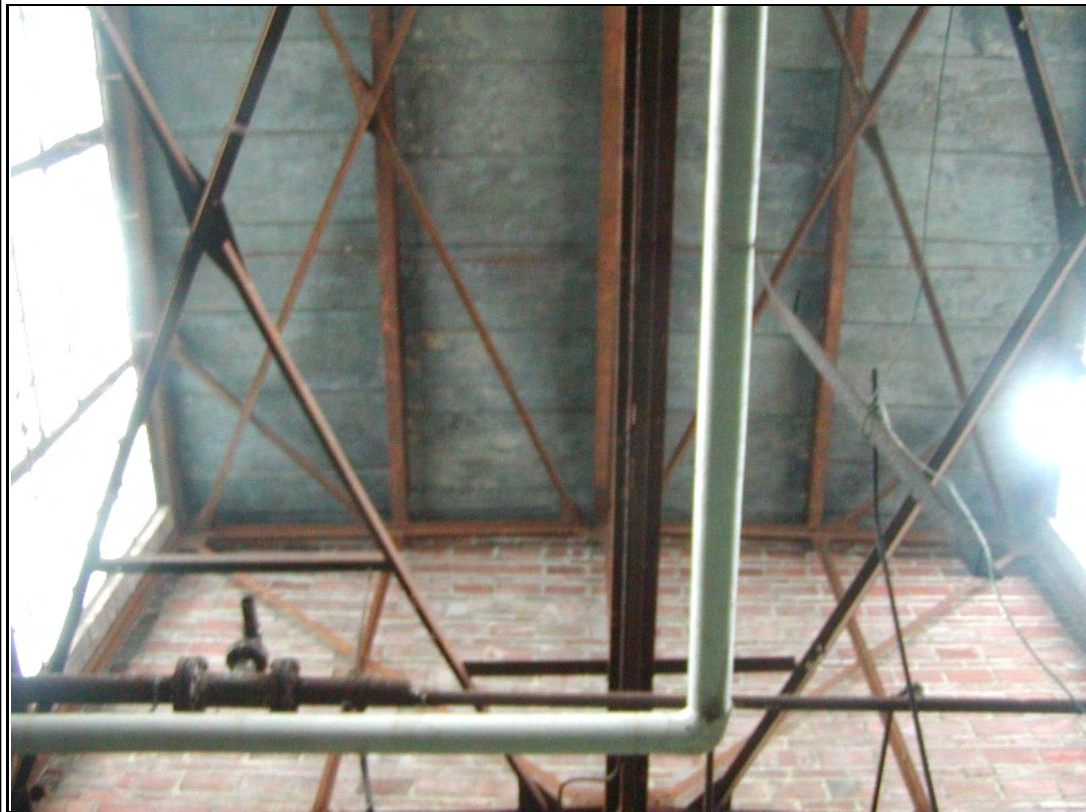
Photograph #: 9 Monitor roof with corroded steel framing and surface deterioration on concrete plank roof deck
