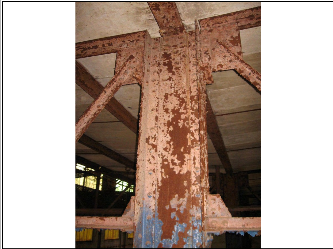
Photograph #: 8 Severely corroded steel framing
