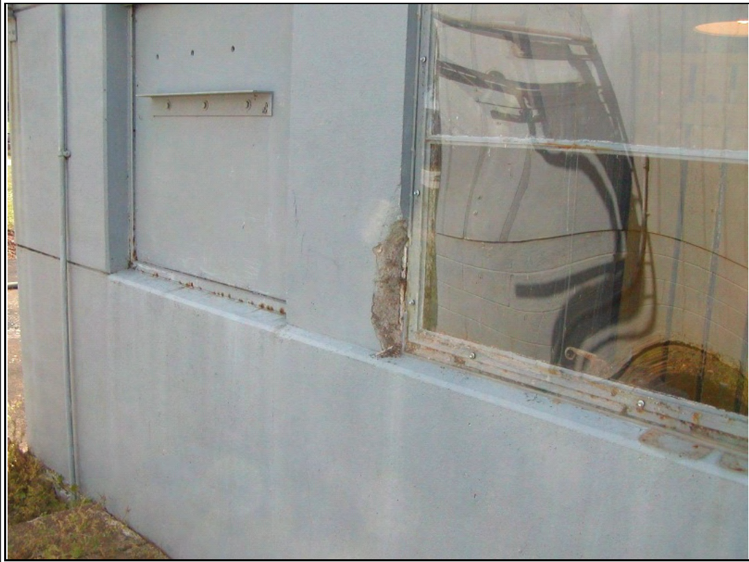
Photograph #: 8 Minor spall at window on east side
