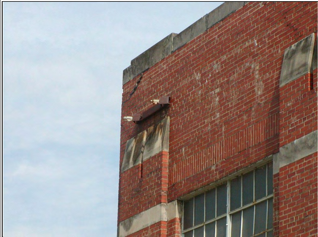
Photograph #: 7 Cracked masonry partially dislodged at west end of south wall
