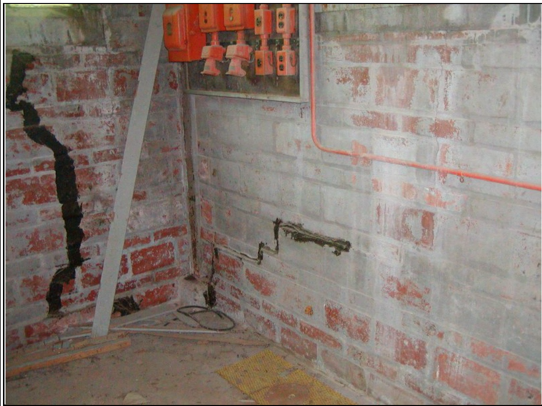
Photograph #: 13 Previously repaired cracks in wall at northwest corner
