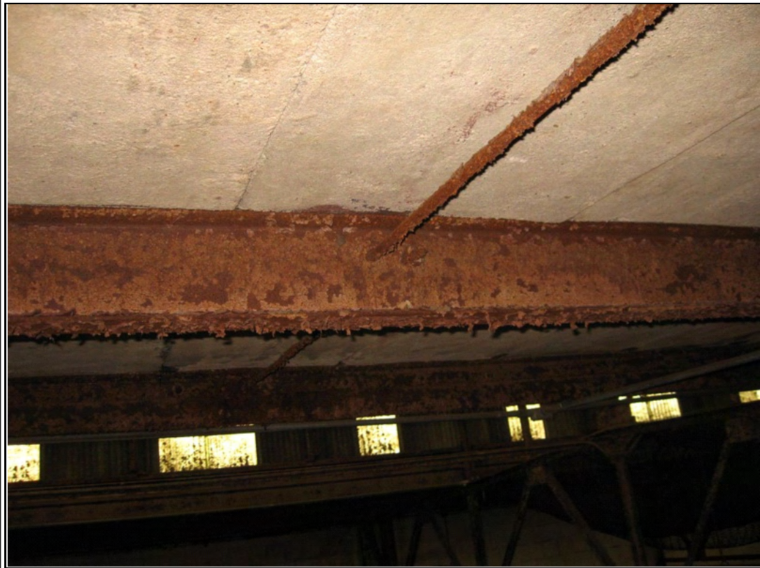
Photograph #: 9 Severely corroded steel framing
