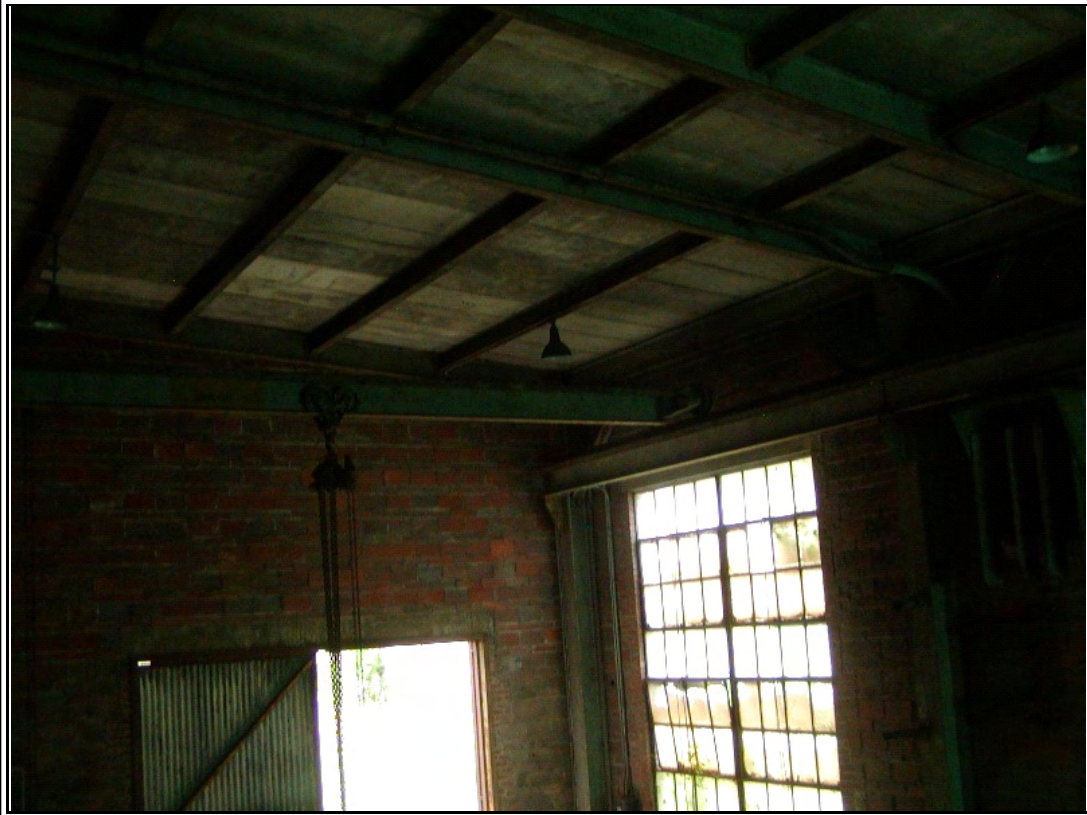
Photograph #: 10 Deteriorated wood roof at west addition
