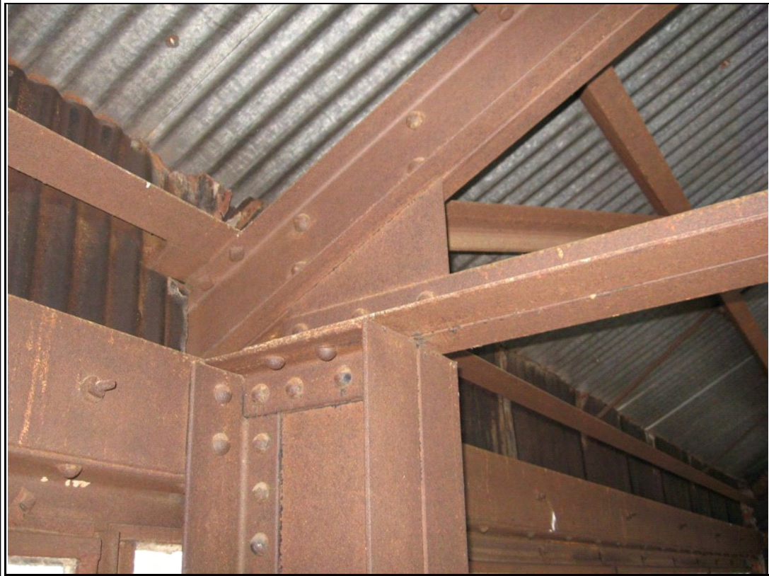
Photograph #: 15 Surface corrosion on steel framing.
