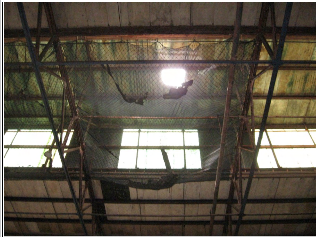
Photograph #: 11 Large hole in deteriorated concrete plank roof deck
