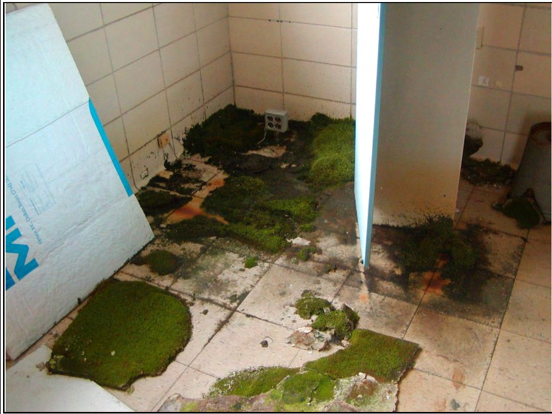
Photograph #: 12 Interior water intrusion damage
