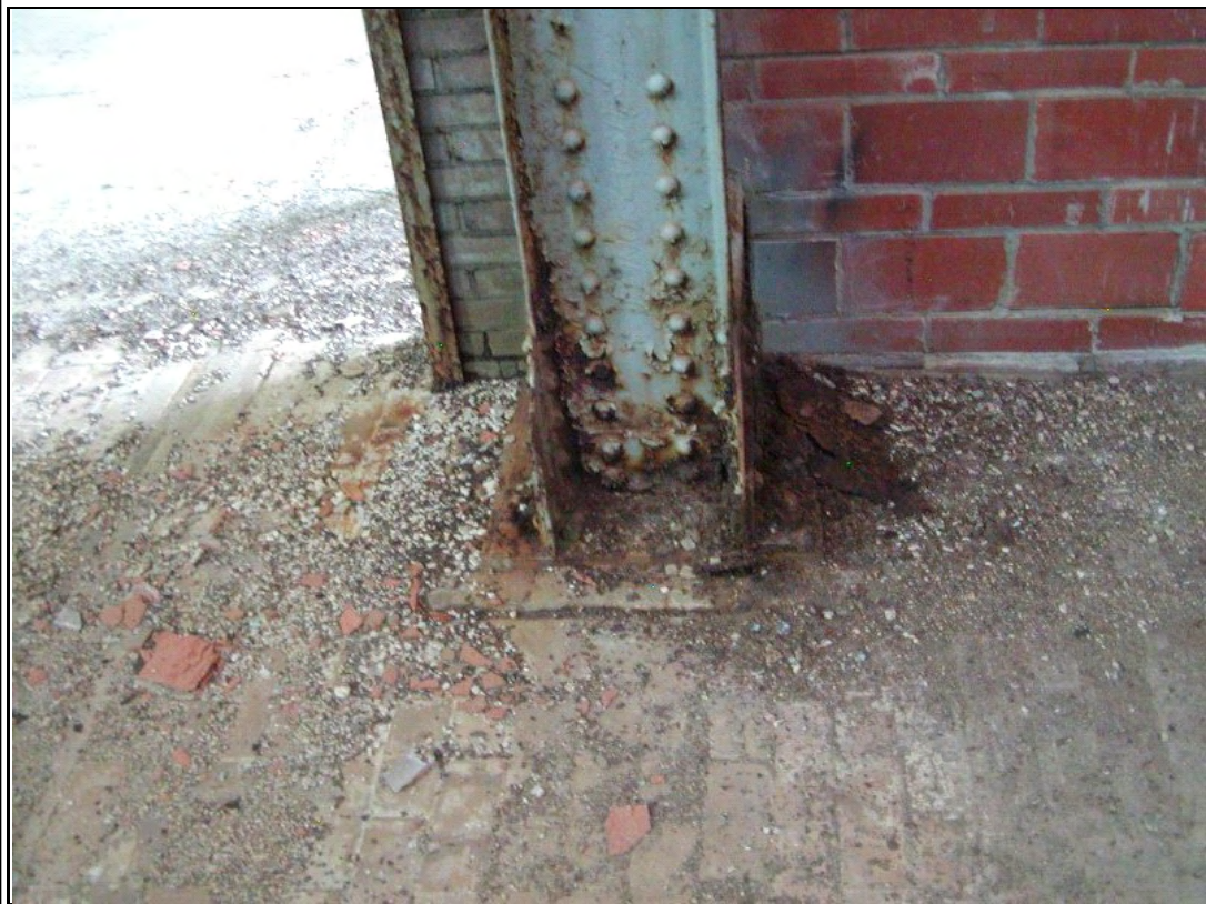
Photograph #: 9 Severe corrosion at column base plate attachment
