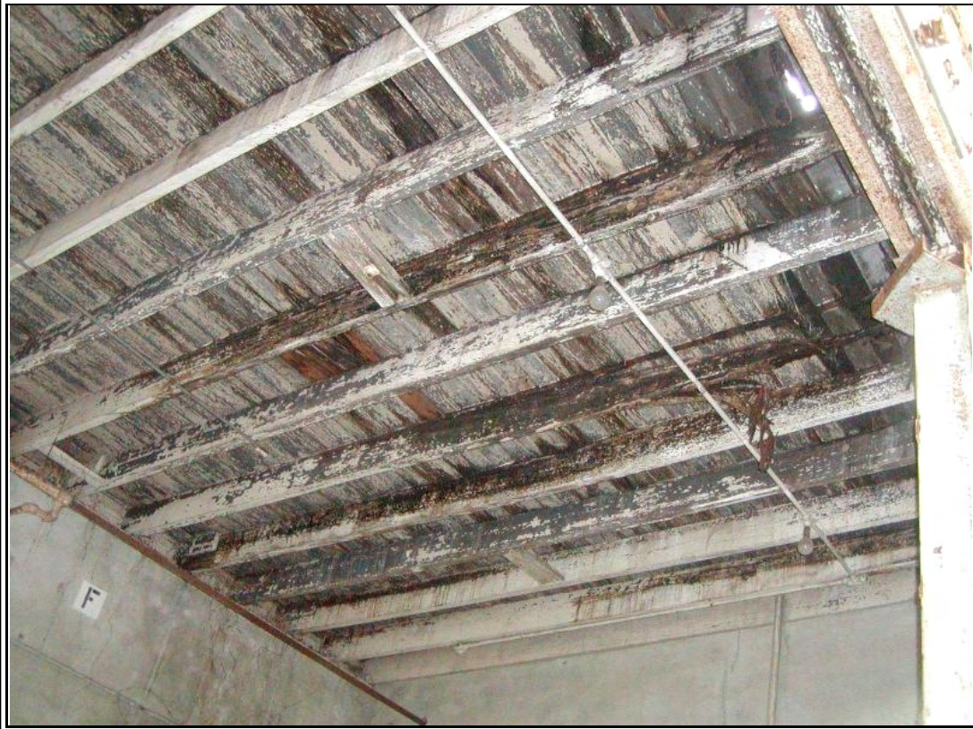
Photograph #: 4 Severely deteriorated wood roof structure.
