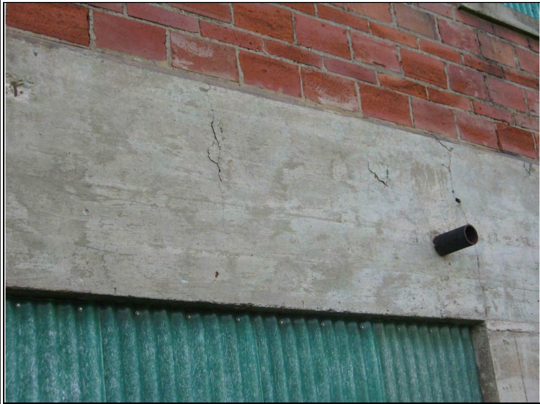
Photograph #: 9 Minor cracks and spalls in exterior face of mezzanine concrete frame
