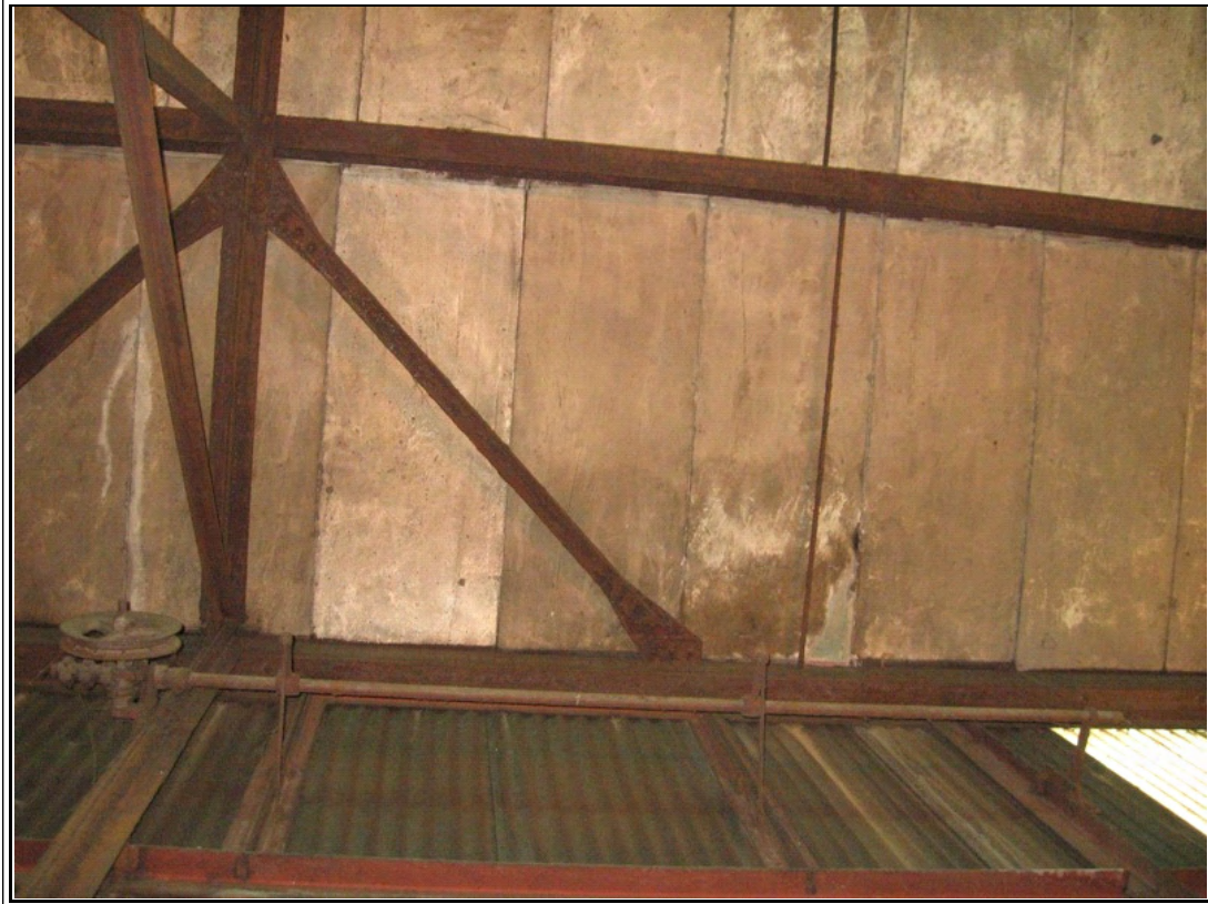
Photograph #: 22 Surface deterioration at roof deck and moderately corroded steel framing at monitor
