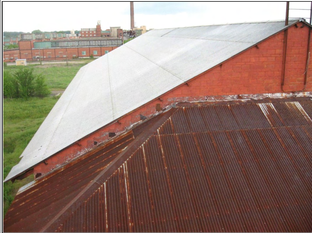
Photograph #: 3 New metal roof on main building and original metal roof on shed at south end
