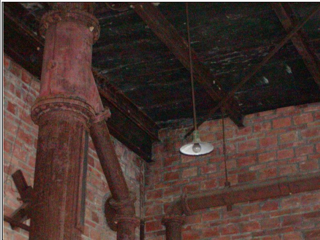
Photograph #: 9 Severely deteriorated roof structure at west end of building.
