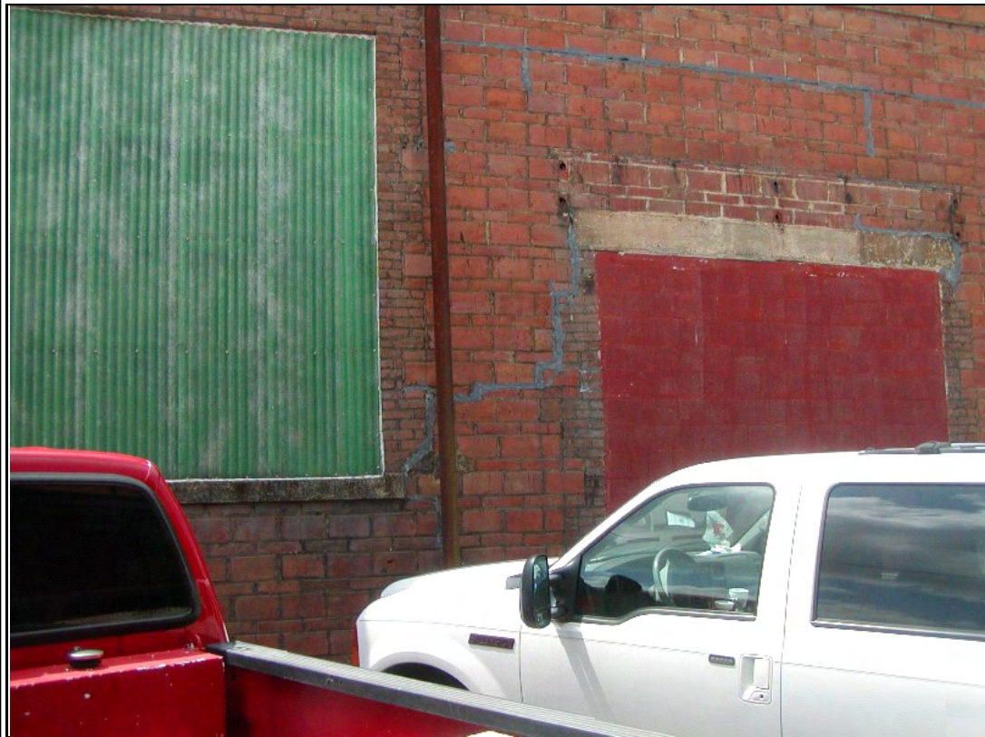
Photograph #: 11 Cracks in masonry at north wall
