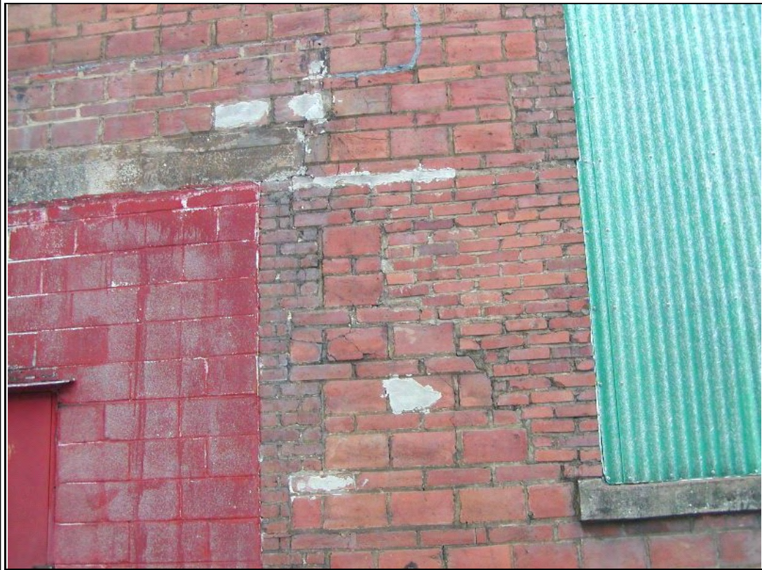
Photograph #: 8 Cracks in masonry (same location as Photo No. 7)
