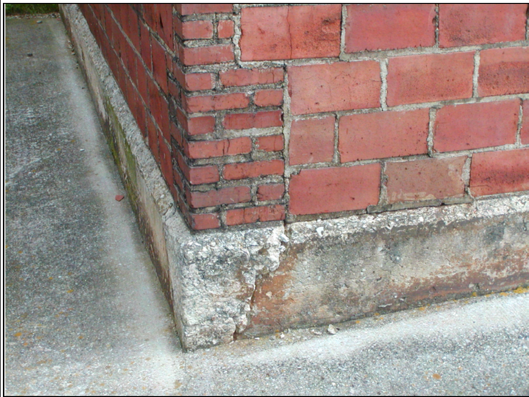
Photograph #: 4 Minor crack on turned down slab
