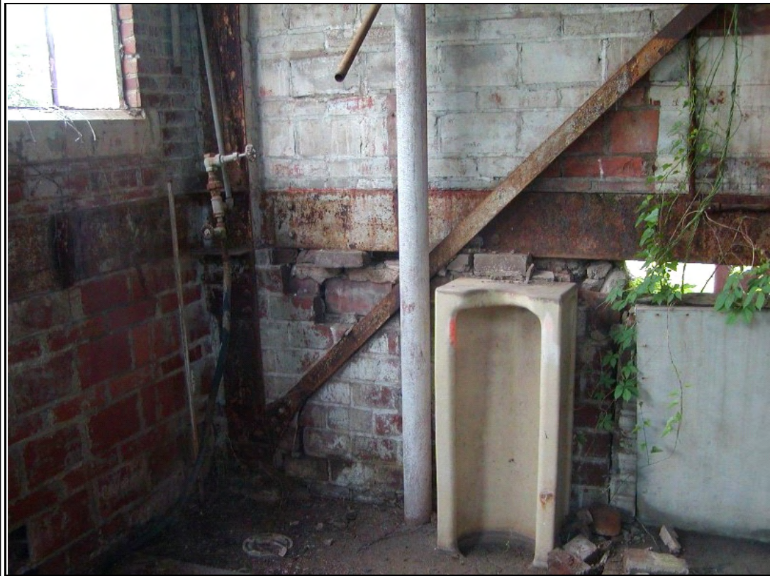
Photograph #: 10 Damaged masonry infill at southeast corner.
