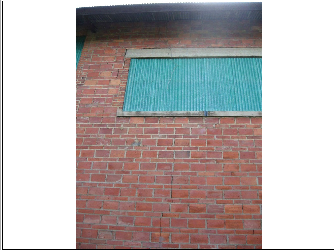
Photograph #: 4 Vertical cracks in masonry
