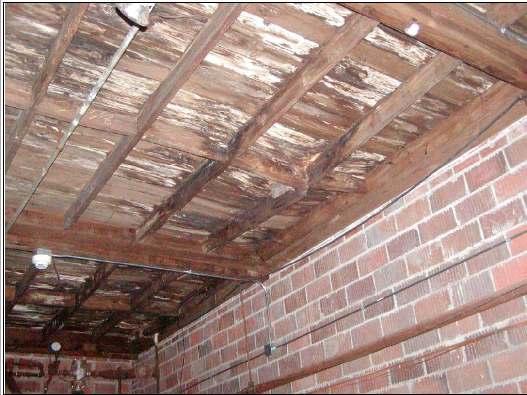
Photograph #: 19 Ruined roof deck of interior enclosure
