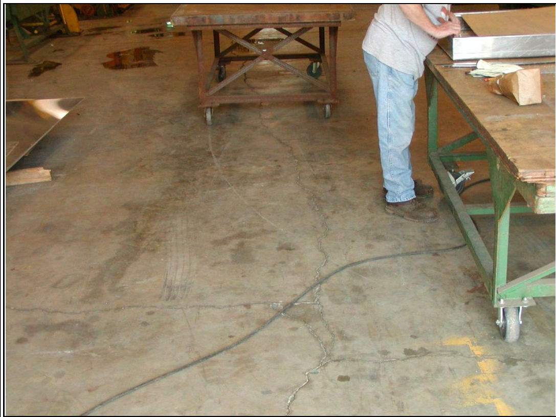
Photograph #: 10 Large cracks in concrete floor slab
