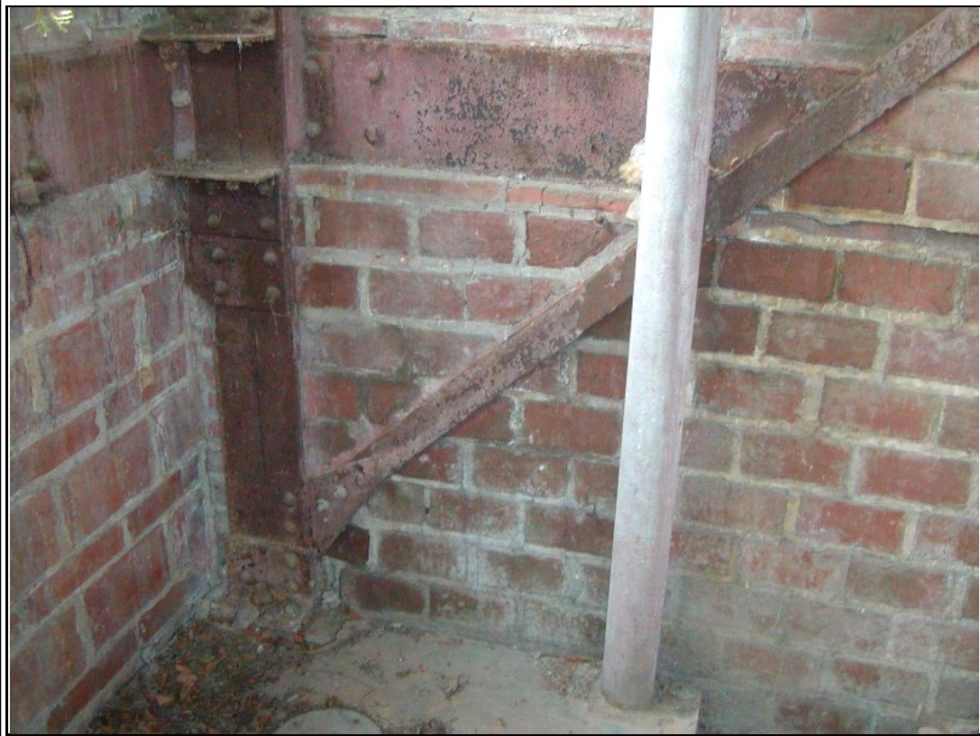
Photograph #: 9 Deteriorated steel column and wall framing
