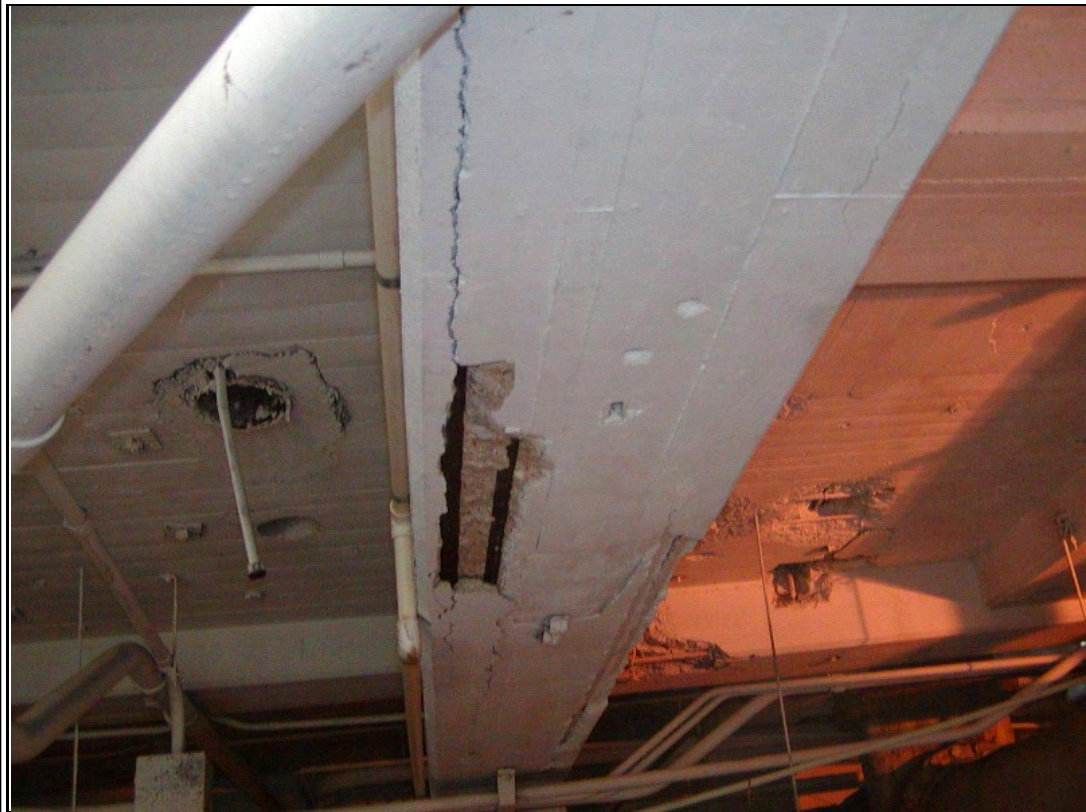
Photograph #: 21 Severely spalled concrete beam at basement ceiling
