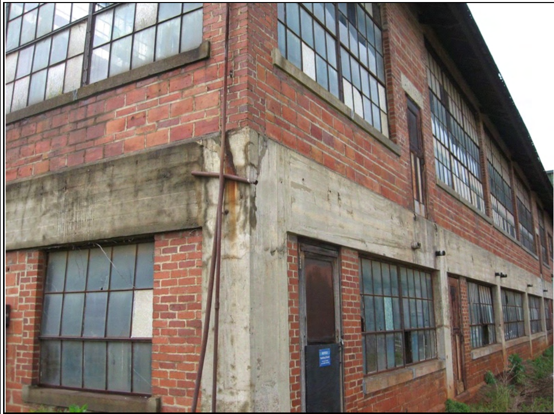
Photograph #: 3 Exterior cracks in concrete mezzanine frame at southeast corner.
