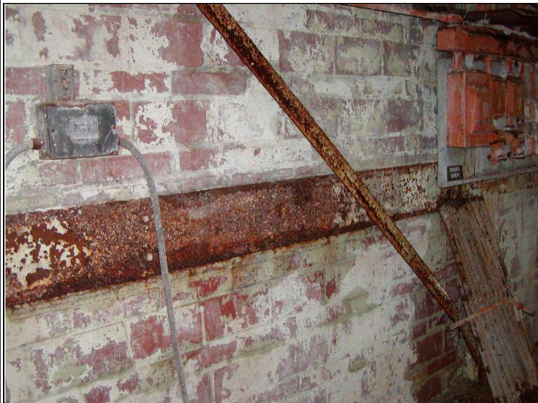
Photograph #: 11 Heavily corroded steel framing at north wall
