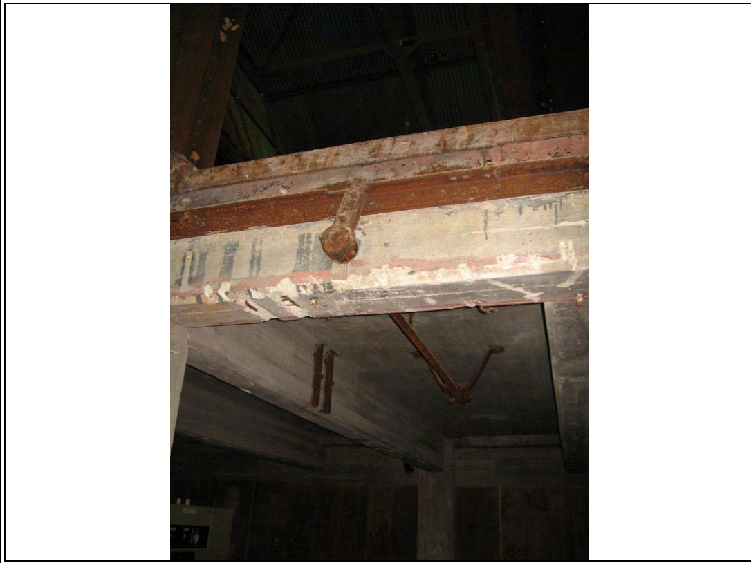
Photograph #: 26 Damaged mezzanine concrete beam
