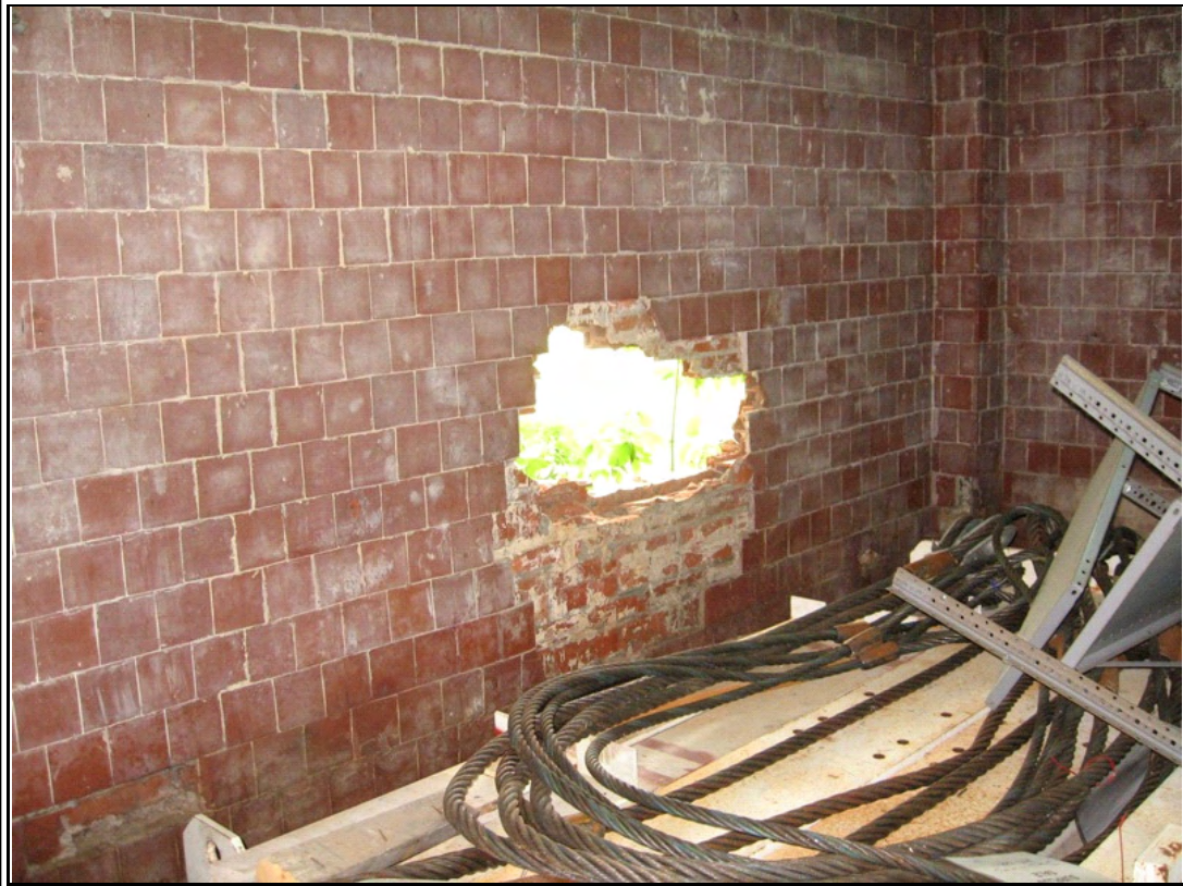
Photograph #: 19 Large hole in exterior masonry wall
