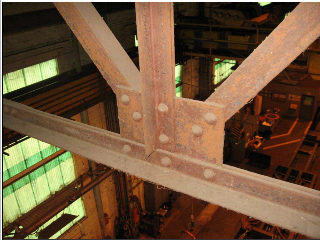
Photograph #: 18 Moderately corroded roof framing
