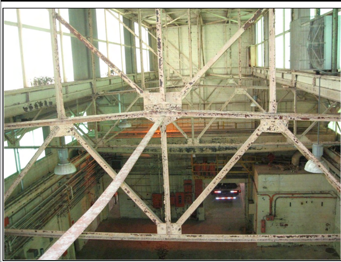
Photograph #: 16 View of steel roof trusses
