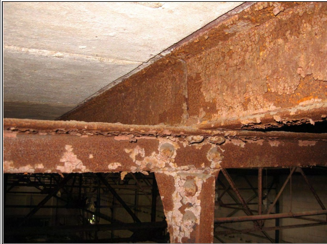
Photograph #: 7 Severely corroded steel framing
