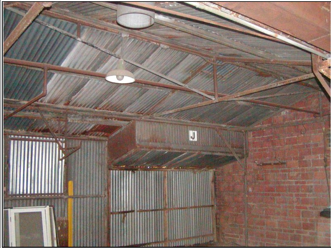
Photograph #: 8 Corroded metal roof deck and steel framing at east addition.
