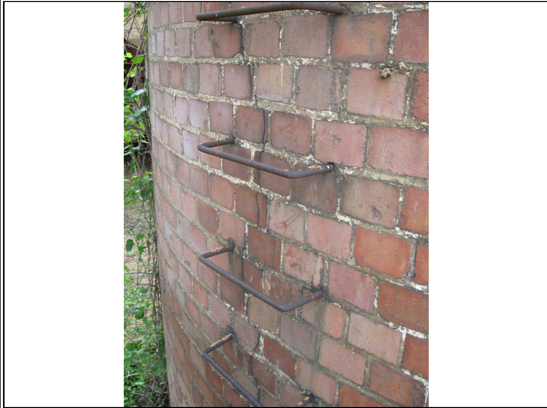
Photograph #: 20 Cracked masonry at smokestack
