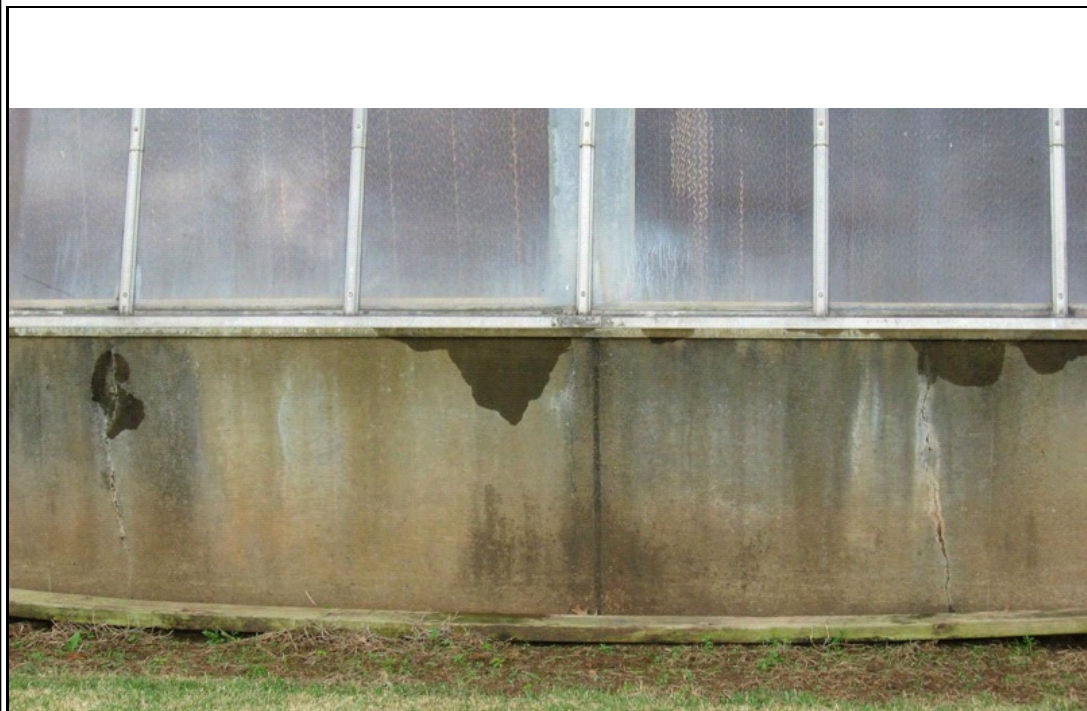
Photograph #: 14 Cracks in foundation wall at greenhouse 1
