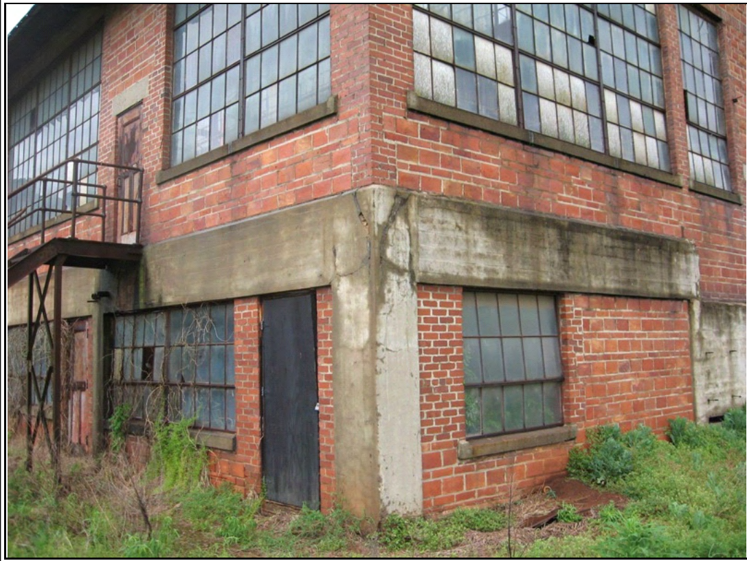
Photograph #: 2 Exterior cracks in concrete mezzanine frame at southwest corner
