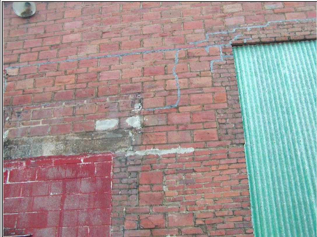
Photograph #: 7 Cracks in masonry in south wall
