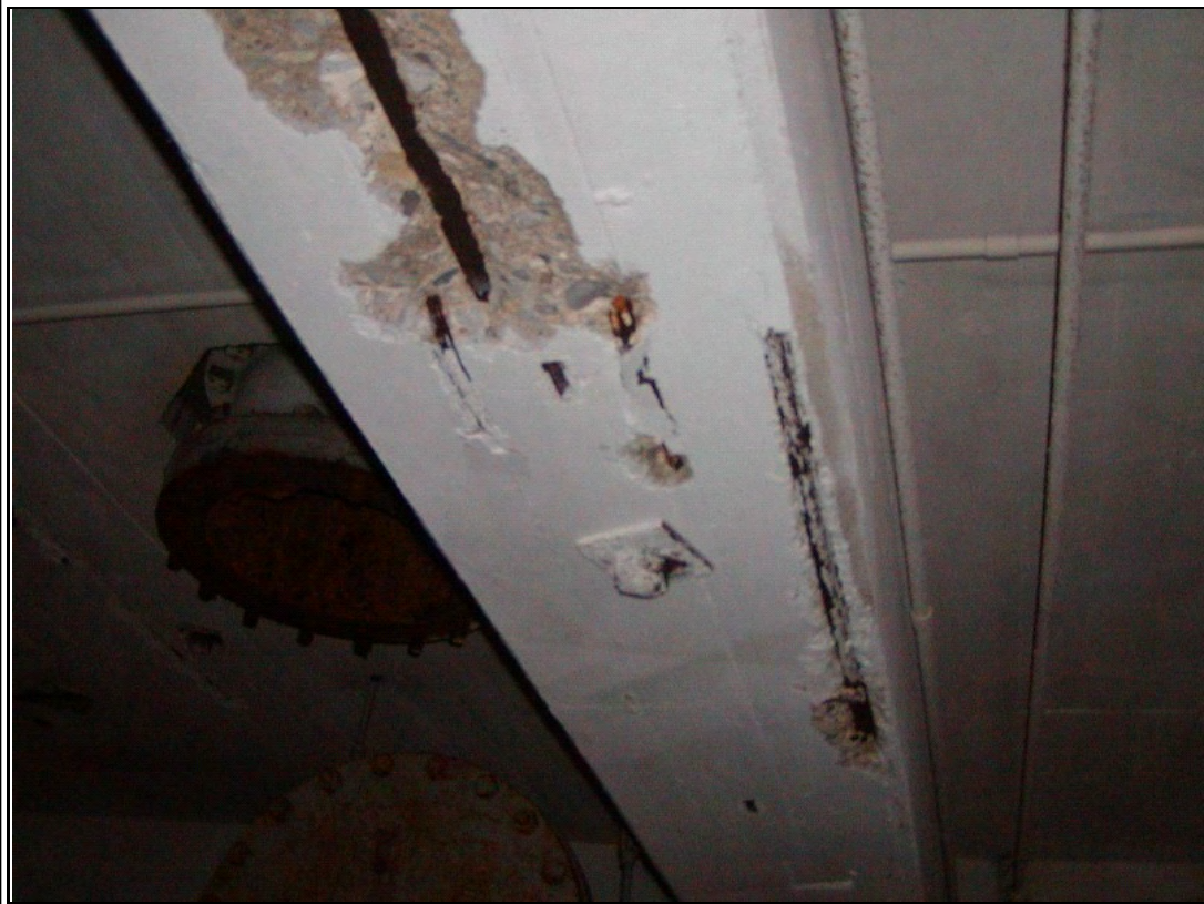
Photograph #: 22 Severely spalled concrete beam at basement ceiling
