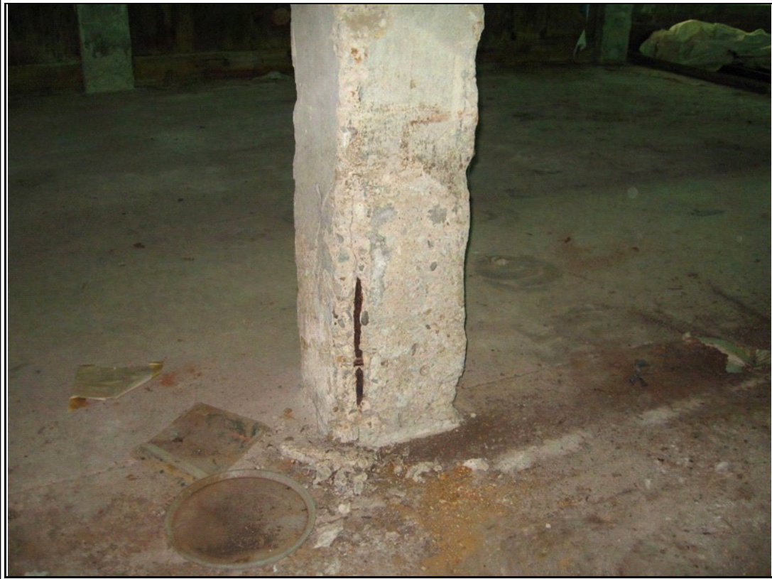
Photograph #: 22 Severely spalled mezzanine concrete column
