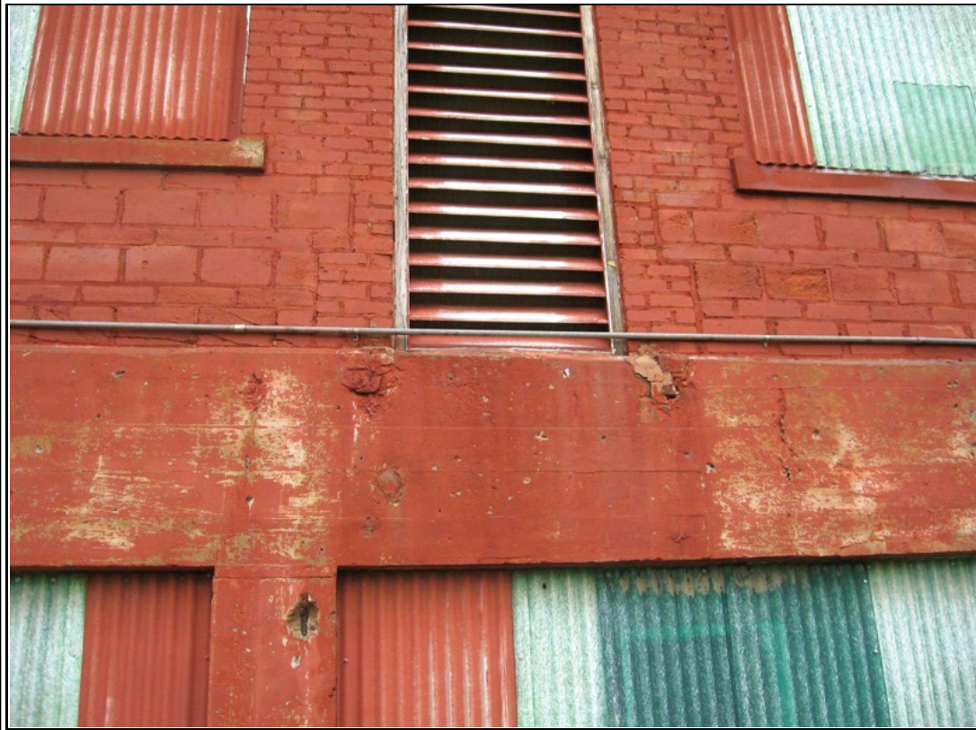
Photograph #: 6 Cracks and spalls in exterior face of concrete mezzanine frame
