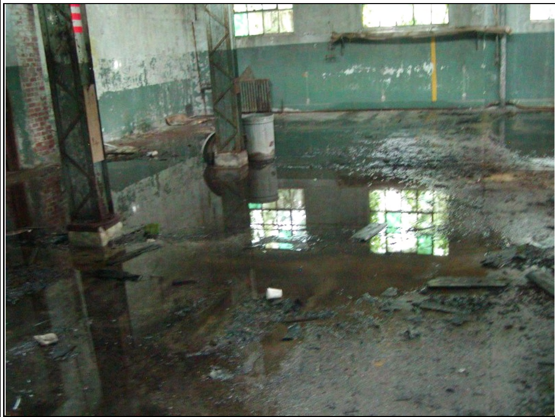
Photograph #: 5 Standing water on floor inside building; corroded steel columns.
