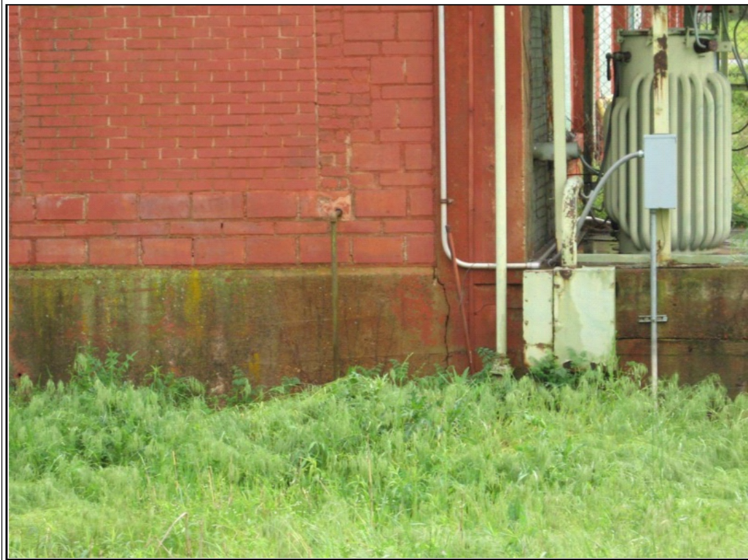
Photograph #: 8 Crack in turned-down slab at northwest corner
