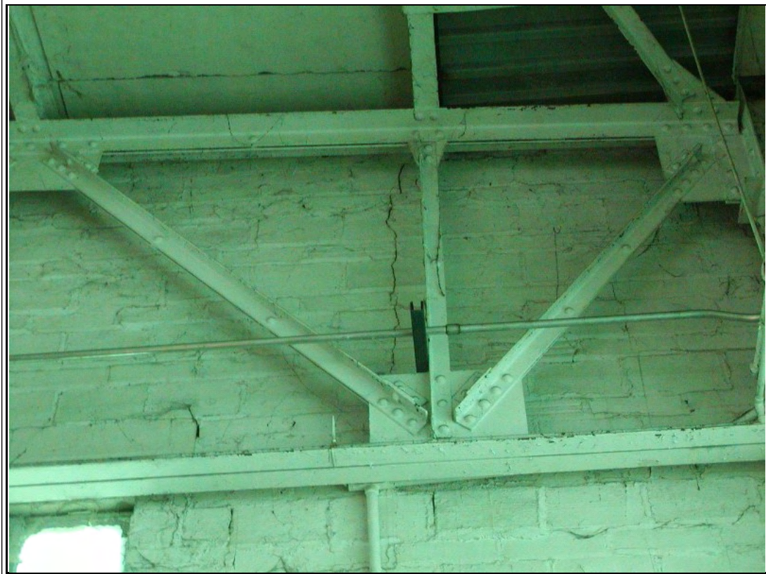
Photograph #: 11 Crack in masonry at end wall
