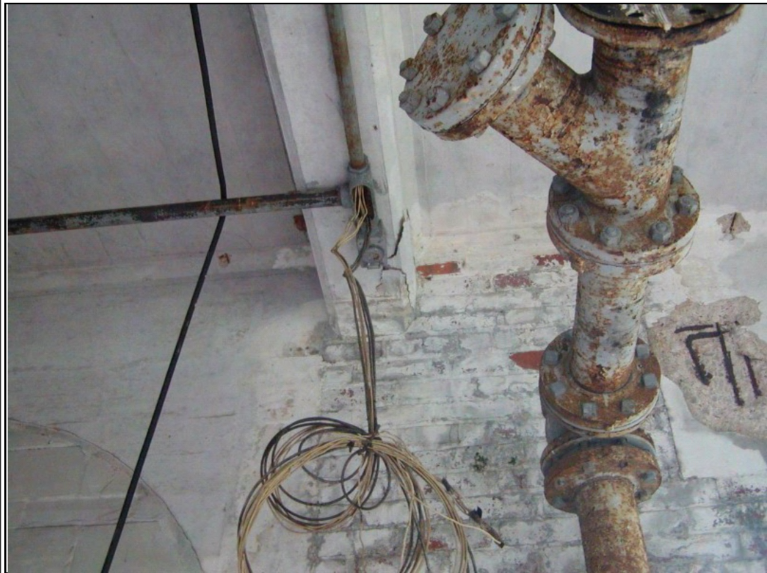
Photograph #: 11 Cracked roof beam and spalled concrete wall at upper floor
