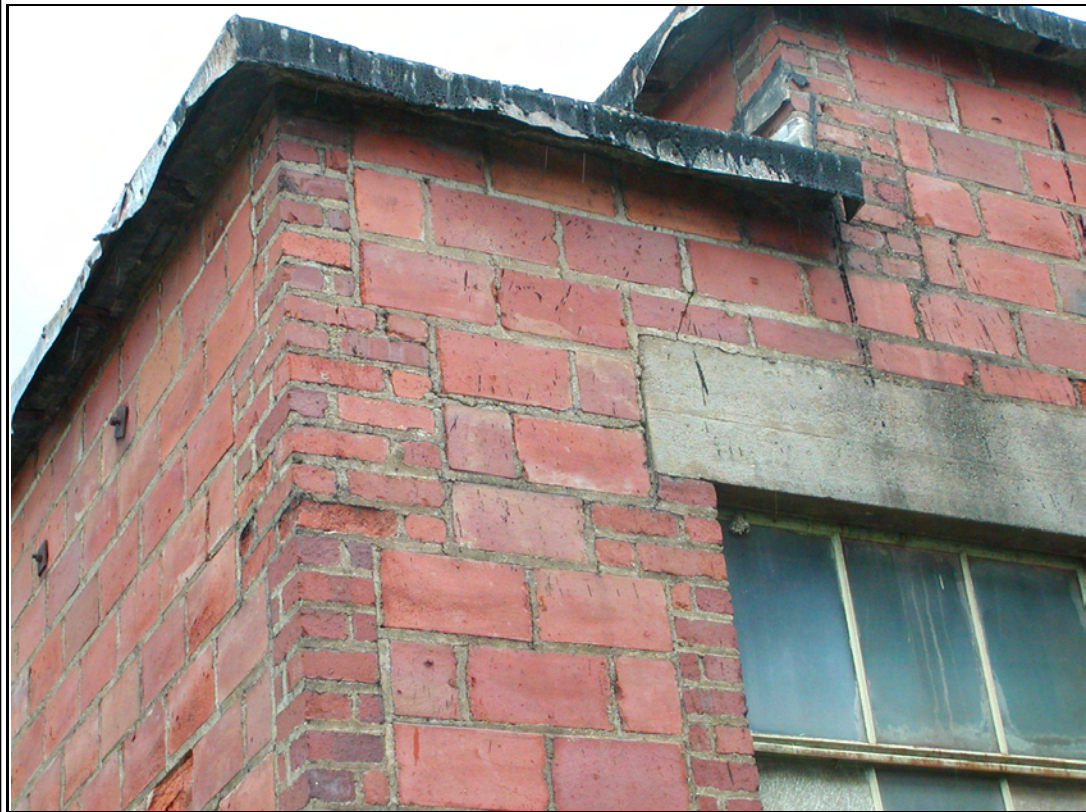
Photograph #: 3 Minor spalls in exterior masonry
