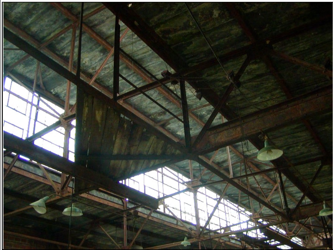
Photograph #: 7 Corroded steel framing and deteriorated concrete plank roof deck.
