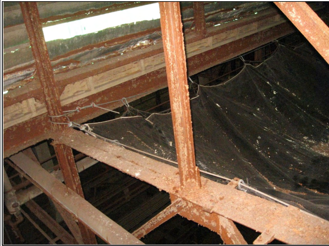
Photograph #: 12 Severely corroded structural steel
