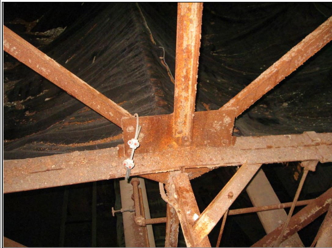
Photograph #: 11 Severely corroded structural steel
