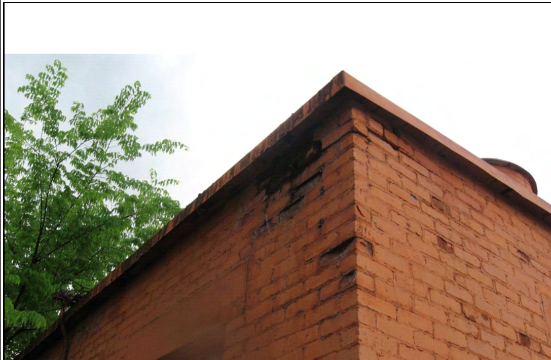
Photograph #: 3 Deteriorated masonry wall at northeast corner with water intrusion damage - see Photograph # 5.
