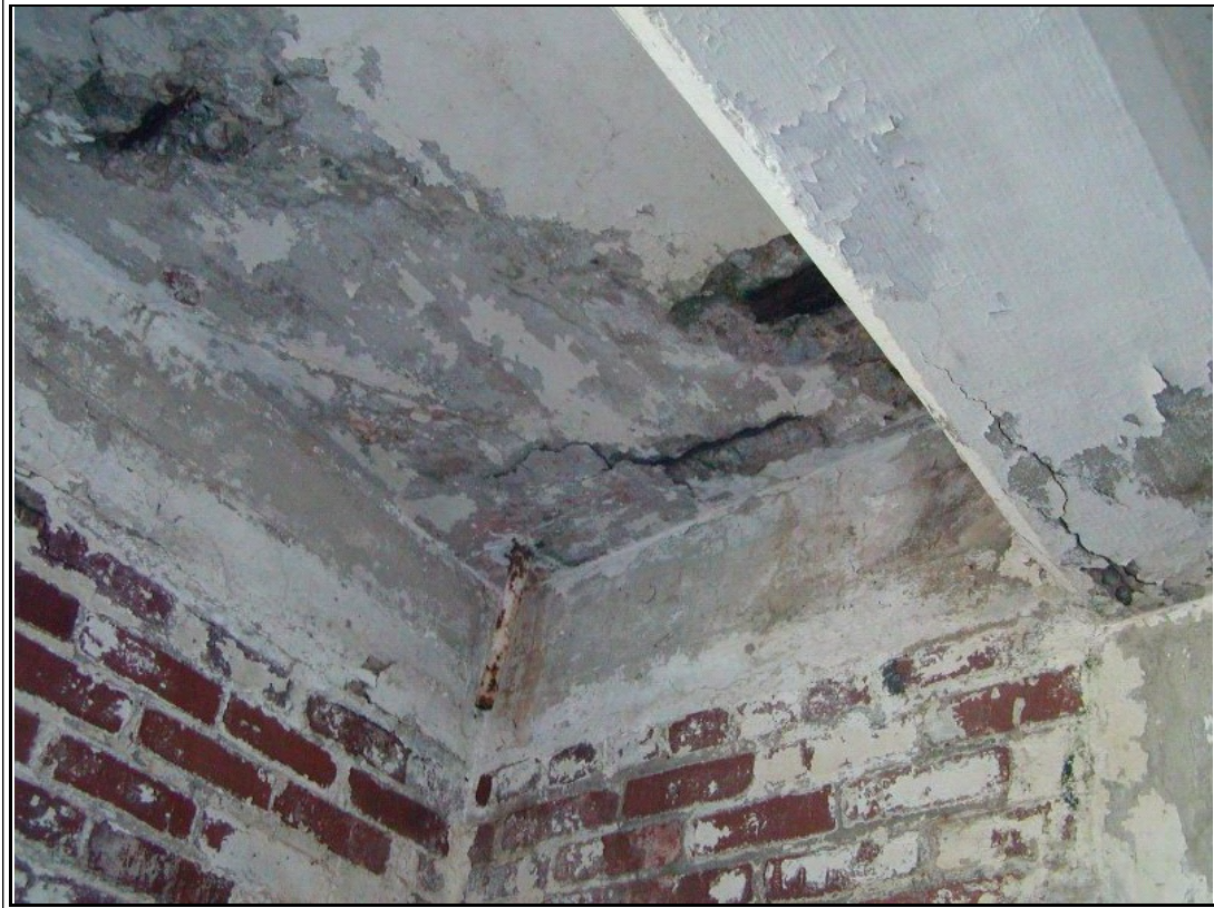
Photograph #: 16 Deteriorated concrete of underside of upper floor
