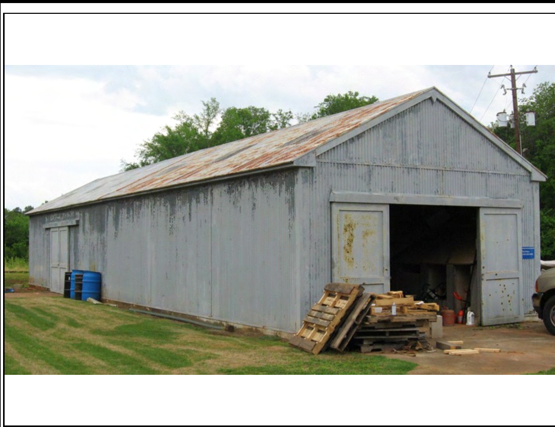
Photograph #: 19 Exterior view of metal storage building with surface corrosion at roof
