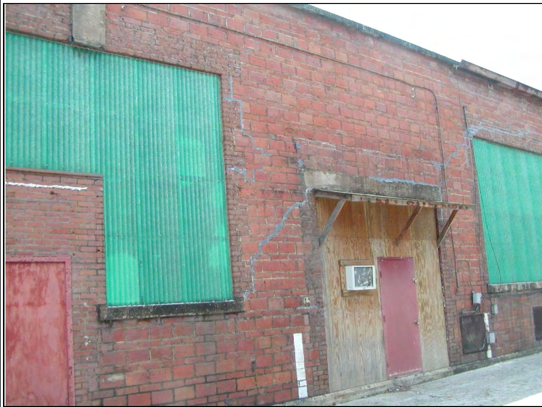
Photograph #: 12 Cracks in masonry at north wall
