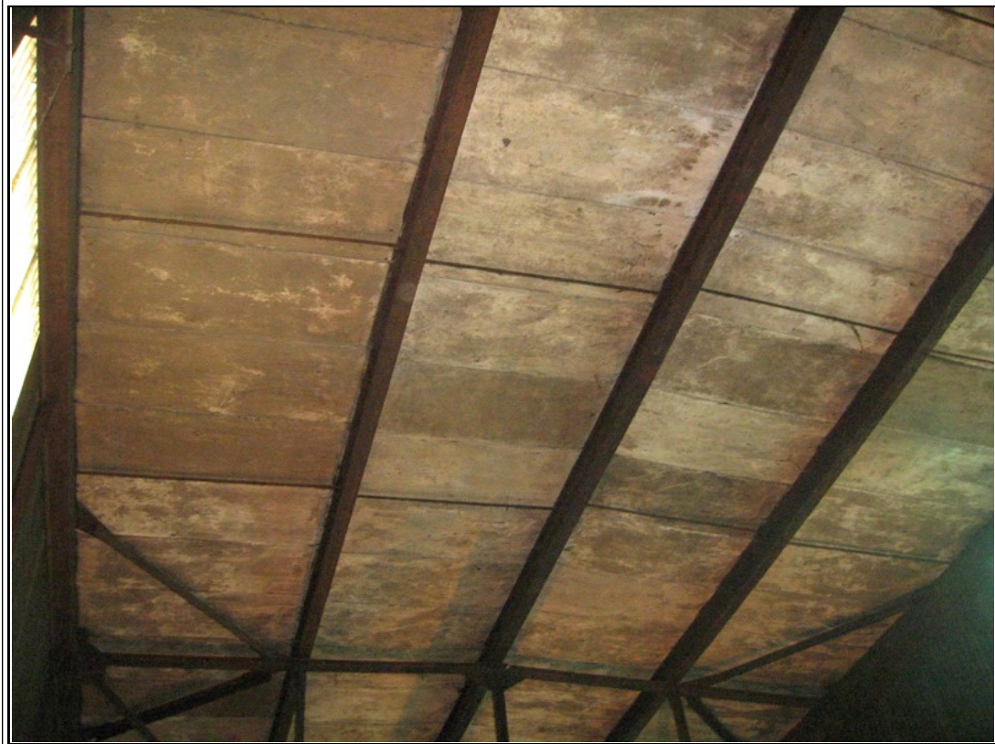
Photograph #: 21 Surface deterioration of roof deck at monitor
