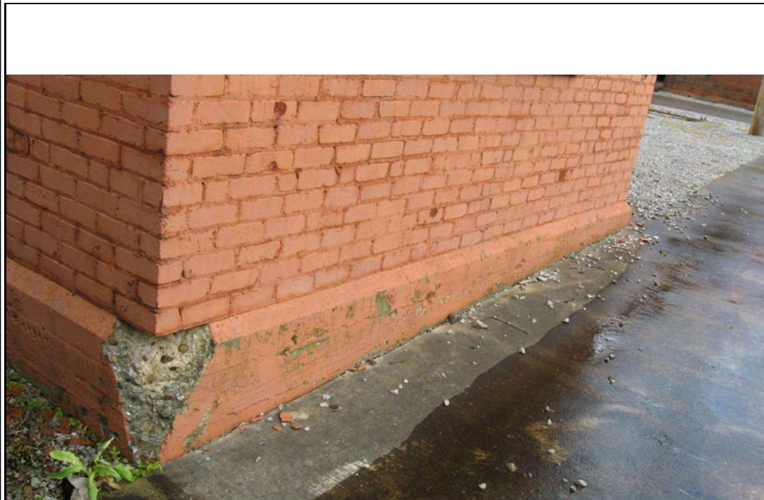
Photograph #: 4 Spalled concrete foundation at northeast corner.
