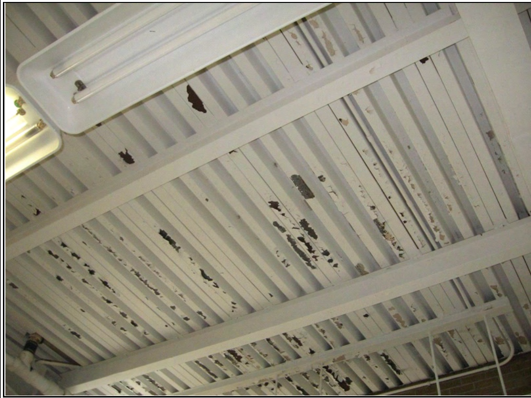
Photograph #: 16 Service Building - flaking paint at metal roof deck in vehicle storage area
