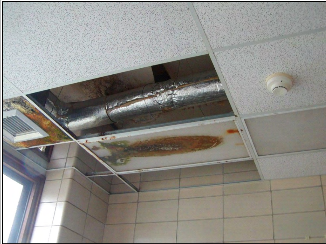
Photograph #: 11 Interior water intrusion damage
