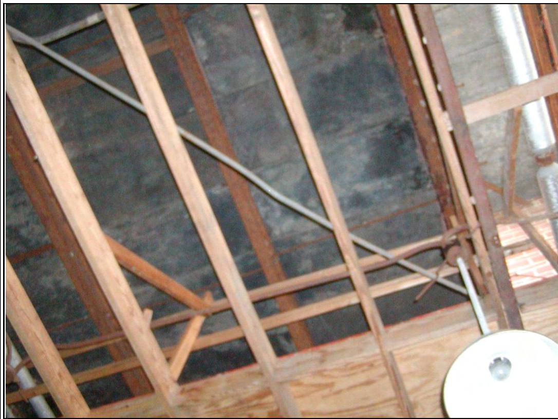
Photograph #: 10 Corroded steel framing and deteriorated roof deck at low roof
