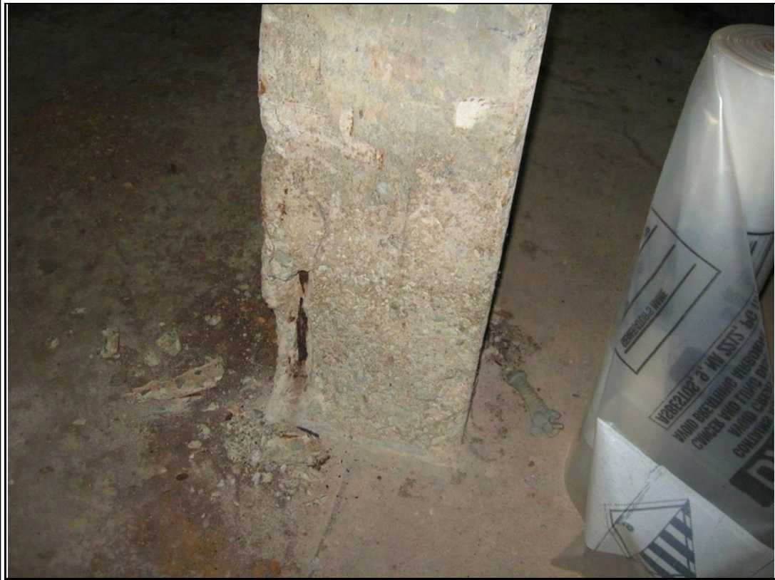
Photograph #: 21 Severely spalled mezzanine concrete column
