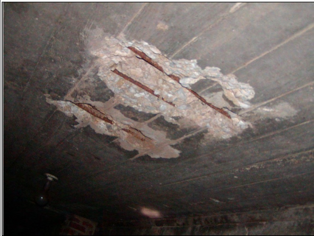
Photograph #: 18 Severely spalled concrete at basement ceiling
