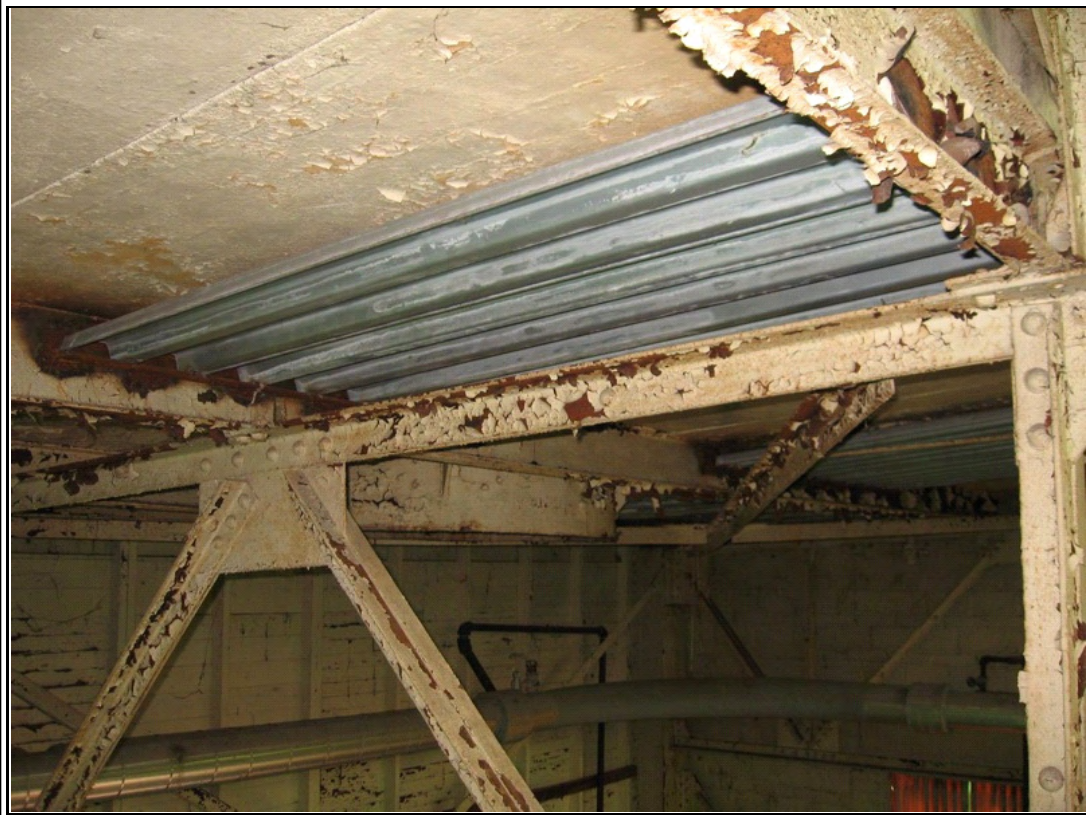
Photograph #: 20 Flaking paint at corroded steel roof framing
