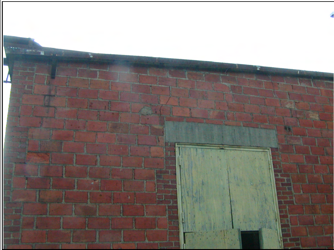
Photograph #: 2 Minor cracks in masonry at east wall of substation
