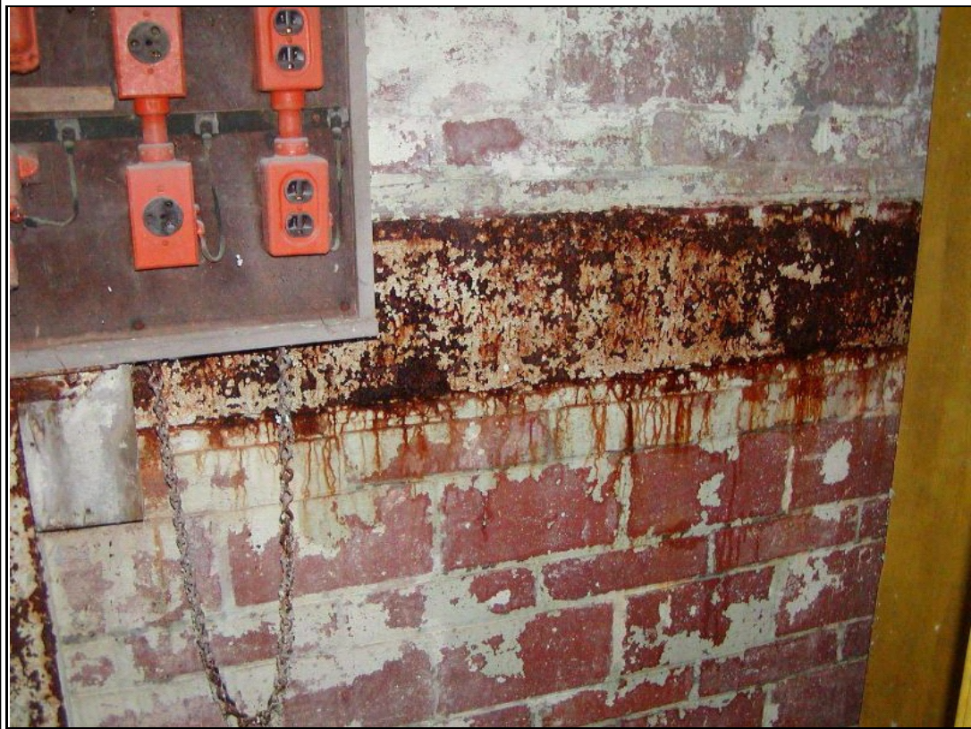
Photograph #: 12 Heavily corroded steel framing at north wall
