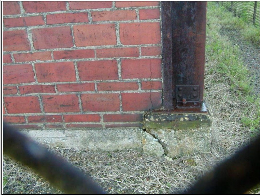
Photograph #: 4 Cracked concrete pier and masonry at northwest corner
