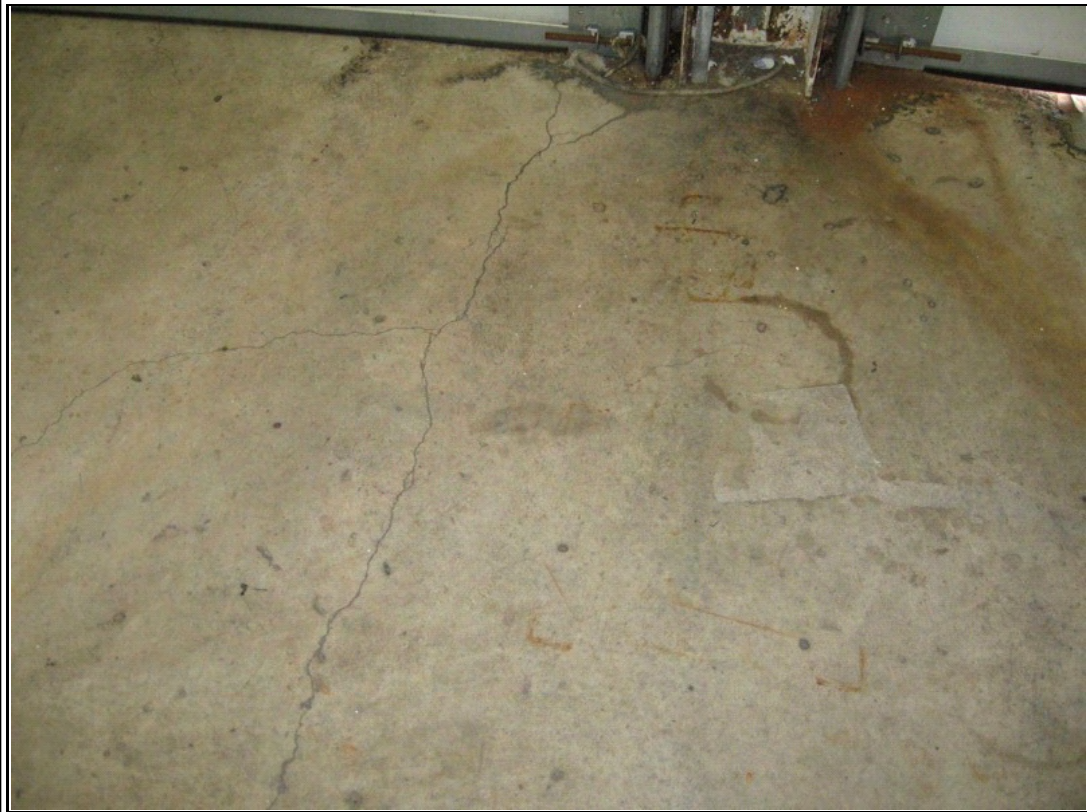
Photograph #: 19 Service Building - cracks in slab at vehicle storage area
