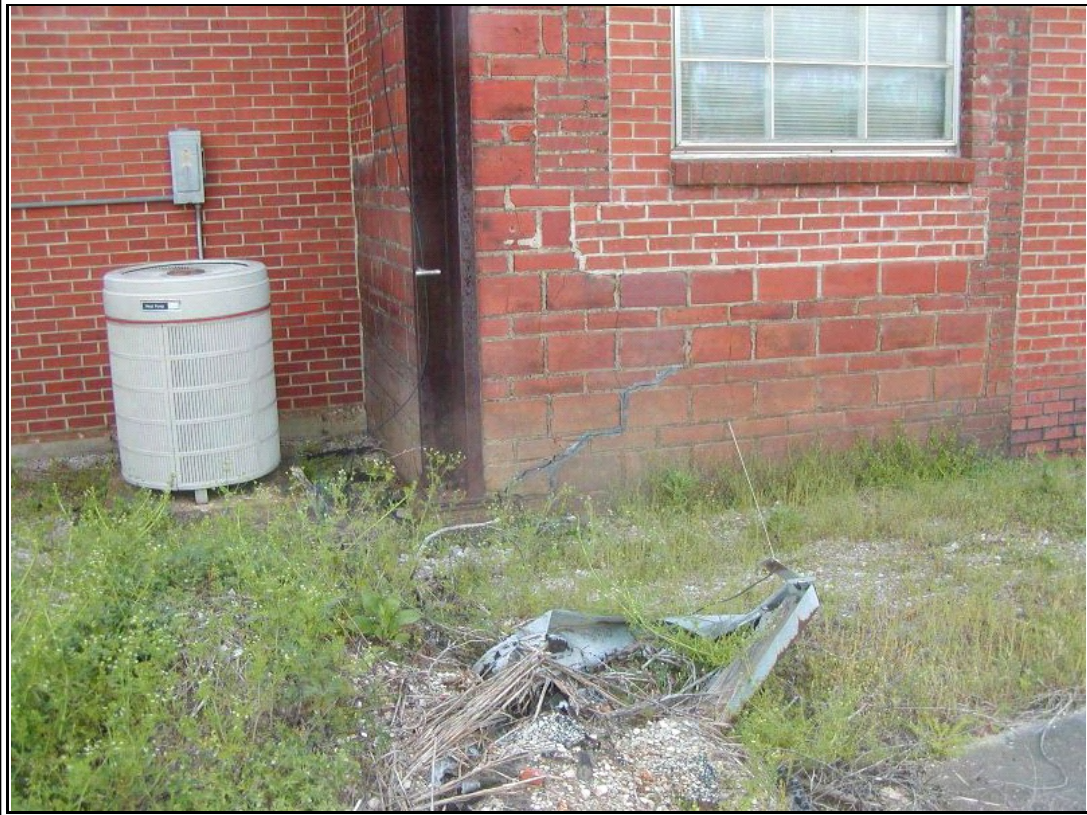
Photograph #: 4 Crack in masonry at northwest corner where north addition adjoins original building
