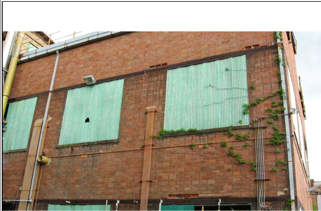
Photograph #: 15 Spalled masonry and corroded steel lintel beams - north side.
