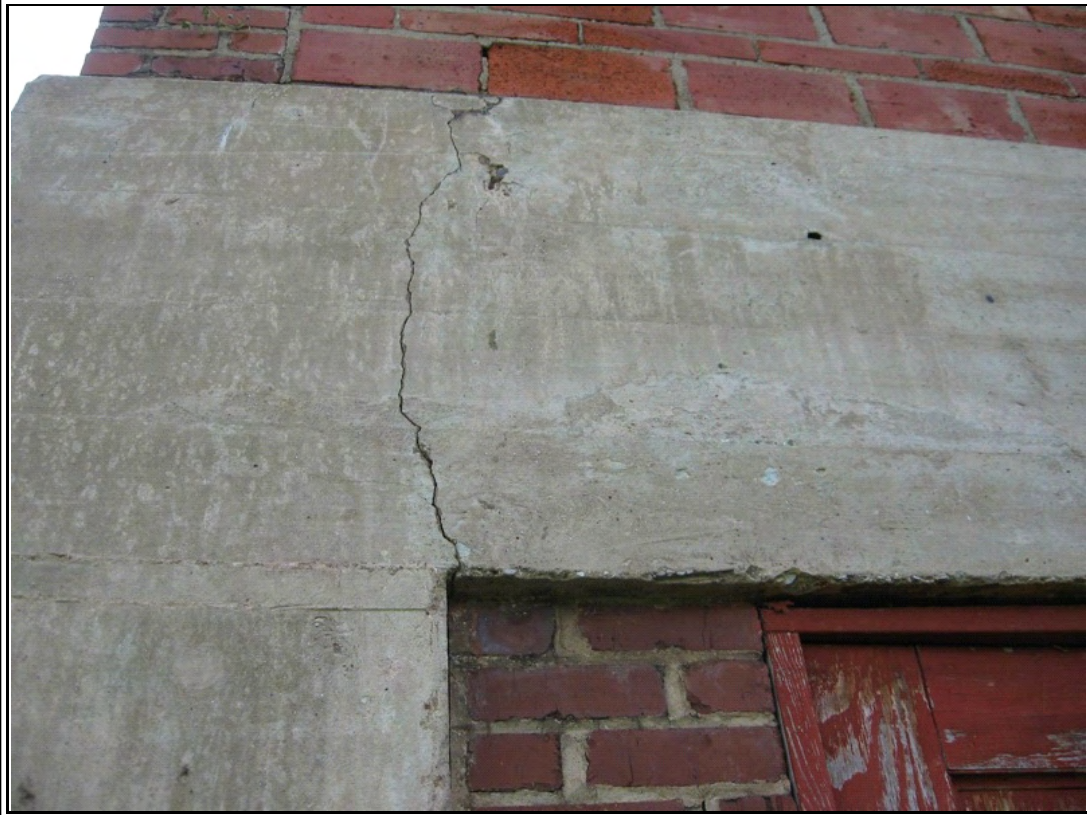
Photograph #: 10 Substantial crack in exterior mezzanine concrete frame
