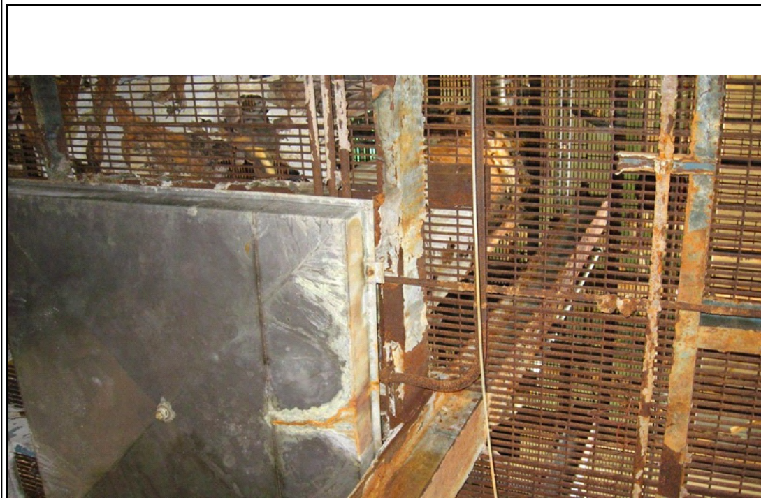
Photograph #: 22 Severely corroded steel at multi-level interior mezzanine.
