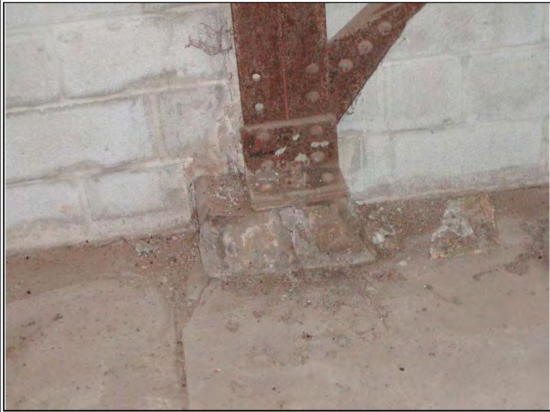
Photograph #: 10 Deteriorated concrete pier at column
