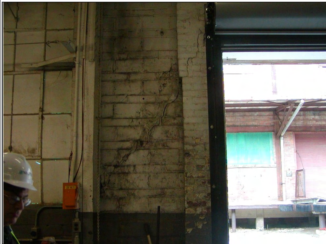
Photograph #: 21 Diagonal crack in masonry at north wall
