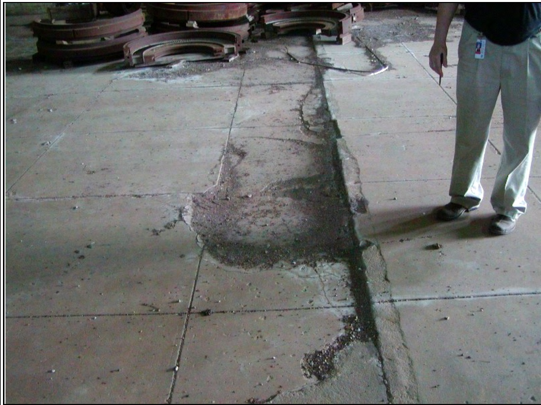
Photograph #: 10 Defective area of elevated slab above basement
