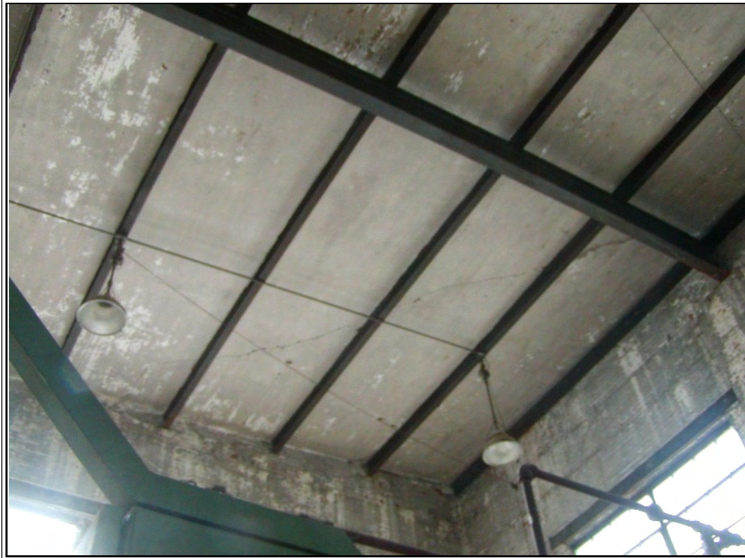
Photograph #: 14 Crack in concrete roof deck
