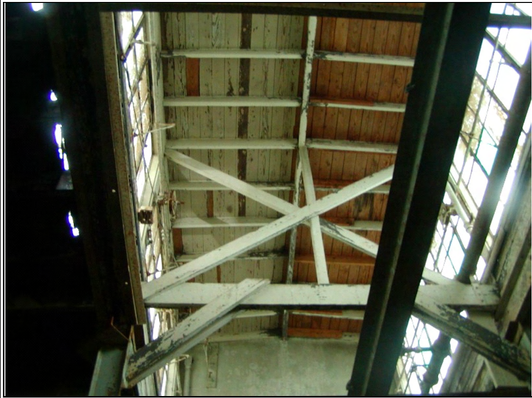
Photograph #: 6 Partially repaired roof deck at clerestory monitor.
