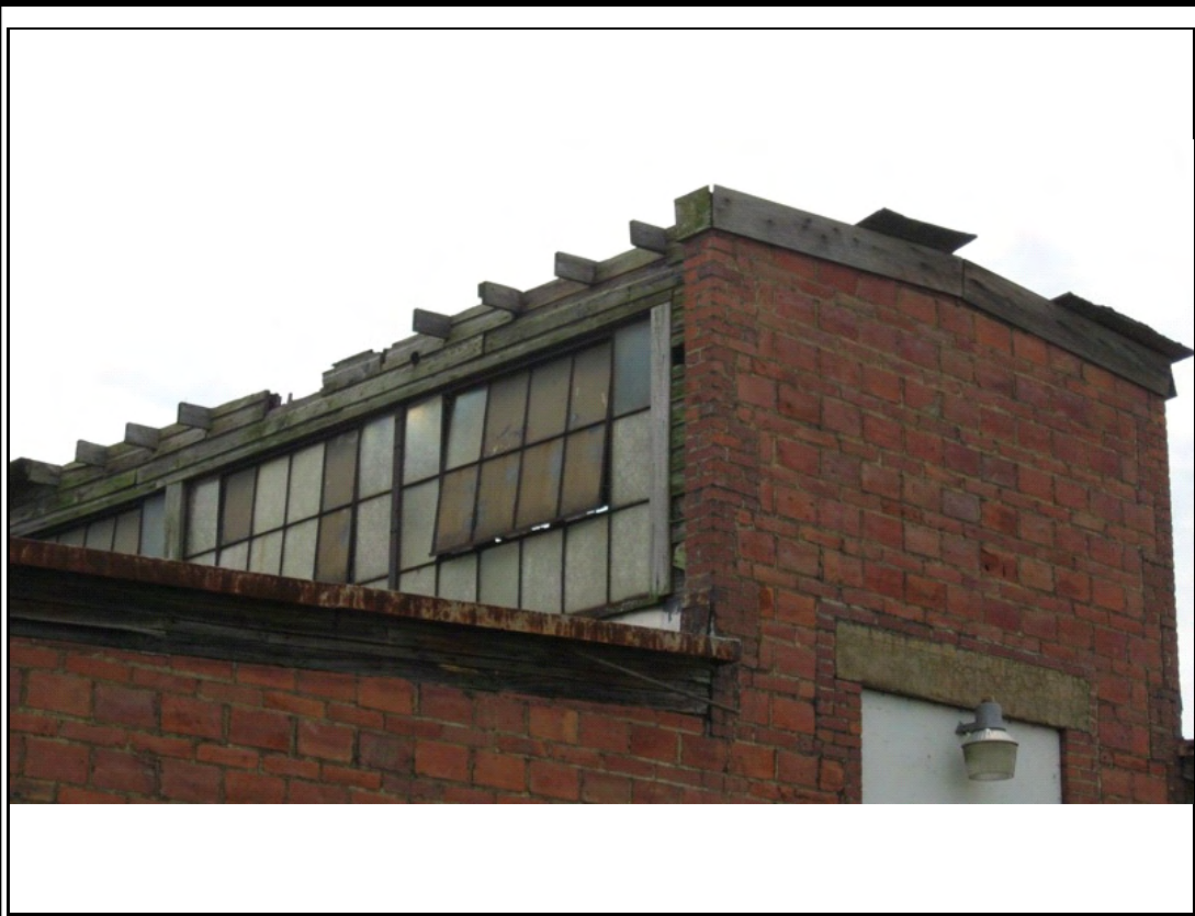
Photograph #: 3 View of clerestory monitor with deteriorated roof structure.
