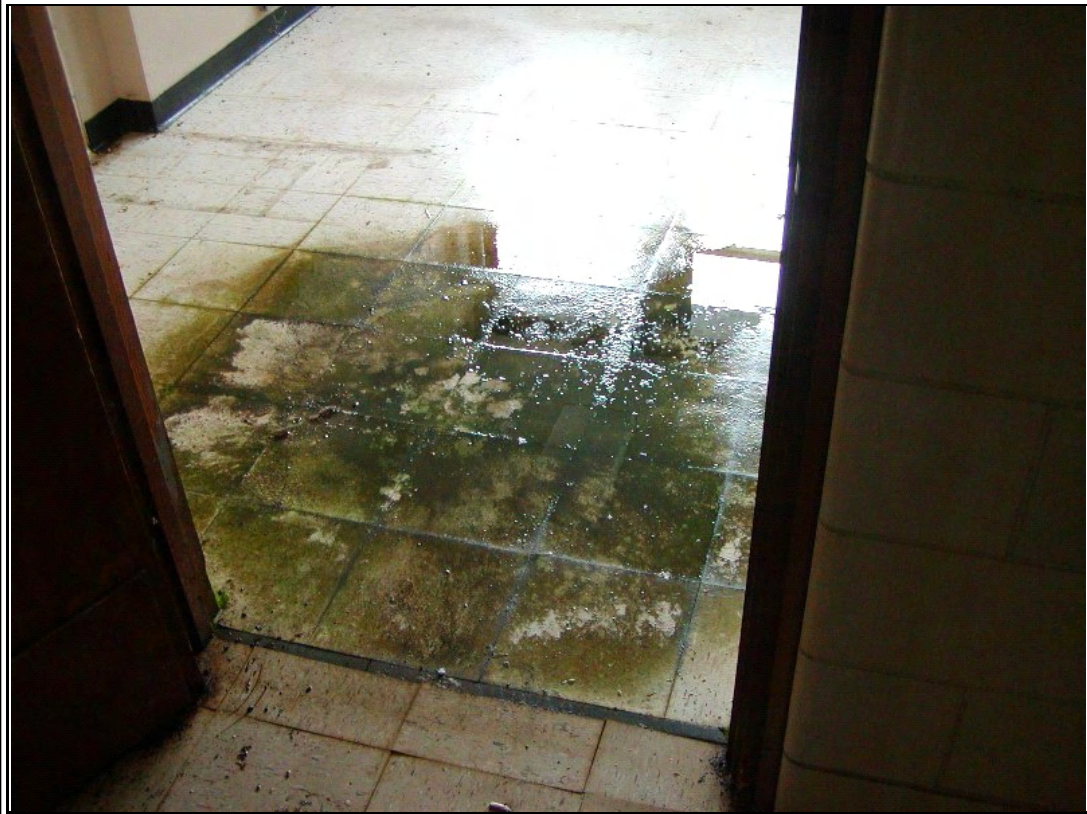
Photograph #: 13 Interior water intrusion damage
