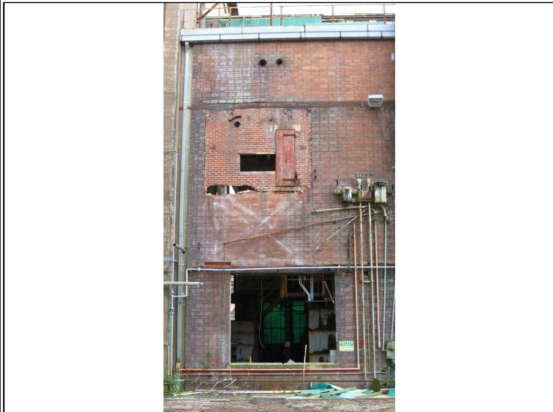
Photograph #: 16 Defective exterior masonry, including partially collapsed brick infill - north side.
