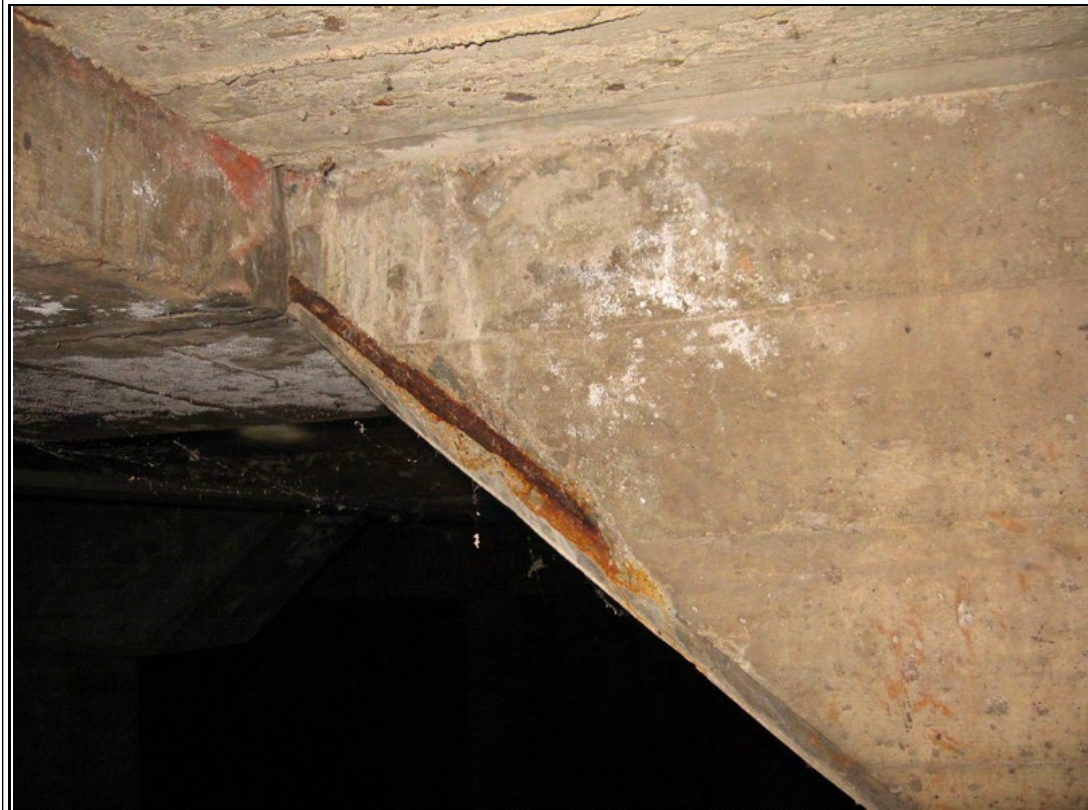
Photograph #: 18 Spalled concrete at basement structure
