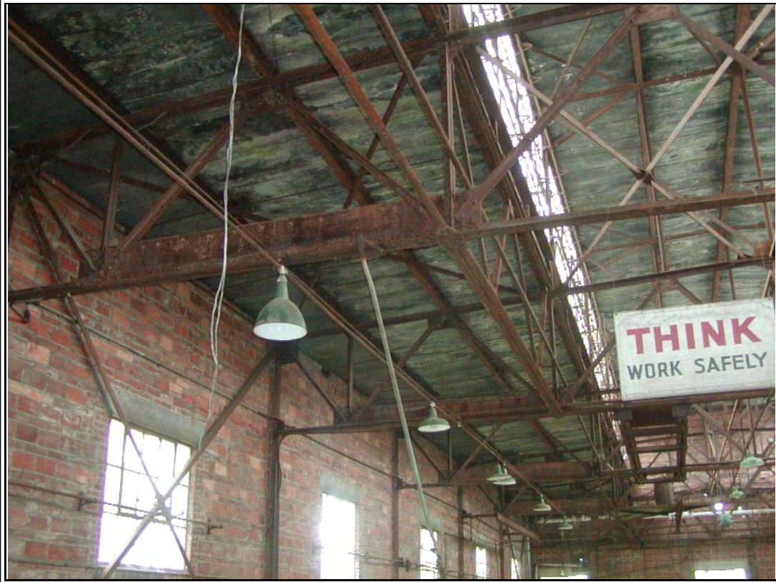
Photograph #: 6 Corroded steel framing and deteriorated concrete plank roof deck.
