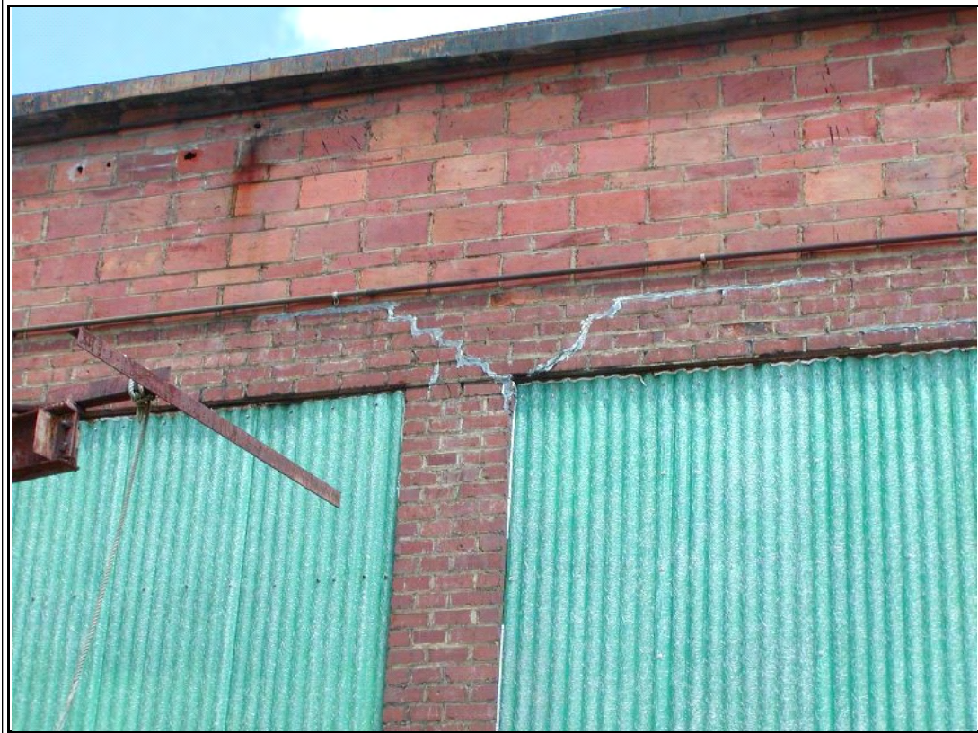
Photograph #: 9 Cracks in masonry lintels at south wall
