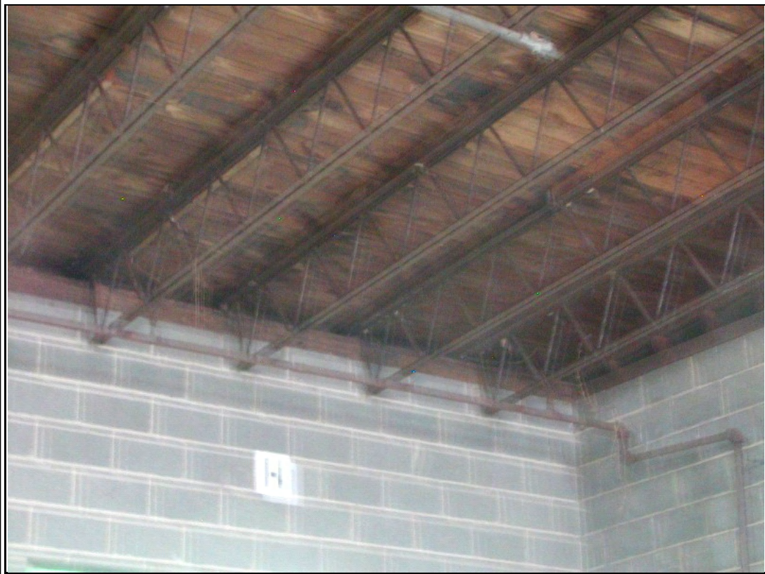
Photograph #: 7 Wood plank roof deck at east addition is damaged by water intrusion.
