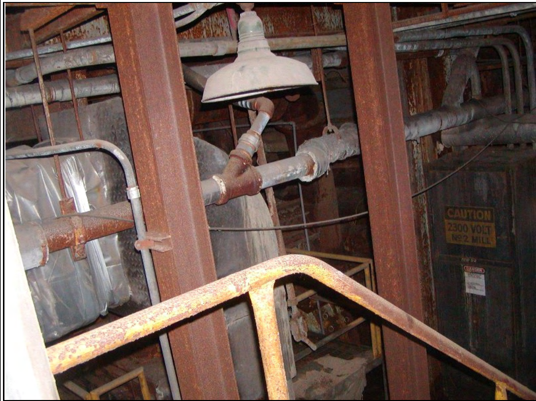
Photograph #: 14 Corroded steel framing in basement
