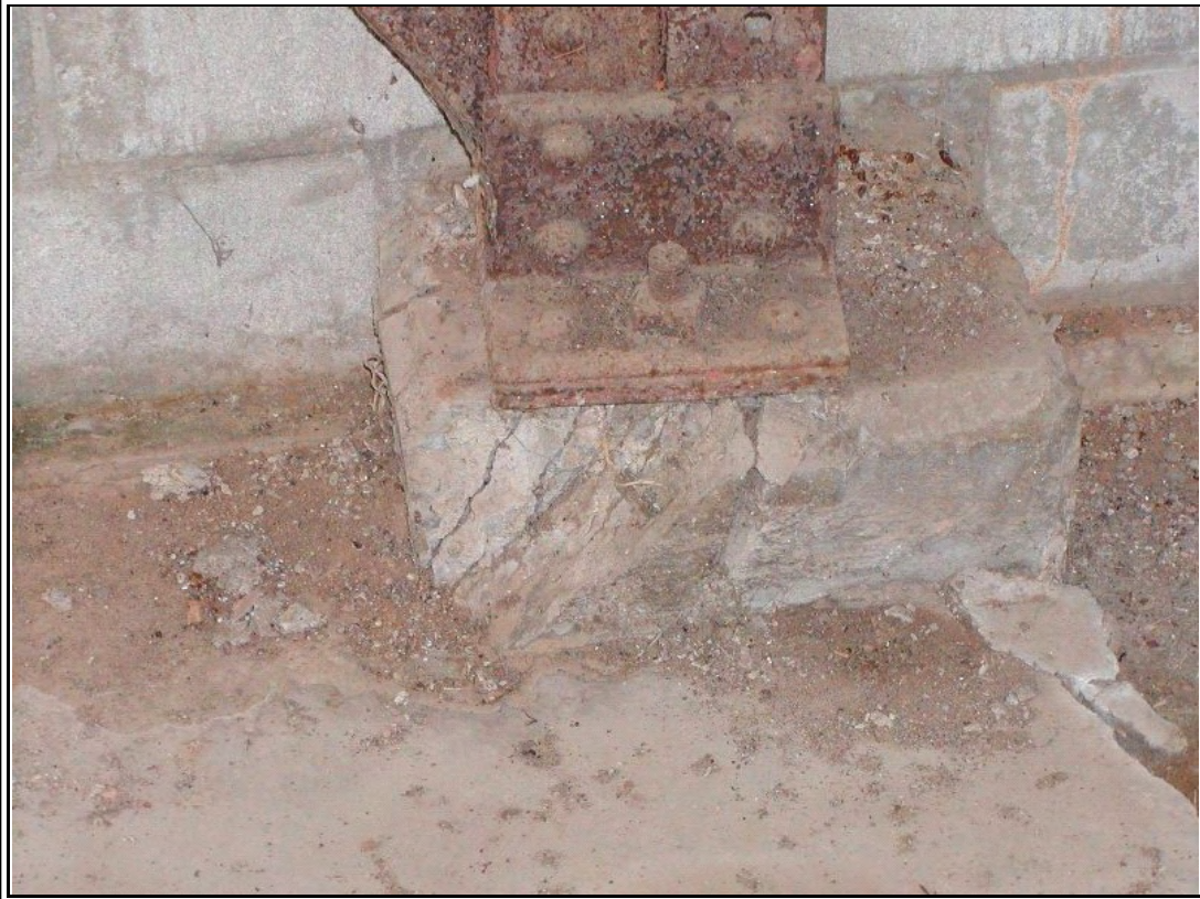
Photograph #: 8 Close-up of deteriorated column attachment at concrete pier
