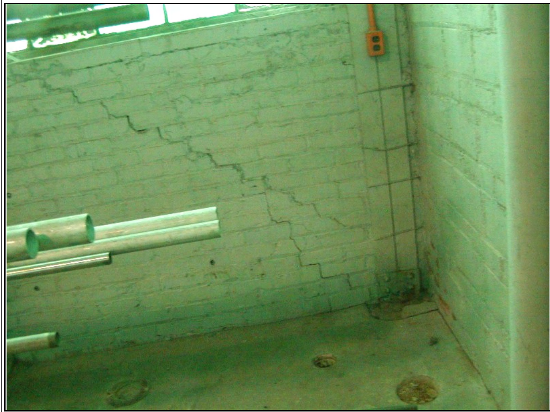
Photograph #: 12 Diagonal crack in masonry at corner of building below window
