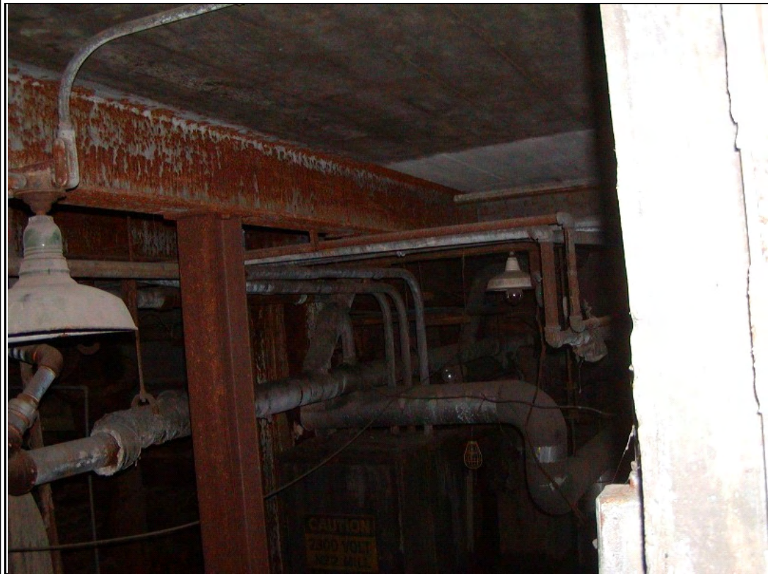
Photograph #: 13 Corroded steel framing in basement
