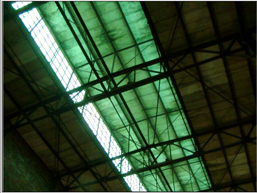
Photograph #: 14 Deteriorated concrete roof planks
