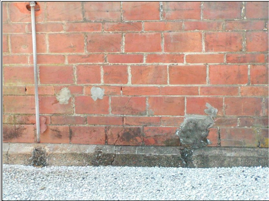
Photograph #: 9 Cracks in masonry and exposed slab edge on north side
