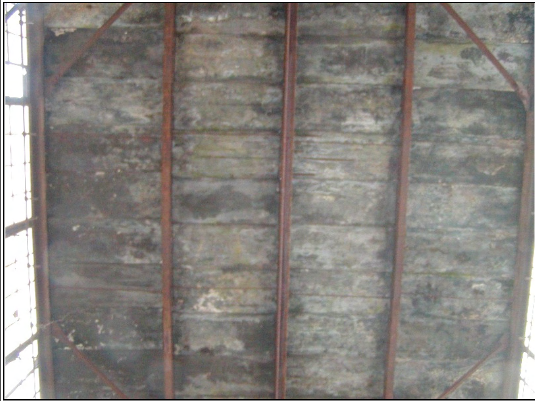
Photograph #: 8 Deteriorated concrete plank roof deck at monitor. Exposed reinforcing steel is visible.
