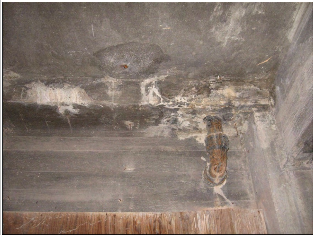
Photograph #: 20 Deterioration from water intrusion at mezzanine concrete frame
