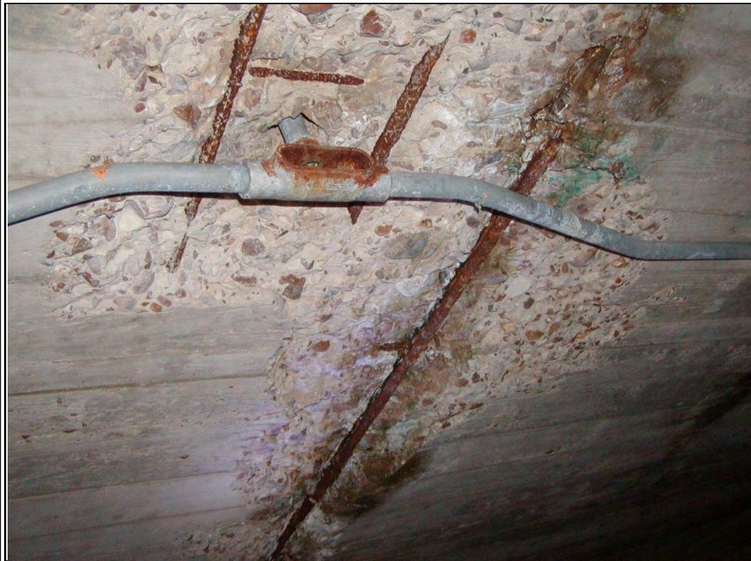
Photograph #: 17 Severely spalled concrete at basement ceiling
