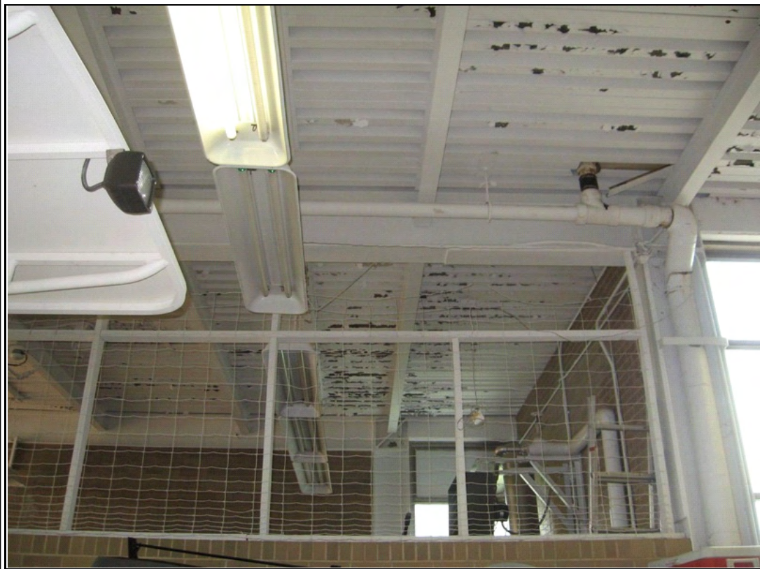
Photograph #: 15 Service Building - flaking paint at metal deck in vehicle storage area
