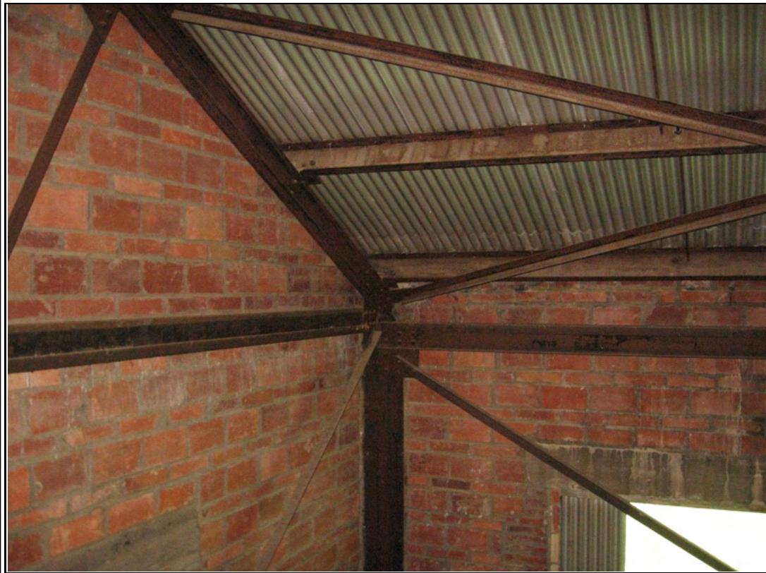
Photograph #: 15 Unpainted corroded steel framing below new metal roof deck
