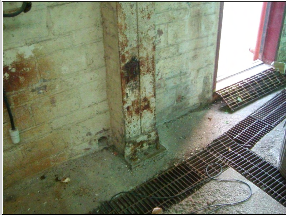
Photograph #: 14 Corroded steel column and deteriorated steel trench grates at south side of main building
