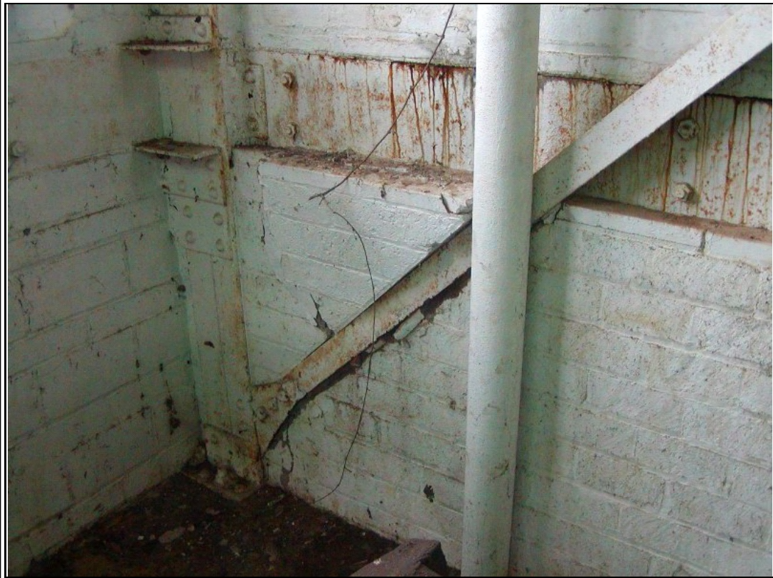
Photograph #: 12 Infill cracking and displacement at southeast corner
