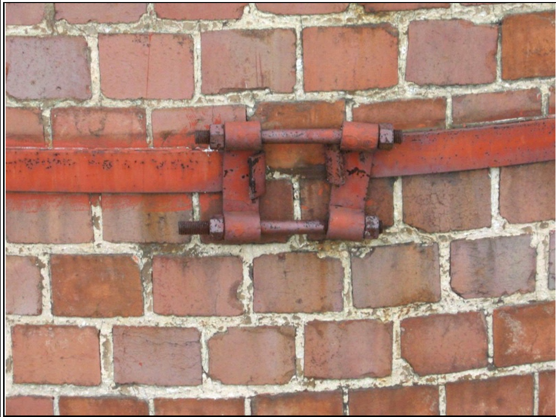
Photograph #: 19 Deteriorated steel coupling at smokestack
