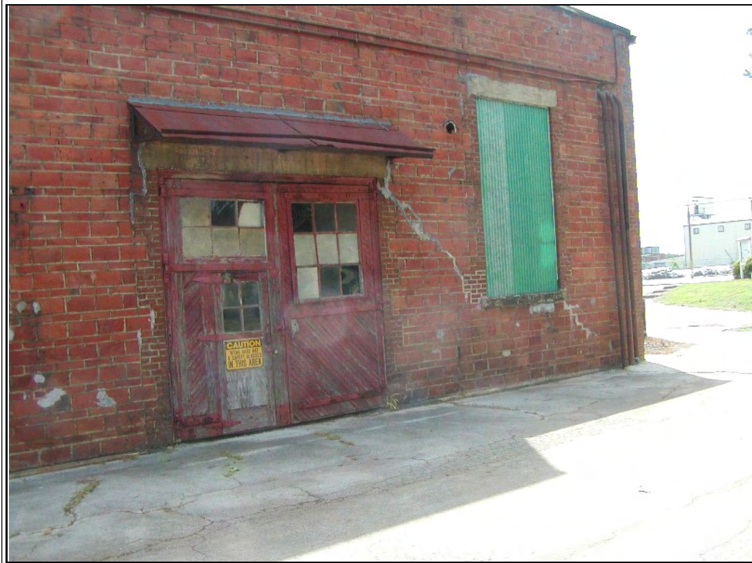
Photograph #: 4 Cracks in masonry south end of west wall
