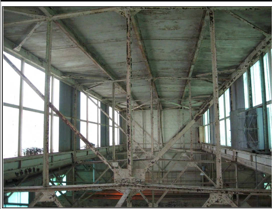
Photograph #: 15 View of monitor framing and roof deck
