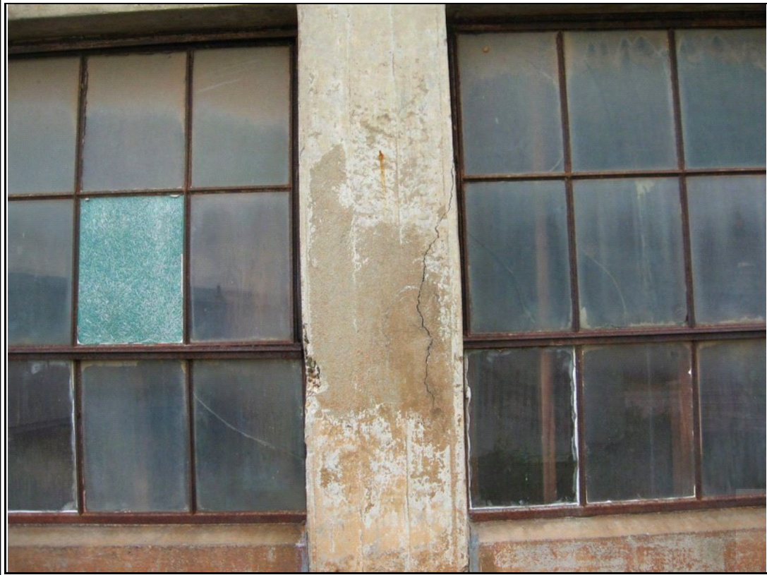
Photograph #: 4 Exterior crack in concrete mezzanine column.
