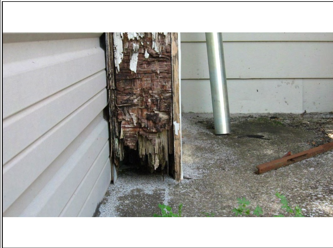
Photograph #: 2 Deteriorated structural supports at overhead door at south courtyard.
