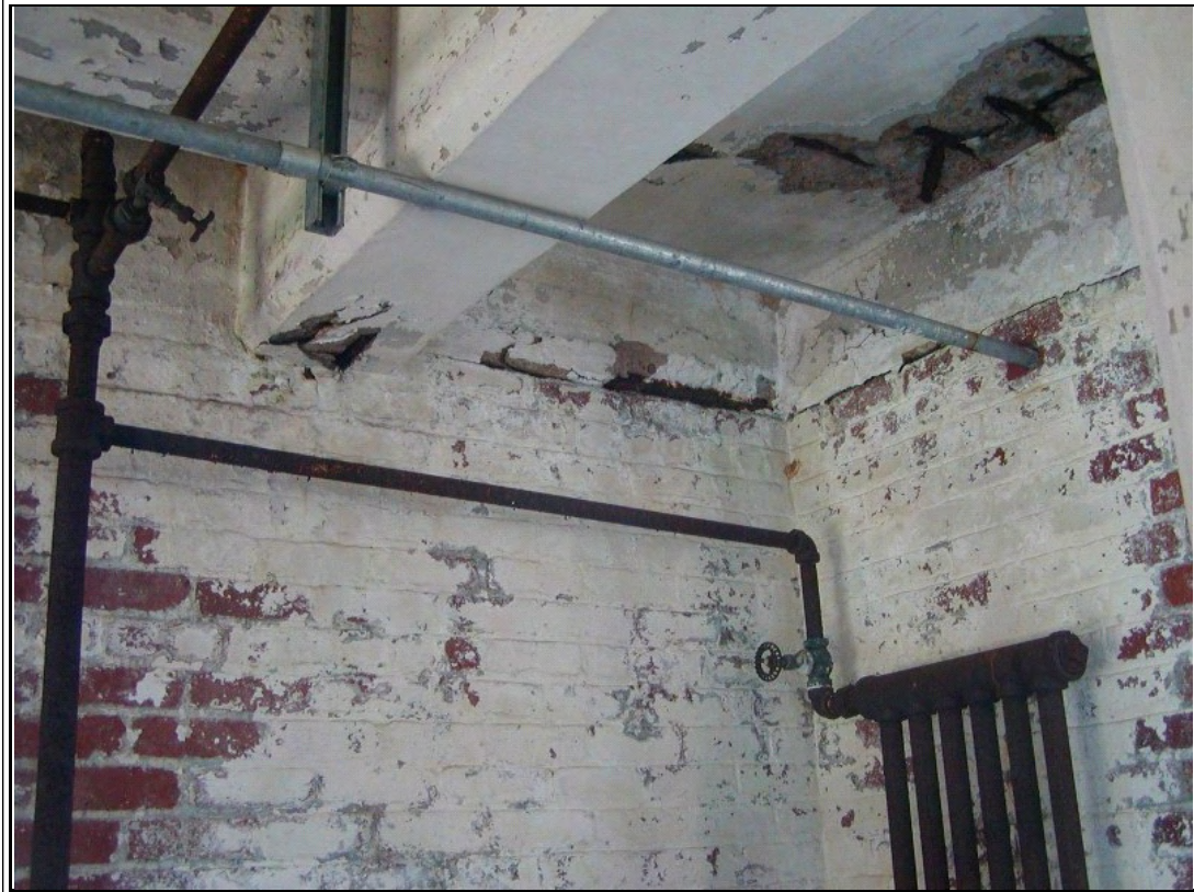
Photograph #: 15 Severe spalls in concrete at underside of upper floor
