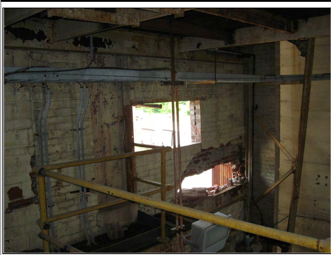
Photograph #: 21 View of collapsed brick infill from inside masonry building - note steel beam embedded in wall below collapsed masonry.
