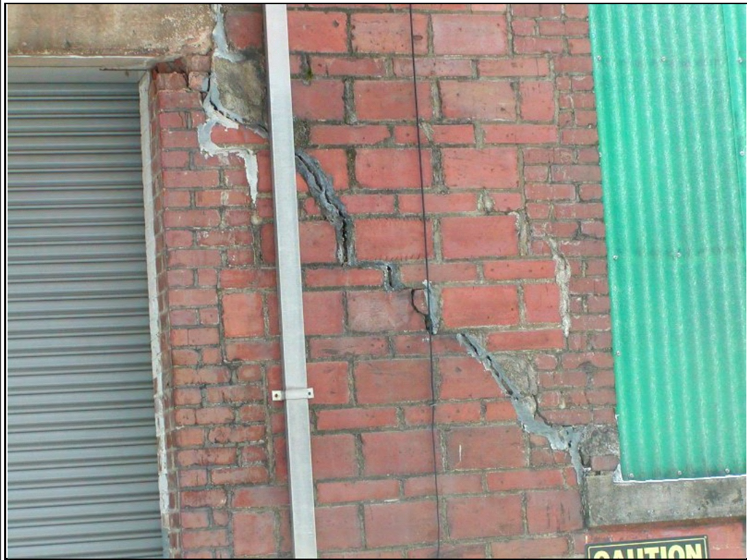
Photograph #: 13 Crack in masonry at north wall
