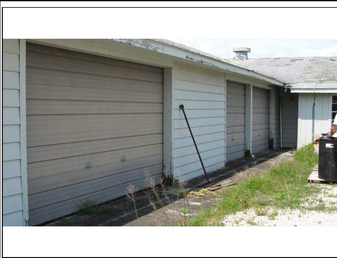
Photograph #: 1 Deteriorated structural supports between overhead doors at south courtyard.
