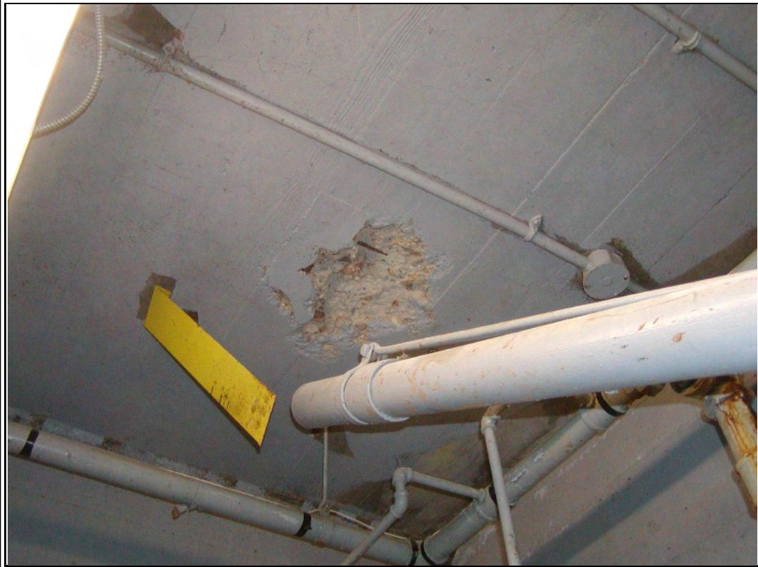
Photograph #: 7 Spall in soffit of floor slab above basement
