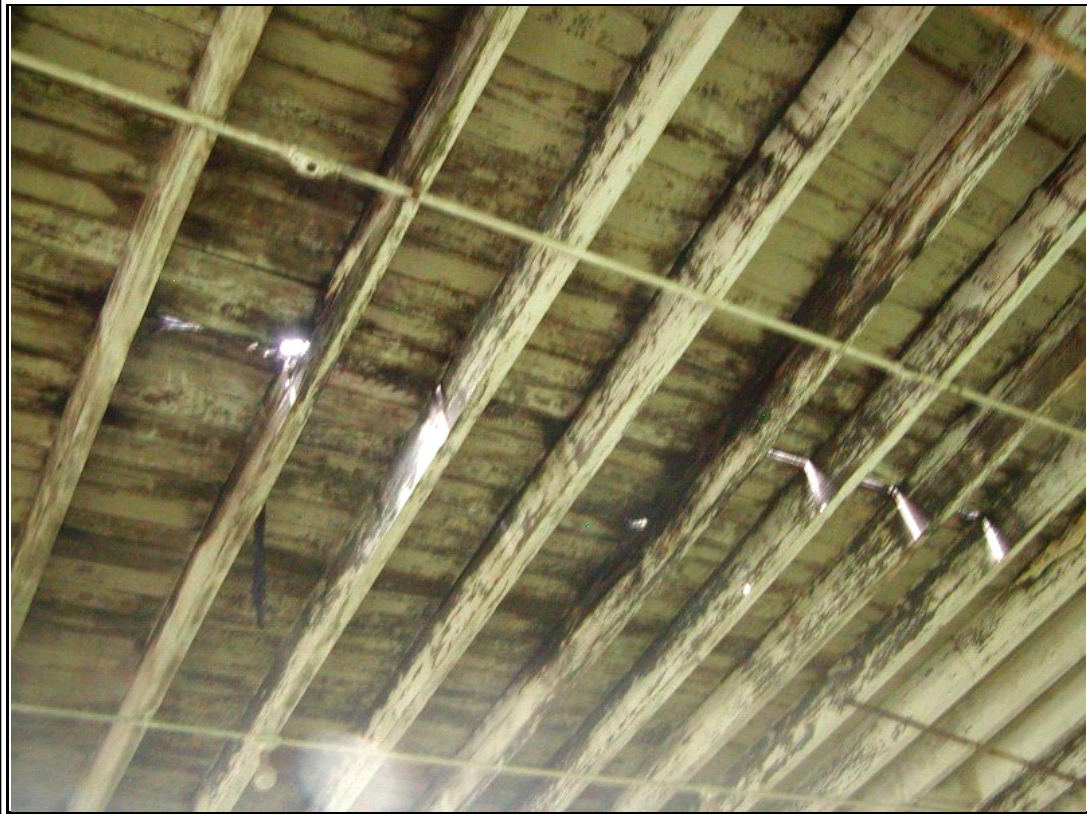
Photograph #: 3 Severely decayed wood roof structure with daylight visible through voids in wood plank deck.
