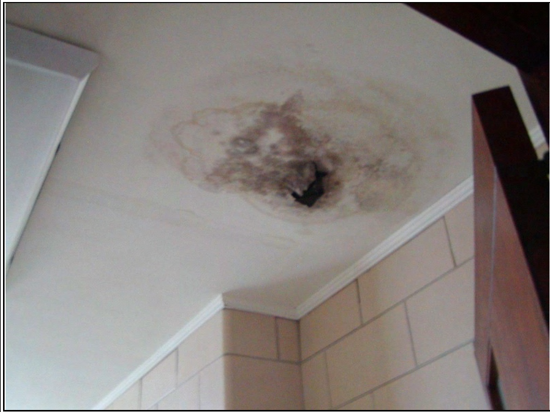
Photograph #: 14 Interior water intrusion damage
