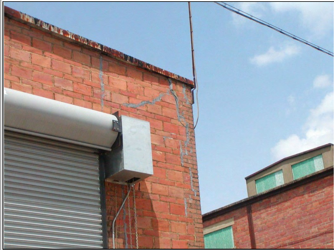
Photograph #: 10 Cracks in masonry north end of east wall
