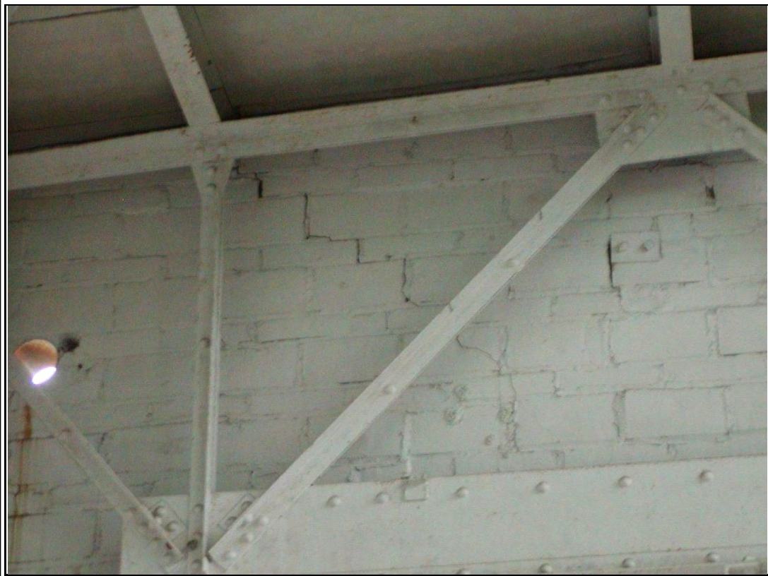
Photograph #: 11 Interior crack in masonry at east wall
