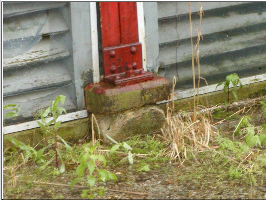
Photograph #: 5 Deteriorated concrete pier at column
