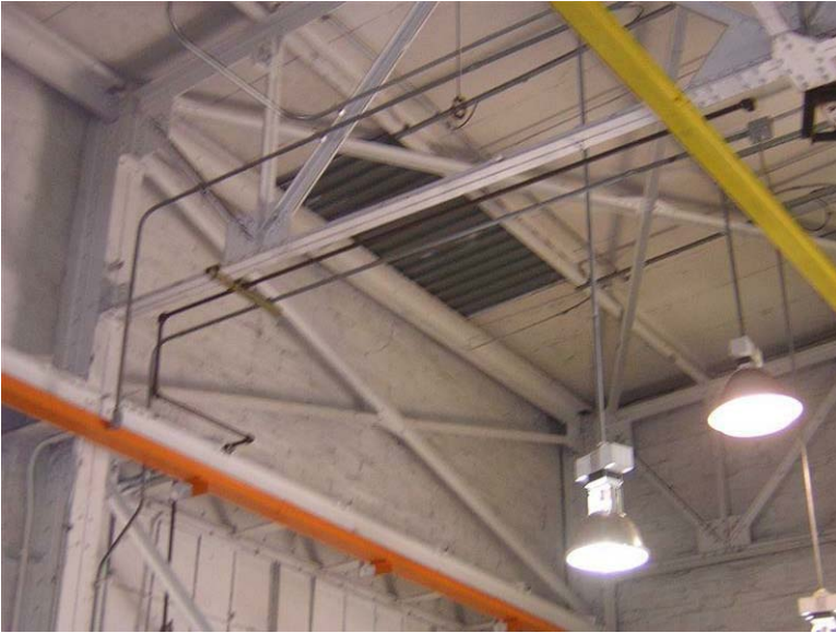
Building 41 – Sheet Metal Shop: Some of the concrete ceiling panels have been replaced with metal panels.
