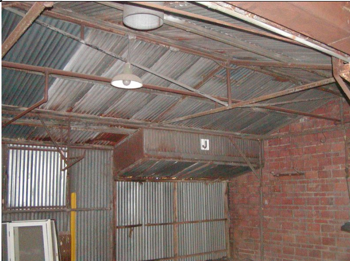
2009 Photo #8: Corroded metal roof deck and steel framing at East addition
