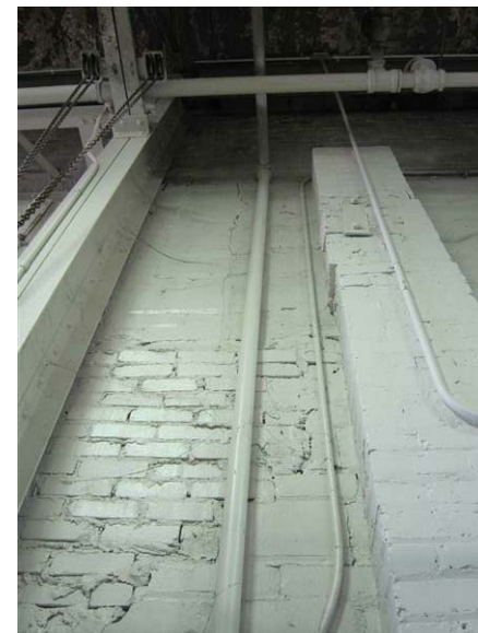
Building 38 – Machine Shop - Gas and Diesel Repair Shop: Although covered with paint, cracking is visible along the hollow clay tile wall.
