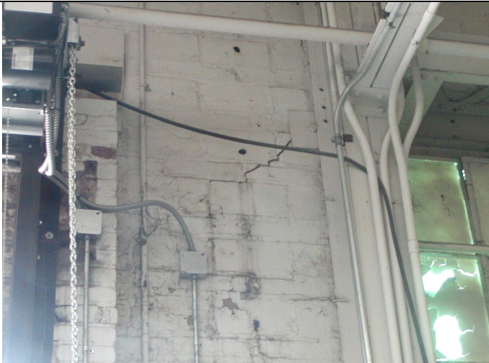
2009 Photo #24: Diagonal crack in masonry at South wall
