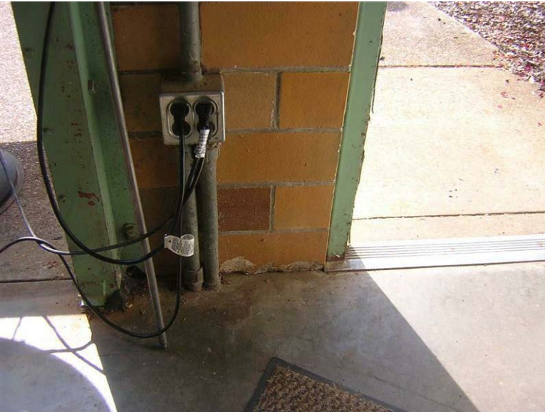
Building 118 – Greenhouse A: The glazed tiles are chipped at the base adjacent to the main entrance.
