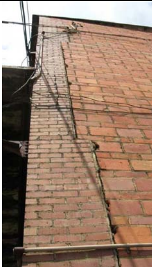
2009 Photo #22: Vertical crack in masonry on East side of Southeast corner.
