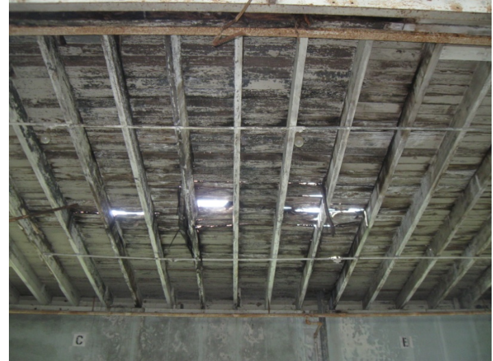
2013 Photo #3: More severely decayed wood roof structure with more daylight visible through voids in wood plank deck
