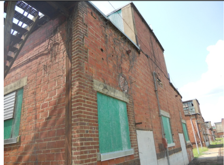
2013 Photo #2: SE corner of building. Vegetation covering portions of exterior walls is now dead, making masonry defects more visible.
