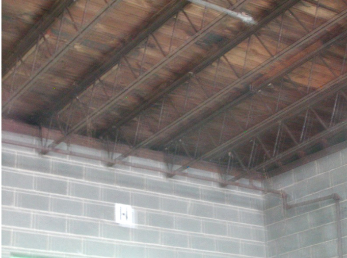
2009 Photo #7: Wood plank roof deck at East addition is damaged by water intrusion
