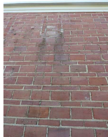
Building 25 – L / N Warehouse Z: Localized staining and efflorescence are visible on the wall.
