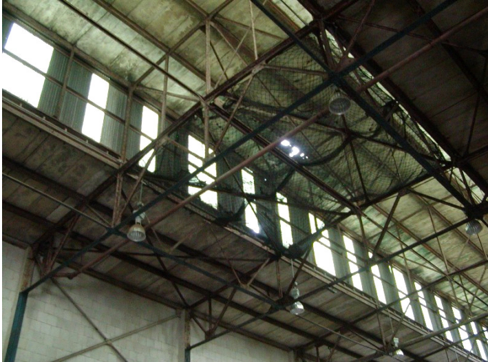
2009 Photo #5: Holes in deteriorated concrete plank roof deck
