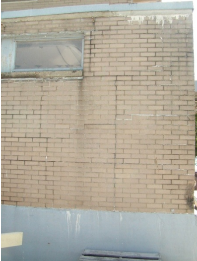
2009 Photo #3: Cracks in masonry on North side
