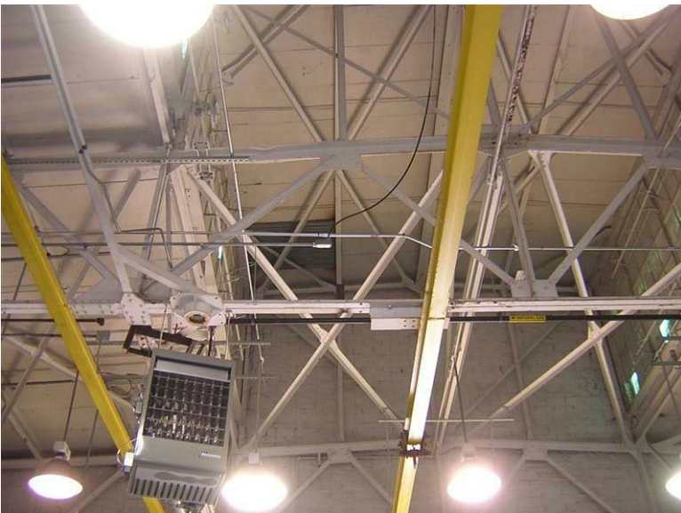
Building 41 – Sheet Metal Shop: Although the steel truss system is painted, rusting occurs and paint is flaking.
