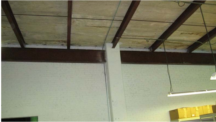
2009 Photo #39: Spalls and surface deterioration at concrete roof planks at interior wall.
