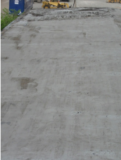
2009 Photo #7: View of building roof membrane in fair condition
