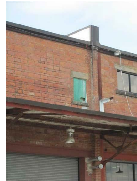
Building 33, 34, 35, 36 – Chemical Plant Warehouse: Tops of the brick buttresses are failing.
