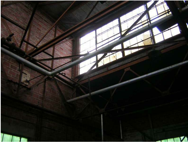
Building 69 – Catalyzer Building No. 1: The steel structure is rusted.
