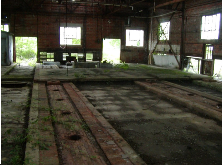
2009 Photo #11: Irregular, deteriorated floor system in main building
