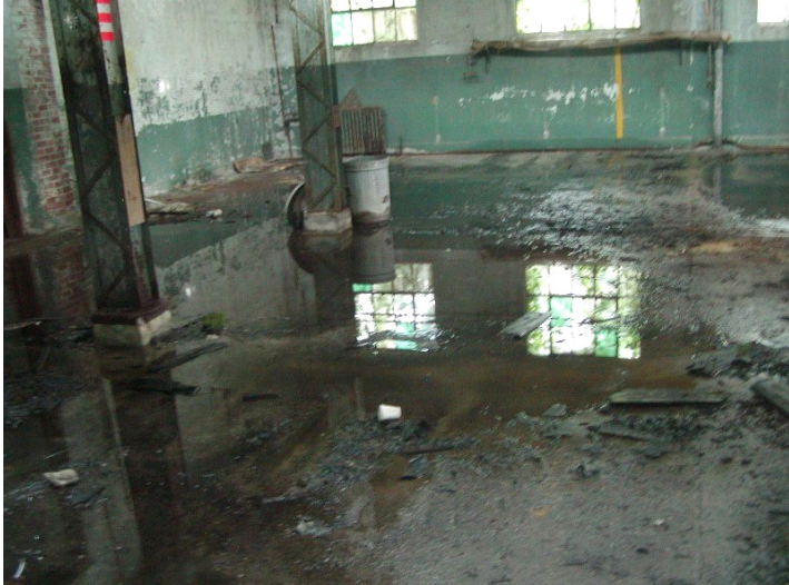
2009 Photo #5: Standing water on floor inside building; corroded steel columns
