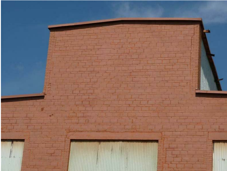
Building 39 – Engineering Lab: Cracking is visible at the hollow clay tile and brick quoins on the upper wall.
