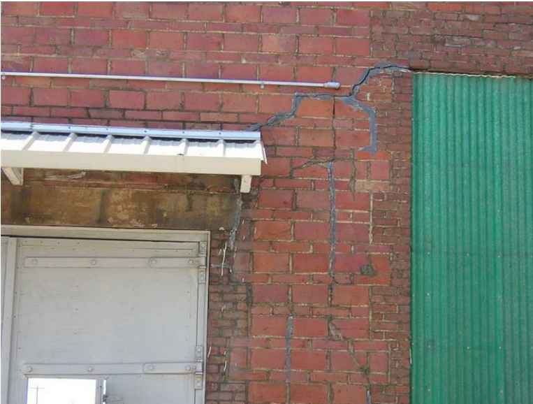
Building 42 – Pipe Shop: Severe cracking is visible on the south wall especially above windows and between openings. Some cracks have been sealed with a material incompatible with the mortar.
