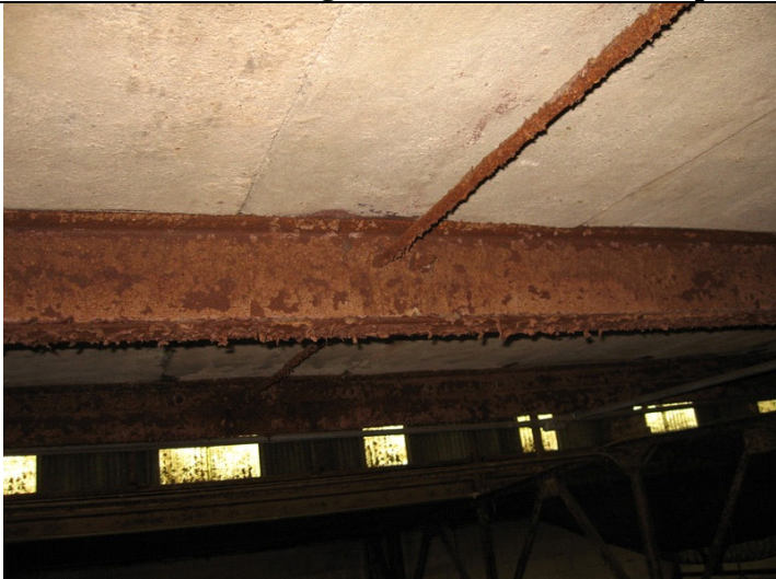
2009 Photo #9: Severely corroded steel framing
