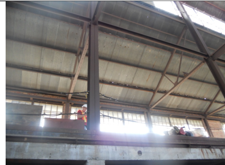
2013 Photo #8: More holes and more corrosion were observed on underside of metal roof deck
