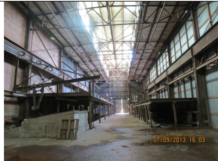
2013 Photo #4: Steel and wood mezzanines at building interior
