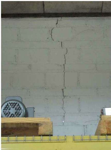
Building 36 – Chemical Plant Warehouse - Projects Operations Storage Warehouse: A large horizontal crack penetrates the hollow clay tile.
