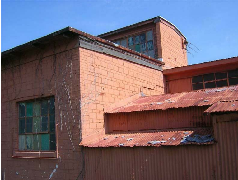
Building 53 – Tin Shop: The wood fascia board is in poor condition and the metal roof is rusted.
