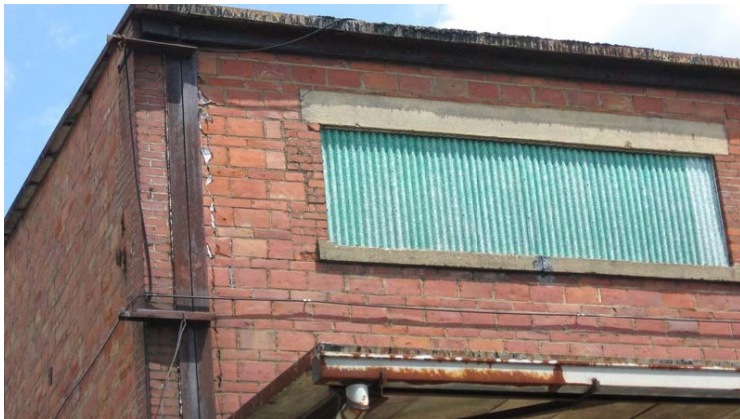
2009 Photo #14: Cracks in exterior masonry on South side Southwest corner.
