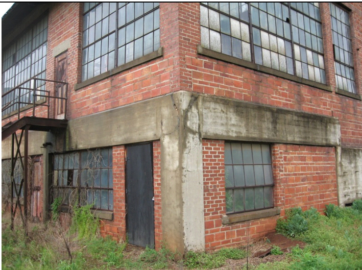
2009 Photo #2: Exterior cracks in concrete mezzanine frame at Southwest corner
