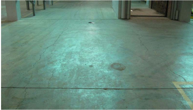
2009 Photo #31: Cracks in East area of second floor slab.
