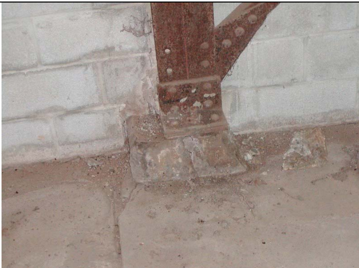
2009 Photo #10: Deteriorated concrete pier at column
