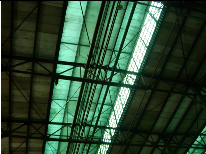
2009 Photo #15: Deteriorated concrete roof planks
