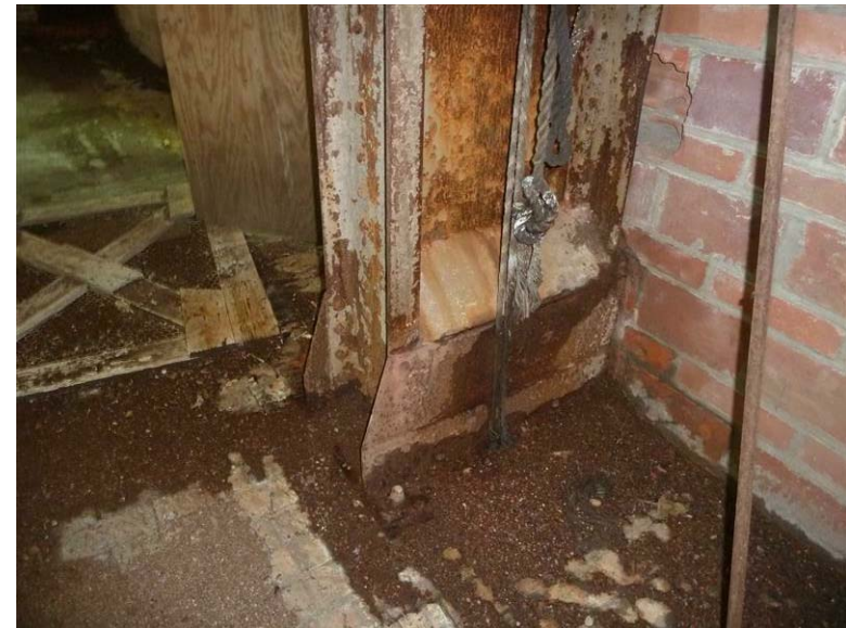
Building 24 – Warehouse No. 4: The steel column is severely rusted.
