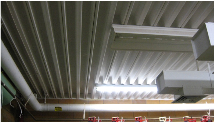
2009 Photo #8: Metal roof deck at lab building in generally good condition
