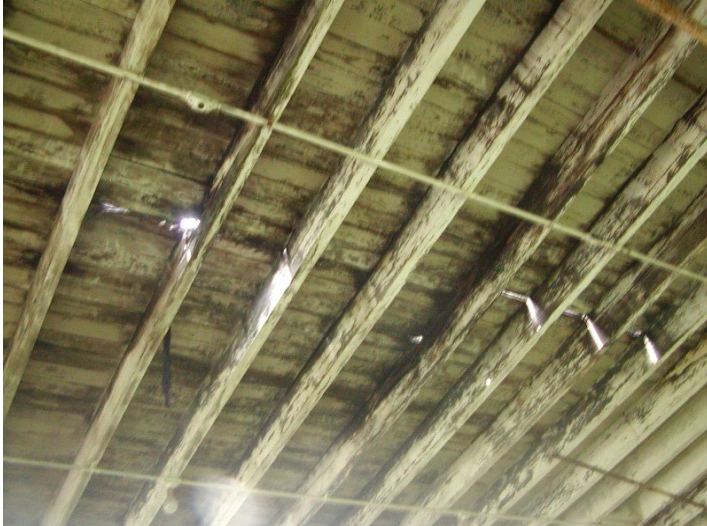
2009 Photo #3: Severely decayed wood roof structure with daylight visible through voids in wood plank deck
