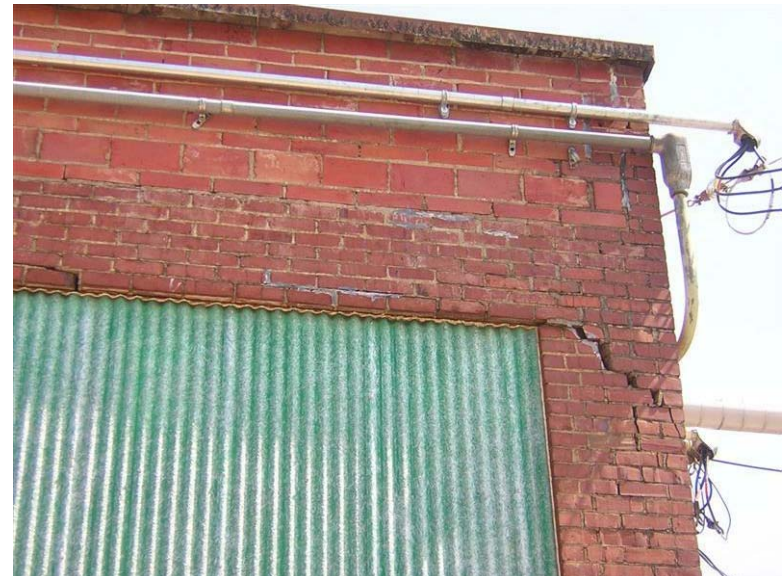
Building 42 – Pipe Shop: There is severe cracking of the brick at the southeast corner of the building.
