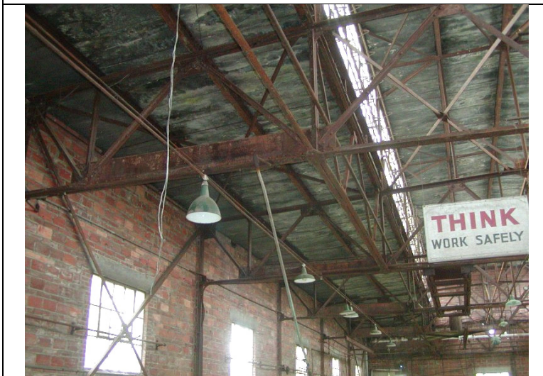
2009 Photo #6: Corroded steel framing and deteriorated concrete plank roof deck
