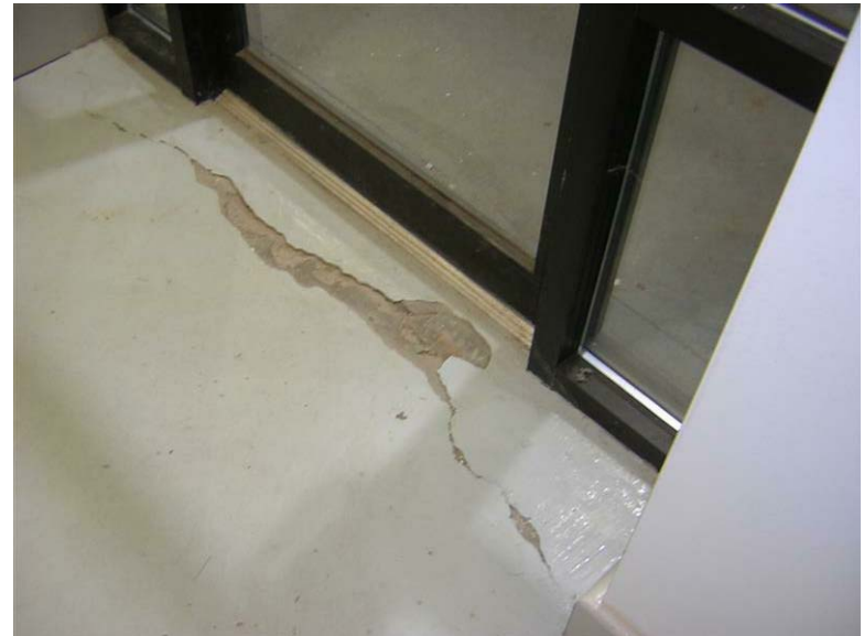
Building 44 – Project Operations Bath House: The concrete floor is cracked at the west entrance.
