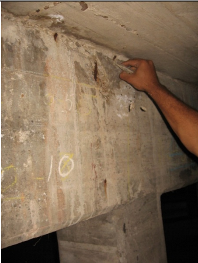
2009 Photo #20: Spalled concrete at basement structure
