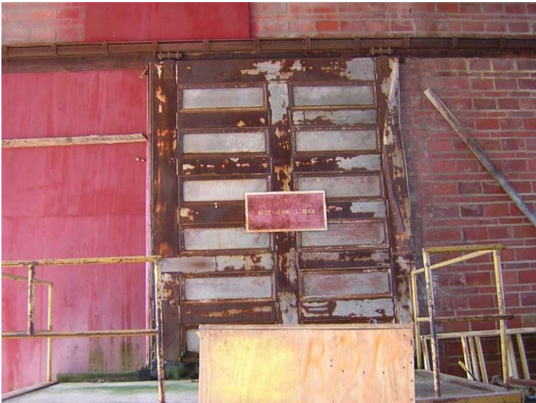
Building 81 – 5A – Nitrate House: The exterior doors are rusted.
