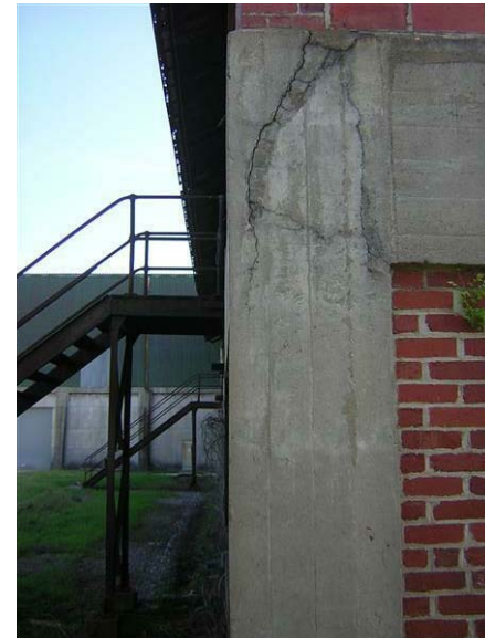
Building 81 – 5A – Nitrate House: Localized cracking is visible in the concrete structure.
