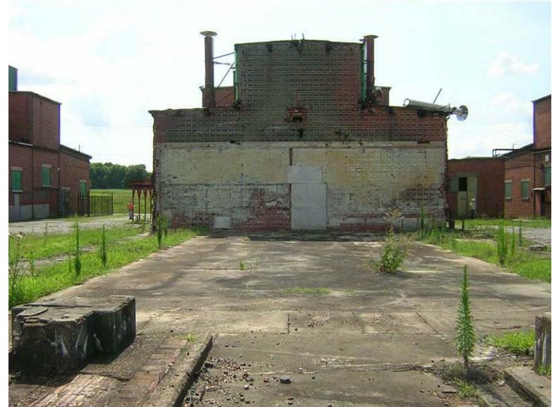
Building 70 – Catalyzer Building No. 2: The rear of the building was damaged in a fire and has been demolished.
