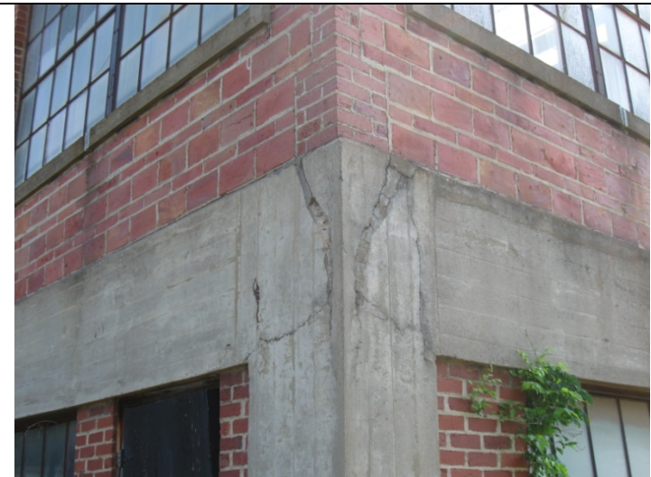
2013 Photo #2: Exterior cracks in concrete mezzanine frame at Southwest corner exhibit progressive deterioration
