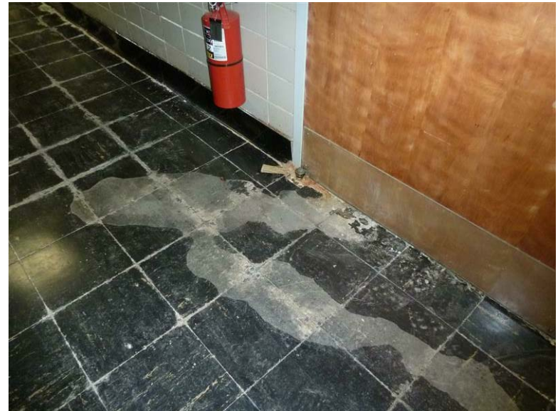
Building 17A - Environmental Research Center: Water damage is visible on the floor tiles adjacent to this mechanical room.
