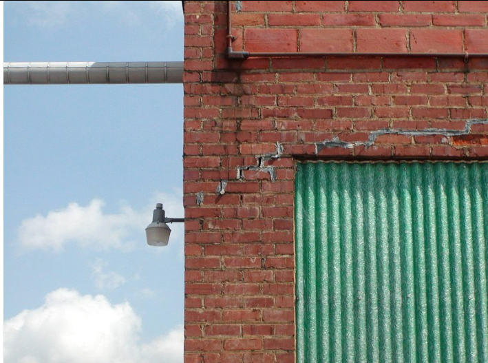
2009 Photo #5: Horizontal crack in masonry at Southwest corner
