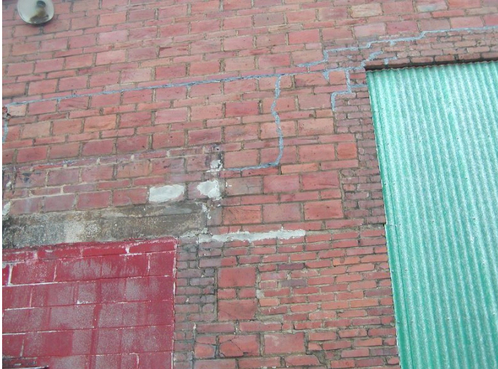
2009 Photo #7: Cracks in masonry in South wall
