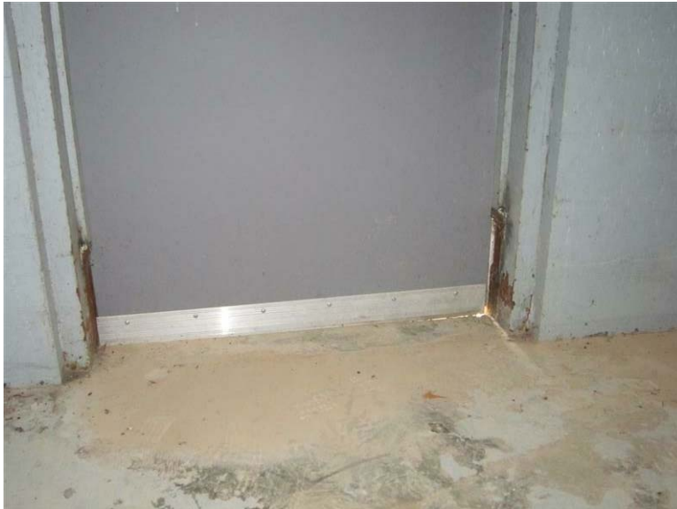
Building 01A - Chemical Feed House: The jambs of the exterior door are badly rusted.
