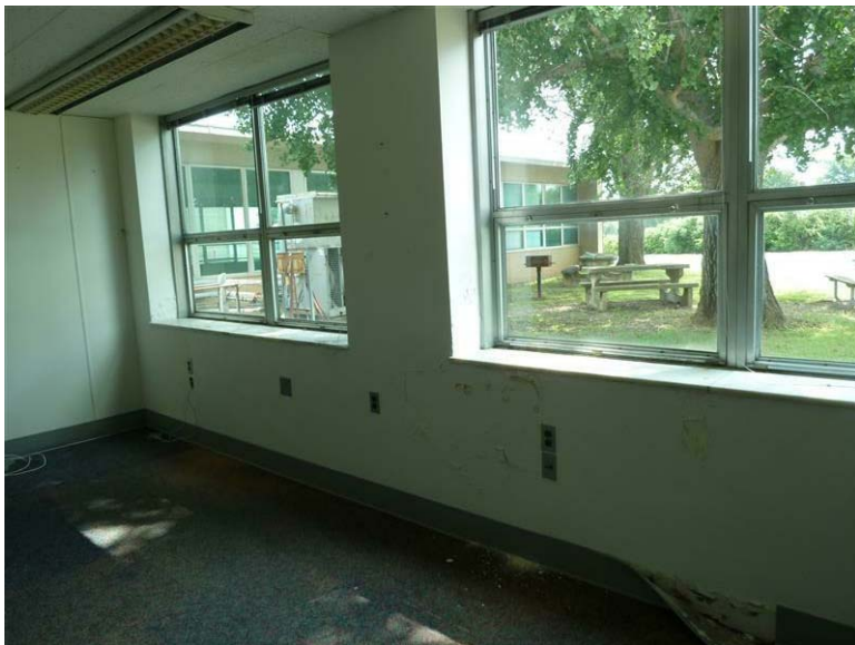
17B - Service Building: Damage to interior finishes due to moisture in the space.
