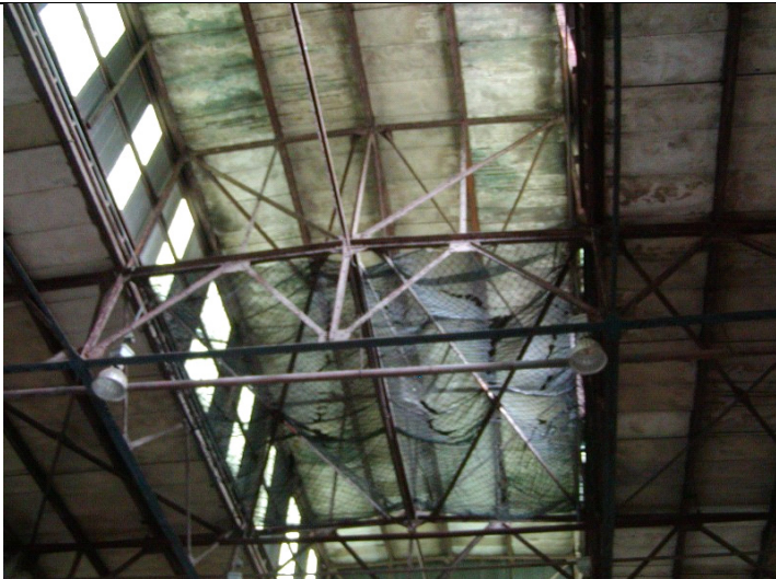
2009 Photo #4: Deteriorated concrete plank roof deck
