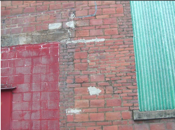
2009 Photo #8: Cracks in masonry (Same locations as Photo No. 7)
