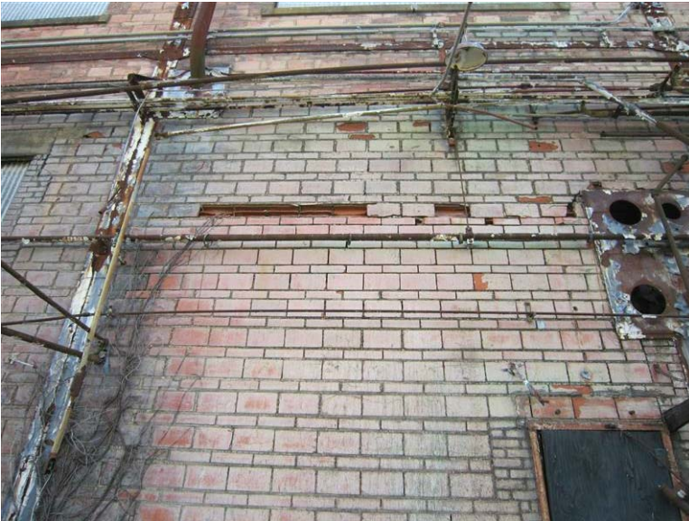
Building 22, 23 – L / N Building: Localized spalled and broken hollow clay tile and rusted steel are prevalent.
