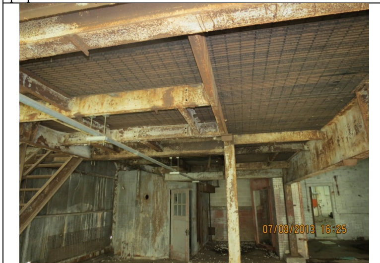
2013 Photo #23: Severely corroded steel framing at west end of structure.
