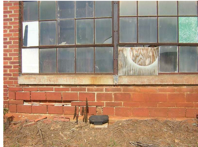
Building 81 – 5A – Nitrate House: Hollow clay tile and window panes are broken. The window has been partially covered with plywood.
