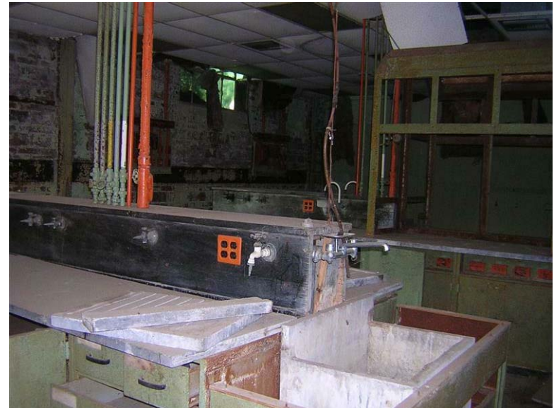
Building 69 – Catalyzer Building No. 1: Acoustical ceiling tiles are missing.
