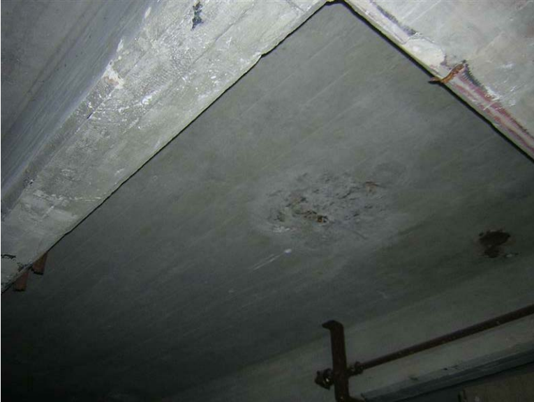
Building 79 – 3A – Nitrate House: Rebar is exposed at the underside of the mezzanine floor.
