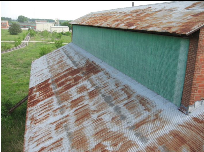
2009 Photo #8: Deteriorated metal roof on West side
