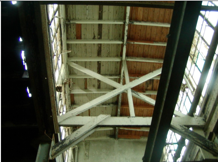
2009 Photo #6: Partially repaired roof deck at clerestory monitor
