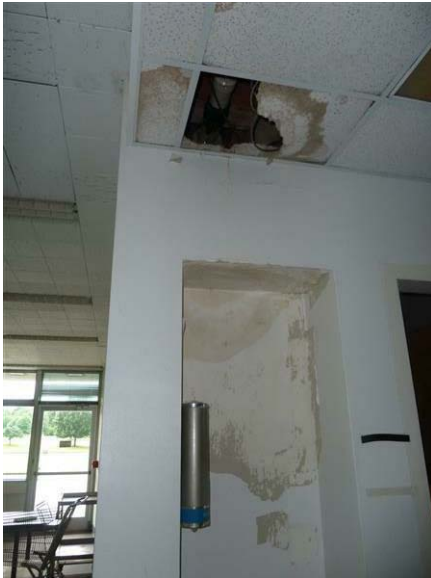
17B - Service Building: The ceiling and wall are damaged from water infiltration adjacent to the water fountain.
