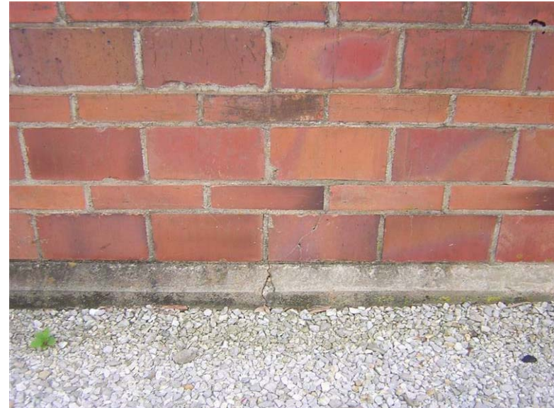
Building 44 – Project Operations Bath House: The concrete foundation is cracked in several areas.
