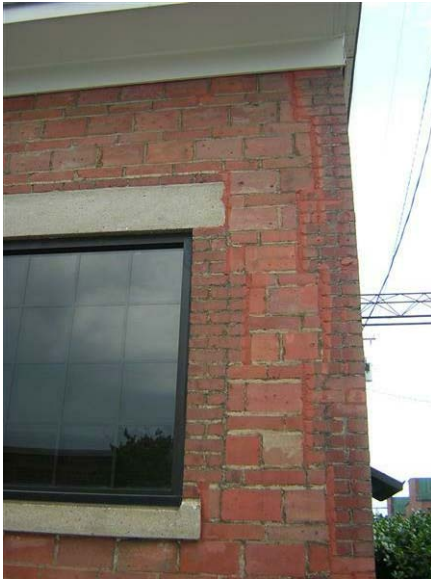
Building 44 – Project Operations Bath House: The cracks along the quoins have been infilled with red mortar.
