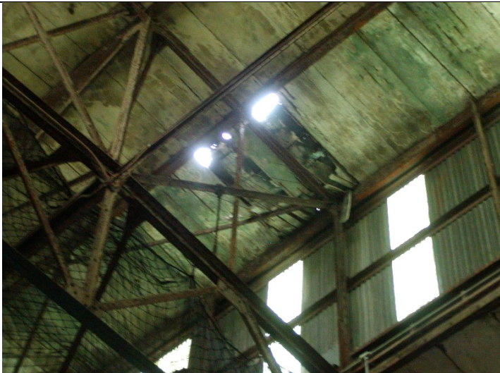
2009 Photo #6: Areas of ruined concrete plank roof deck
