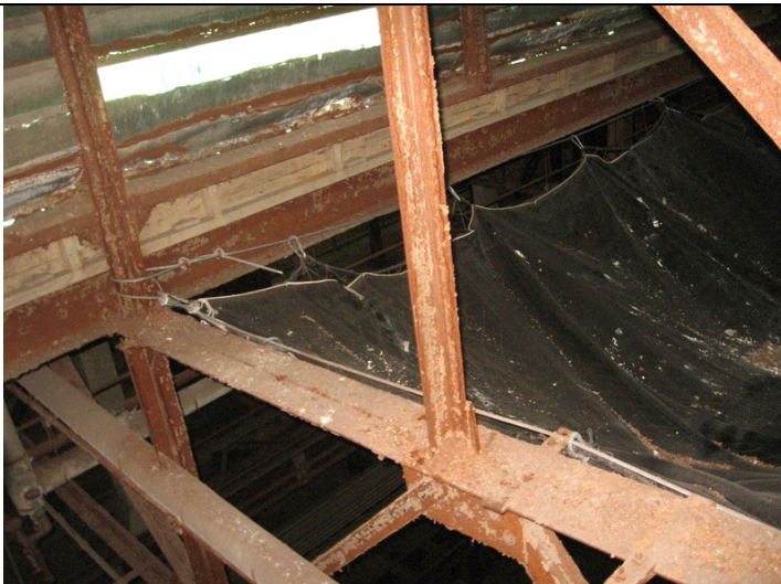
2009 Photo #12: Severely corroded structural steel
