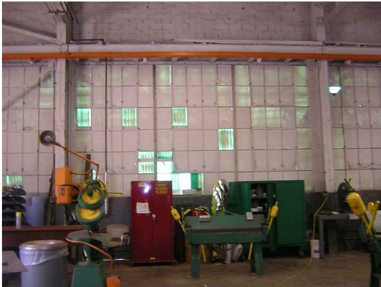
Building 41 – Sheet Metal Shop: Glass panes are missing in many windows. The exterior of the windows are covered with fiberglass panels.
