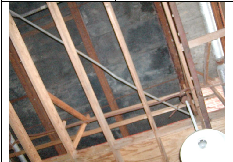
2009 Photo #10: Corroded steel framing and deteriorated roof deck at low roof
