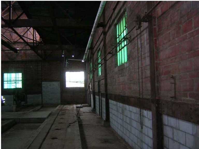
Building 74 – Catalyzer Building No. 6: The exposed steel is rusted.
