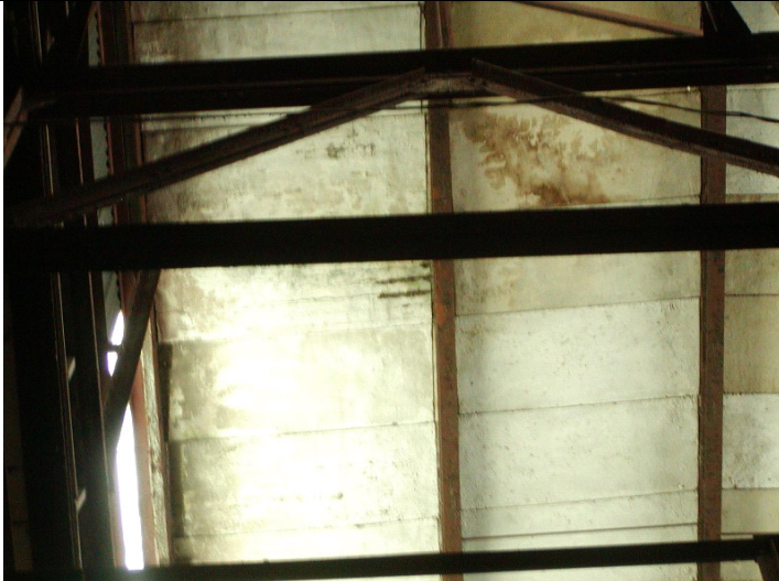
2009 Photo #7: Structurally deficient concrete roof plank
