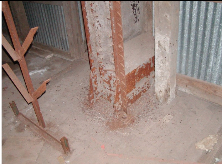
2009 Photo #10: Severely corroded steel column
