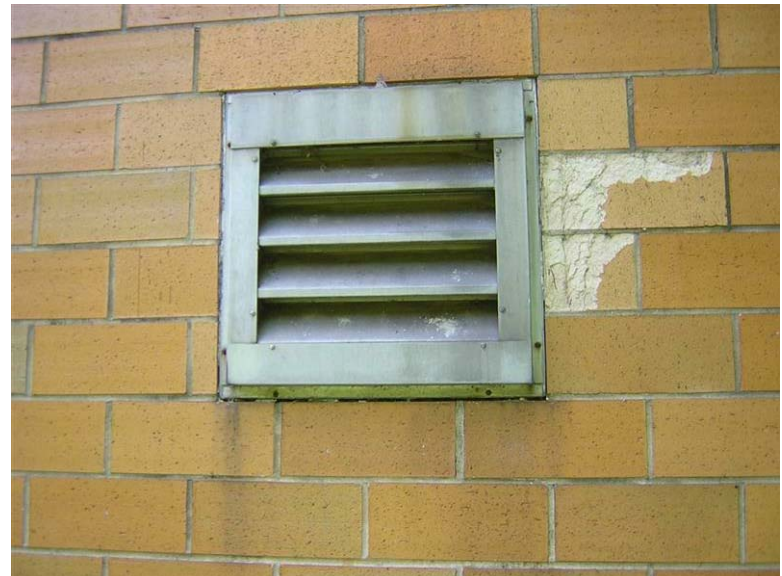
Building 118 – Greenhouse A: The glazed tiles have spalled adjacent to the vent opening.
