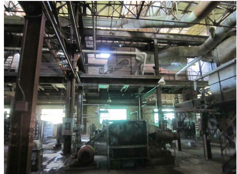
Building 22, 23 – L / N Building: Probable asbestos pipe wrap is present in the building.
