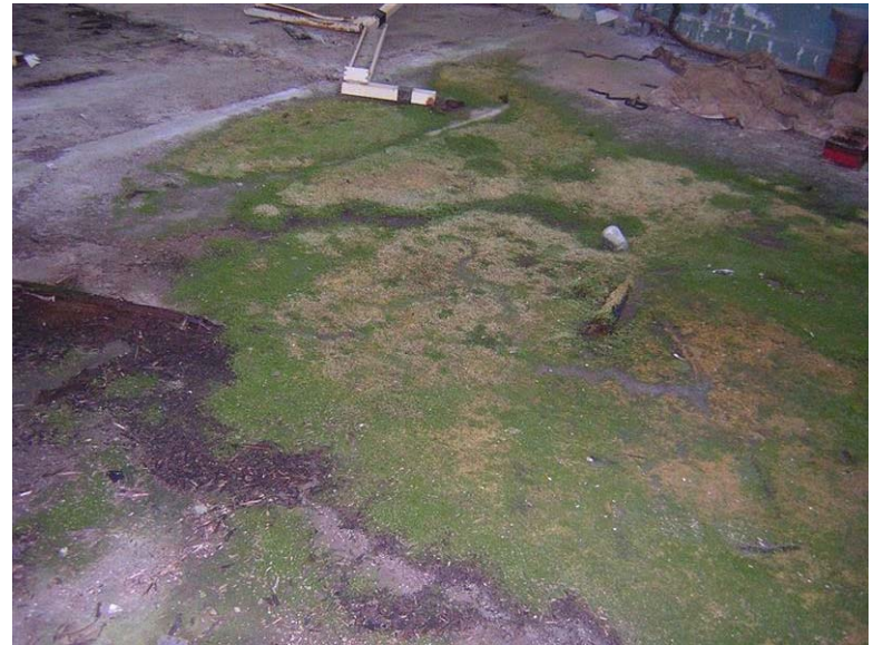
Building 53 – Tin Shop: Moss growth is prevalent on the concrete floor in the primary space.
