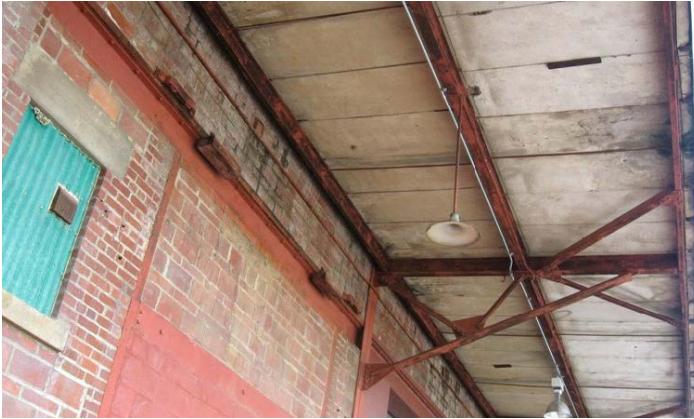
2009 Photo #5: Deteriorated concrete roof planks at North canopy.
