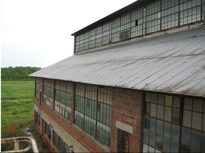
2009 Photo #5: Deteriorated metal roof on East side
