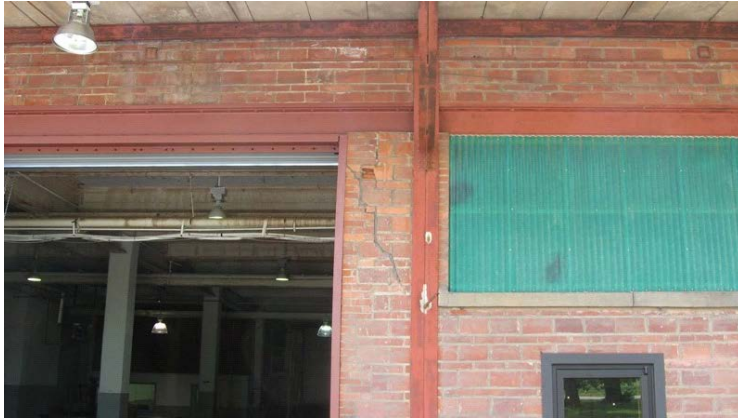
2009 Photo #9: Cracks in exterior masonry below North canopy.
