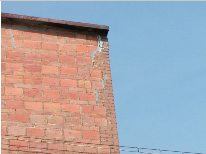
2009 Photo #6: Cracks in masonry at Northeast corner
