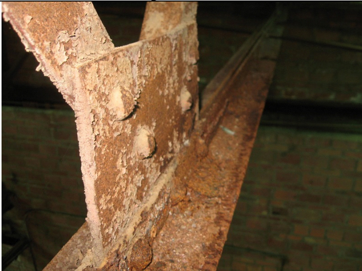
2009 Photo #5: Severely corroded steel framing
