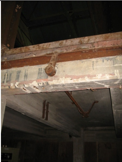
2009 Photo #26: Damaged mezzanine concrete beam
