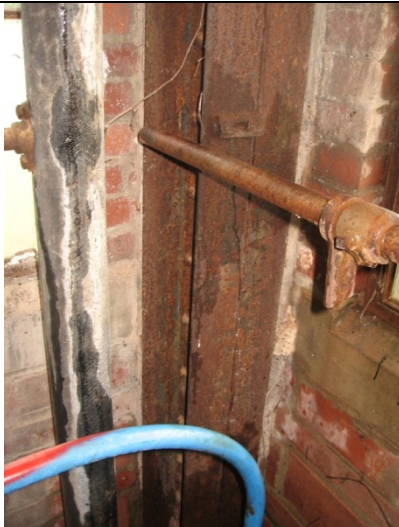
2009 Photo #16: Corroded steel column
