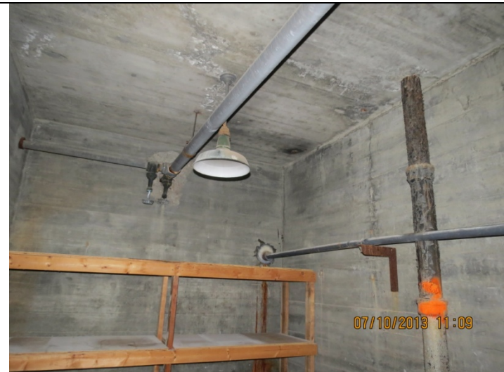
2013 Photo #8: Evidence of water intrusion at basement wall and ceiling. Intrusion appears to be worse than previously reported.
