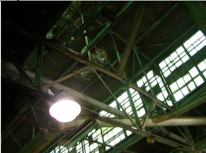
2009 Photo #20: Deteriorated concrete plank roof deck at monitor
