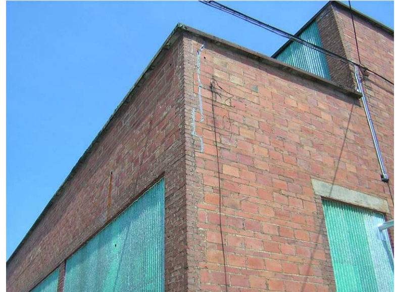
Building 41 – Sheet Metal Shop: Cracking is visible in the hollow clay tile and brick quoins located at the upper corners of the building.
