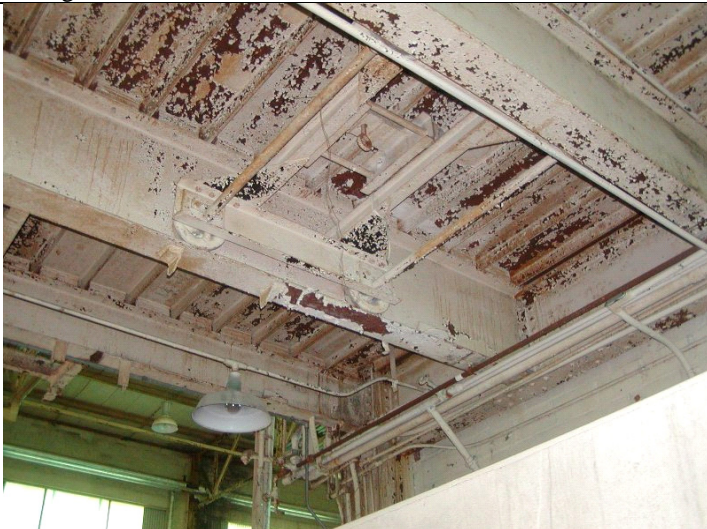
2009 Photo #12: Corroded steel below second floor at Southwest corner
