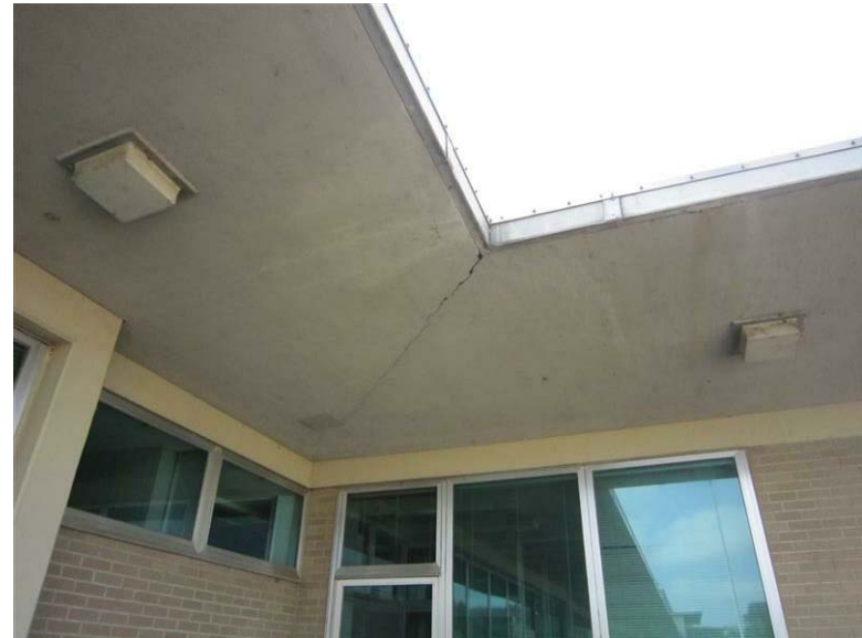
17B - Service Building: The concrete overhang is cracked at the interior corner.
