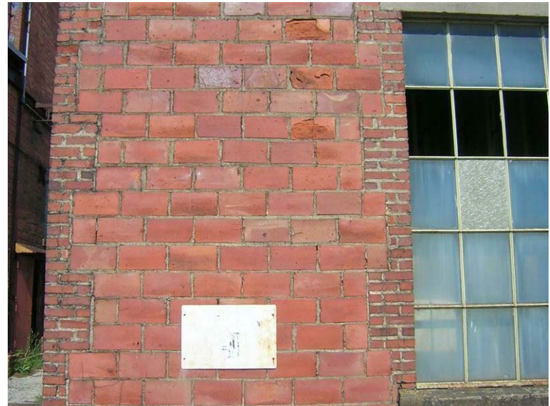
Building 68 – Substation No. 4: Hollow clay tile is spalling on the west facade. Several window panes are broken.
