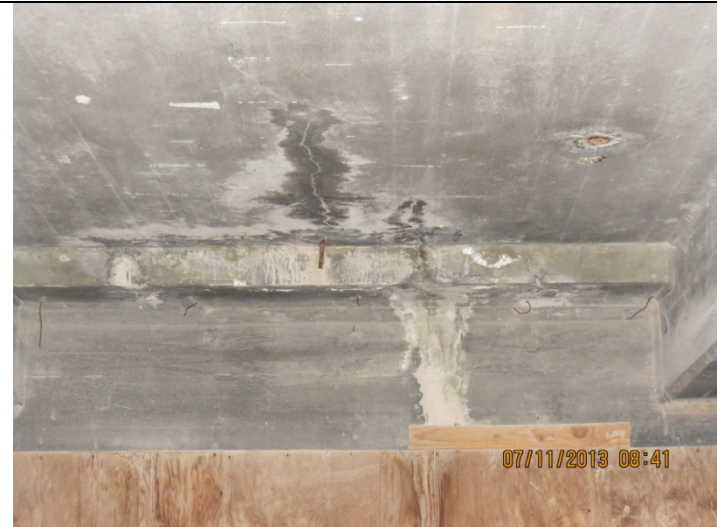
2013 Photo #20: Additional deterioration from water intrusion at mezzanine concrete frame was observed
