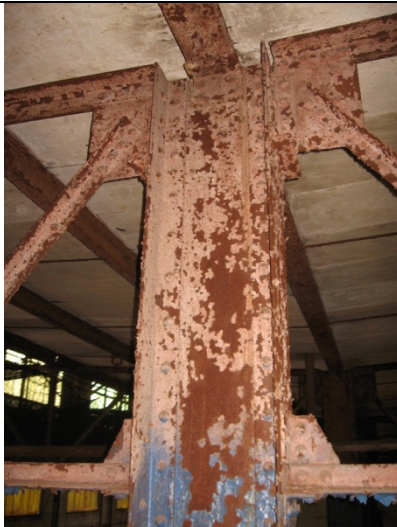
2009 Photo #8: Severely corroded steel framing
