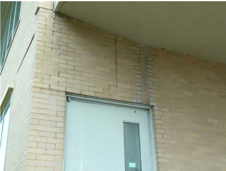
Building 17A - Environmental Research Center : The brick facade has shifted where the awning connects to the building at the southeast corner of this wing.
