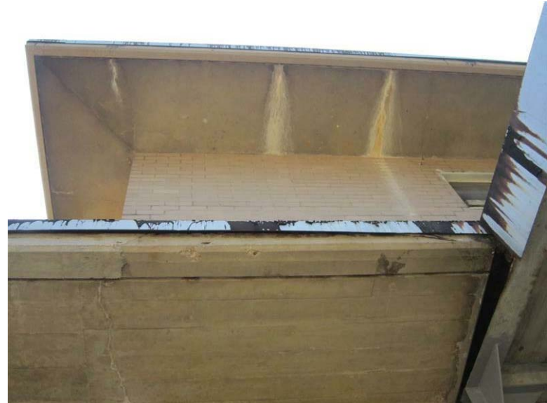
Building 01A - Chemical Feed House: The metal copings have failed and are rusted. There is cracking and staining at the concrete overhangs.
