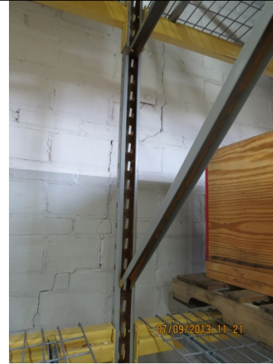
2013 Photo #37: Interior crack in East wall. Crack continues to perpetuate since 2009.
