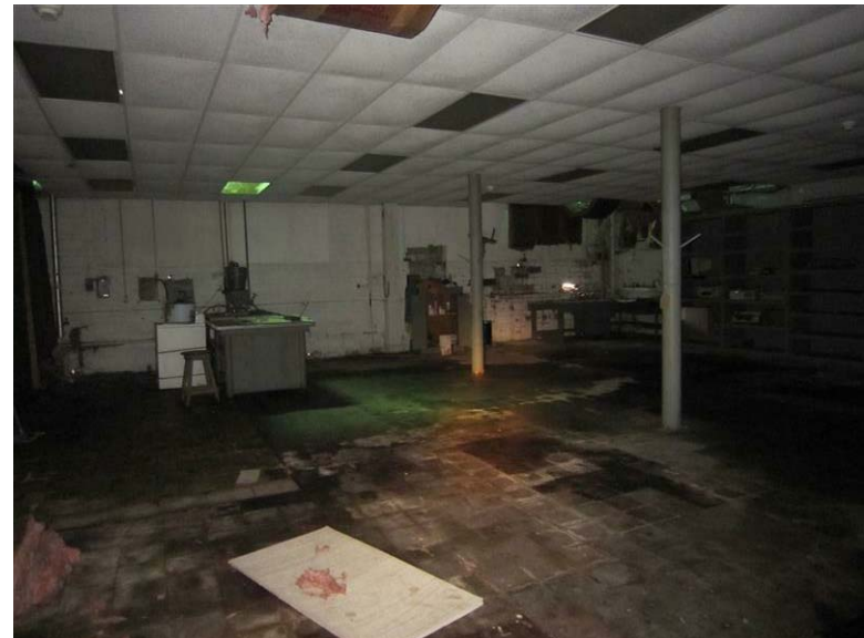
Building 26 – L / N Building Grounds Maintenance Shop: Considerable water damage, mold growth and possible asbestos containing floor tiles are present in the secondary space.
