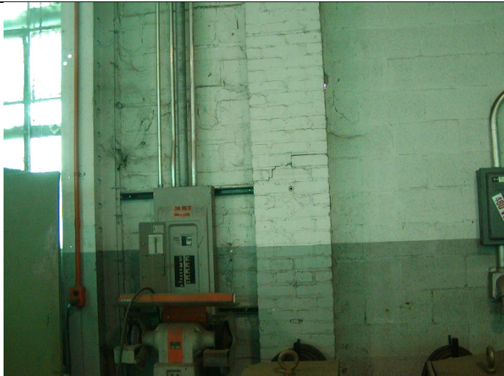
2009 Photo #10: Horizontal crack in brick pier
