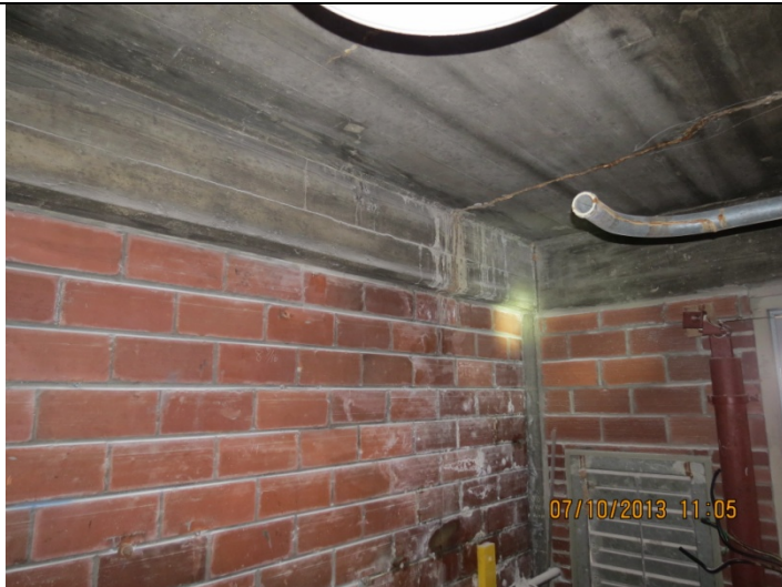
2013 Photo #11: Crack in roof slab runs across entire width of room; Efflorescence present; horizontal beam cracked
