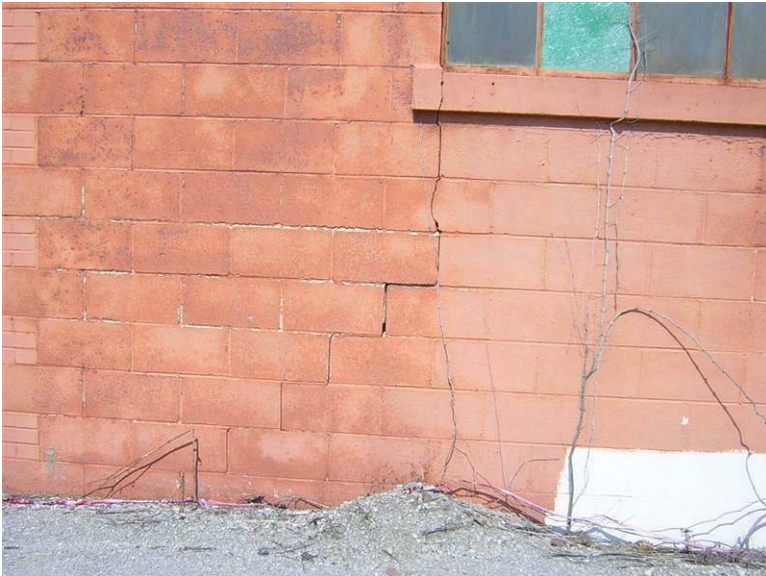
Building 53 – Tin Shop: Diagonal cracking is located beneath this window on the south facade.
