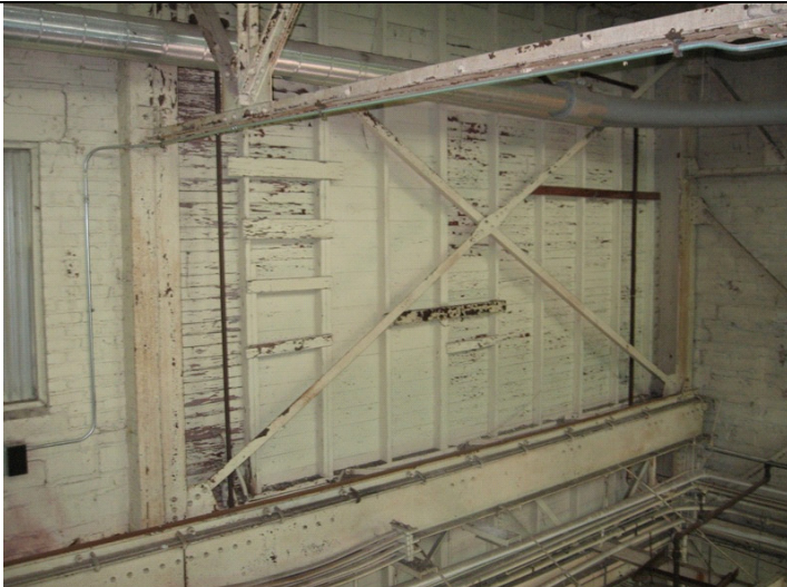
2009 Photo #18: Wood frame interior wall at second floor
