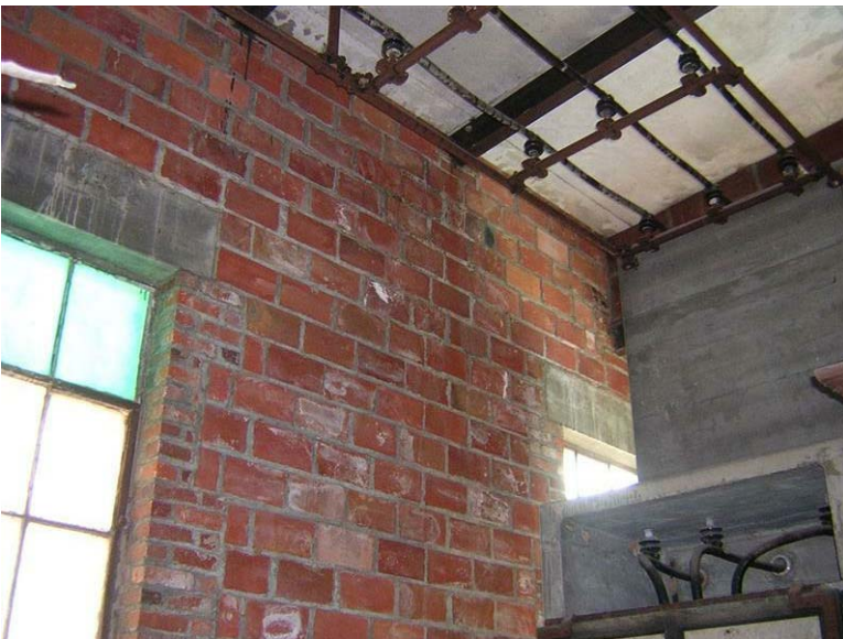
Building 68 – Substation No. 4: The steel structure is rusted and efflorescence is visible on the wall.
