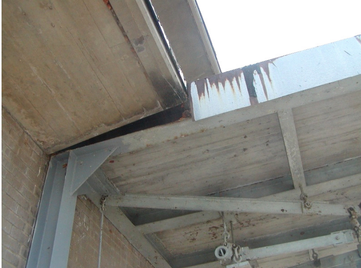
2009 Photo #5: Corroded steel framing and flashing at West canopy
