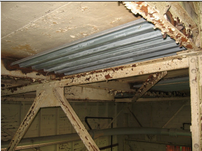
2009 Photo #20: Flaking paint at corroded steel roof framing
