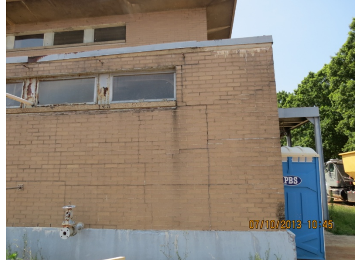
2013 Photo #3: Cracks in masonry on North side. Corrosion evident to the steel framing around windows and roof edging
