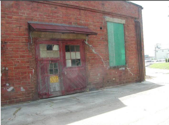
2009 Photo #4: Cracks in masonry South end of West wall
