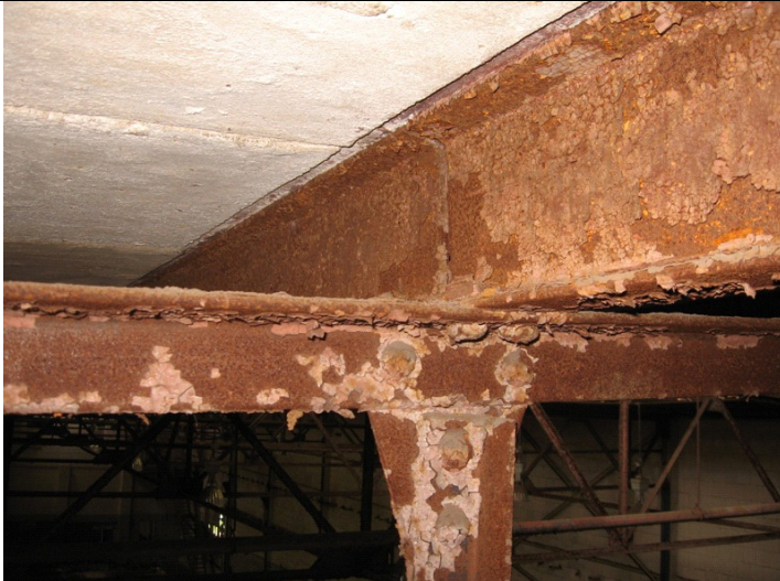
2009 Photo #7: Severely corroded steel framing
