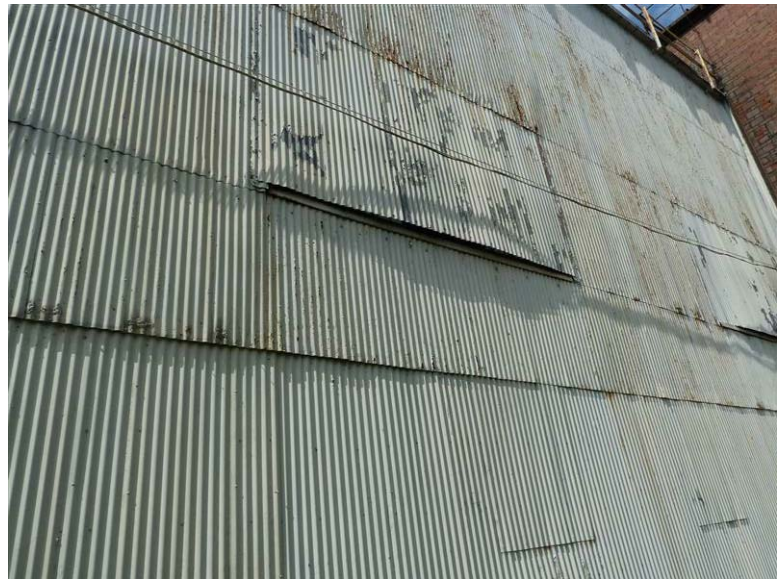
Building 24 – Warehouse No. 4: The openings are covered with corrugated metal panels.
