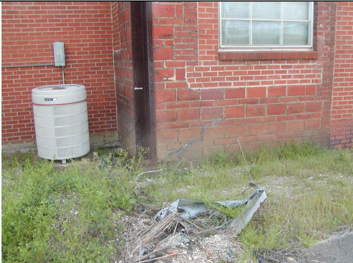
2009 Photo #4: Crack in masonry at Northwest corner where North addition adjoins original building
