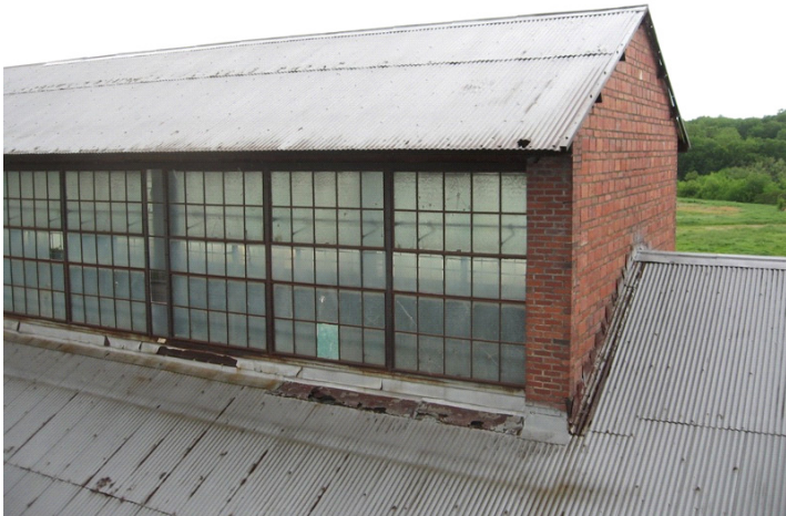
2009 Photo #6: Deteriorated metal roof on East side
