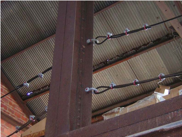
Building 81 – 5A – Nitrate House: Penetrations have been made in the steel columns for railings on the mezzanine.
