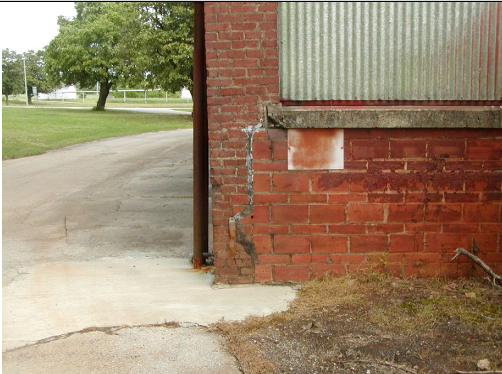
2009 Photo #6: Cracks in masonry at Southwest corner
