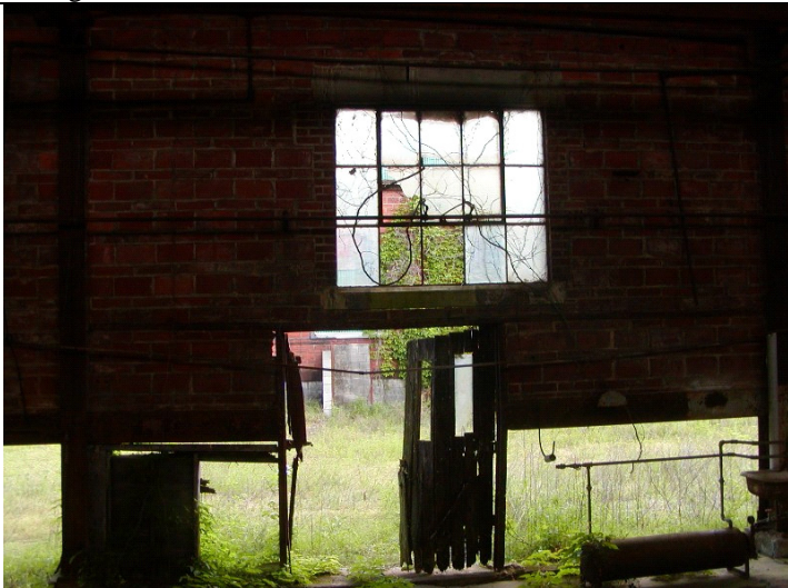
2009 Photo #12: Structurally unstable masonry infill and supporting steel framing
