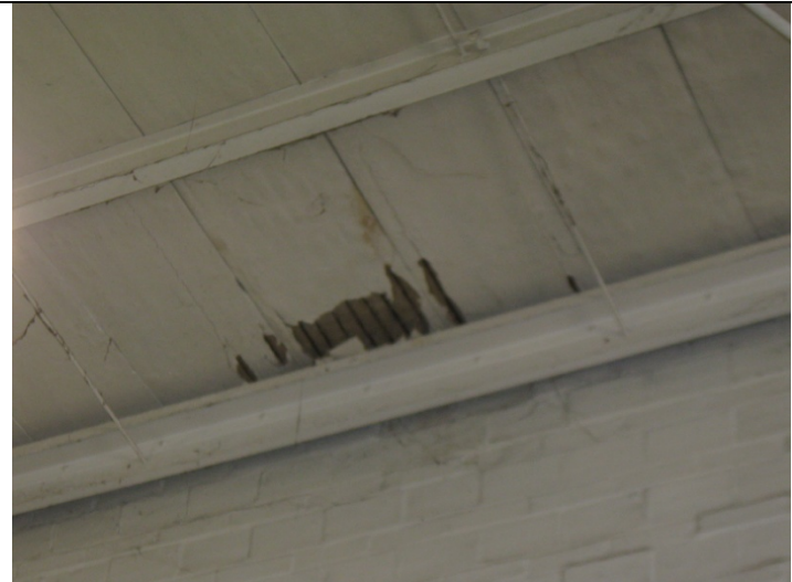
2013 Photo #12: Additional structurally defective concrete roof deck panels – condition in 2009 was not documented
