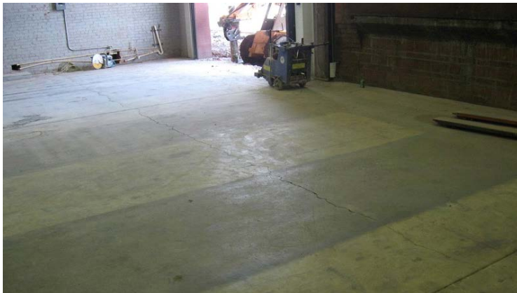
2009 Photo #28: Crack in floor in Northwest area of first level.
