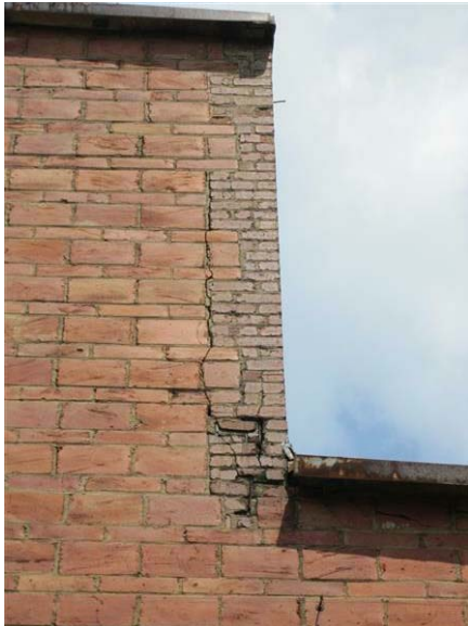
Building 37, 38 – Machine Shop: Cracking in the brick quoins the corners of the building.
