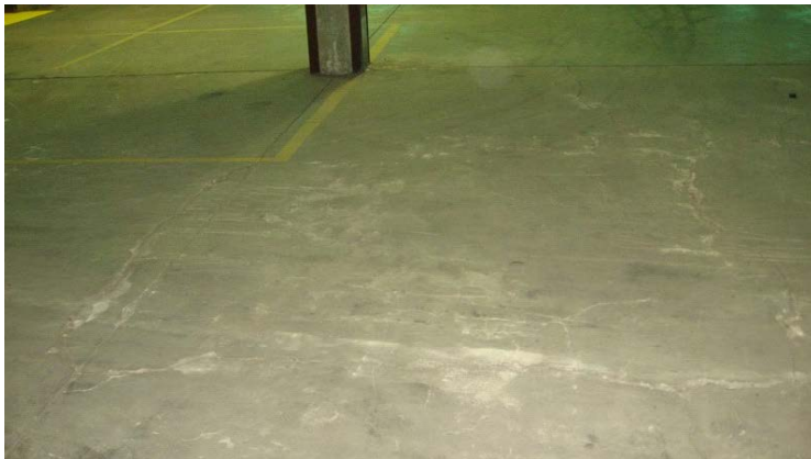
2009 Photo #32: Cracks in West area of second floor slab.
