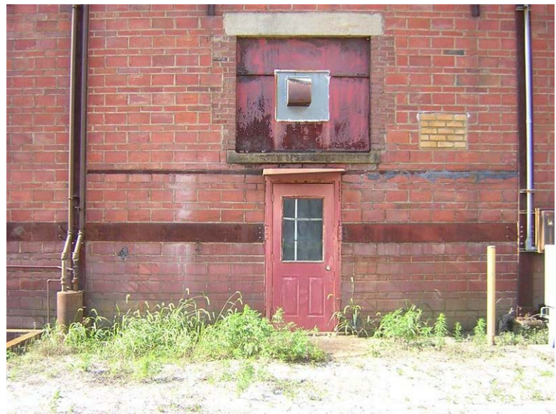
Building 69 – Catalyzer Building No. 1: The metal covering this window opening is rusted and the exposed steel structure is rusted.
