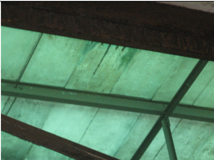
2009 Photo #12: Structurally deficient concrete roof planks
