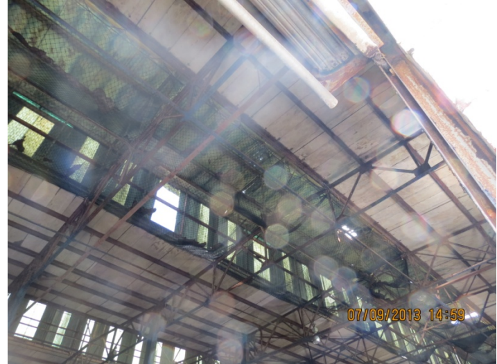
2013 Photo #5: Holes in deteriorated concrete plank roof deck. Condition has continued to decline and may be accelerating.
