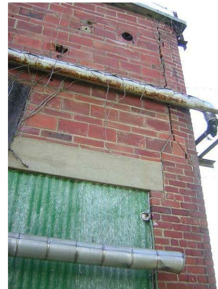
Building 69 – Catalyzer Building No. 1: Visual separation of the corner at the east wall.
