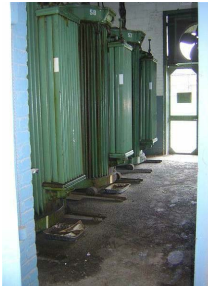
Building 57 – Substation No. 2: Moisture is visible on the concrete slab.
