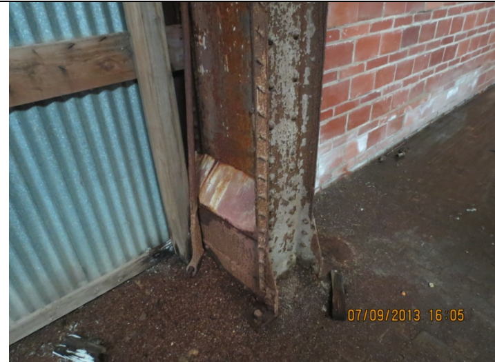
2013 Photo #10: Severely corroded steel column. Continued corrosion evident.
