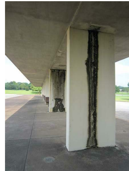
17B - Service Building: Water damage at the concrete canopy has accelerated since the previous assessment.
