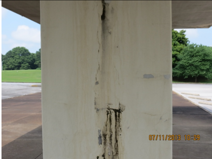
2013 Photo #11: Columns at canopy exhibit mold growth due to leaking interior drains.
