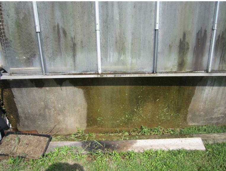
Building 118 – Greenhouse B-D: Staining from moisture and cracking is visible on the lower concrete wall.
