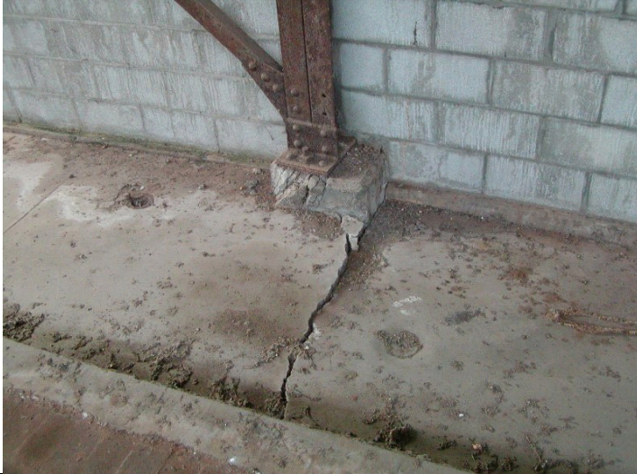
2009 Photo #7: Deteriorated concrete pier and slab at column
