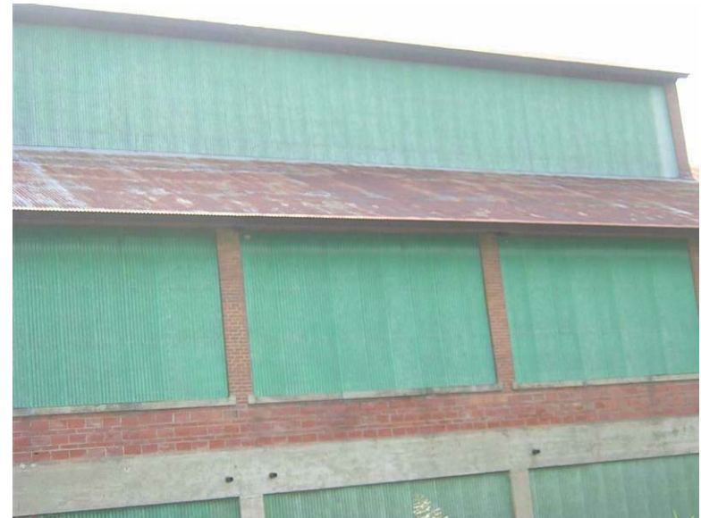
Building 79 – 3A – Nitrate House: Rusting of the metal roof is visible from the exterior.
