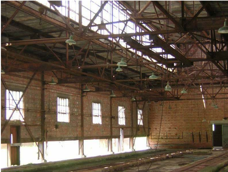
Building 73 – Catalyzer Building No. 5: The steel structure is rusted and several concrete panels are stained from water damage.
