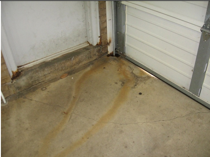
2009 Photo #8: Crack in slab at vehicle storage area
