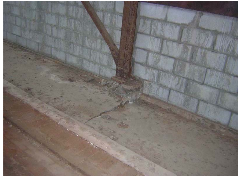
Building 74 – Catalyzer Building No. 6: The concrete footing is broken beneath the steel column.
