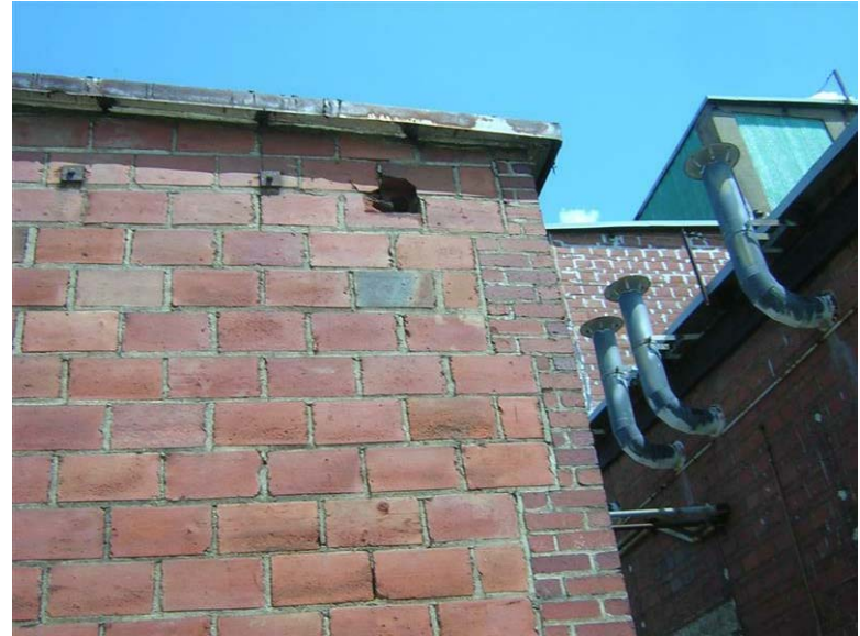
Building 68a – Substation No. 5: Holes penetrate the upper west facade.
