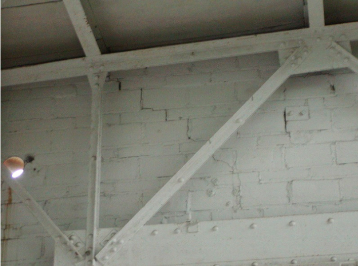
2009 Photo #11: Interior crack in masonry at East wall
