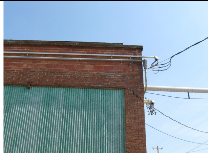
2013 Photo #4: Crack and partially dislodged masonry at Southeast corner exhibits minor progressive deterioration
