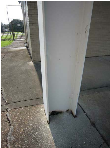
17B - Service Building: The base of the steel columns is rusting adjacent to the concrete.
