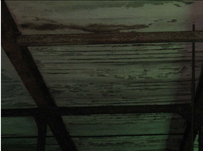
2009 Photo #7: Ruined concrete roof planks
