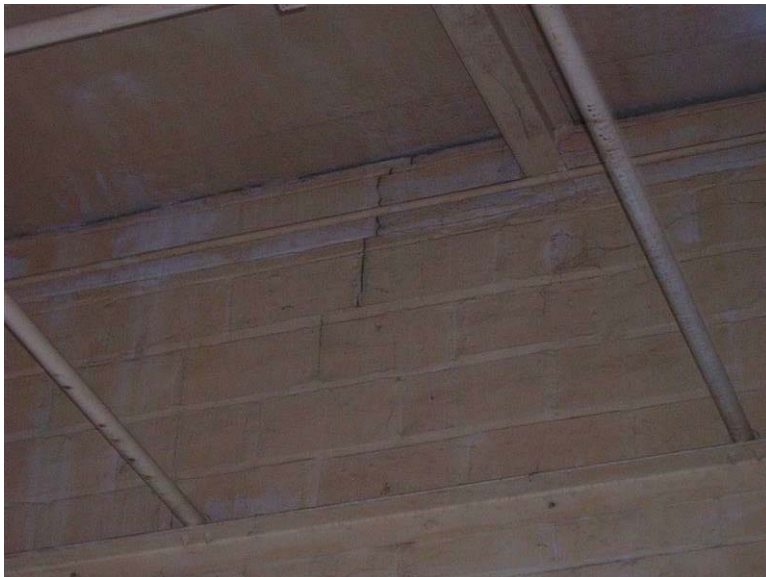
Building 57 – Substation No. 2: Diagonal cracks are visible at the upper walls.
