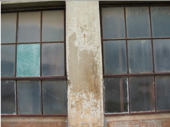
2009 Photo #4: Exterior crack in concrete mezzanine column
