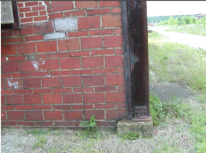
2009 Photo #4: Crack in wall at Northwest corner
