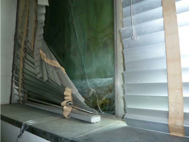
Building 17A - Environmental Research Center: This window has cracked on the east facade.
