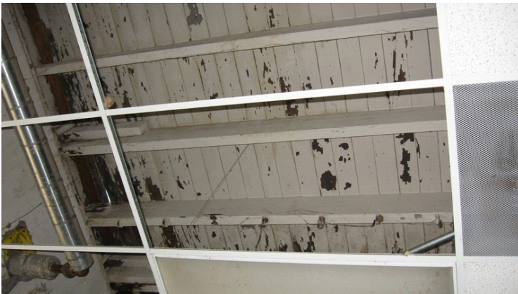
2009 Photo #10: Moisture damage at wood plank roof deck above partially removed lay-in ceiling
