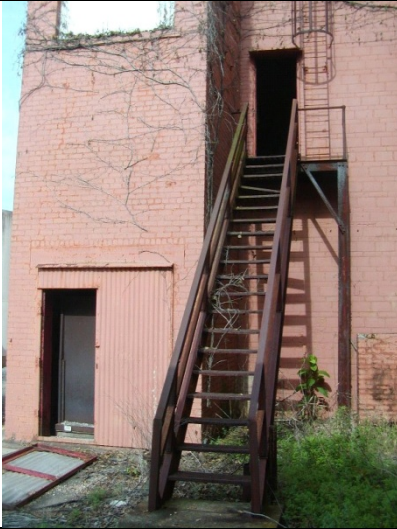
2009 Photo #7: Deteriorated exterior steel stair
