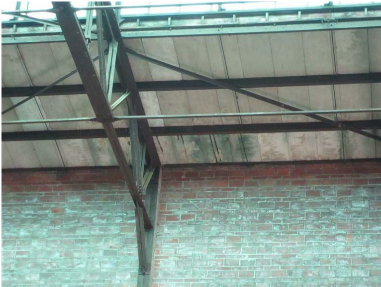
Building 26 – L / N Building Grounds Maintenance Shop: Rebar is exposed where spalling has occurred on the concrete ceiling panels.
