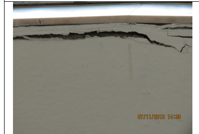
2013 Photo #16: Unoccupied: Broken marble window sill and large crack in wall finish below window
