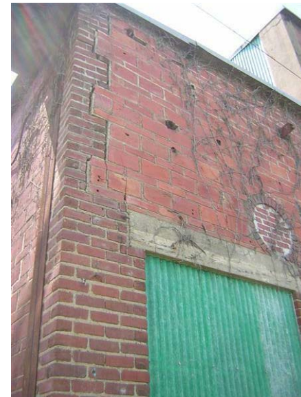
Building 72 – Catalyzer Building No. 4: Cracking has separated the brick quins from the hollow clay tile on the east elevation.
