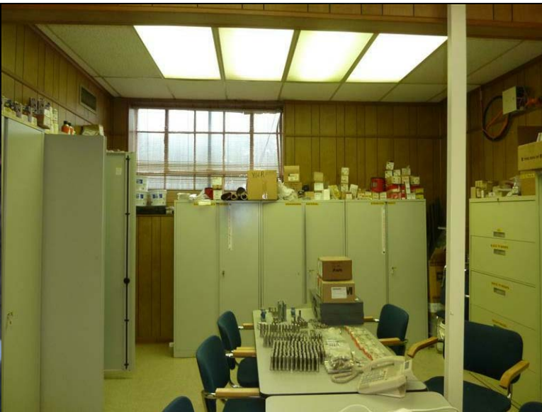
Building 33 – Chemical Plant Warehouse - Shipping and Receiving Office: One of the historic steel windows remains in this office space, but the walls have been clad in paneling.
