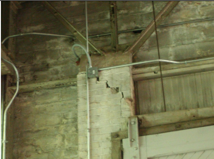
2009 Photo #26: Cracked and partially dislodged masonry at Northeast corner
