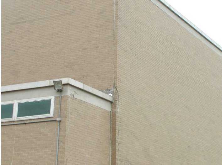
2009 Photo #7: Crack at corner of auditorium wall
