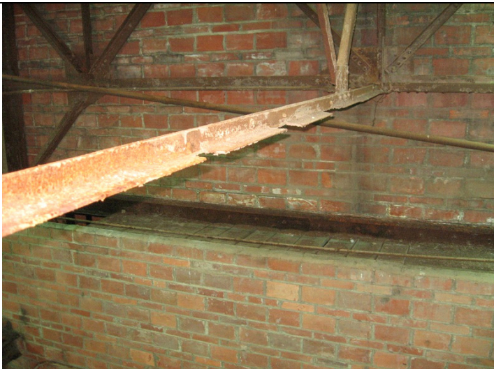
2009 Photo #6: Severely deteriorated steel framing
