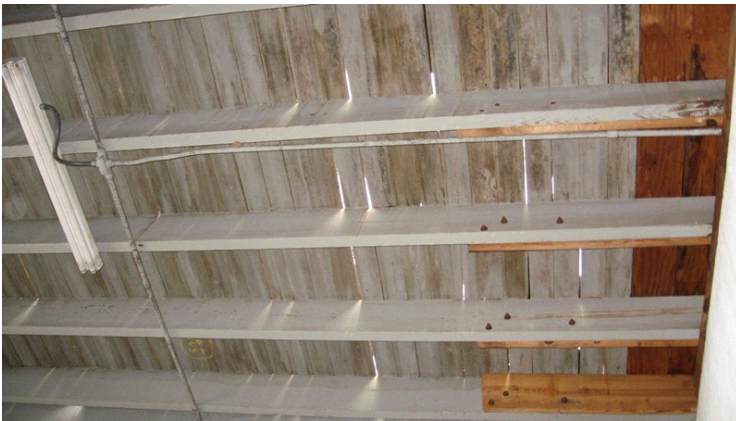
2009 Photo #6: Existing wood plank roof with no roof covering (Bright spots are daylight visible through roof deck)
