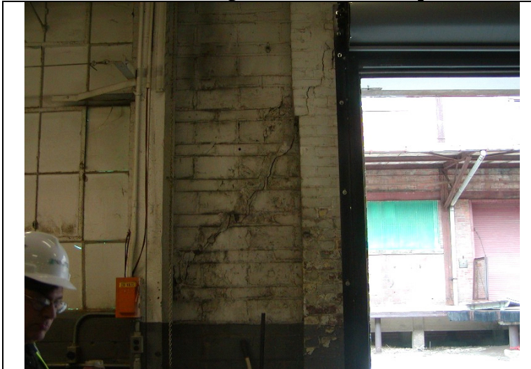
2009 Photo #21: Diagonal crack in masonry at North wall
