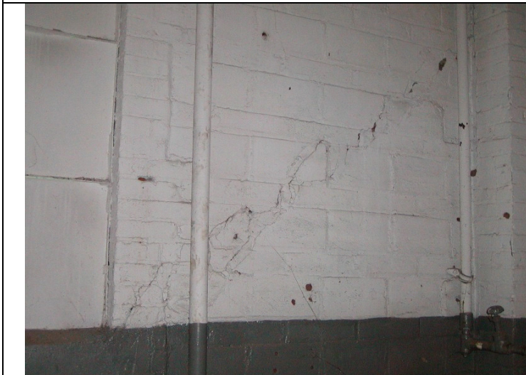
2009 Photo #22: Diagonal crack in masonry at West wall
