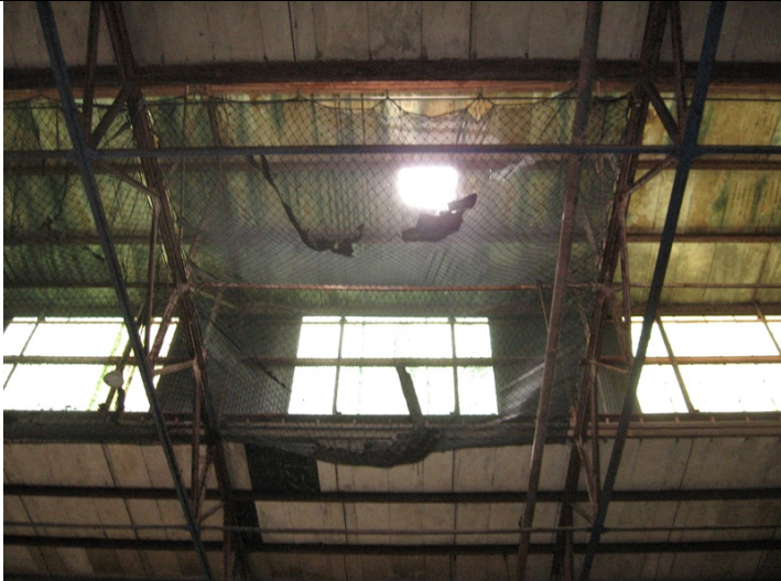
2009 Photo #11: Large holes in deteriorated concrete plank roof deck
