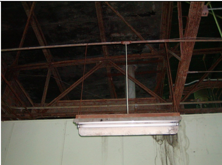
2009 Photo #10: Corroded steel framing and deteriorated roof deck
