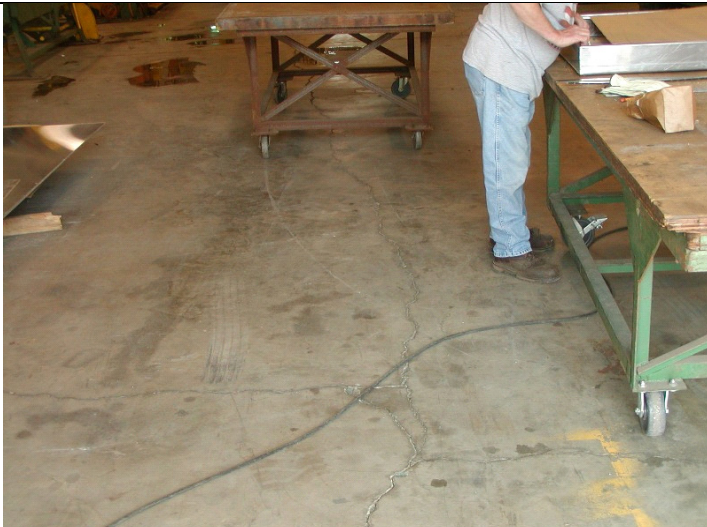
2009 Photo #10: Large cracks in concrete floor slab
