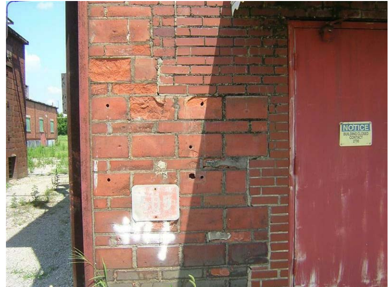
Building 72 – Catalyzer Building No. 4: The hollow clay tile is spalling on the west façade.
