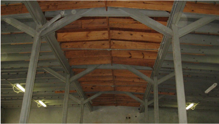
2009 Photo #5: Partially reconstructed wood frame roof structure
