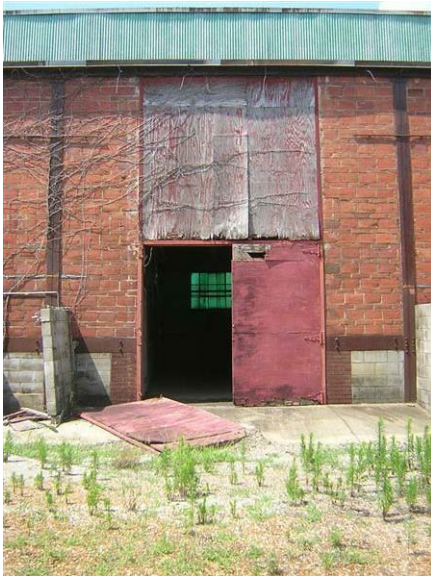
Building 72 – Catalyzer Building No. 4: The doors at this opening are in poor condition. One door is missing from its hinges.
