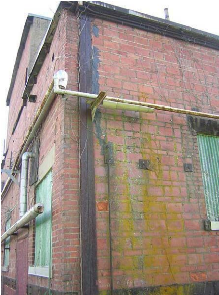
Building 69 – Catalyzer Building No. 1: Staining and mold growth are visible on the north facade.
