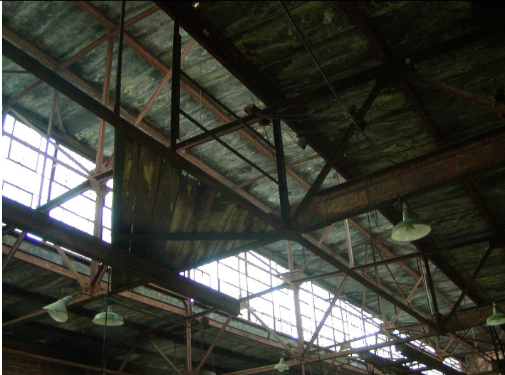
2009 Photo #7: Corroded steel framing and deteriorated concrete plank roof deck
