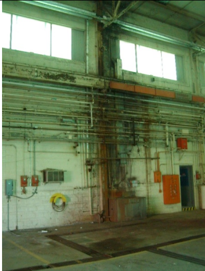
2009 Photo #11: Deteriorated wall construction North side of main building
