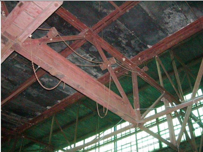
2009 Photo #8: Corroded steel roof framing and deteriorated concrete roof planks
