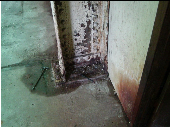
2009 Photo #13: Corroded steel column North side of main building
