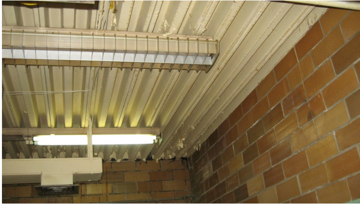
2009 Photo #5: Interior evidence of moisture intrusion at lab building roof
