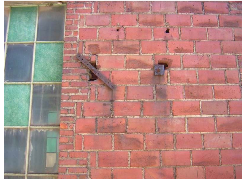
Building 68 – Substation No. 4: Portions of the hollow clay tile are damaged where through-wall ties are located on the south façade.
