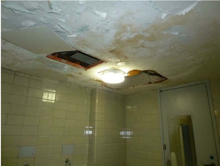
Building 17A - Environmental Research Center: A burst pipe has damaged the plaster ceiling in this lower level restroom.
