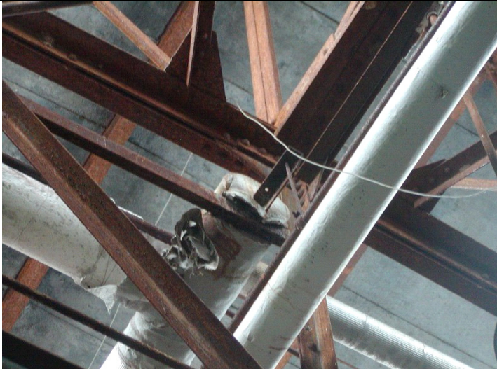
2009 Photo #7: Moderately corroded steel roof framing
