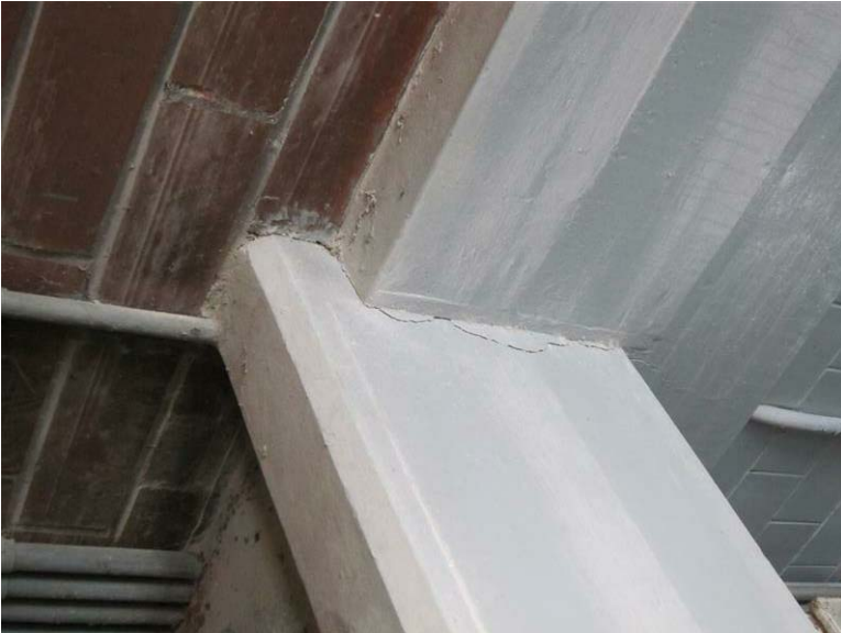
Building 01A - Chemical Feed House: There is a crack at the concrete beam of the second floor stair.
