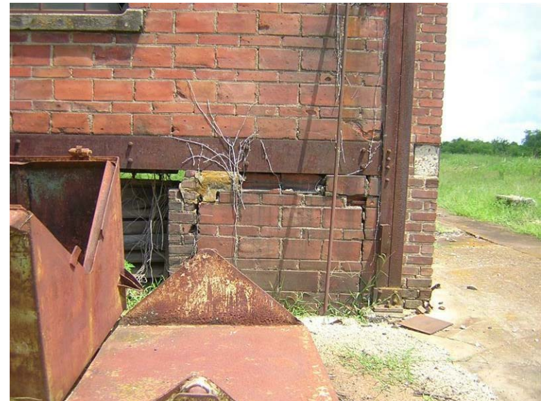
Building 73 – Catalyzer Building No. 5: There is a crack in the hollow clay tile adjacent to the exposed steel structure.
