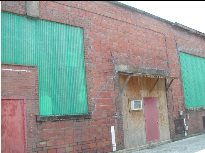
2009 Photo #12: Cracks in masonry at North wall
