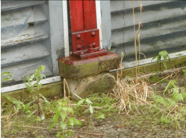
2009 Photo #5: Deteriorated concrete pier at column
