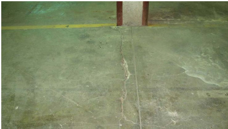
2009 Photo #34: Cracks in West area of second floor slab.
