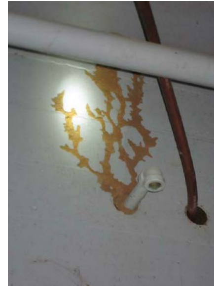
Building 01A - Chemical Feed House: Termites have left a trail along the wall at the pipe penetration.
