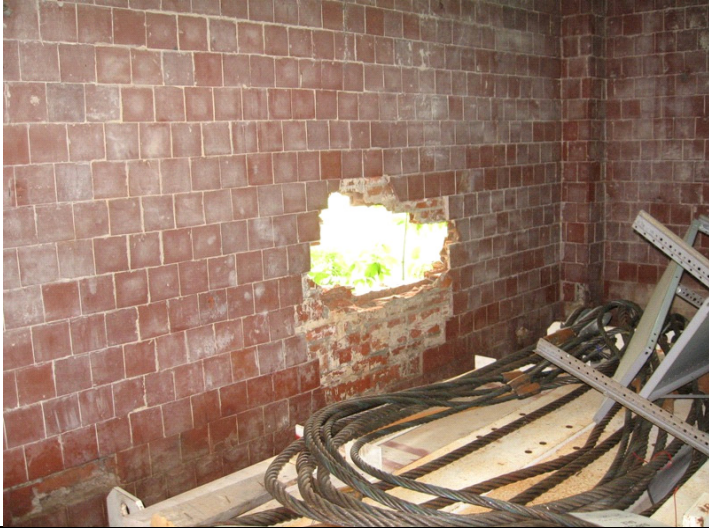
2009 Photo #19: Large hole in exterior masonry wall
