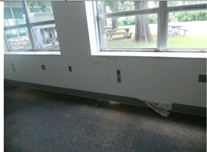
2013 Photo #14: Deterioration of interior finishes observed at several locations.
