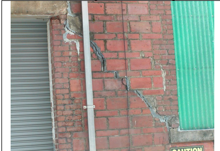
2009 Photo #13: Cracks in masonry at North wall
