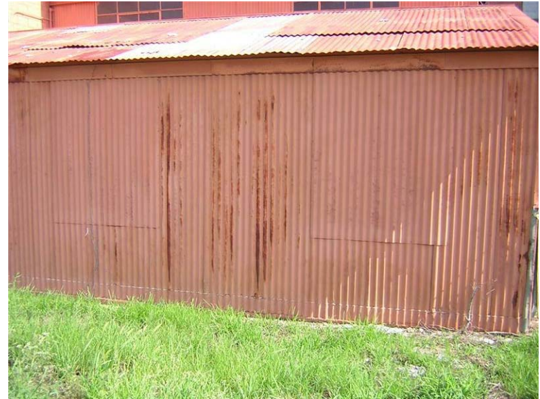
Building 53 – Tin Shop: The corrugated metal panels are rusting at the rear addition.
