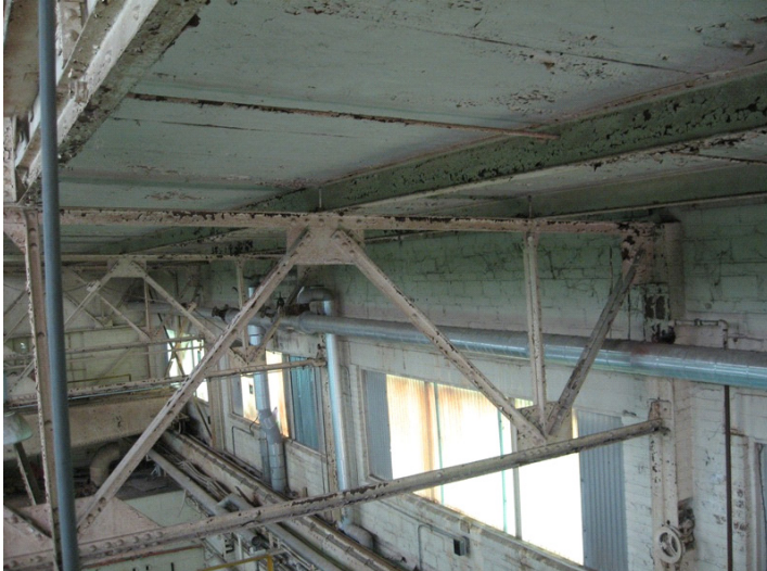
2009 Photo #17: View of main roof framing and roof deck
