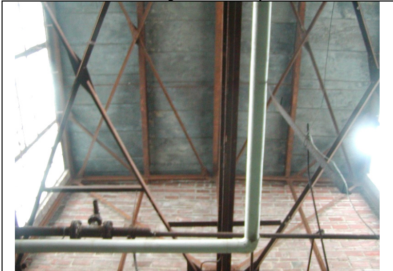
2009 Photo #9: Monitor roof with corroded steel framing and surface deterioration on concrete plank roof deck
