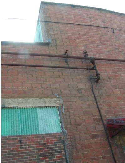
2009 Photo #7: Surface deterioration and cracks in exterior masonry at West wall
