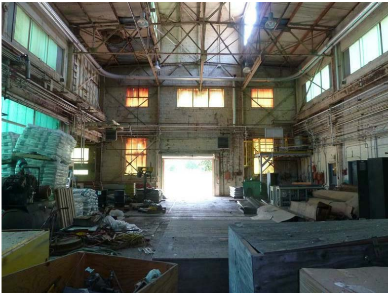
Building 39 – Engineering Lab: This portion of the building is a double height space. Several concrete ceiling panels have been replaced with metal panels.
