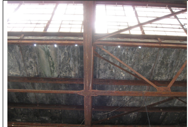
2013 Photo #5: Progressive deterioration of concrete plank roof deck observed – note holes through deck below clerestory
