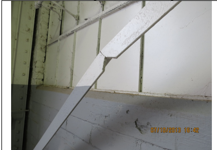
2013 Photo #27: Failed cross-bracing at the South face at the East end of the building.
