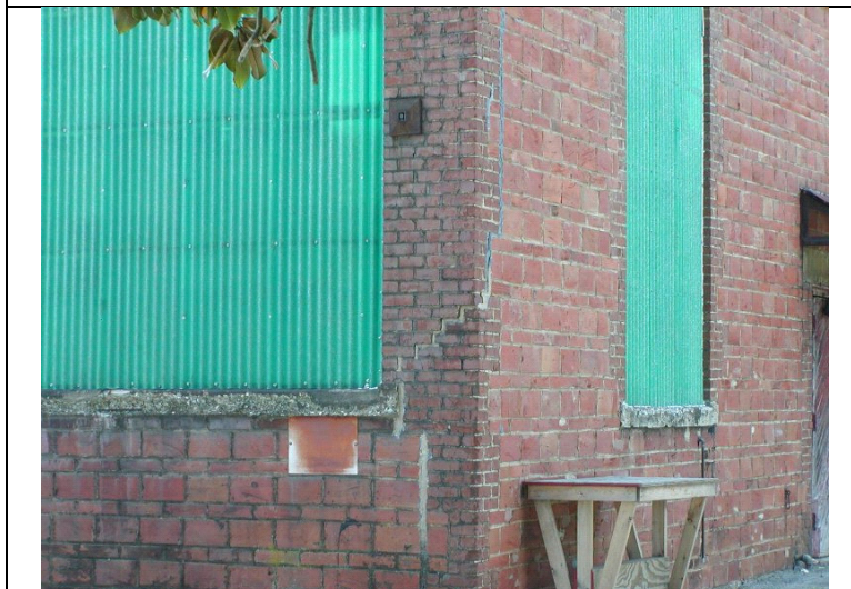
2009 Photo #14: Cracks in masonry at Northwest corner
