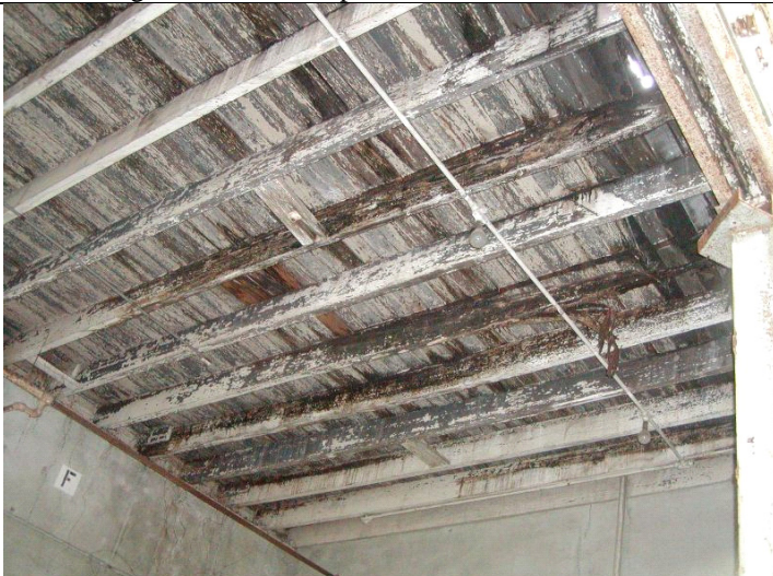
2009 Photo #4: Severely deteriorated wood roof structure
