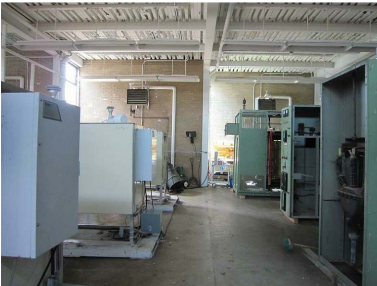
17B - Service Building: Paint is flaking at the metal ceiling.
