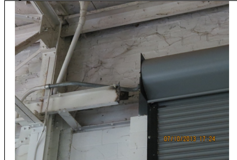
2013 Photo #28: Brace cut to facilitate installation of roll-up door.
