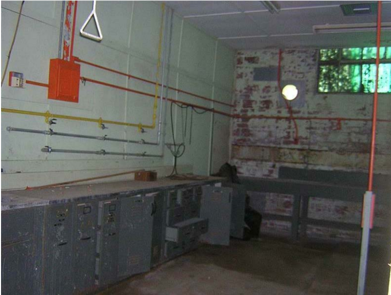
Building 69 – Catalyzer Building No. 1: Paint is flaking from the hollow clay tile walls in the laboratory space.
