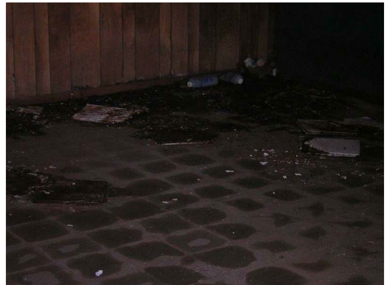
Building 74 – Catalyzer Building No. 6: The floor tiles are damaged from water infiltration.
