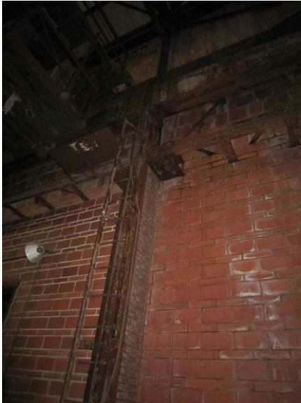
Building 24 – Warehouse No. 4: Water is dripping down the face of the north masonry wall.
