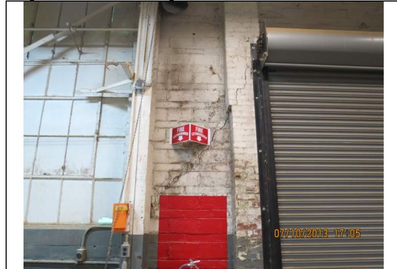
2013 Photo #21: Diagonal crack in masonry at North wall
