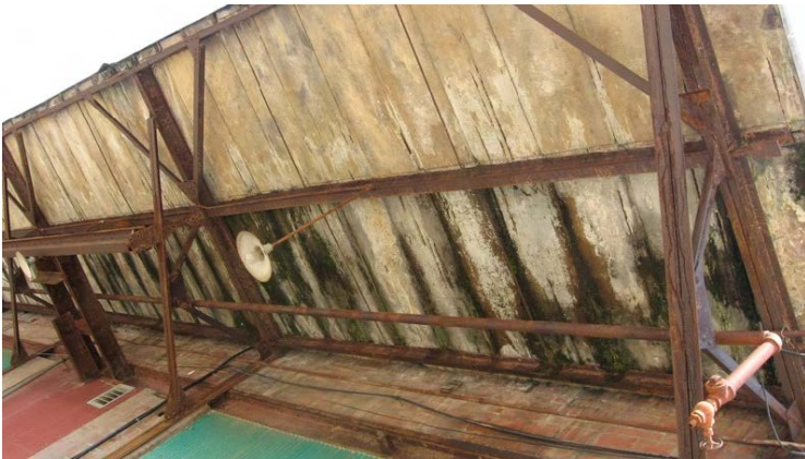
2009 Photo #20: Deteriorated and ruined concrete roof planks at South canopy.
