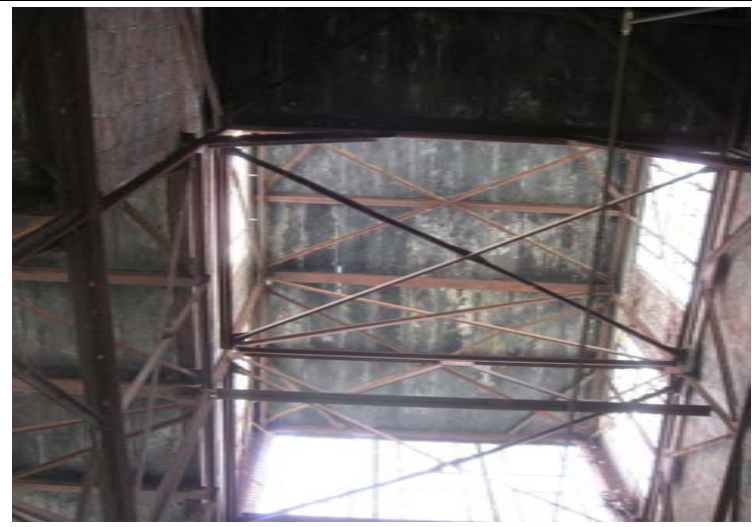
2013 Photo #7: Progressive deterioration of the concrete roof deck was observed
