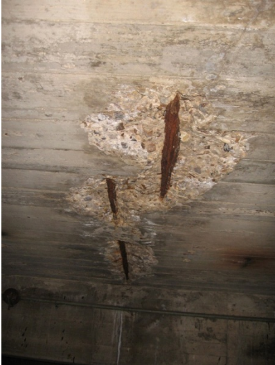
2009 Photo #19: Spalled concrete at basement structure
