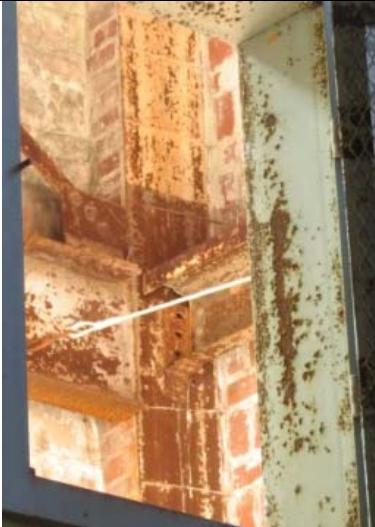
2013 Photo #19: Severely corroded steel and failed connection at Northwest corner of building.
