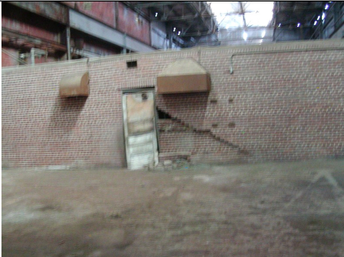
2009 Photo #8: Partially collapsed interior masonry partition
