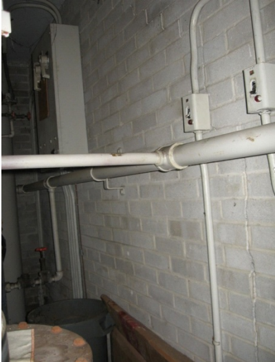
2009 Photo #9: Minor crack in interior brick wall
