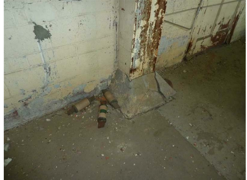
Building 39 – Engineering Lab: The concrete footing at this column is cracked.
