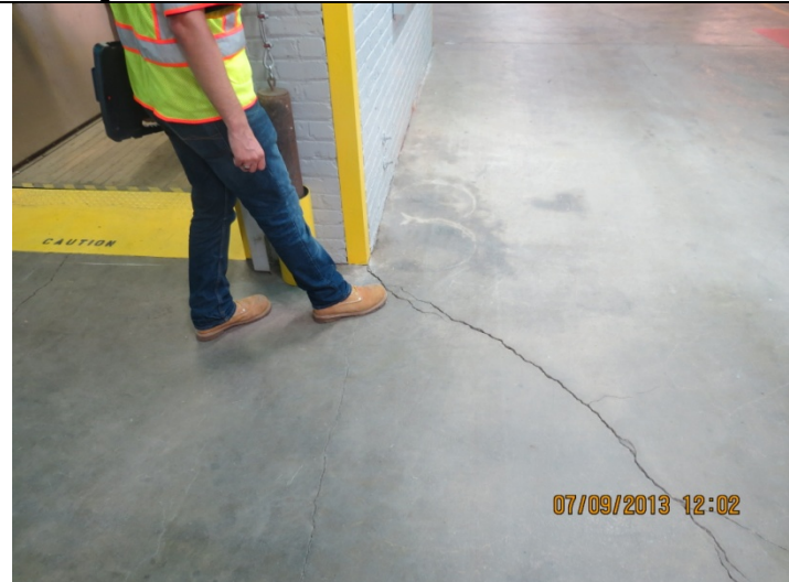
2013 Photo #31: Cracks in second floor slab at Northeast corner of East elevator. Different location than 2009 photo.
