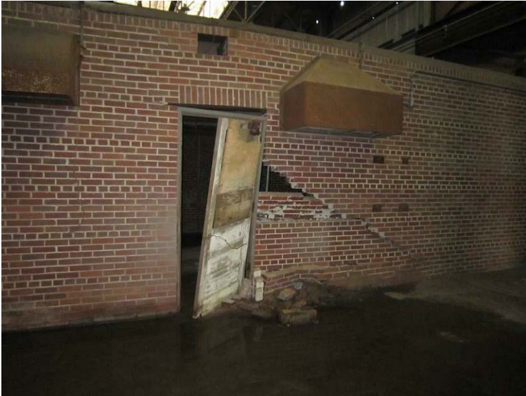
Building 24 – Warehouse No. 4: The brick demising wall has failed and the floor has settled where the water has accumulated.
