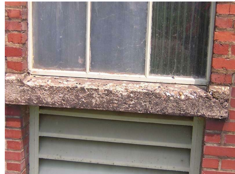
Building 57 – Substation No. 2: The concrete sill is damaged at several of the windows.
