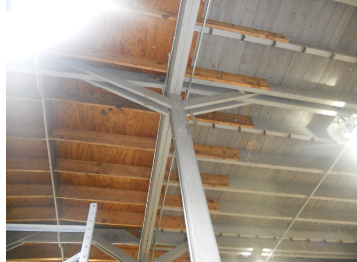
2013 Photo #7: Wood roof framing has been repaired and deteriorated portions of wood roof deck have been replaced
