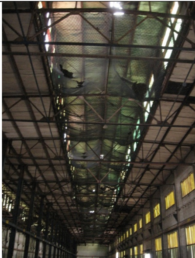
2009 Photo #12: Holes in deteriorated concrete plank roof deck
