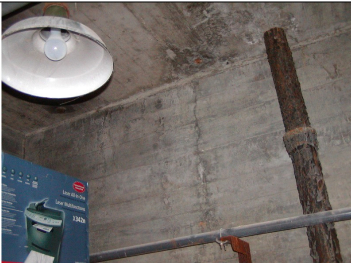
2009 Photo #8: Evidence of water intrusion at basement wall and ceiling.
