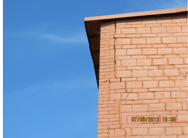
2013 Photo #5: Crack in masonry at end wall West side. Movement of exterior wall observed.
