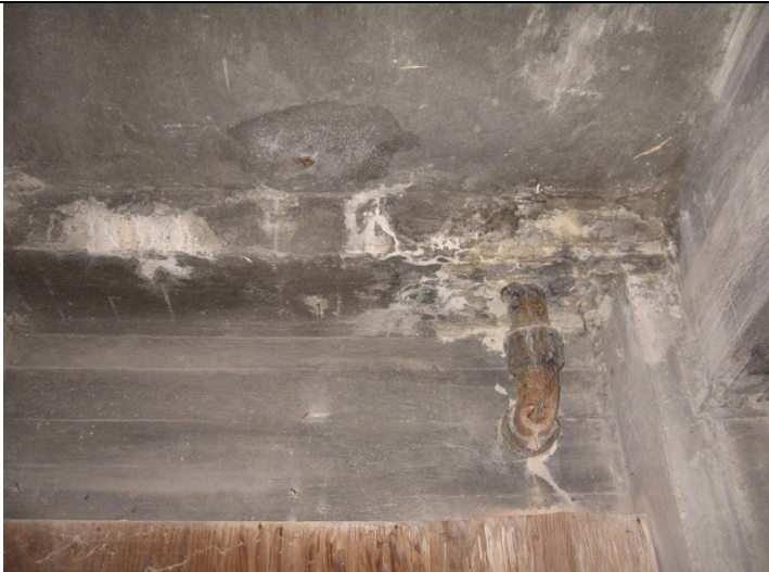
2009 Photo #20: Deterioration from water intrusion at mezzanine concrete frame
