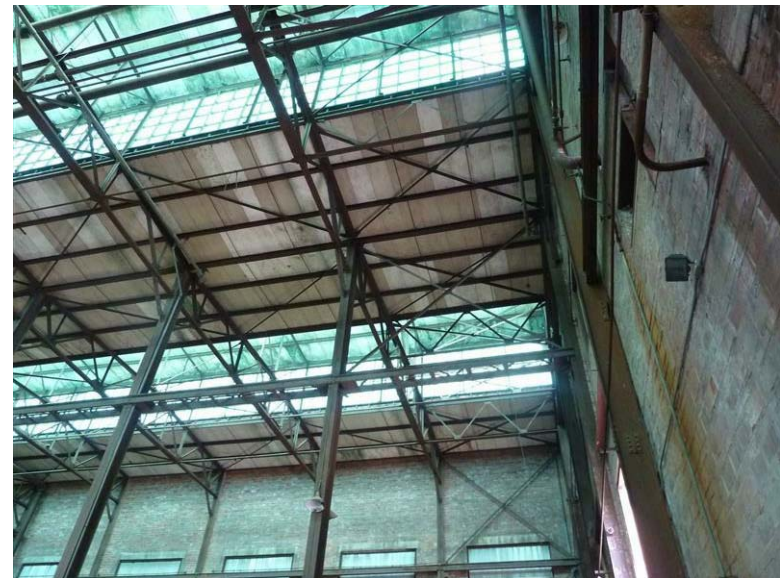
Building 26 – L / N Building Grounds Maintenance Shop: Staining on the north wall adjacent to the pipe.
