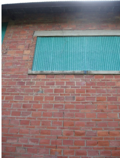
2009 Photo #4: Vertical cracks in masonry
