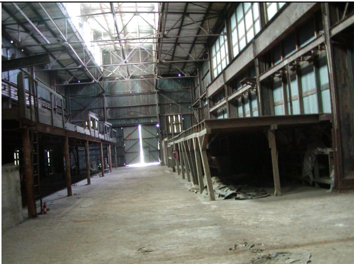
2009 Photo #4: Steel and wood mezzanines at building interior
