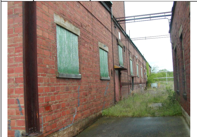
2009 Photo #2: Exterior building looking at South wall – note cracks in masonry above foundation wall
