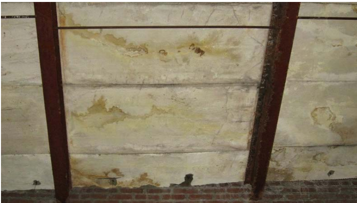
2009 Photo #44: Deteriorated concrete roof plank at interior wall.
