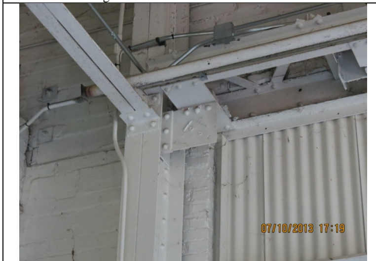
2009 Photo #29: Cross-bracing removed at Southwest corner.
