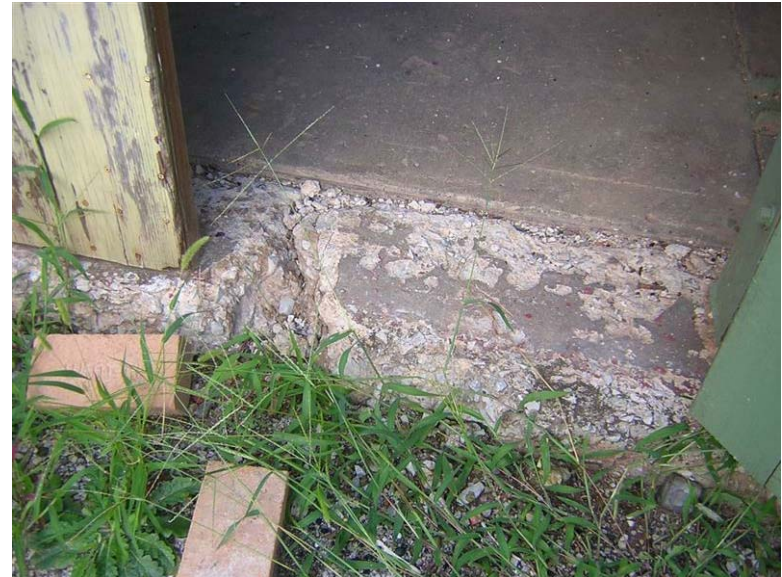
Building 68 – Substation No. 4: The concrete slab is broken at the door opening.
