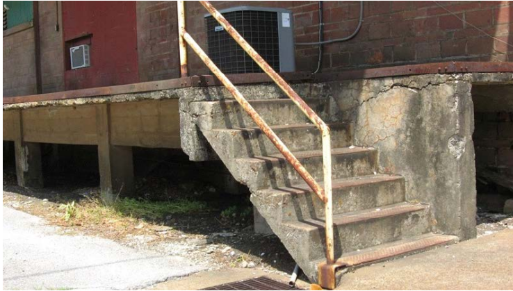
2009 Photo #23: Deteriorated concrete steps and support at East and South loading dock.
