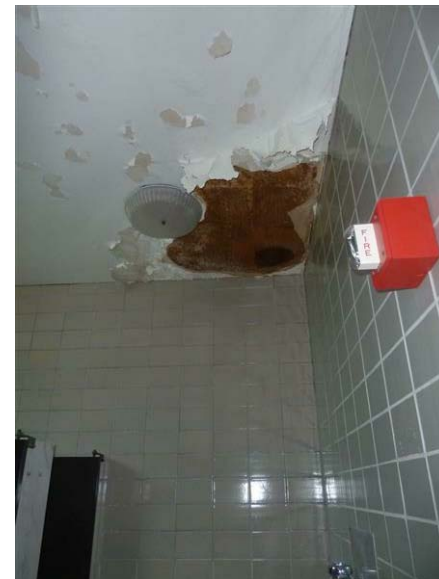
17B - Service Building: Water damage at the restroom ceiling.
