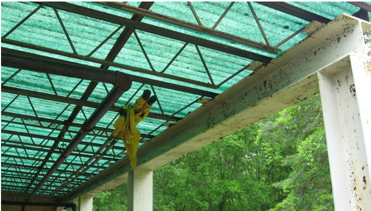
2009 Photo #4: Mildly to moderately corroded steel at open covered storage area
