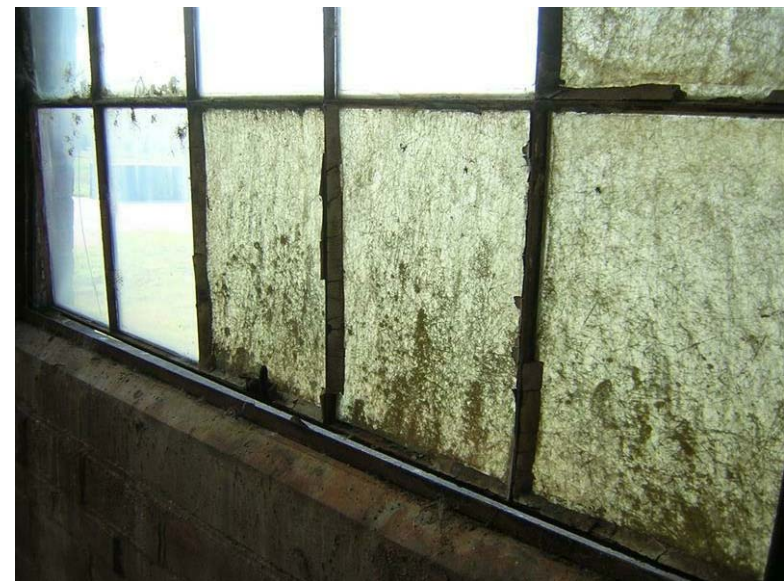
Building 81 - 5A - Nitrate House: The metal muntins are rusted and several window panes have been replaced.
