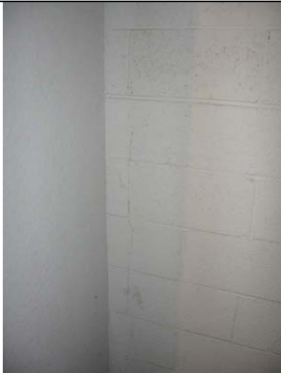
2009 Photo #12: Minor crack in interior concrete masonry wall
