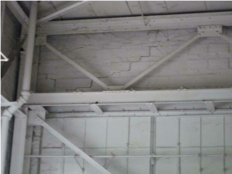
Building 37 – Machine Shop: Diagonal cracking along the upper portion of the wall above the window.
