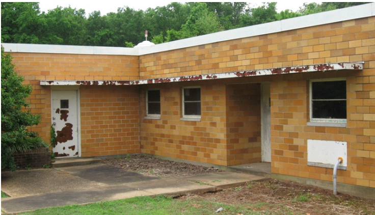
2009 Photo #2: Corroded awning at lab building
