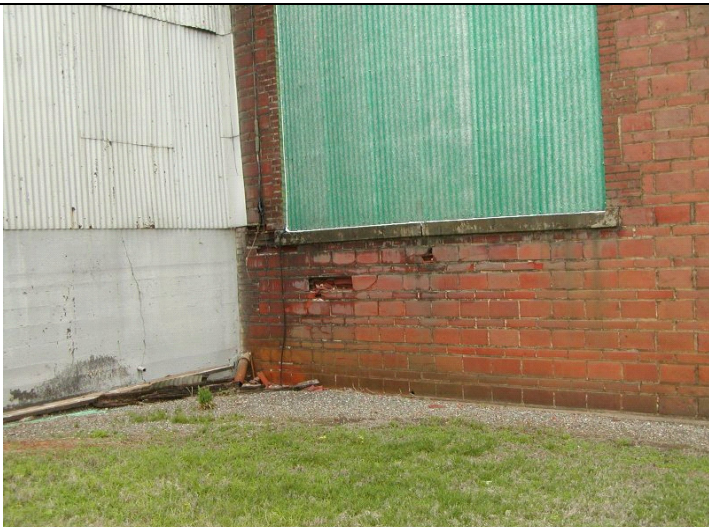
2009 Photo #4: Spalled masonry on West side at intersection with Building 24
