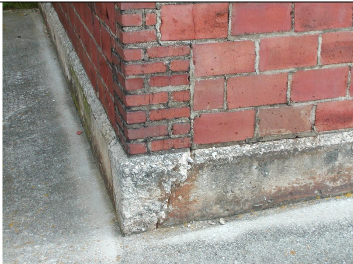
2009 Photo #4: Minor crack on turned down slab
