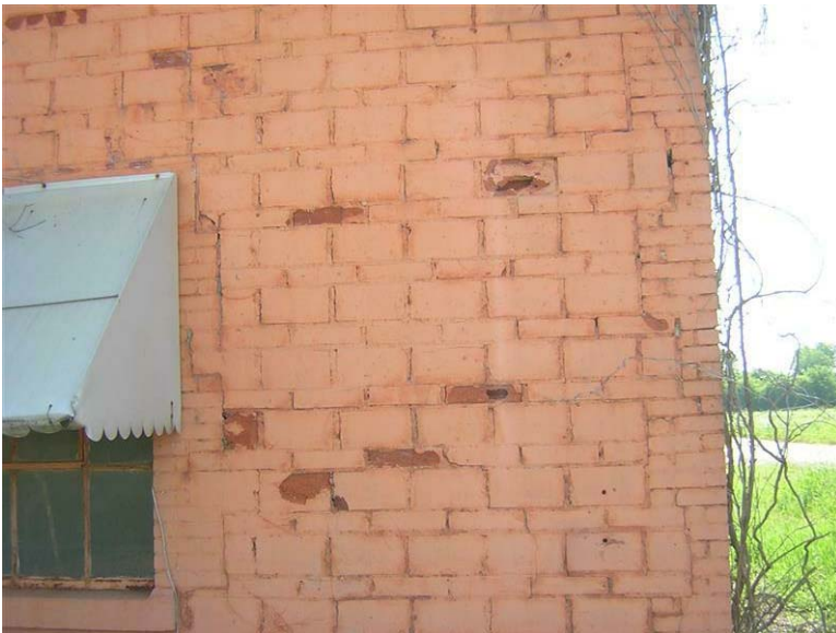
Building 53 – Tin Shop: The hollow clay tile is spalling on the west facade.
