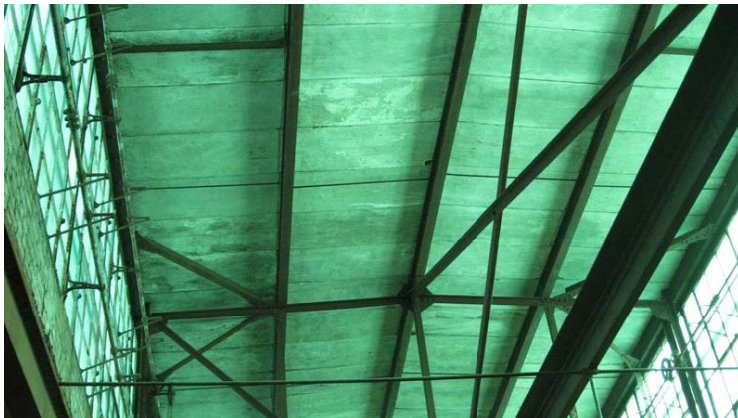
2009 Photo #46: Concrete roof planks with surface deterioration at clerestory monitor.
