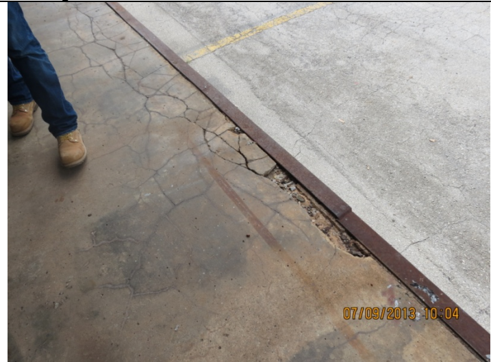
2013 Photo #25: Cracks in South loading deck slab. Different location than 2009 photo.
