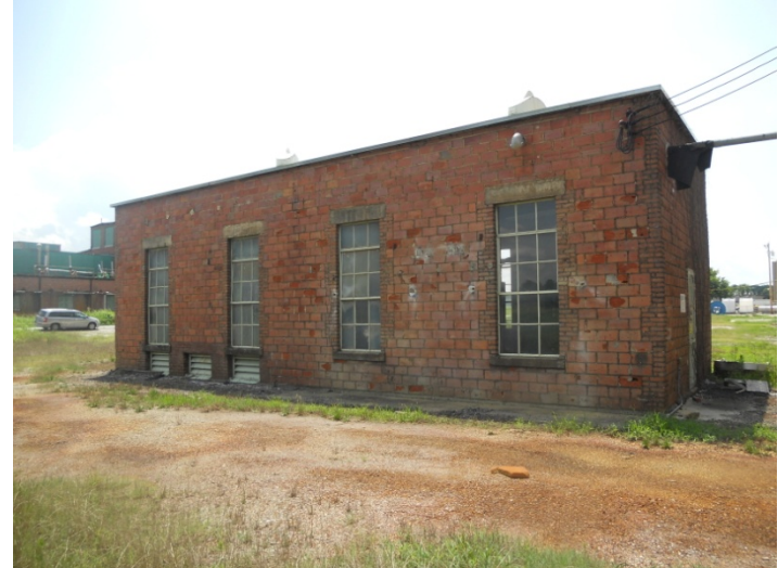
2013 Photo #2: Minor progressive deterioration of exterior masonry
