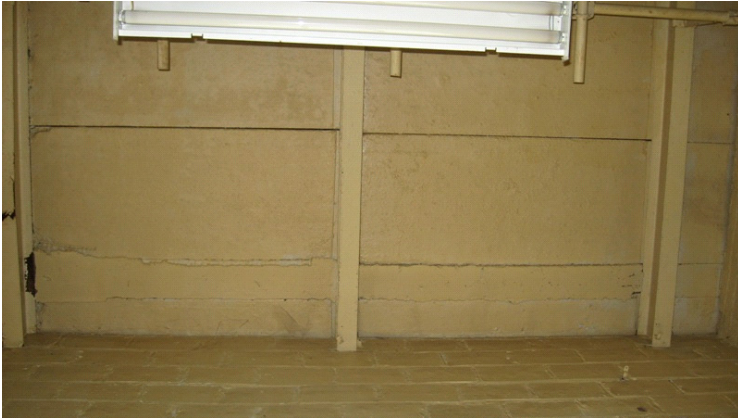
2009 Photo #7: Concrete roof plank appears to have been repaired; note corroded steel beam at left end of irregular surface at roof deck
