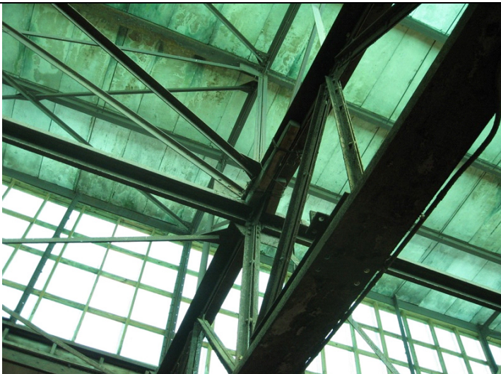
2009 Photo #16: Deteriorated concrete roof planks
