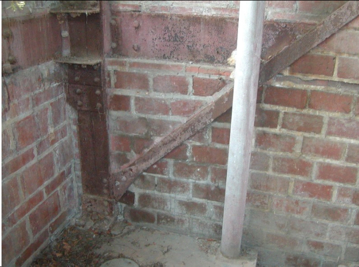
2009 Photo #9: Deteriorated steel column and wall framing
