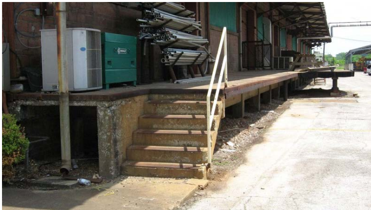
2009 Photo #24: Deteriorated concrete steps and support at West and South loading dock.
