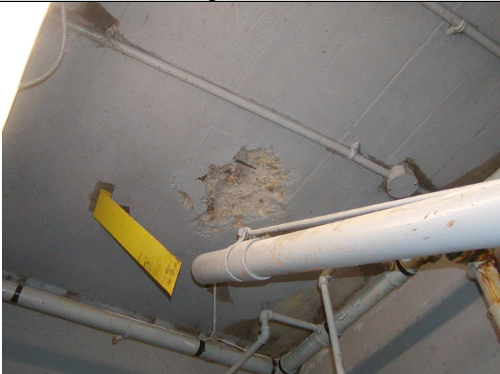
2009 Photo #7: Spall in soffit of floor slab above basement.
