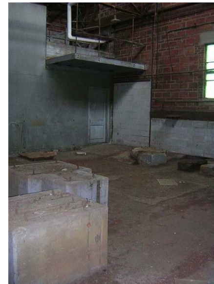
Building 69 – Catalyzer Building No. 1: The steel supporting the mezzanine is rusted.
