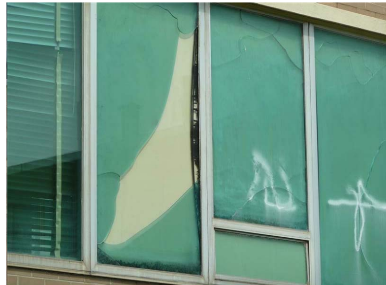
Building 17A - Environmental Research Center: Broken panes occur on the east facade of the building where the window sills are heaving.
