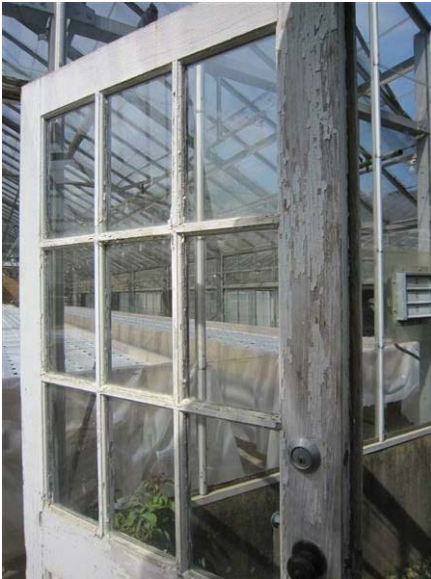
Building 118 – Greenhouse B-D: Although paint is flaking from several of the wooden doors, the wood remains in good condition.
