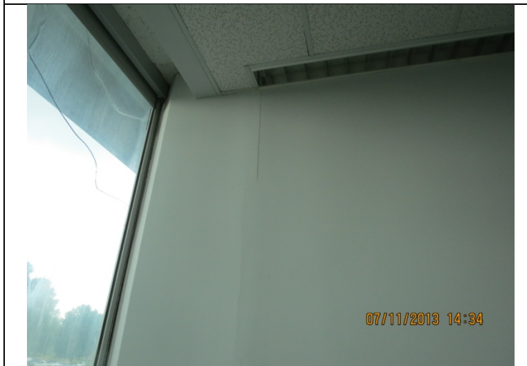
2013 Photo #15: Unoccupied: Crack and ripple in interior finish. (Left) Broken window.
