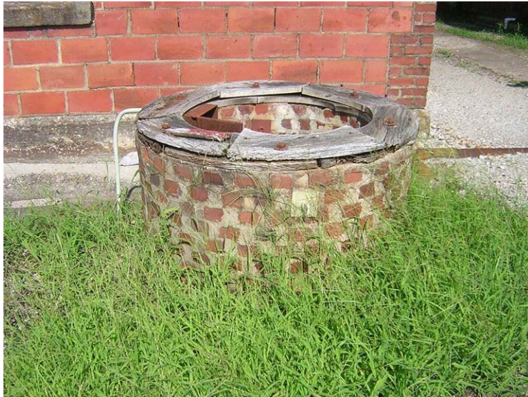
Building 68 – Substation No. 4: The wood is warped and damaged on top of this well structure.
