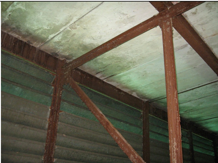
2009 Photo #10: Deteriorated concrete roof planks
