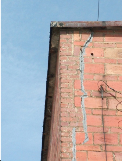
2009 Photo #5: Cracked and partially dislodged masonry at Southeast corner
