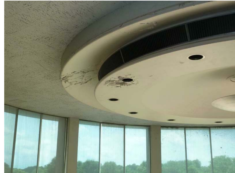
Building 17A - Environmental Research Center: Plaster damage is present at the circular ceiling medallion in the main entry.
