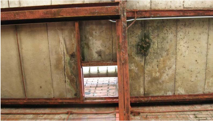
2009 Photo #7: Deteriorated concrete roof planks at North canopy.
