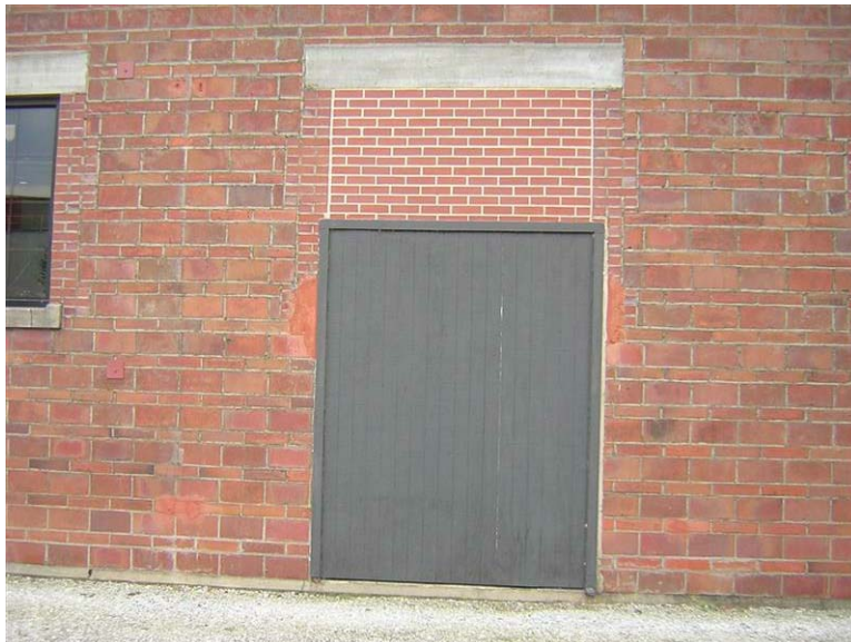
Building 44 – Project Operations Bath House: This window opening has been infilled with brick and made into a door opening, which is filled with T-111 siding.
