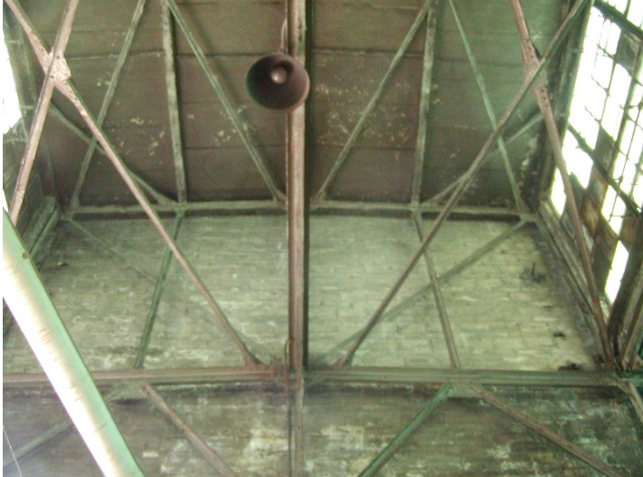
2009 Photo #19: General moderate deterioration of monitor framing, wall, and roof deck
