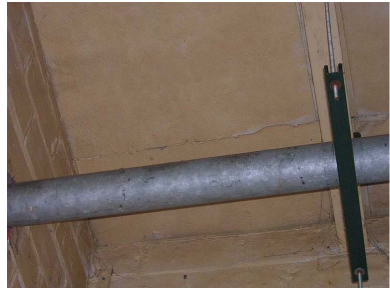
Building 57 – Substation No. 2: A line of concrete ceiling panels is broken.
