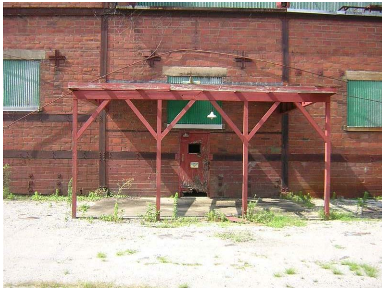
Building 70 – Catalyzer Building No. 2: The wood door and awning are damaged.
