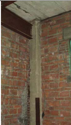
2009 Photo #38: Interior crack/void at column and wall at Northwest corner.
