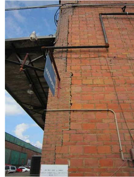
Building 33, 34, 35, 36 – Chemical Plant Warehouse: Severe cracking at the brick quoins at the corners of the building.
