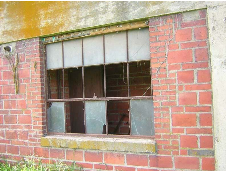
Building 79 – 3A – Nitrate House: Panes are missing and broken in this uncovered window.
