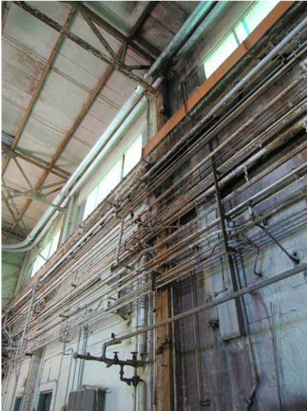
Building 39 – Engineering Lab: Severe water damage has rusted the steel column and stained the wall.
