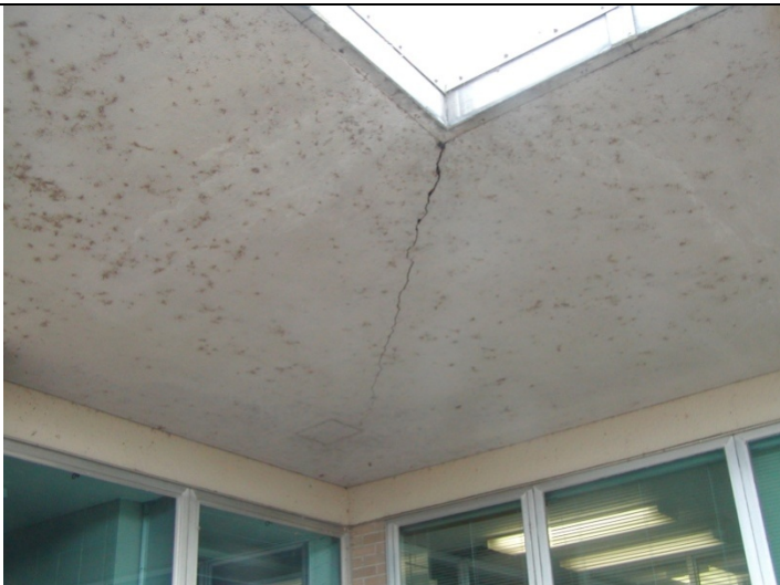
2009 Photo #2: Crack in concrete soffit near main entrance
