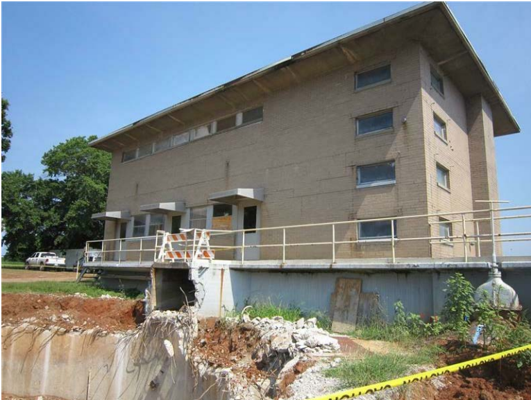
Building 01A - Chemical Feed House: There is a large, deep hole in the ground south of the building that could potentially affect the building's foundation.
