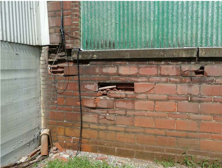
Building 26 – L / N Building Grounds Maintenance Shop: Spalling masonry and eroded mortar joints where water is flowing down the face of the building.
