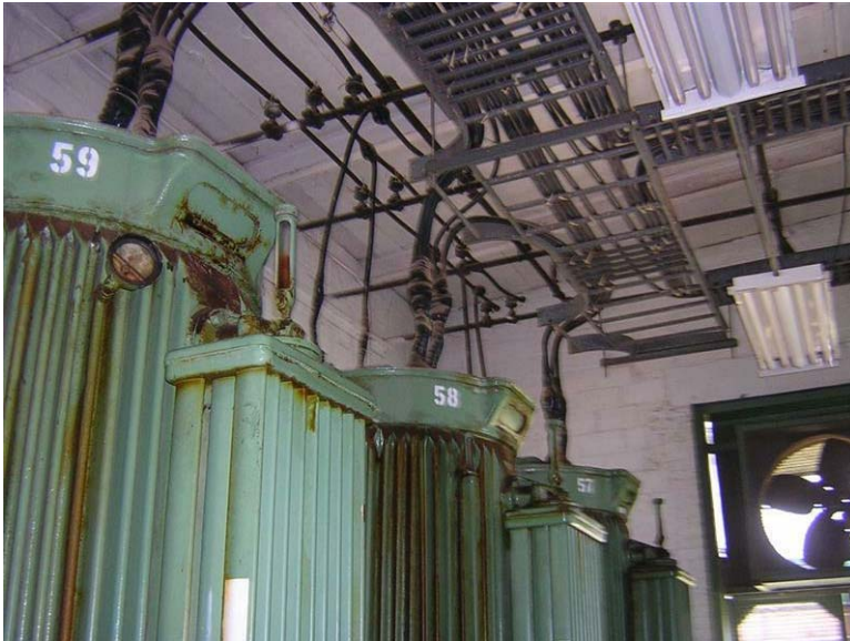
Building 57 – Substation No. 2: Interior view of the ceiling and raceways for electrical conduits overhead.
