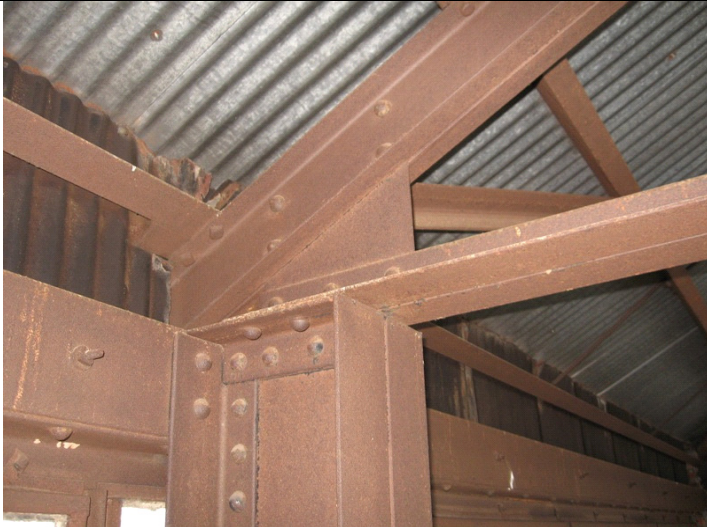
2009 Photo #15: Surface corrosion on steel framing
