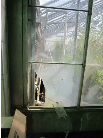
Building 118 – Greenhouse B-D: There are several localized broken panes.
