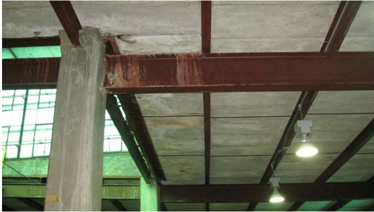
2009 Photo #41: Water intrusion damage at concrete roof planks, steel beams, and concrete column.
