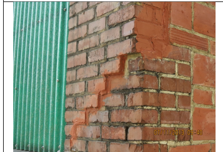
2013 Photo #14: Repaired cracks in masonry at Northwest corner.
