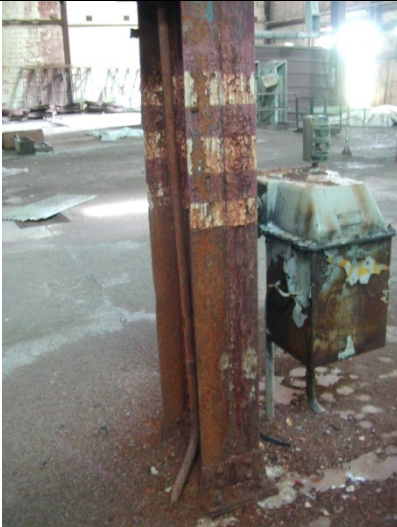
2009 Photo #5: Severely corroded steel column
