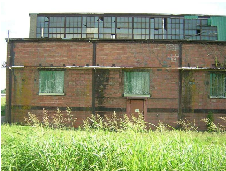
Building 69 – Catalyzer Building No. 1: Extant clerestory windows have several broken panes and the lower windows are covered with fiberglass.
