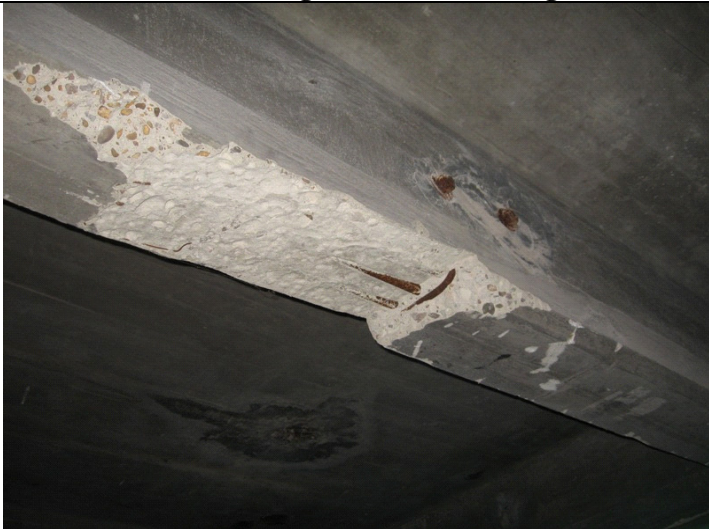
2009 Photo #23: Heavily damaged mezzanine concrete beam
