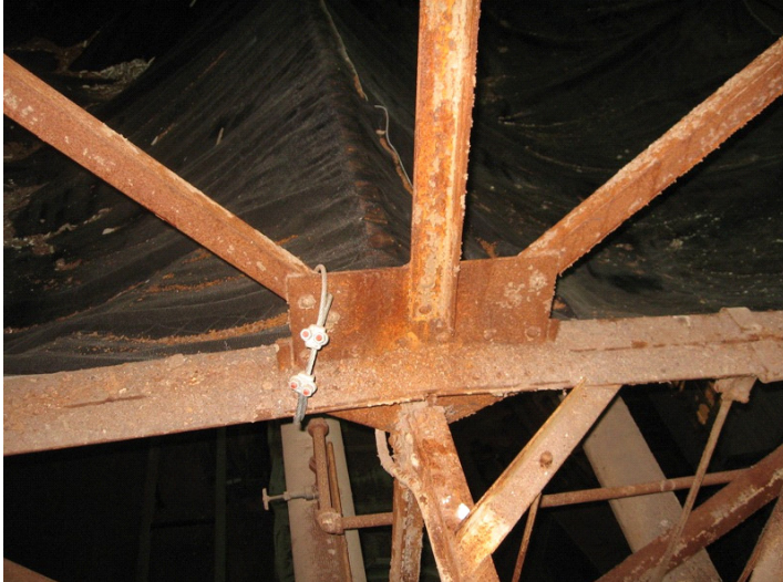
2009 Photo #11: Severely corroded structural steel
