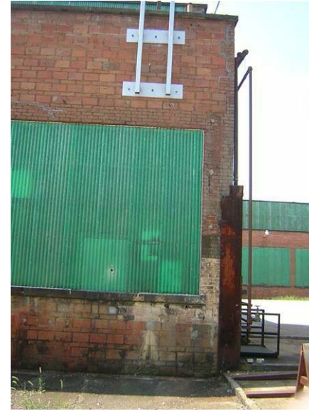
Building 41 – Sheet Metal Shop: Water staining and efflorescence are visible on the west side of the north wall.
