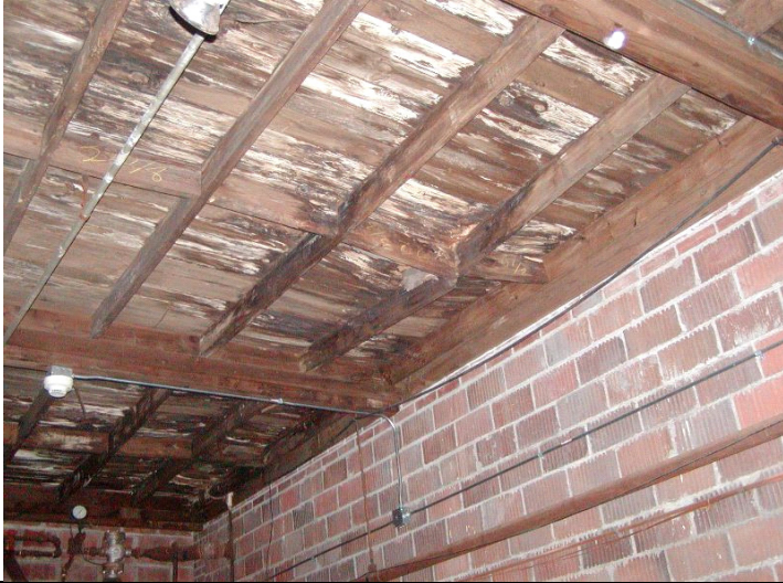
2009 Photo #19: Ruined roof deck of interior enclosure
