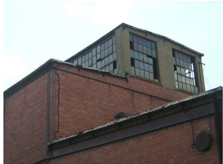
Building 73 – Catalyzer Building No. 5: There are several broken panes at the clerestory. The crack at the upper corner of the wall has been patched with a substance incompatible with the mortar.
