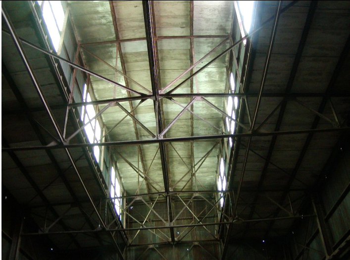
2009 Photo #5: Deteriorated concrete plank roof deck
