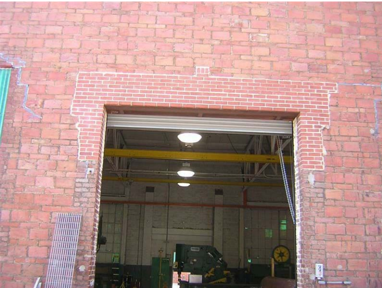
Building 41 – Sheet Metal Shop: The brick door surround has been replaced with incompatible brick in a non-historic pattern.
