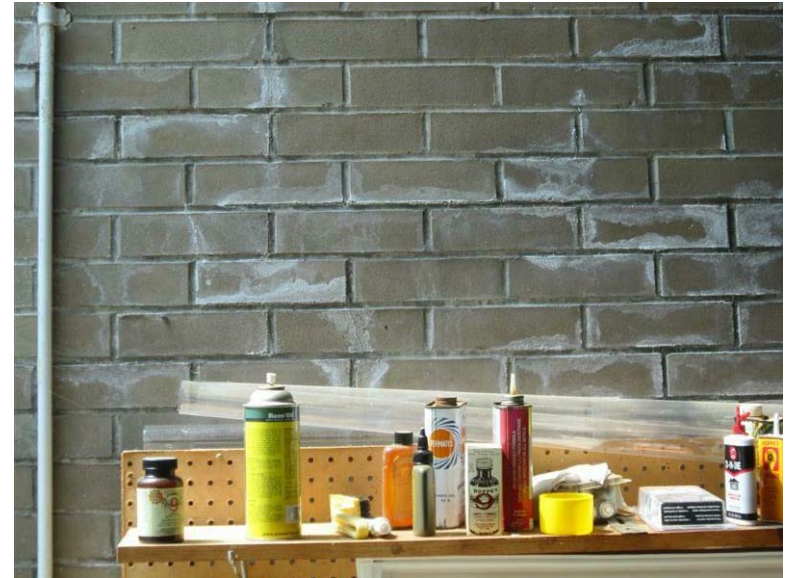
17B - Service Building: Efflorescence is visible on the brick wall.
