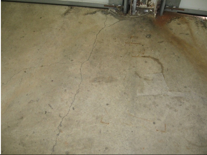
2009 Photo #7: Cracks in slab at vehicle storage area
