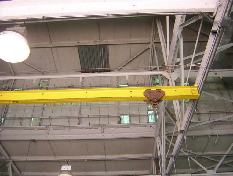
Building 42 – Pipe Shop: Some concrete ceiling panels have been replaced with metal panels.
