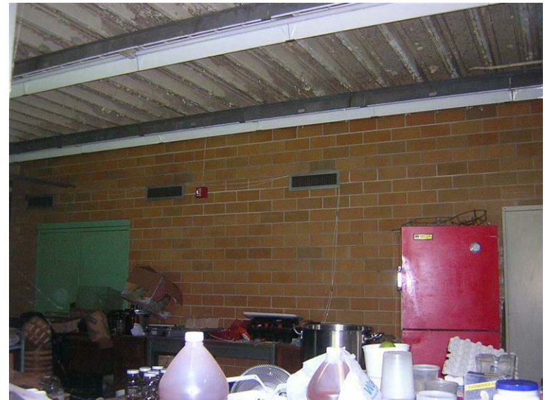
Building 118 – Greenhouse A: Paint is flaking from the metal ceiling.
