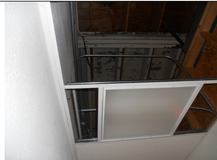
2013 Photo #10: Repairs to roof deck visible above partially removed lay-in ceiling
