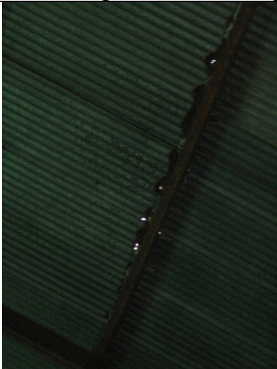
2009 Photo #17: Holes in metal roof deck
