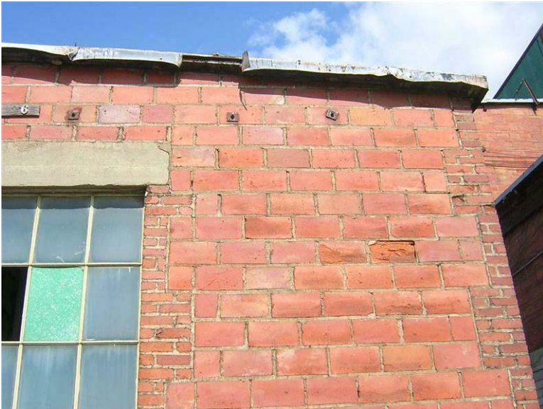
Building 68 – Substation No. 4: Hollow clay tile is spalling on the west facade and the metal coping is damaged.
