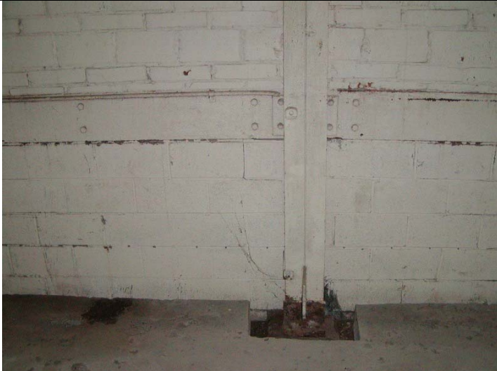
2009 Photo #9: Box-out in topping slab at column
