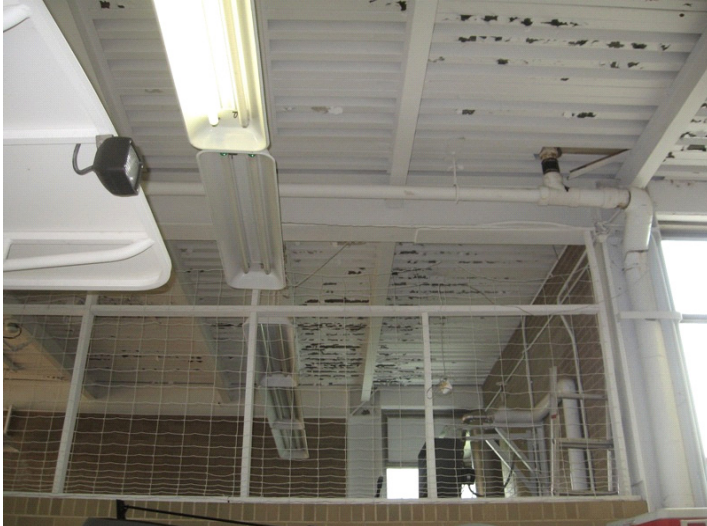
2009 Photo #3: Flaking paint at metal deck in vehicle storage area
