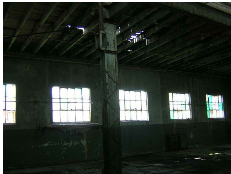
Building 53 – Tin Shop: Daylight is shining through holes in the roof decking.
