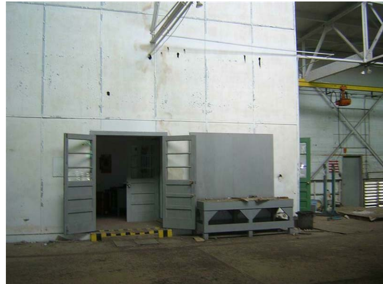
Building 71 – Catalyzer Building No. 3: Paint is flaking from the interior partition wall, which has several holes.
