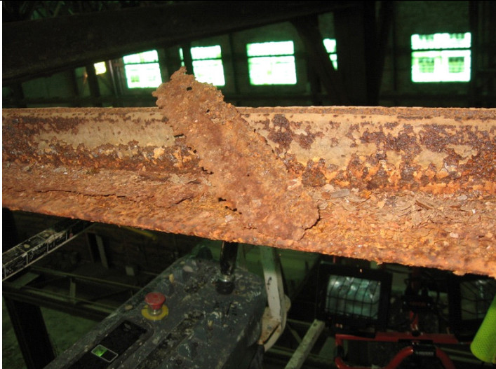
2009 Photo #7: Severely corroded steel framing
