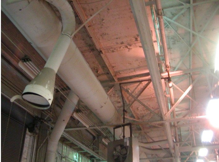
2009 Photo #17: Surface deterioration at concrete plank deck
