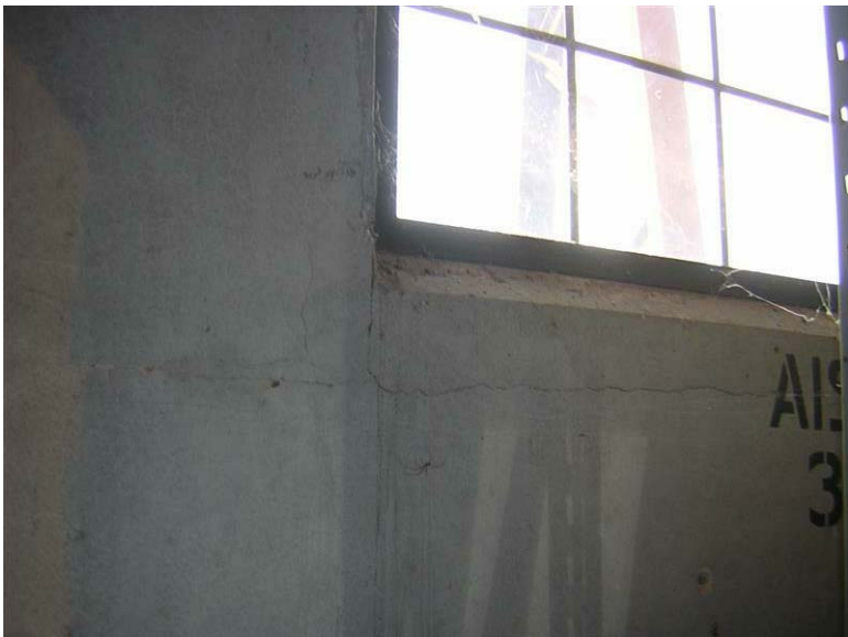
Building 44 – Project Operations Bath House: A horizontal crack is visible on the south wall beneath the sill in the storage area.
