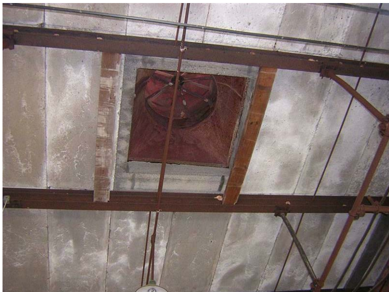
Building 68a – Substation No. 5: The steel structure is rusted.
