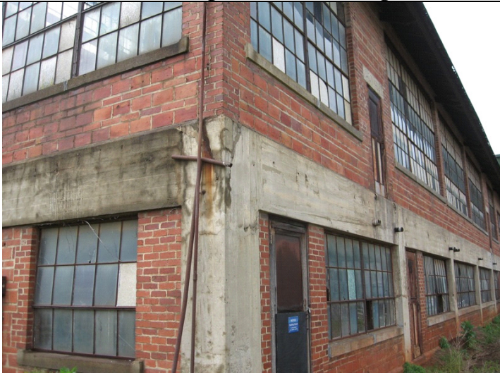
2009 Photo #3: Exterior cracks in concrete mezzanine frame at Southeast corner
