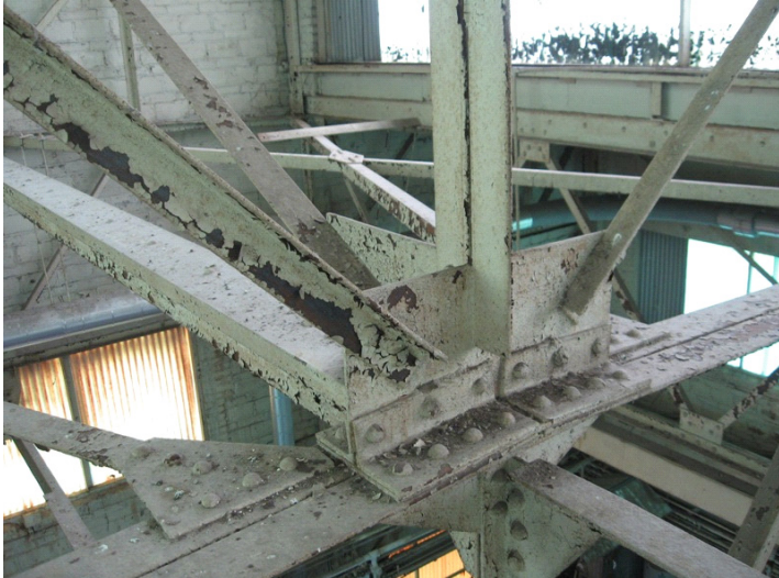
2009 Photo #19: Flaking paint at corroded steel roof framing
