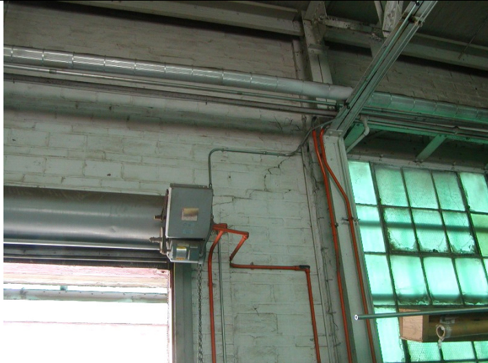
2009 Photo #9: Example of diagonal crack in masonry at overhead doors
