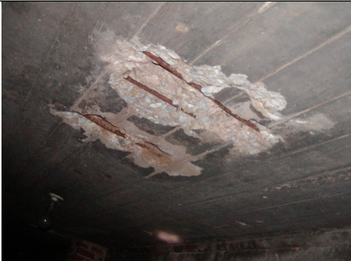
2009 Photo #18: Severely spalled concrete at basement ceiling
