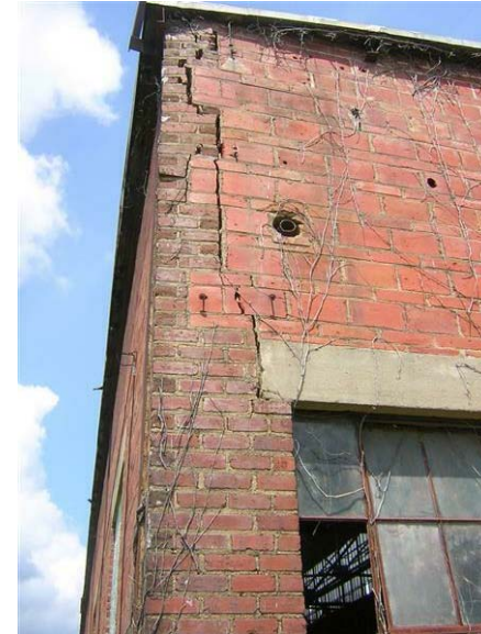
Building 74 – Catalyzer Building No. 6: The wall is cracked along the brick quoins.
