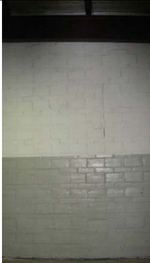
2009 Photo #37: Interior crack in East wall.
