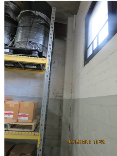
2013 Photo #50: Southeast corner column. Severe cracking of brick observed. Post installed tie back installed.
