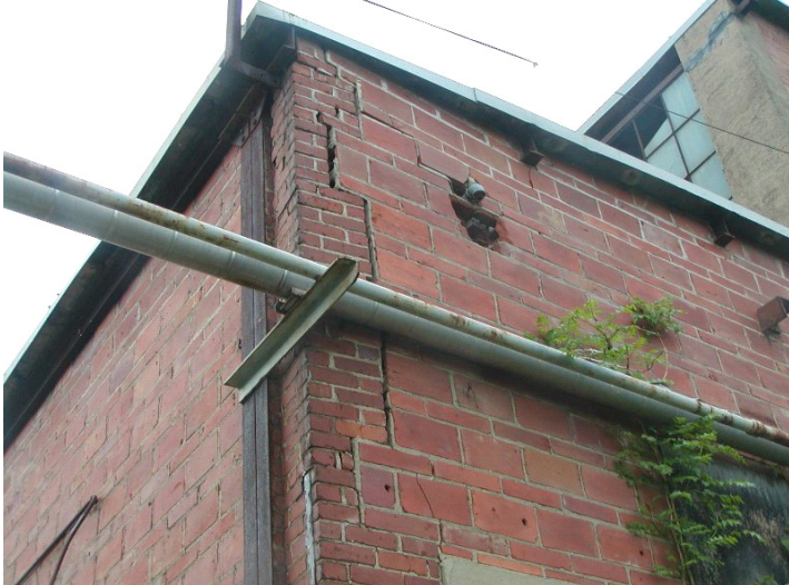
2009 Photo #3: Cracked and partially dislodged masonry at Southeast corner
