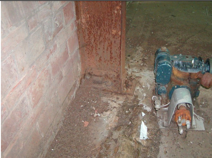
2009 Photo #8: Severely corroded steel framing
