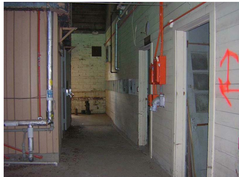
Building 72 – Catalyzer Building No. 4: The infill consists of wood stud walls clad in horizontal wood panels and metal panels.
