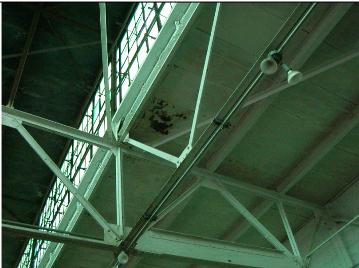
2009 Photo #10: Deteriorated concrete plank at roof deck
