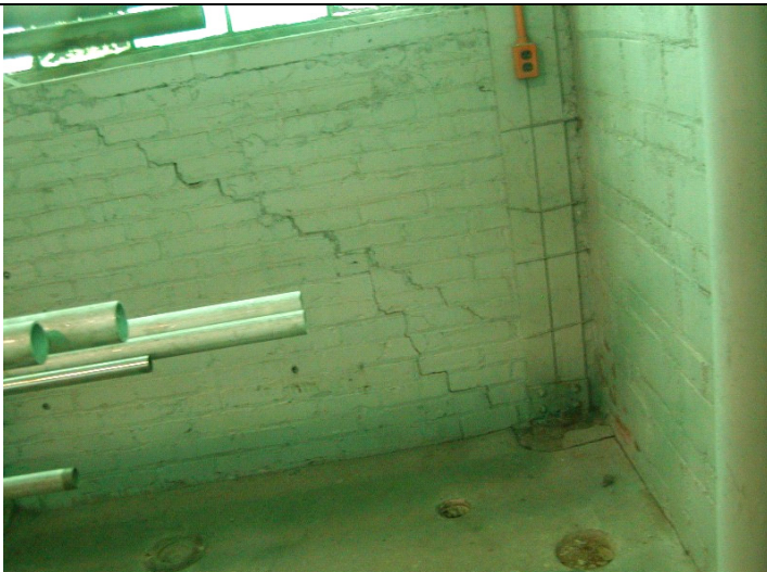
2009 Photo #12: Diagonal crack in masonry at corner of building below window
