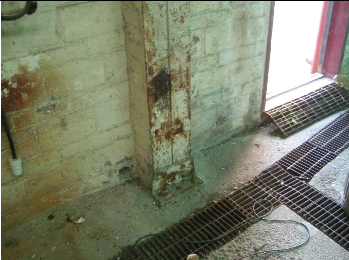
2009 Photo #14: Corroded steel column and deteriorated steel trench grates at South side of main building
