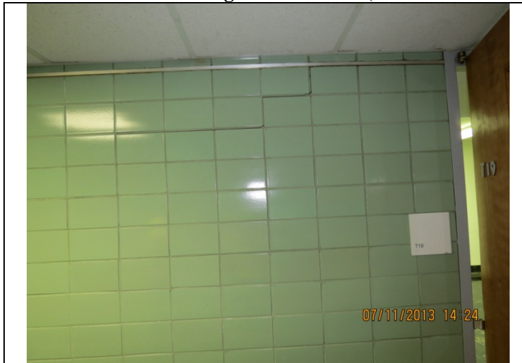
2013 Photo #13: Outside room T19 (Unoccupied): Stair step crack observed at interior wall.
