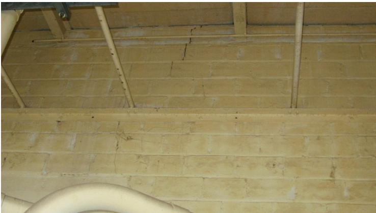
2009 Photo #6: Cracks in masonry – West wall
