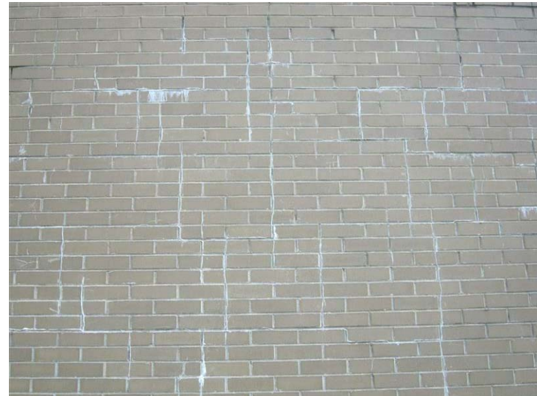
17B - Service Building: Significant thermal cracking and efflorescence is visible on the sawtooth walls.
