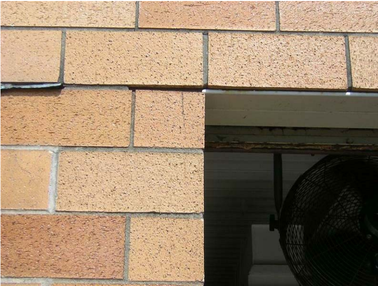
Building 118 – Greenhouse A: The lintels are rusting at the bearing points.
