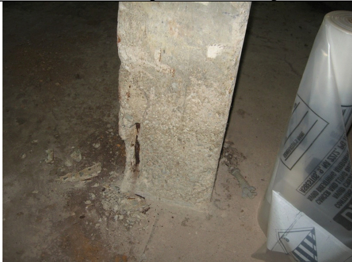
2009 Photo #21: Severely spalled mezzanine concrete column
