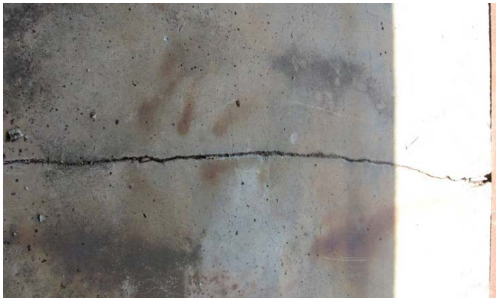
2009 Photo #26: Crack in South loading dock slab.
