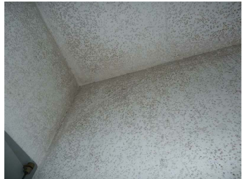
17B - Service Building: Mold and mildew are prevalent in the basement.
