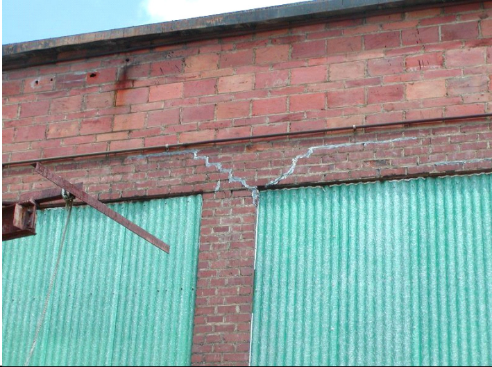
2009 Photo #9: Cracks in masonry lintels at South wall
