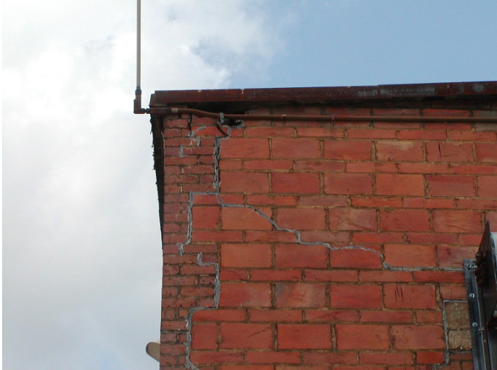
2009 Photo #5: Cracks in masonry at Southeast corner
