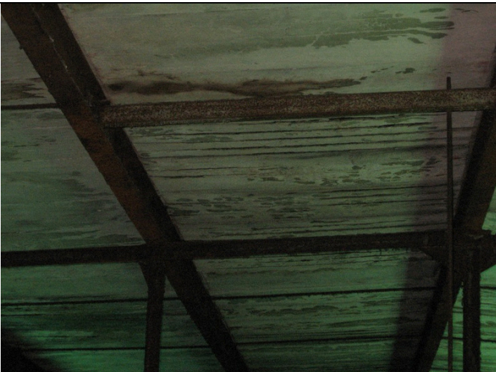
2009 Photo #8: Ruined concrete roof planks
