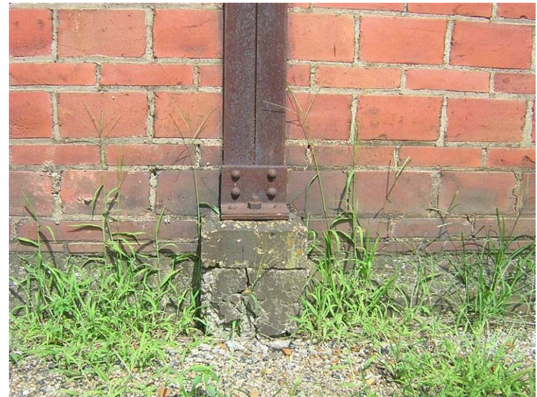
Building 71 – Catalyzer Building No. 3: The concrete footing is broken.
