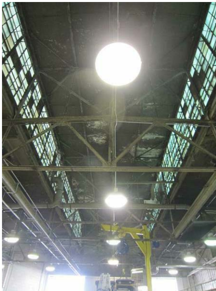
Building 38 – Machine Shop - Gas and Diesel Repair Shop: A majority of the concrete ceiling panels are damaged.
