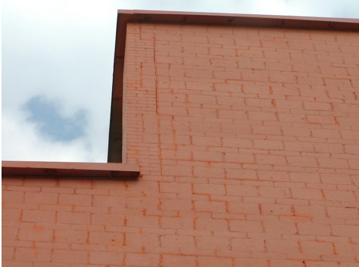
2009 Photo #5: Crack in masonry at end wall East side
