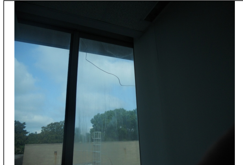
2013 Photo #18: Cracked window in unoccupied space.
