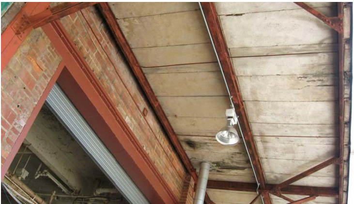
2009 Photo #8: Deteriorated concrete roof plants at North canopy.
