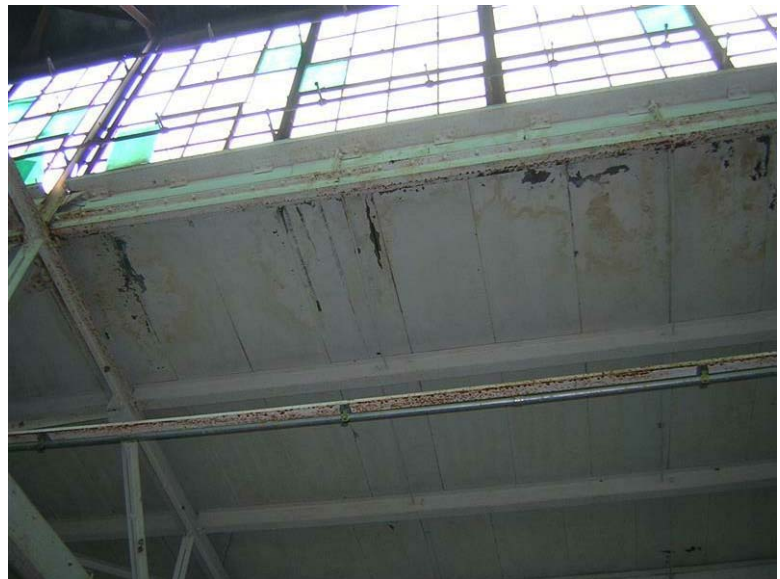
Building 71 – Catalyzer Building No. 3: Water infiltration has stained the concrete ceiling tiles.
