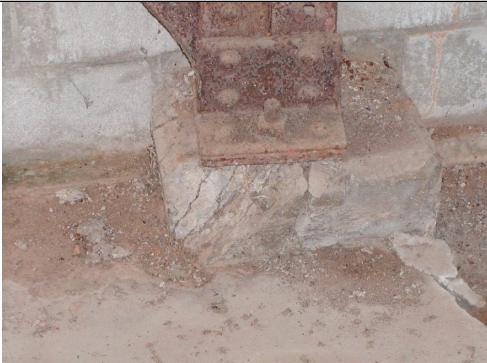
2009 Photo #8: Close-up of deteriorated column attachment at concrete pier
