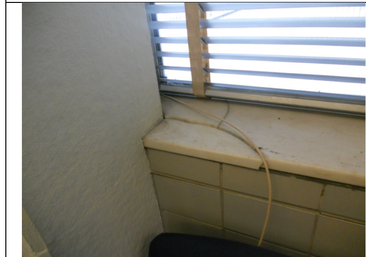
2013 Photo #20: Unoccupied: Broken marble window sill apparently caused by thermal expansion
