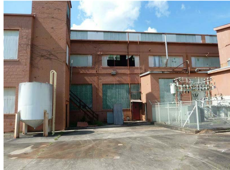
Building 39 – Engineering Lab: The fiberglass panels covering the windows are torn and missing in some areas, exposing the interior to moisture.
