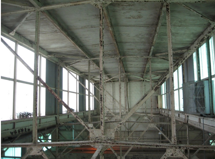
2009 Photo #15: View of monitor framing and roof deck
