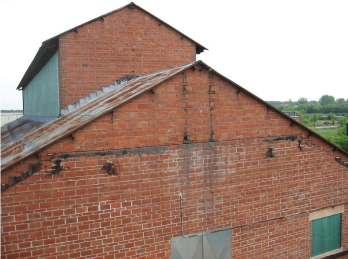
2009 Photo #5: Exterior building South end where track shed was originally attached
