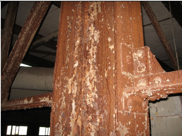
2009 Photo #14: Severely corroded structural steel
