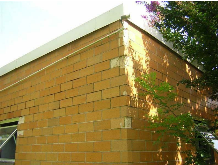
Building 118 – Greenhouse A: Localized spalling has occurred in the tiles at this corner of the building.
