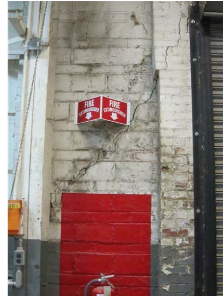
Building 37 – Machine Shop: Severe cracking between the door and window openings.
