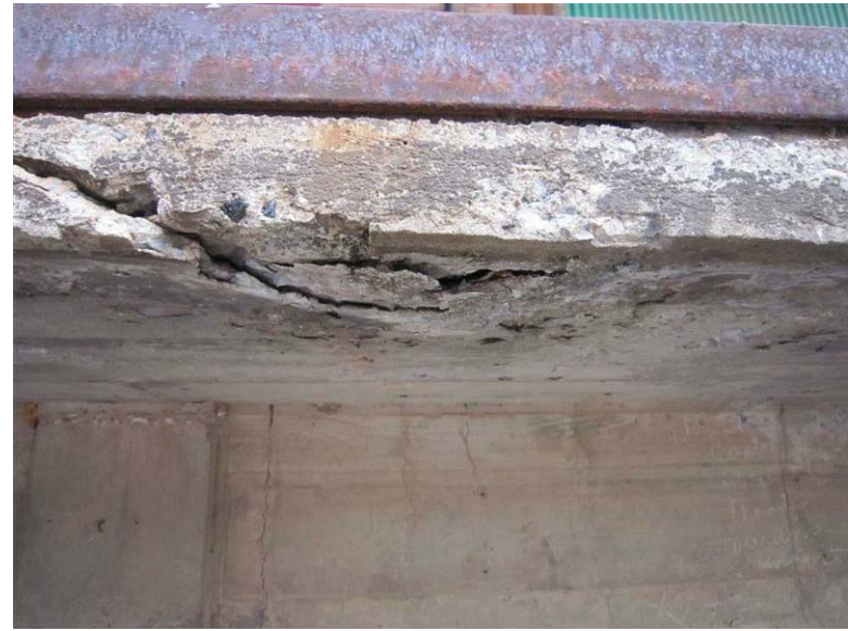
Building 33, 34, 35, 36 – Chemical Plant Warehouse: Concrete at the loading dock is cracking.
