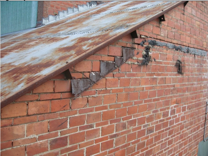
2009 Photo #6: Detail view of where track shed roof was attached to building
