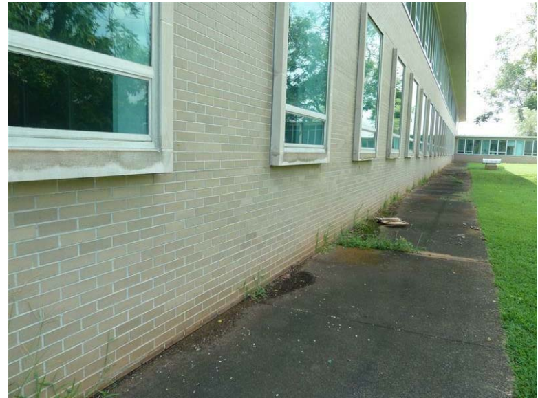
Building 17A - Environmental Research Center: Moisture has collected at the sills where the walkway abuts the buildings on the west elevation.
