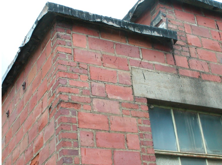
2009 Photo #3: Minor spalls in exterior masonry
