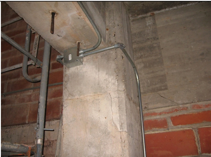
2009 Photo #18: Cracked concrete column at East mezzanine
