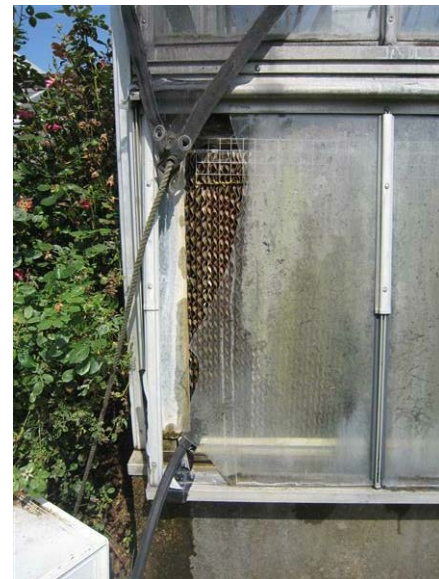
Building 118 – Greenhouse B-D: Localized broken panes occur in the glazed walls.
