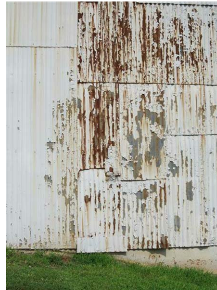
Building 24 – Warehouse No. 4: Rusting occurs and the paint is flaking from the corrugated metal panels.
