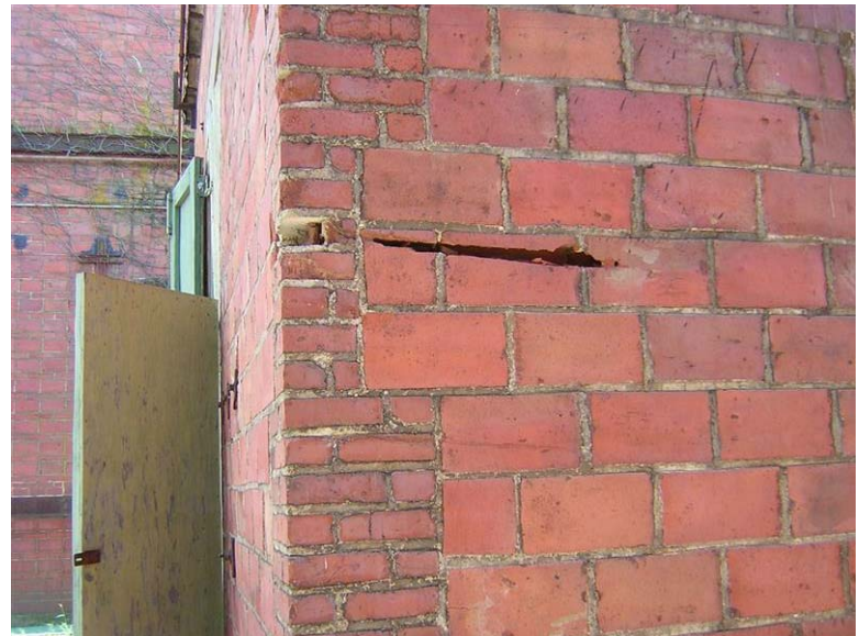
Building 68 – Substation No. 4: The hollow clay tile and brick is damaged at the northeast corner.
