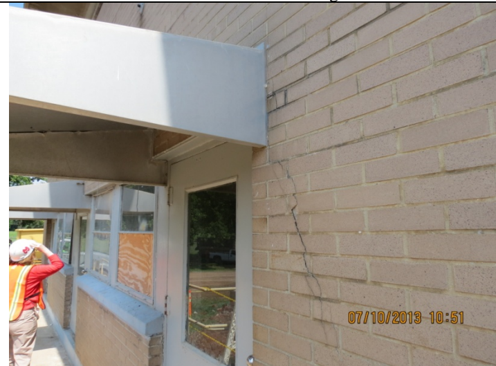
2013 Photo #12: Crack in exterior masonry at awnings on South side of building.
