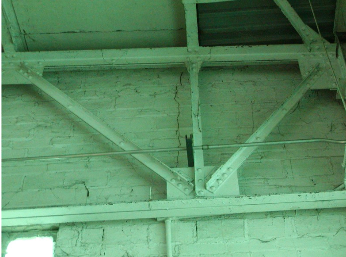
2009 Photo #11: Crack in masonry at end wall
