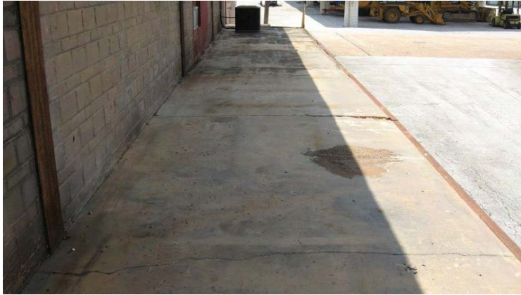
2009 Photo #25: Cracks in South loading deck slab.
