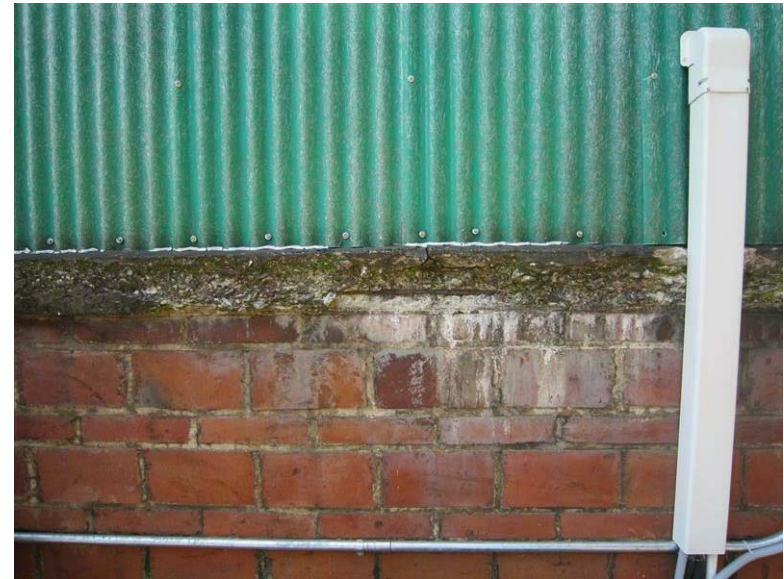
Building 37, 38 – Machine Shop: The concrete sill is deteriorating from water damage. Efflorescence and mold growth has collected on and beneath the window sill.
