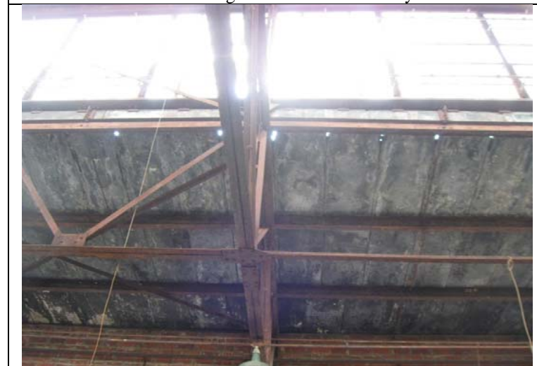
2013 Photo #6: Progressive deterioration of concrete plank roof deck was observed – note holes through deck below clerestory
