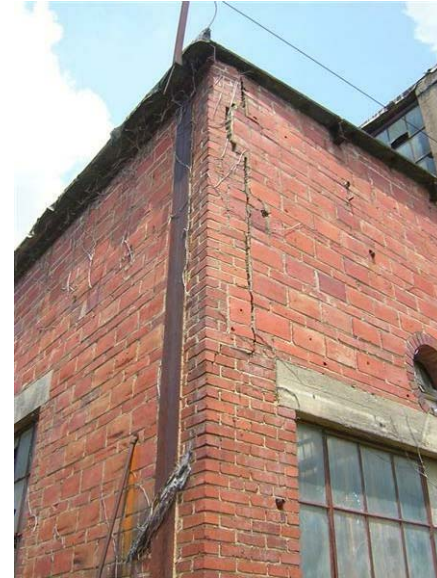
Building 73 – Catalyzer Building No. 5: Visible cracking is located along the quoins at the upper east facade.
