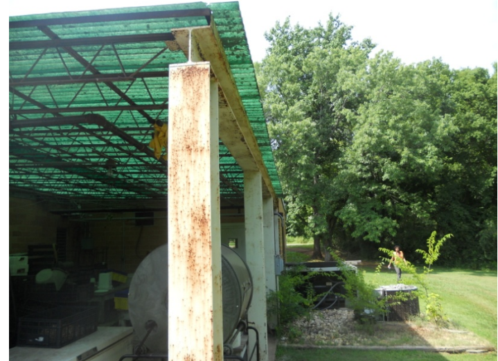
2013 Photo #4: Corroded steel exhibits progressive deterioration.
