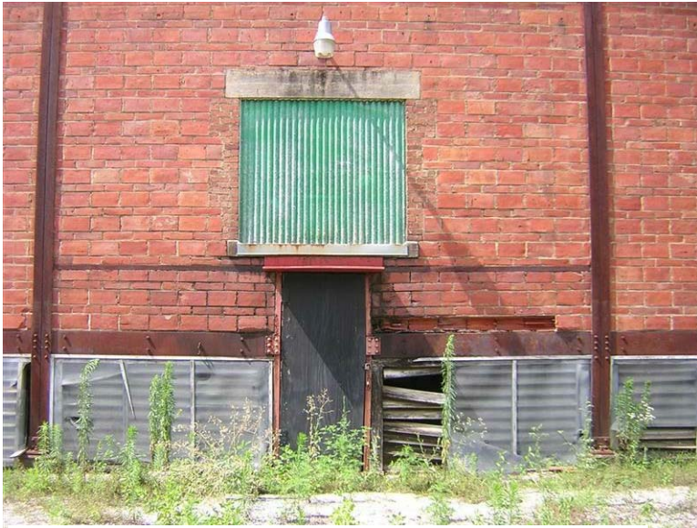
Building 71 – Catalyzer Building No. 3: Several wood louvers are broken and damaged.
