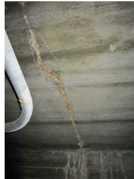
Building 01A - Chemical Feed House: There is a crack at the concrete beam of the second floor stair.
