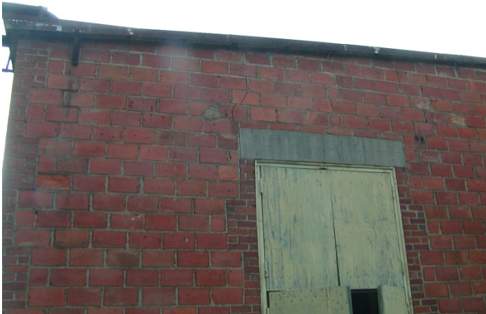
2009 Photo #2: Minor cracks in masonry at East wall of substation
