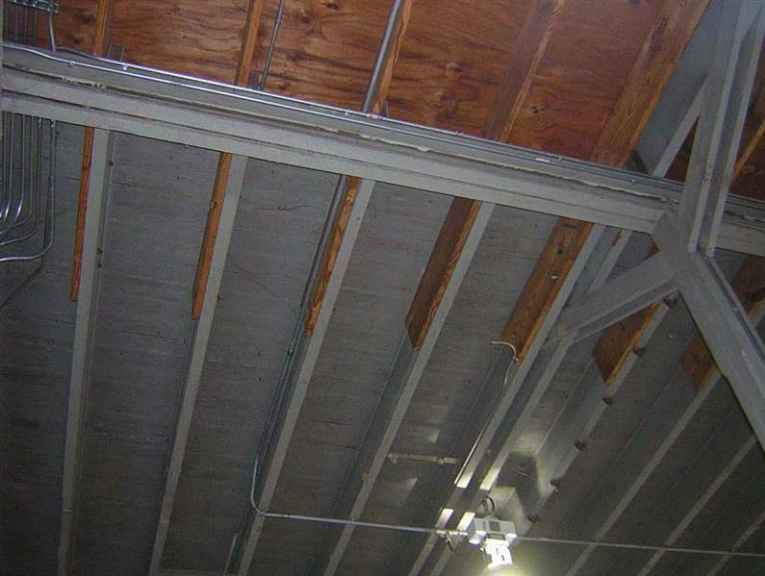
Building 44 – Project Operations Bath House: The wood decking has been partially replaced with plywood in the storage area. New wood structural members have been installed in portions of the roof.
