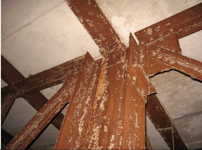
2009 Photo #13: Severely corroded structural steel
