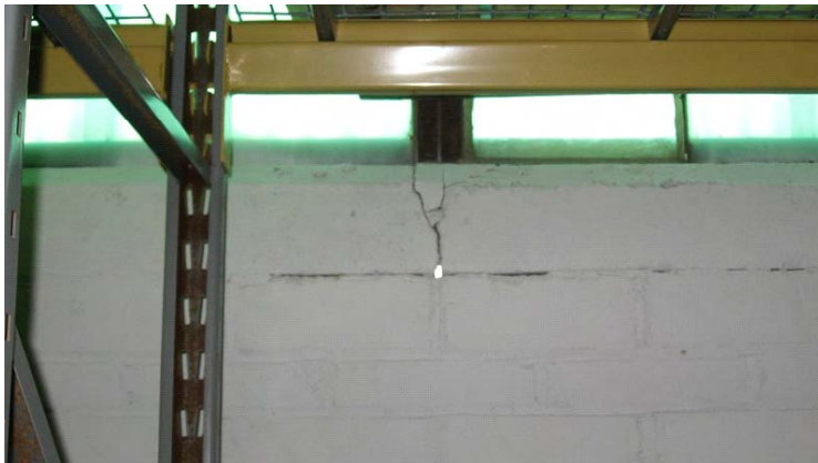
2009 Photo #36: Interior crack/void at window sill on South side near East end.
