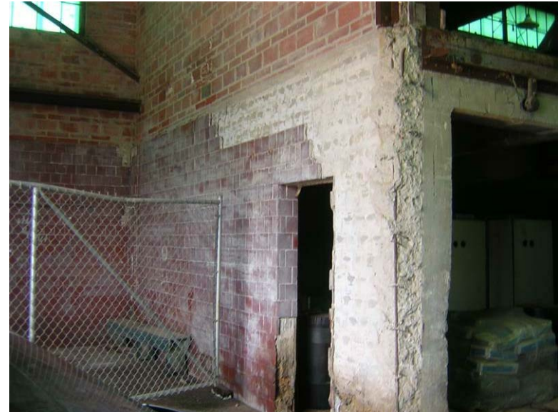
Building 79 – 3A – Nitrate House: Several tiles have detached from the concrete wall and rebar is exposed at the corner.
