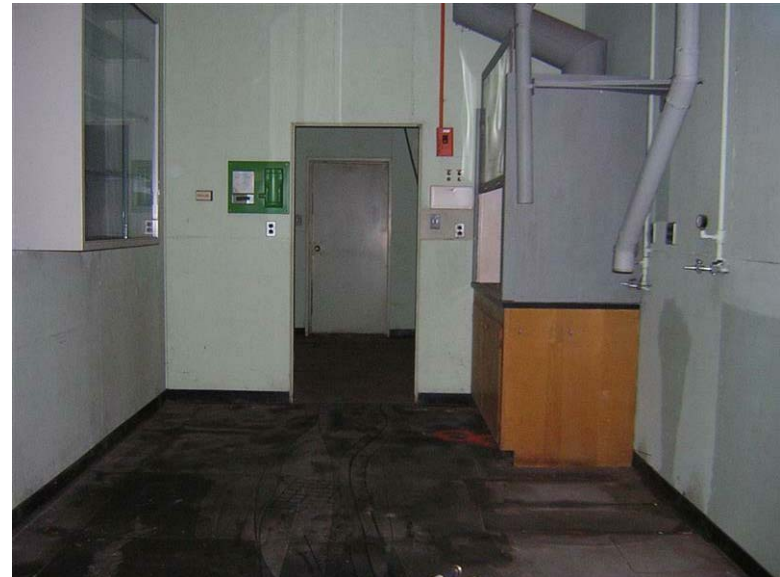
Building 72 – Catalyzer Building No. 4: The floor tiles in the hallway are damaged from moisture.
