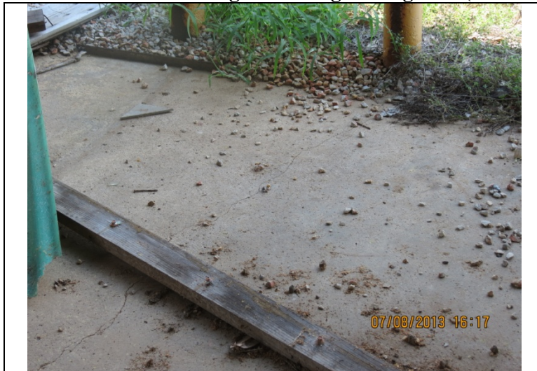
2013 Photo #21: East end of extension, crack in slab on grade perpetuates across entire width of structure.
