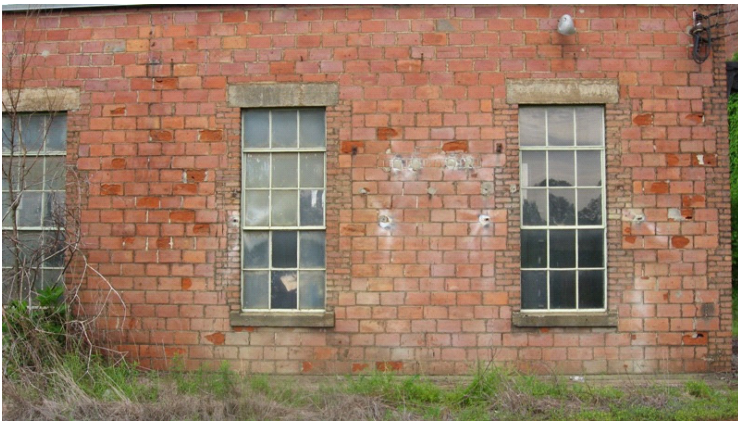
2009 Photo #2: Multiple surface spalls in exterior masonry – East side
