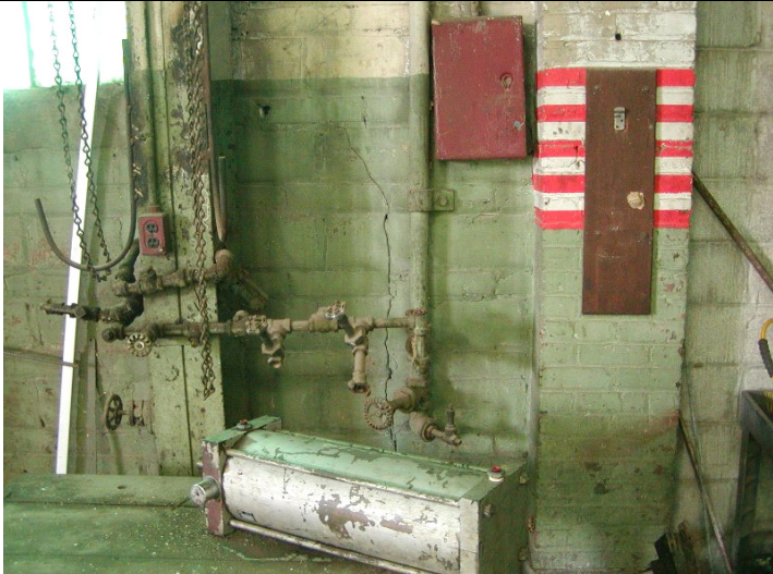
2009 Photo #23: Vertical crack in masonry at South wall
