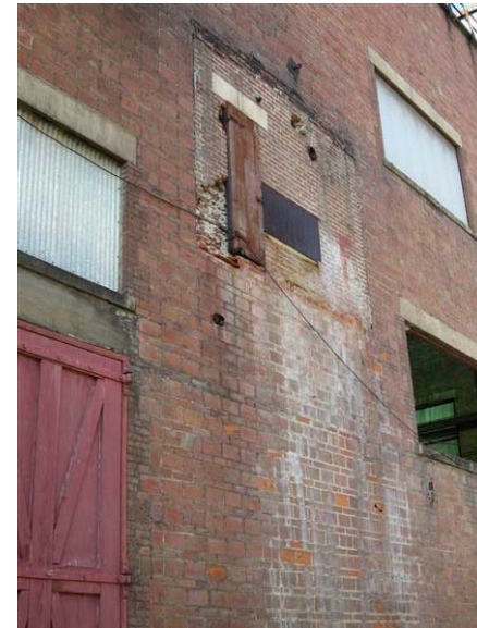
Building 26 – L / N Building Grounds Maintenance Shop: Efflorescence, spalling masonry and eroded mortar joints where water is flowing down the face of the building.
