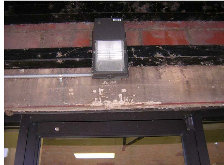
Building 44 – Project Operations Bath House: The concrete lintel is chipped at the main entrance on the west facade.
