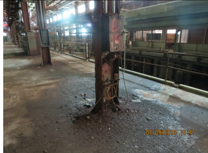
2013 Photo #5: Severely corroded steel column. Above is disconnected roof drain that empties water into the building.
