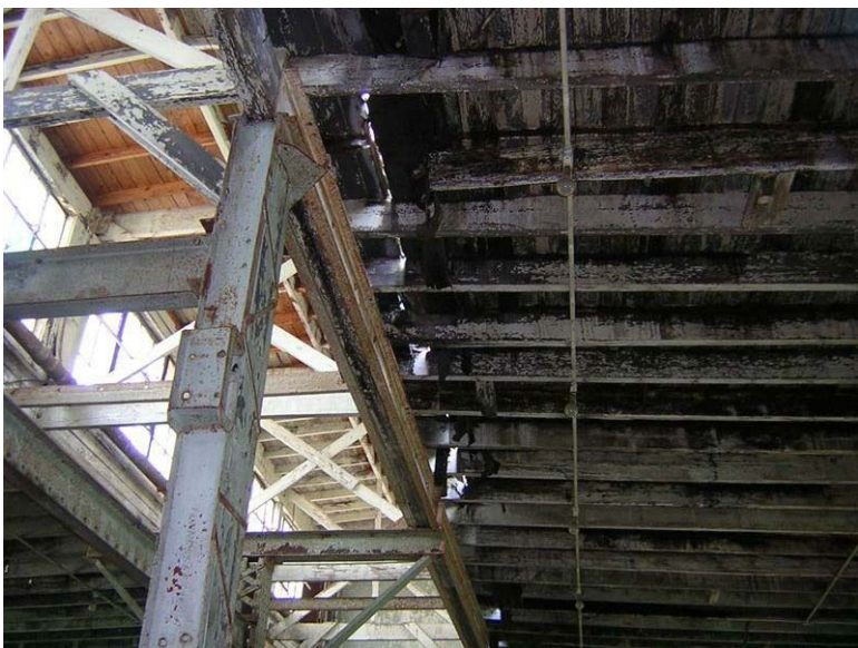
Building 53 – Tin Shop: The roof is stained from water damage.
