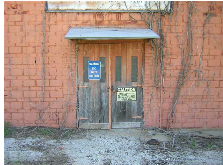
Building 53 – Tin Shop: Paint is flaking from the wooden doors.
