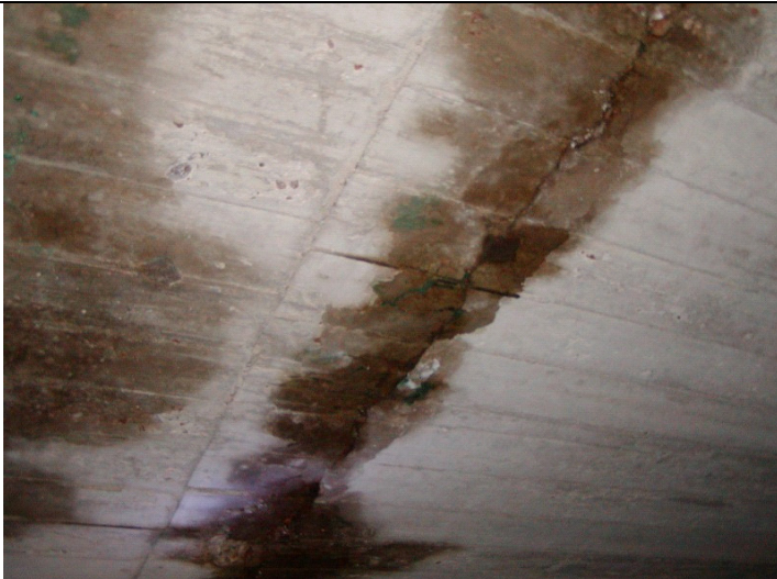
2009 Photo #16: Defective concrete at basement ceiling
