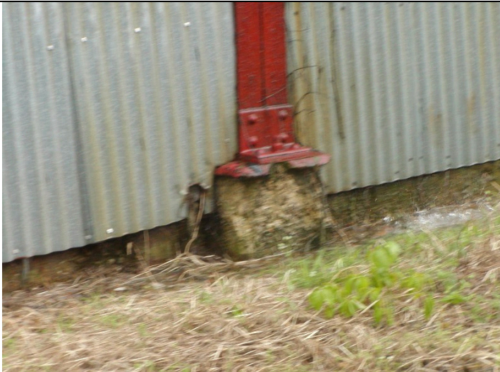
2009 Photo #6: Deteriorated concrete pier at column
