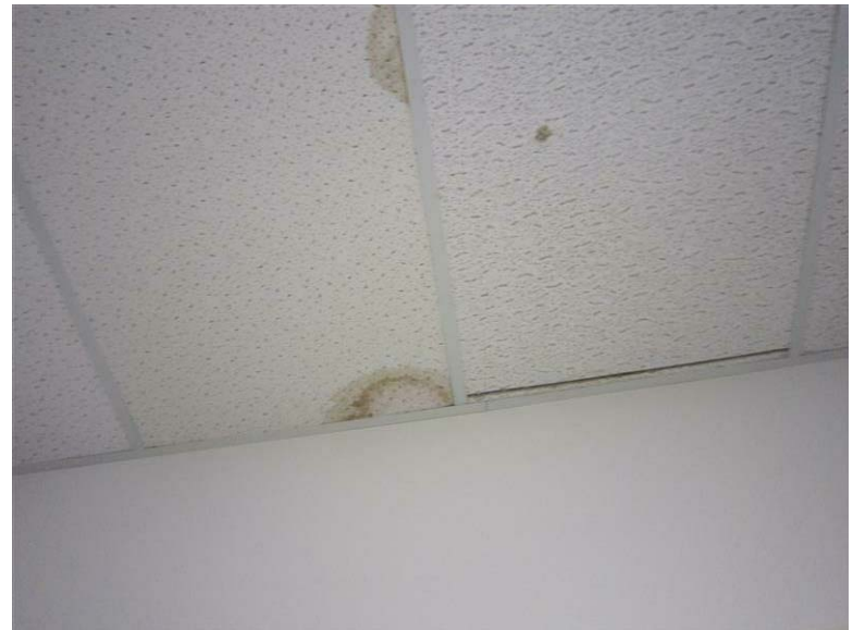
Building 25 – L / N Warehouse Z: Evidence of water infiltration is visible on the acoustical ceiling tiles.
