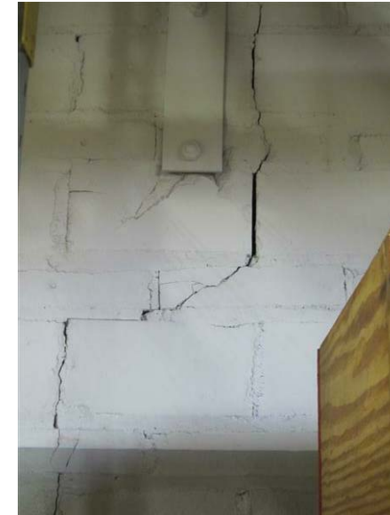
Building 36 – Chemical Plant Warehouse - Projects Operations Storage Warehouse: Severe cracking is separating the wall adjacent to this anchor.
