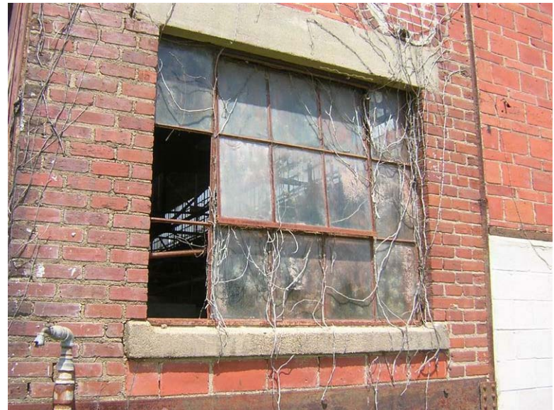
Building 74 – Catalyzer Building No. 6: Panes are missing in several of the steel windows.
