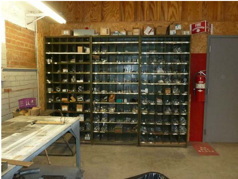
Building 34 – Chemical Plant Warehouse - Instrumentation / Electric Shop: An unfinished wood stud and plywood partition wall was built to enclose the space.
