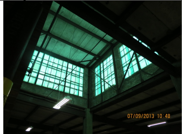
2013 Photo #45: Concrete roof planks at clerestory monitor. Different location than 2009 photo.
