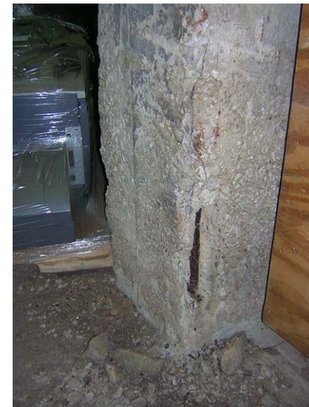
Building 79 – 3A – Nitrate House: Rebar is exposed and the concrete is deteriorating at this column.
