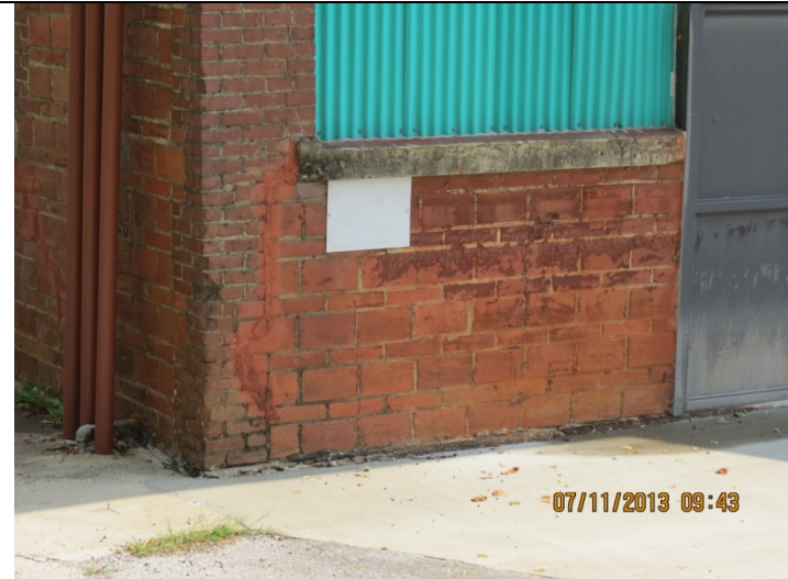
2013 Photo #6: Repaired cracks in masonry at Southwest corner
