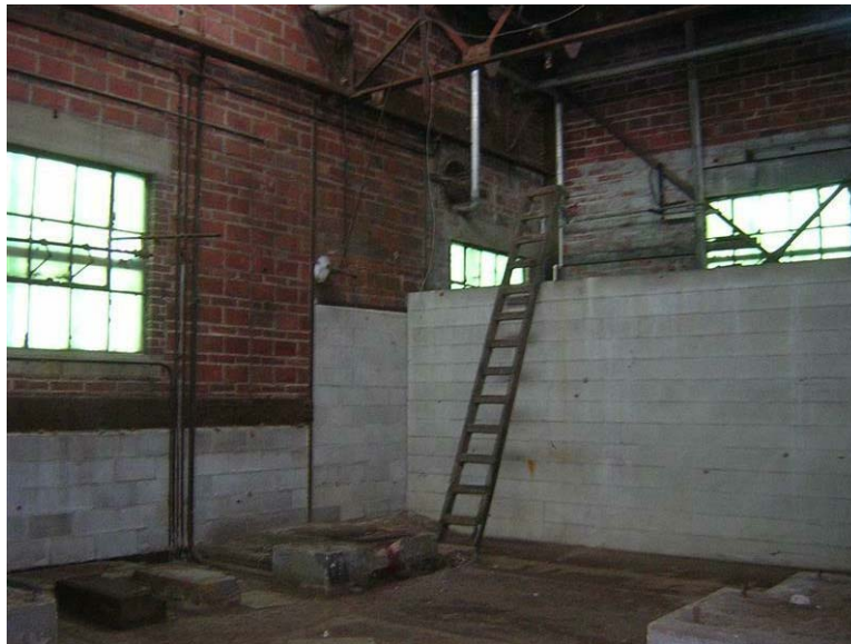
Building 69 – Catalyzer Building No. 1: CMU infill has replaced the wood louvers at the rear of the building.
