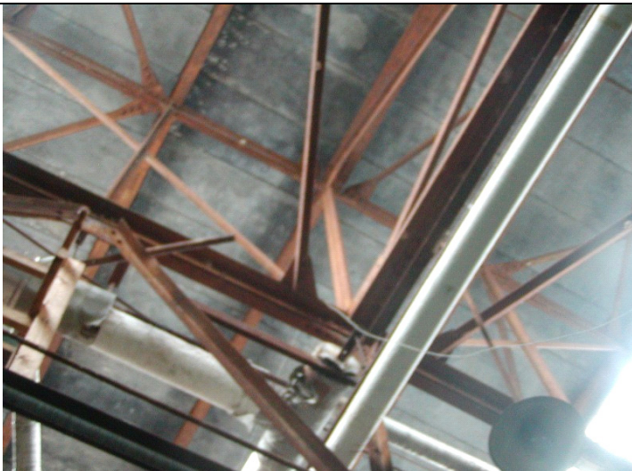
2009 Photo #8: Moderately corroded steel roof framing and surface deterioration on concrete plank roof deck
