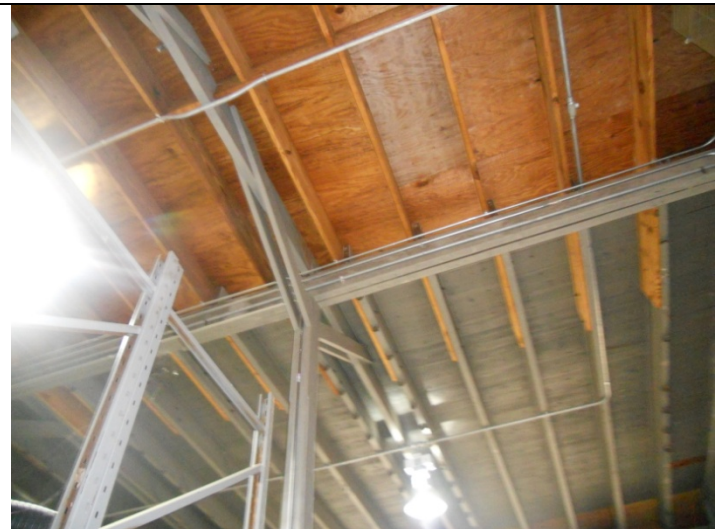
2013 Photo #6: Wood roof framing has been repaired and deteriorated portions of wood roof deck have been replaced
