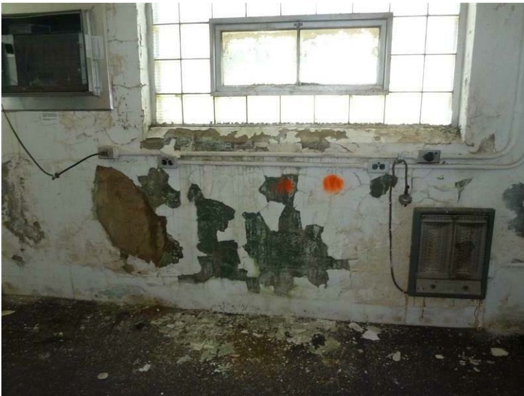
Building 39 – Engineering Lab: Water infiltration has severely damaged this plaster wall on the north facade.
