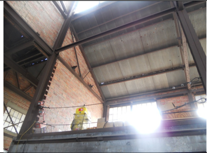
2013 Photo #7: More holes and more corrosion were observed on underside of metal roof deck
