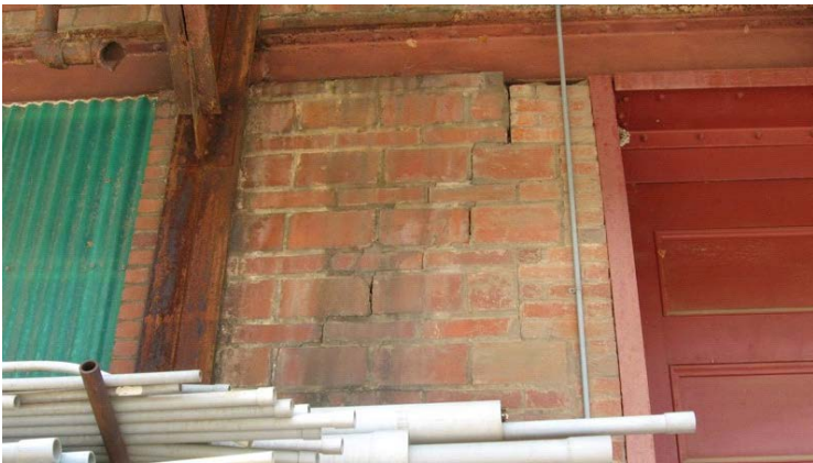
2009 Photo #18: Crack in exterior masonry below South canopy.
