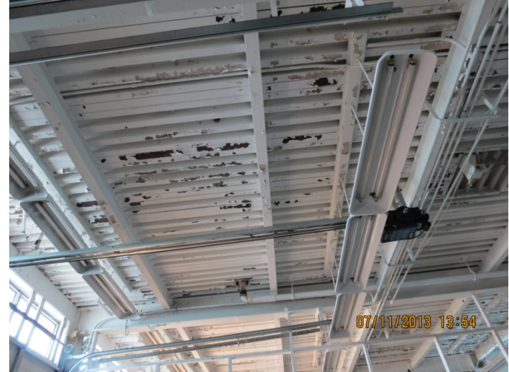
2013 Photo #3: Increased amount of flaking paint and corroded steel decking at vehicle storage area.
