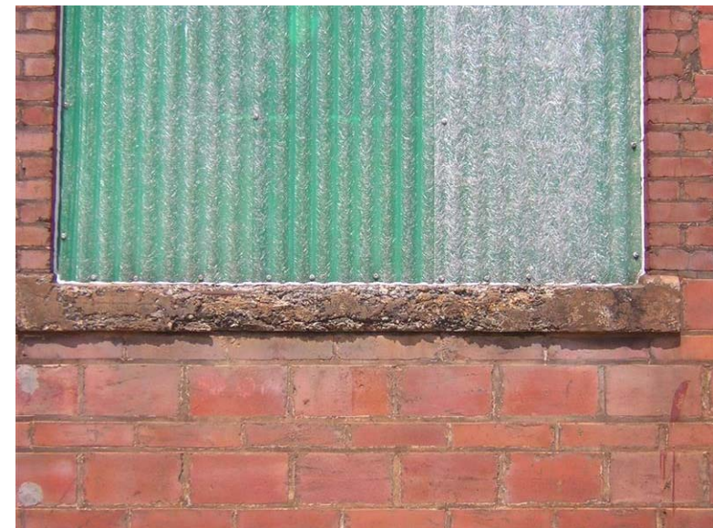
Building 41 – Sheet Metal Shop: Localized spalling of concrete sills is prevalent.
