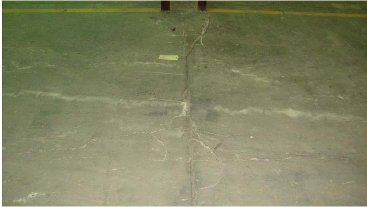
2009 Photo #33: Cracks in West area of second floor slab.
