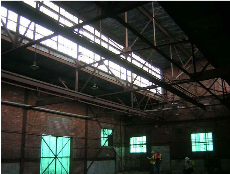
Building 74 – Catalyzer Building No. 6: The steel structure is rusted.
