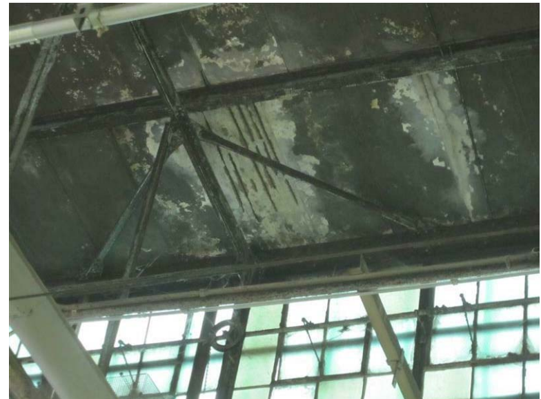
Building 38 – Machine Shop - Gas and Diesel Repair Shop: Several concrete ceiling panels are stained by moisture, which has damaged the concrete, exposing the rebar.
