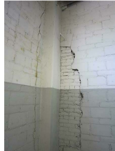
Building 36 – Chemical Plant Warehouse - Projects Operations Storage Warehouse: Severe cracking is visible at the exterior corners of the building.
