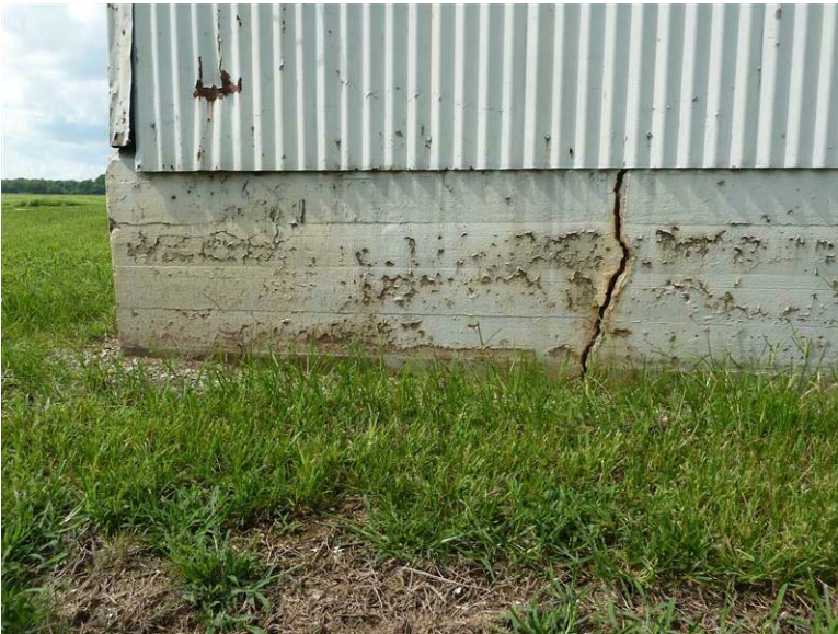
Building 24 – Warehouse No. 4: There is a large crack in the concrete foundation.
