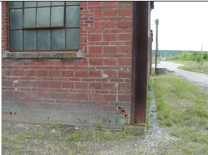
2009 Photo #14: Settlement cracks in masonry at Northwest corner
