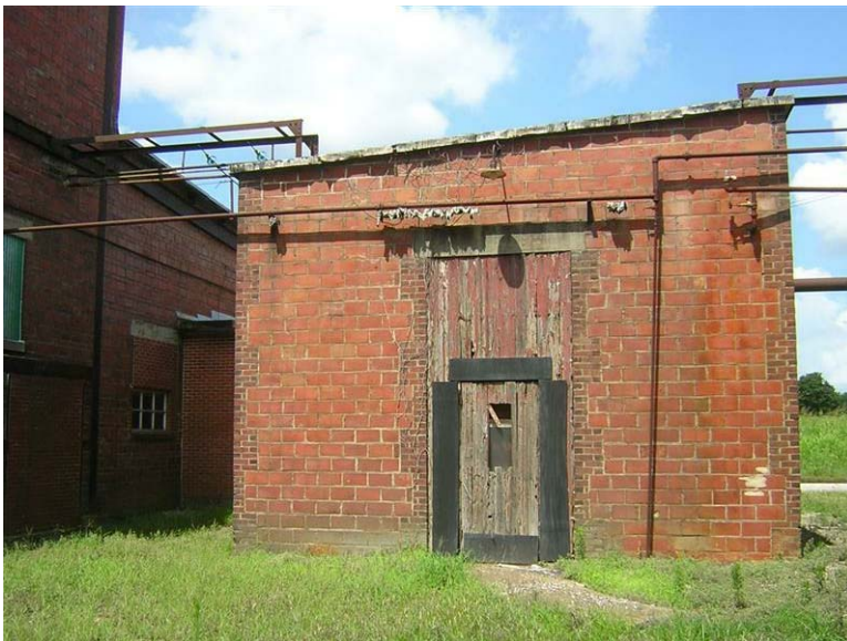
Building 74 – Catalyzer Building No. 6: Paint is flaking and the wood door is damaged at the adjoining substation.
