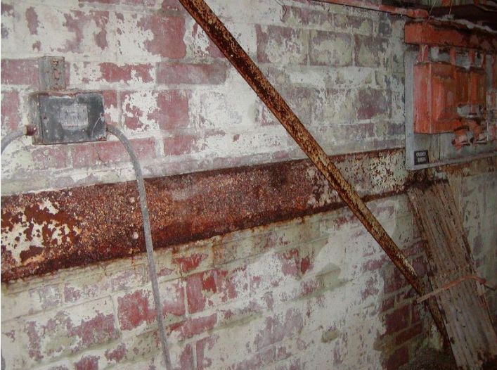
2009 Photo #11: Heavily corroded steel framing at North wall
