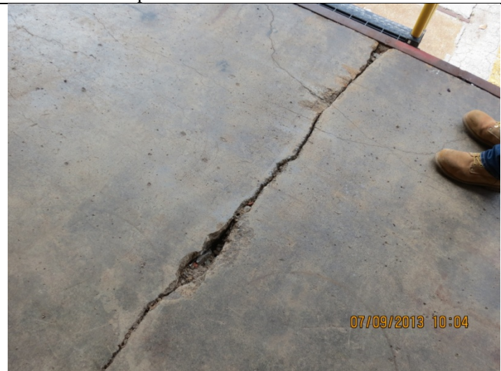
2013 Photo #26: Crack in South loading dock slab. Different location than 2009 photo.
