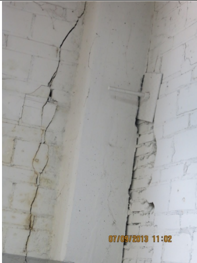
2013 Photo #49: Northeast corner column, Severe cracking of brick finishes observed. Post installed tie back installed.
