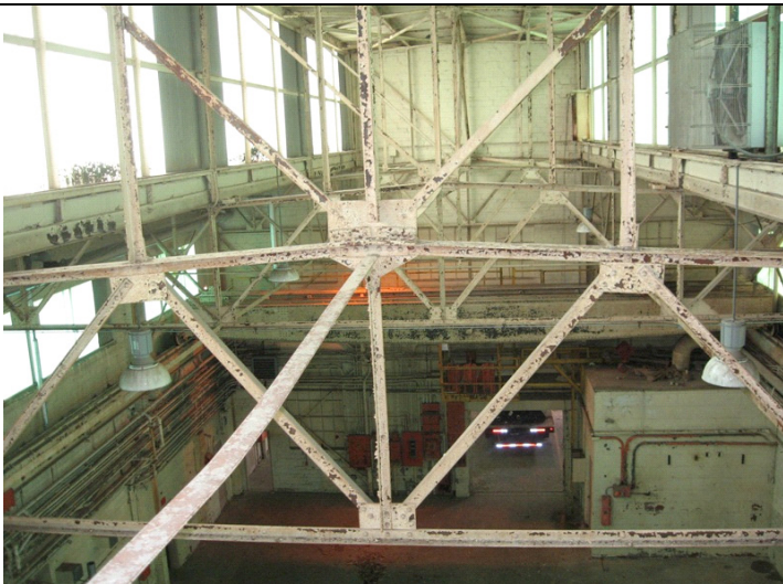
2009 Photo #16: View of steel roof trusses
