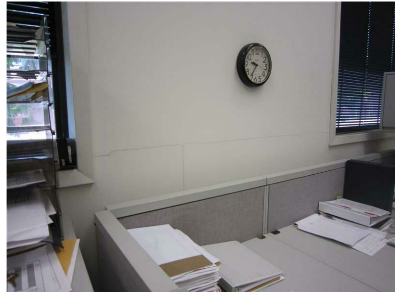
Building 25 – L / N Warehouse Z: Horizontal cracking is visible in the gypsum wallboard at the west end of the south room.
