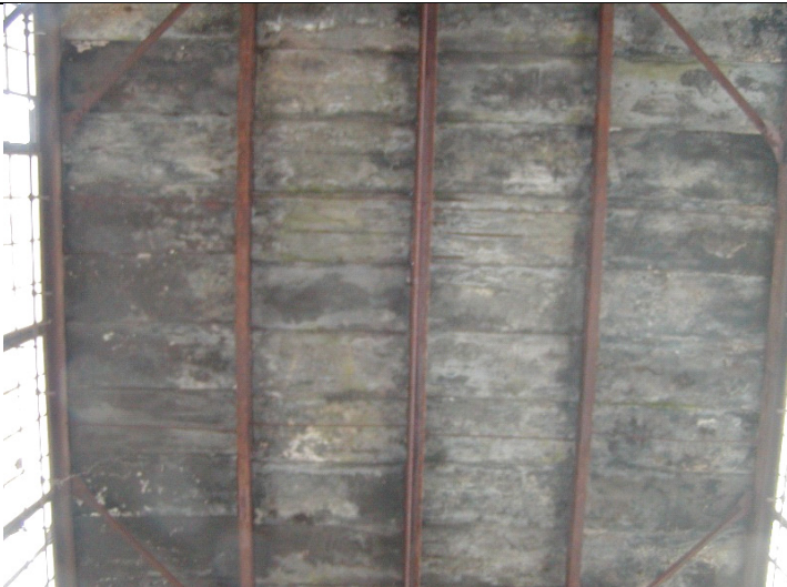
2009 Photo #8: Deteriorated concrete plank roof deck at monitor. Exposed reinforcing steel is visible
