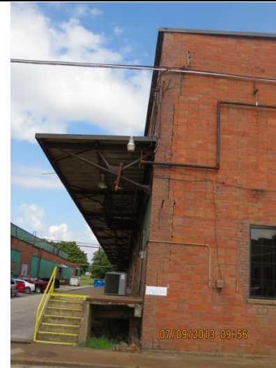
2013 Photo #22: Vertical crack in masonry on East side of Southeast corner. Additional movement observed.
