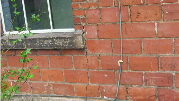
2009 Photo #3: Vertical cracks in masonry – West side
