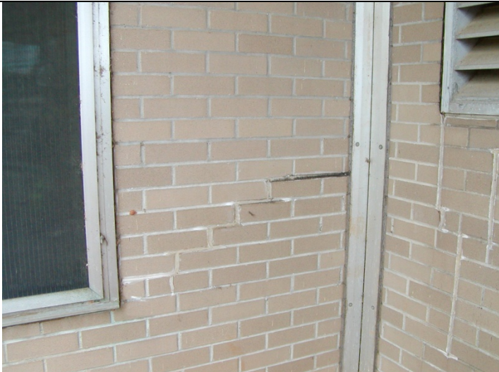
2009 Photo #8: Crack in wall near building entrance
