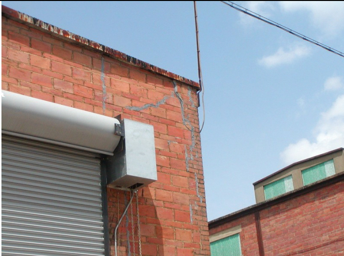
2009 Photo #10: Cracks in masonry North end of East wall
