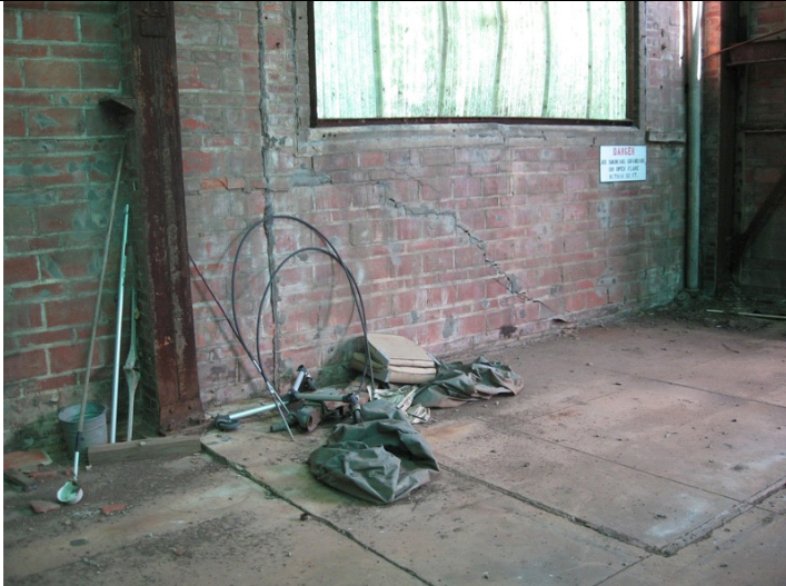
2009 Photo #21: Cracked masonry at outside wall
