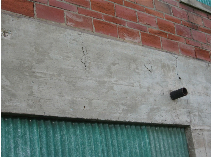
2009 Photo #9: Minor cracks and spalls in exterior face of mezzanine concrete frame
