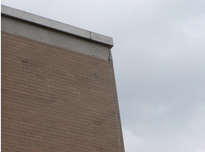
2009 Photo #6: Crack in corner at top of auditorium wall
