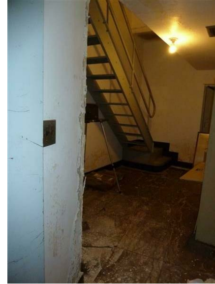
Building 17A - Environmental Research Center: A burst pipe has damaged the plaster wall, ceiling and floor tiles in the room at the rear of the auditorium.
