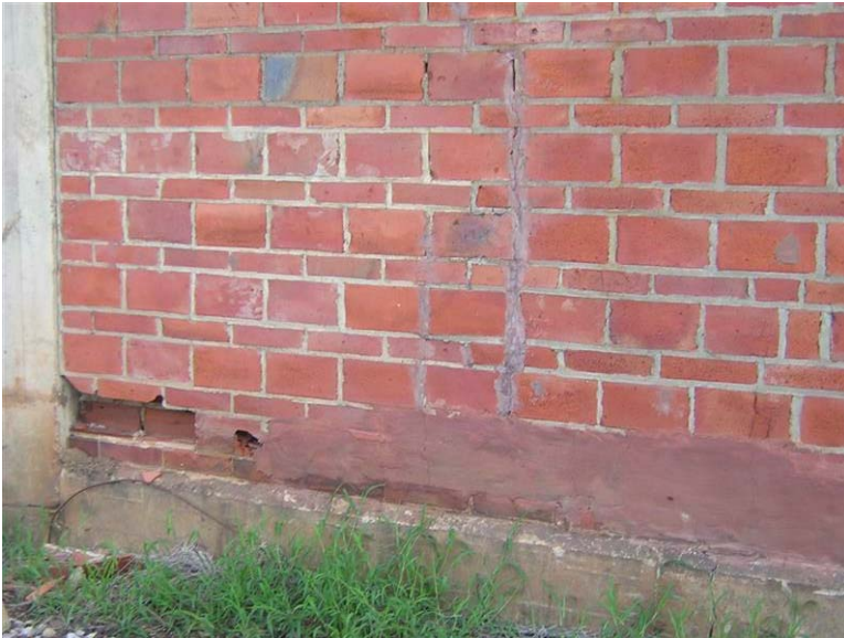
Building 79 – 3A – Nitrate House: Hollow clay tile at the base of this wall has been parged.
