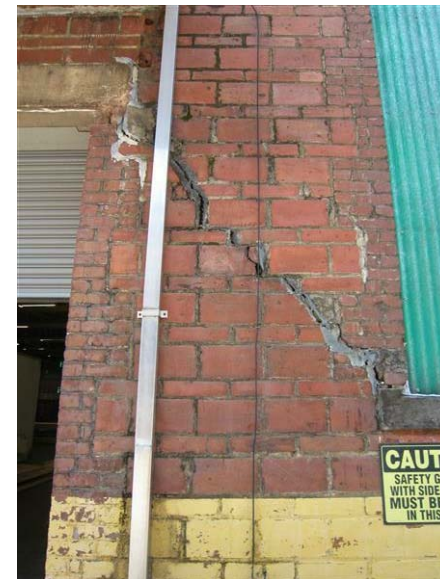
Building 37, 38 – Machine Shop: Although this crack was patched previously, it has continued to separate.
