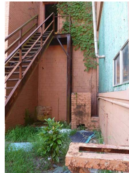
Building 39 – Engineering Lab: This exterior metal stair is severely rusted.
