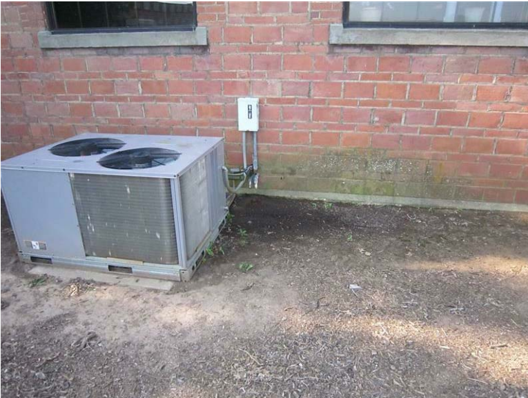
Building 25 – L / N Warehouse Z: There is evidence of water ponding by the HVAC units on the north wall.
