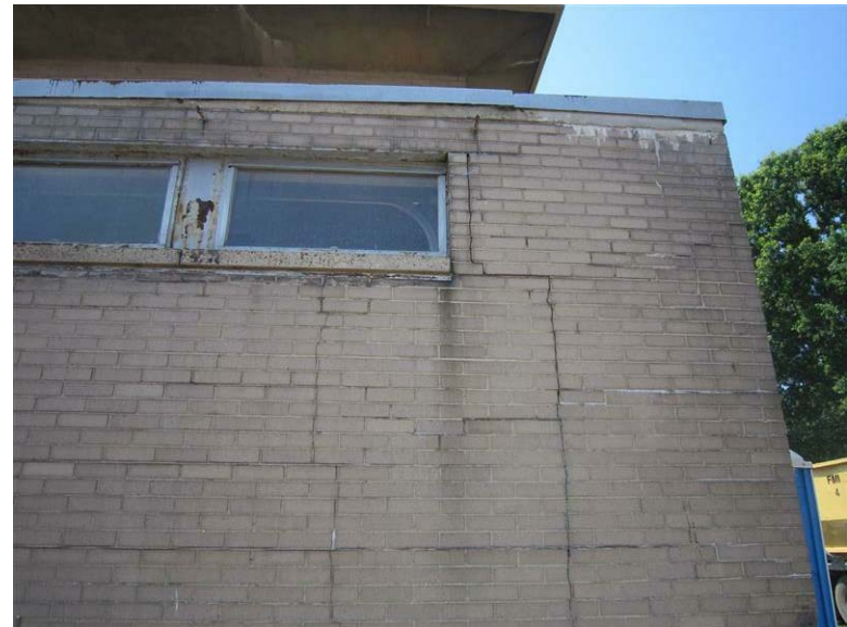
Building 01A - Chemical Feed House: Horizontal cracking is visible on the south facade adjacent to the large hole in ground.
