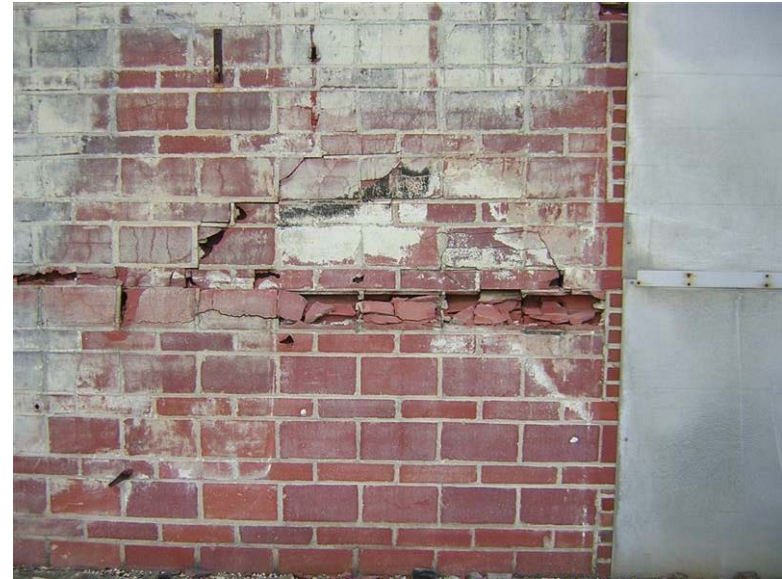
Building 70 – Catalyzer Building No. 2: The wall is caving in at the rear of the building.
