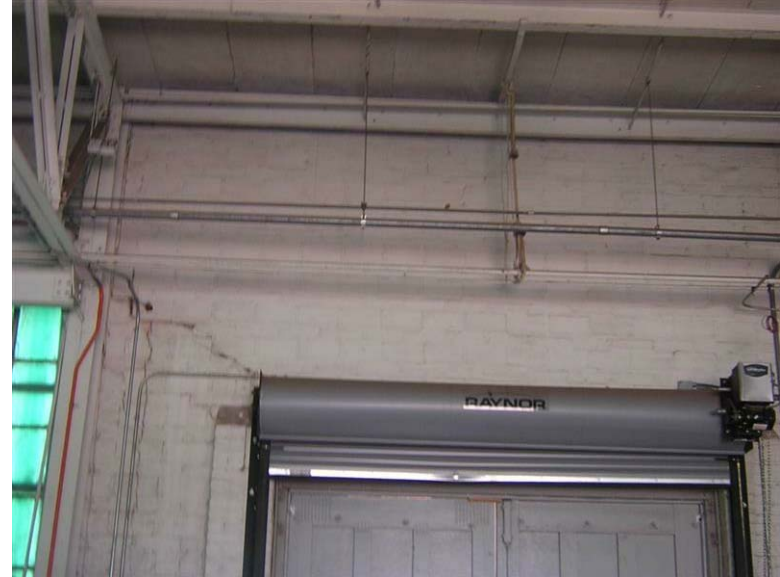
Building 42 – Pipe Shop: Diagonal cracking in the hollow clay tile is prevalent between window and door openings.
