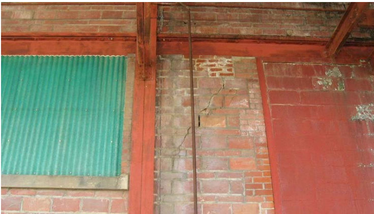
2009 Photo #6: Crack in exterior masonry below North canopy.
