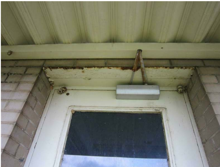
17B - Service Building: Rusting of exterior exposed structural steel.
