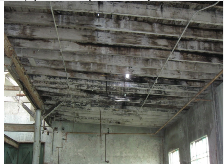
2013 Photo #4: Failure of framing members has begun to occur.
