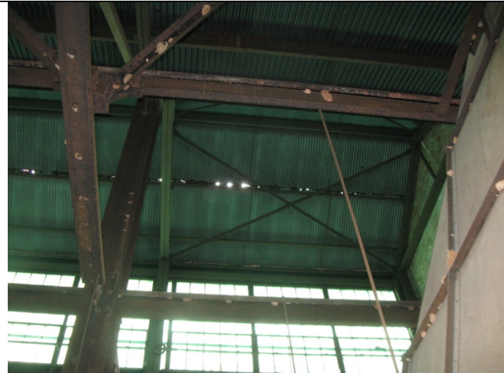
2013 Photo #17: More and larger holes were observed in metal roof deck in 2013
