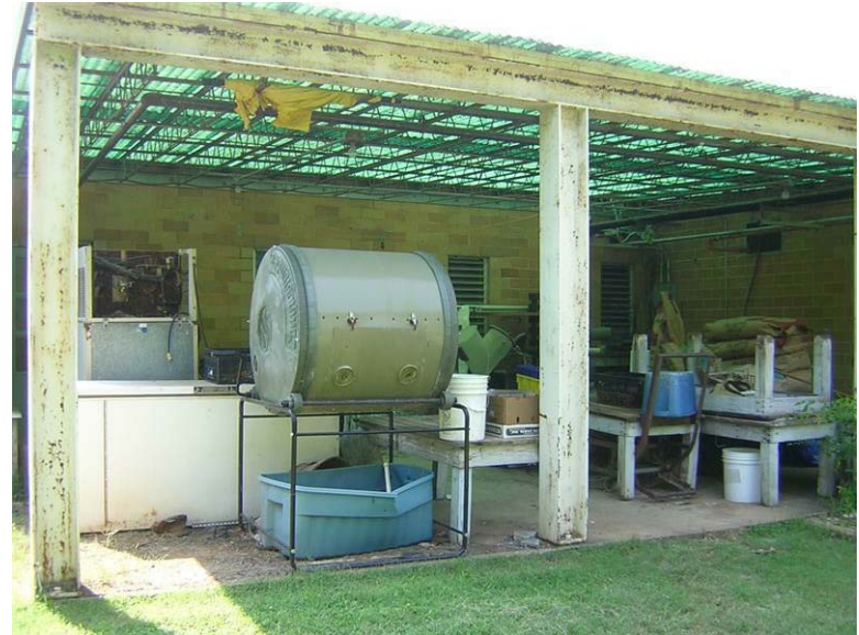
Building 118 – Greenhouse A: Rusting is visible in the steel shed structure at the rear.
