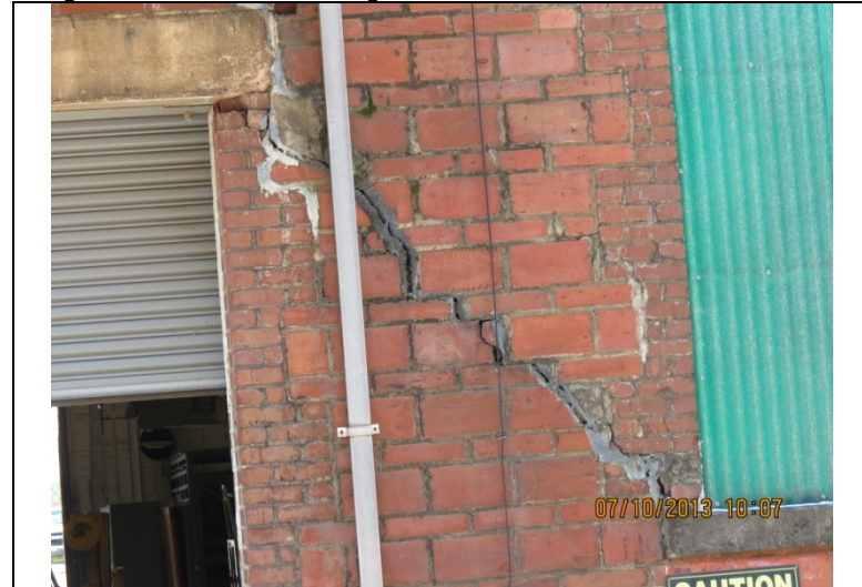
2013 Photo #13: Cracks in masonry at North wall. Additional movement observed.
