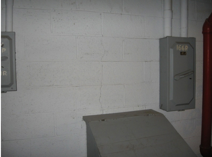
2009 Photo #11: Minor crack in interior concrete masonry wall
