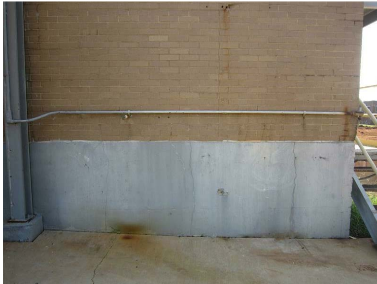
Building 01A - Chemical Feed House: Horizontal cracking is visible in the concrete at the lower wall.
