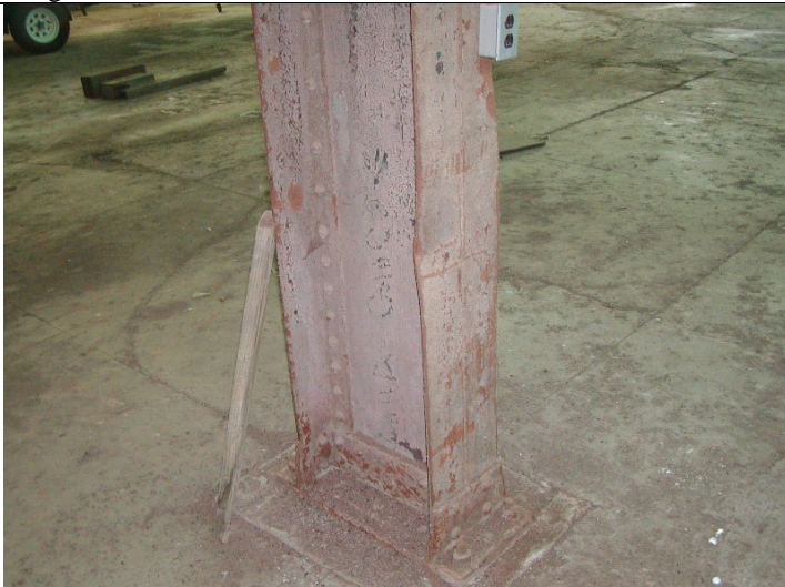
2009 Photo #10: Moderately corroded steel column with impact damage
