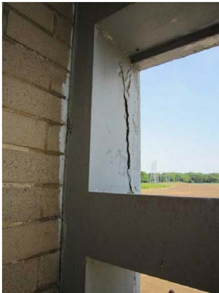
Building 01A - Chemical Feed House: A large vertical crack is visible in the concrete screen at the north entry.
