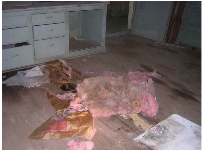
Building 72 – Catalyzer Building No. 4: Water infiltration has caused a hole in the wood flooring.
