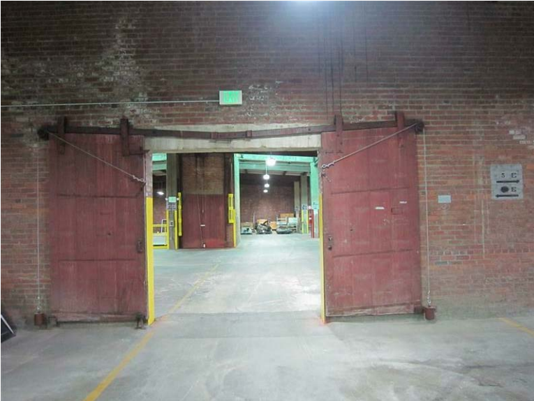
Building 36 – Chemical Plant Warehouse: The historic sliding doors remain intact.
