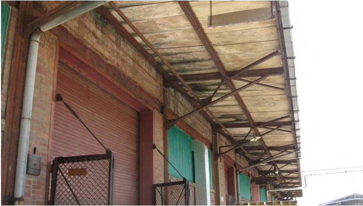
2009 Photo #17: Deteriorated concrete roof planks at South canopy.
