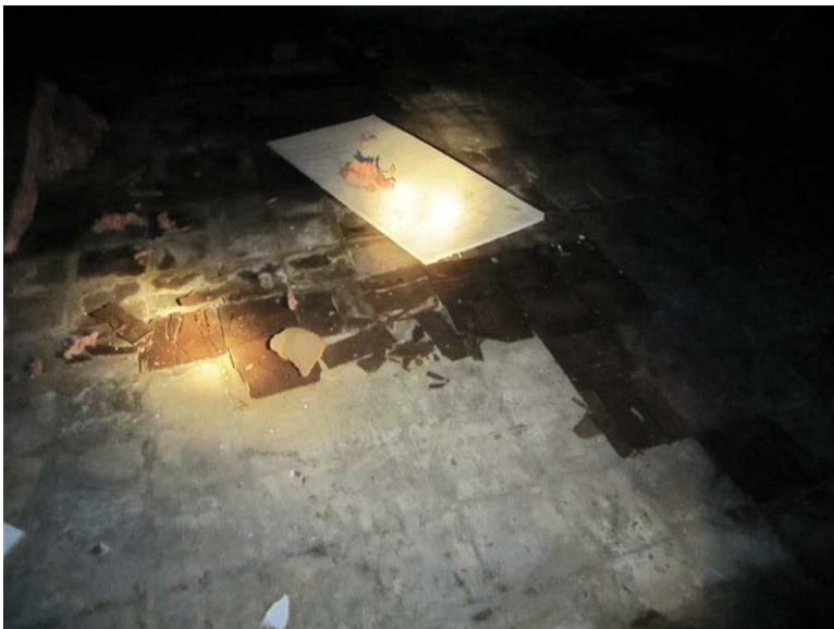
Building 26 – L / N Building Grounds Maintenance Shop: Several possible asbestos containing floor tiles are missing and deteriorated.
