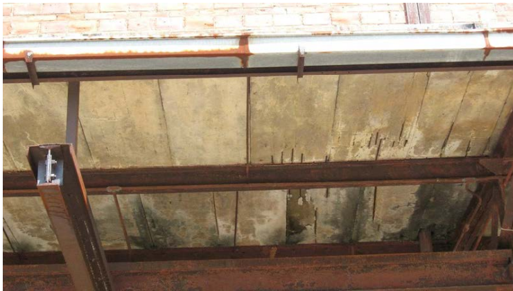
2009 Photo #16: Ruined concrete roof planks at South canopy.
