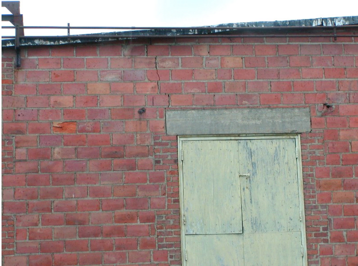
2009 Photo #3: Cracked and spalled masonry at substation
