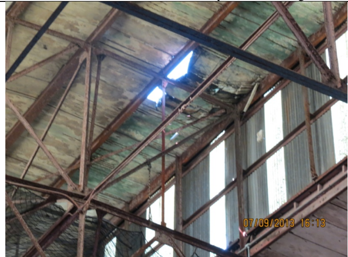
2013 Photo #6: Areas of ruined concrete plank roof deck. Continued deterioration evident.
