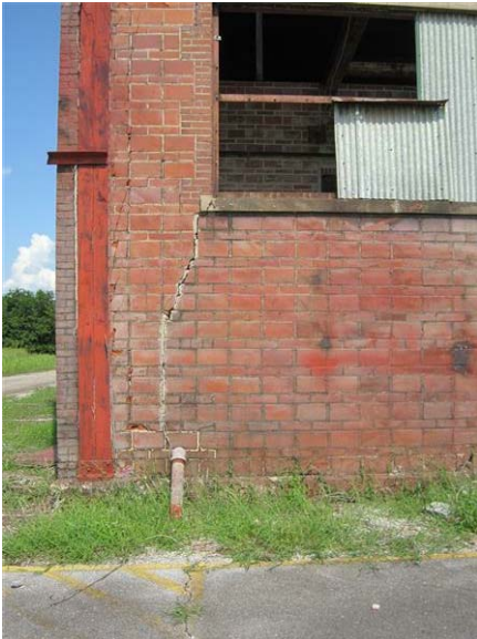
Building 22, 23 – L / N Building: Localized cracking is visible at this window sill.
