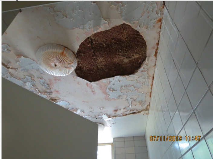
2013 Photo #13: Women's bathroom ceiling. Plaster spalling and rusting steel lath from water infiltration observed.
