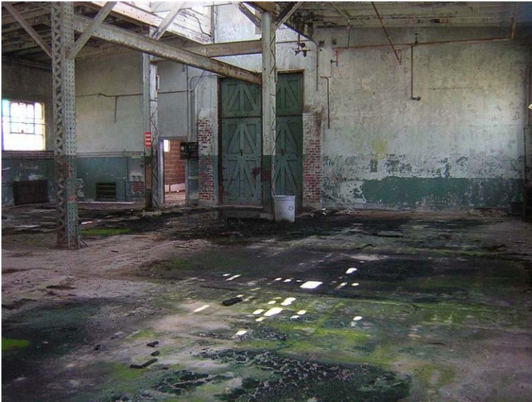
Building 53 – Tin Shop: Standing water has collected on the concrete floor in the primary space.
