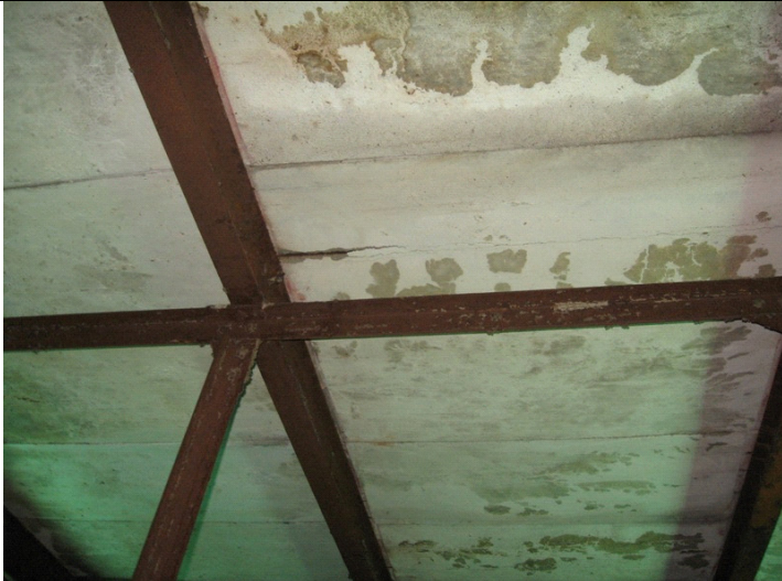
2009 Photo #9: Deteriorated concrete roof planks
