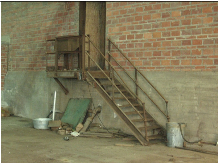
2009 Photo #22: Deteriorated steel stair going up to Building 24
