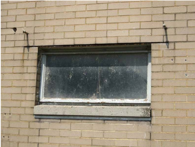
Building 01A - Chemical Feed House: Localized rusting of the steel lintels and metal windows are present.
