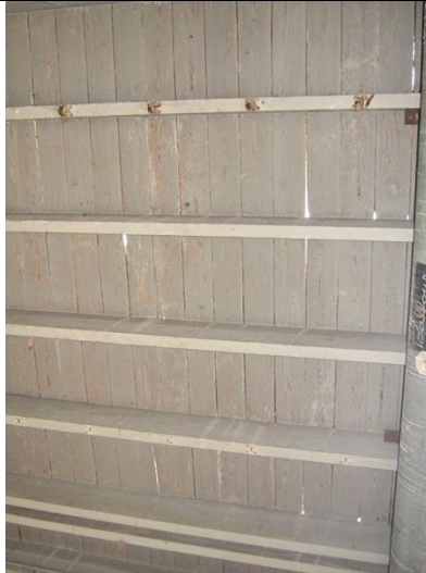
2009 Photo #7: Existing wood plank roof deck with no roof covering (Bright spots are daylight visible through roof deck)
