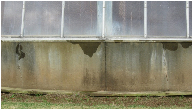
2009 Photo #14: Cracks in foundation wall at greenhouse 1
