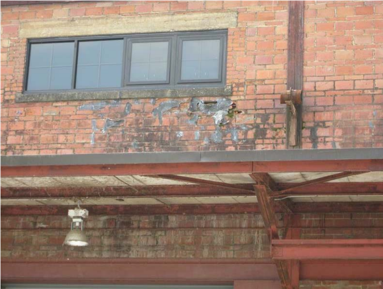
Building 33, 34, 35, 36 – Chemical Plant Warehouse: Most historic windows have recently been replaced with aluminum units
