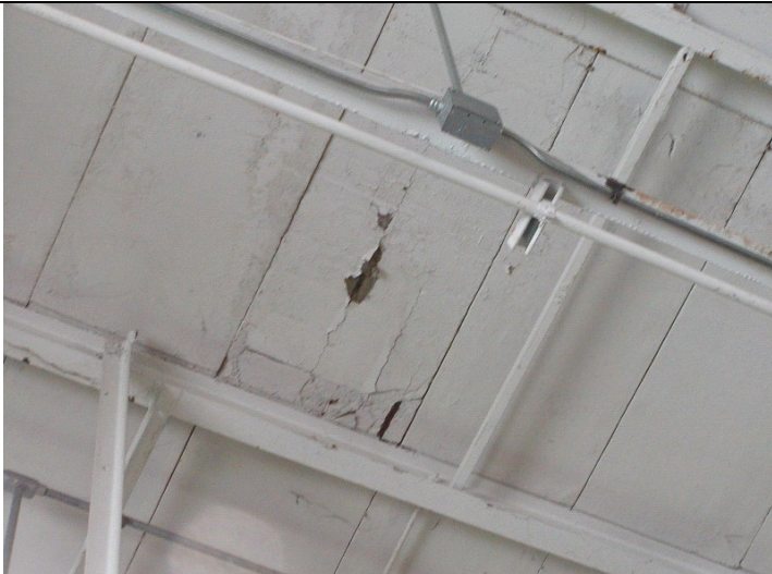
2009 Photo #12: Structurally defective concrete roof deck panel
