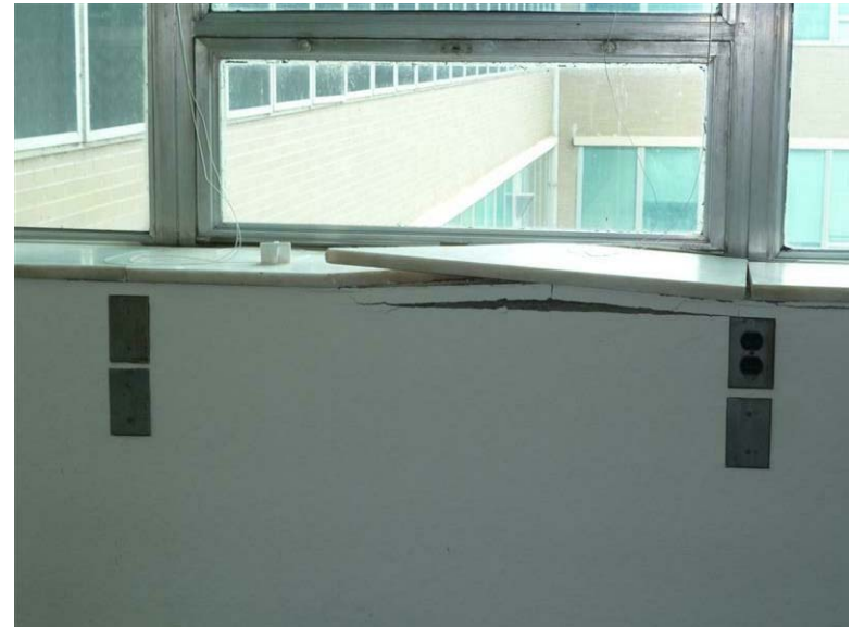
Building 17A - Environmental Research Center: Heaving of the sills in the wings on the east facade.
