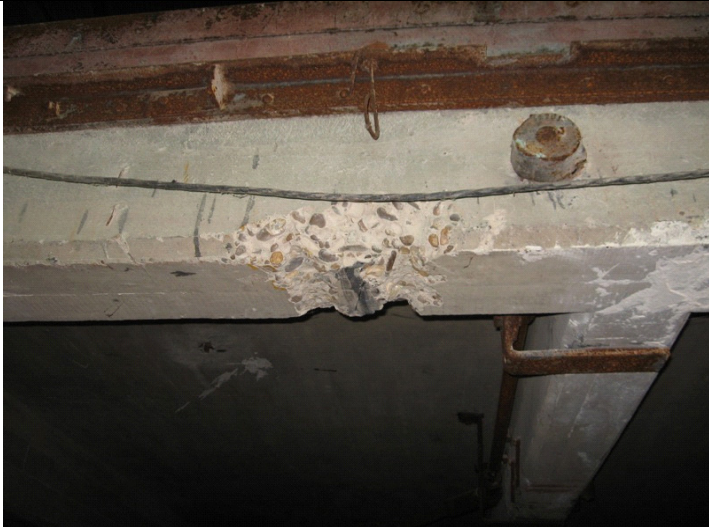
2009 Photo #25: Damaged mezzanine concrete beam
