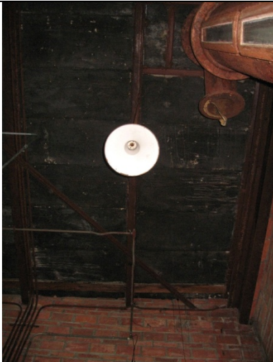
2009 Photo #14: Heavily deteriorated roof deck at West end
