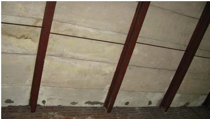
2009 Photo #42: Spalls and surface deterioration at concrete roof planks at interior wall.
