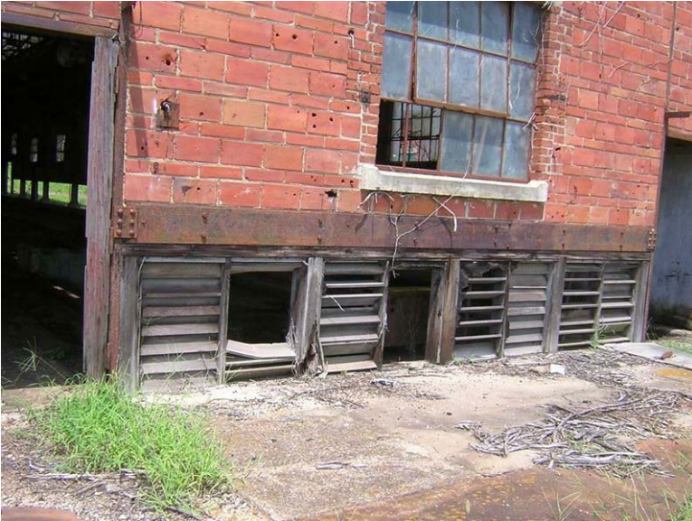
Building 73 – Catalyzer Building No. 5: Several of the wood louvers are broken.
