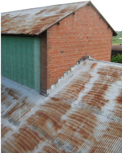
2009 Photo #7: Deteriorated metal roof at South end
