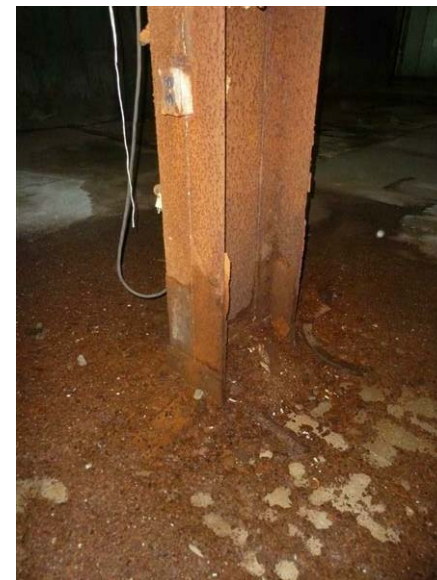
Building 22, 23 – L / N Building: Severe rusting and deterioration are present at this column.
