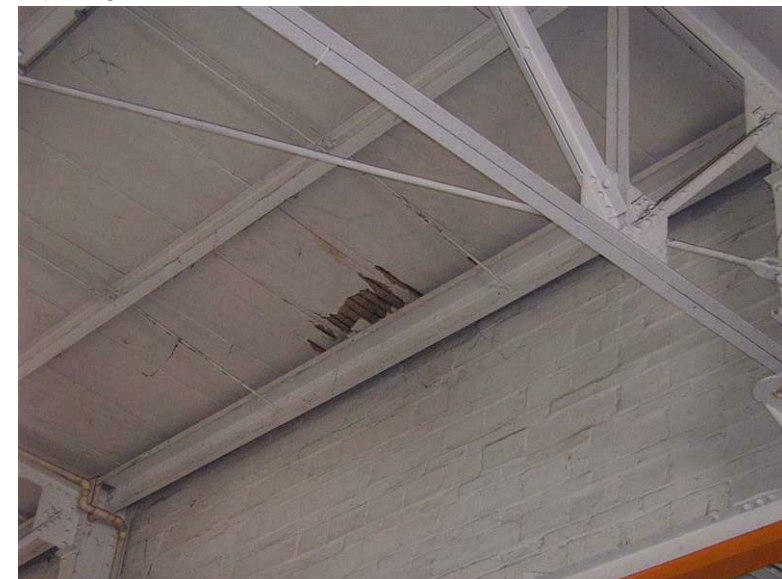
Building 41 – Sheet Metal Shop: The concrete ceiling panel has spalled, exposing the rebar.
