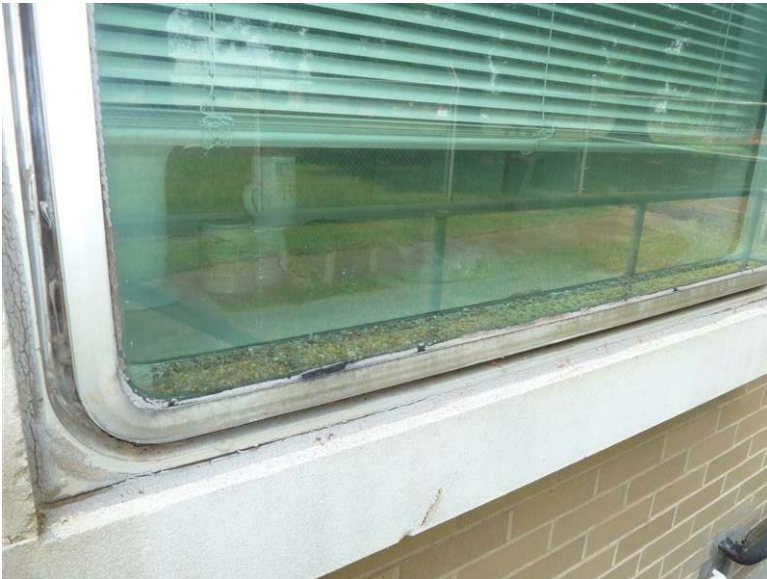
Building 17A - Environmental Research Center: Ladybugs have entered the window cavity indicating the joint/sealant is broken.
