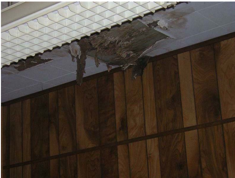
Building 74 – Catalyzer Building No. 6: Water infiltration has damaged the ceiling tiles.
