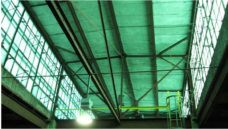
2009 Photo #45: Concrete roof planks at clerestory monitor.
