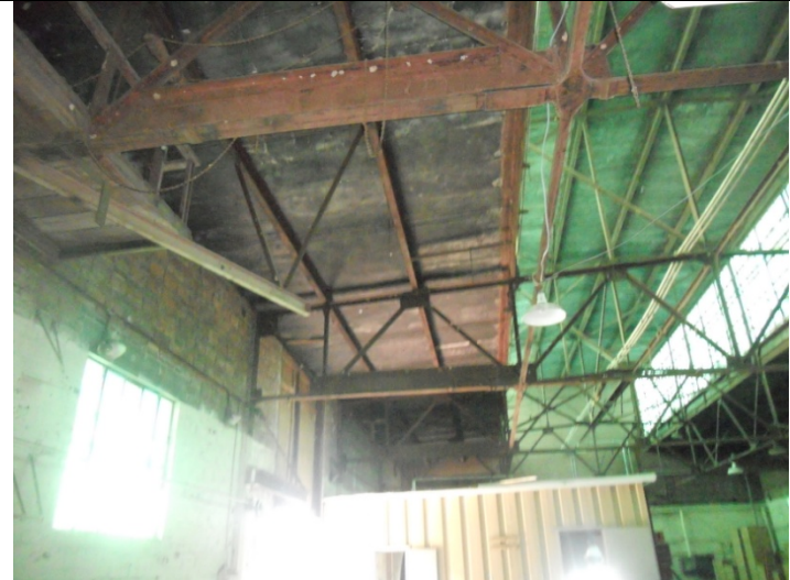
2013 Photo #7: Progressive deterioration of roof framing and deck appears to be evident
