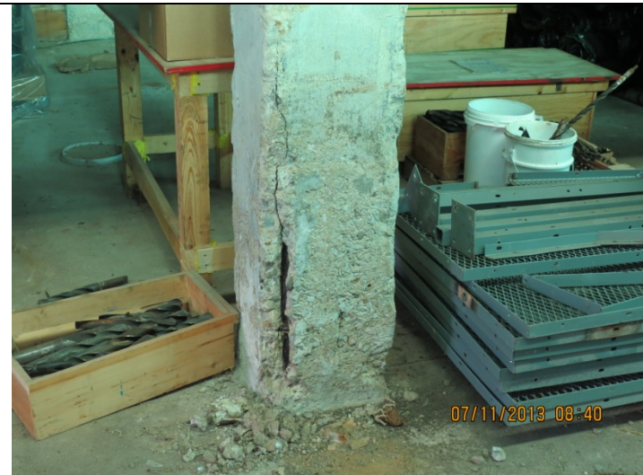
2013 Photo #22: Vertical crack at corner of column is significantly expanded, indicating progressive deterioration of reinforcing steel
