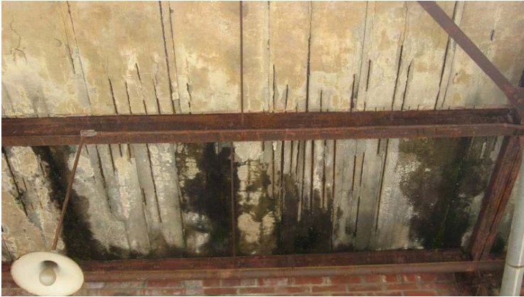
2009 Photo #19: Ruined concrete roof planks at South canopy.
