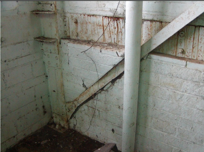
2009 Photo #12: Infill cracking and displacement at Southeast corner
