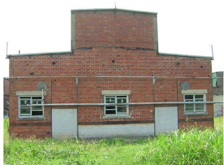
Building 71 – Catalyzer Building No. 3: The original steel windows have been replaced with aluminum windows.
