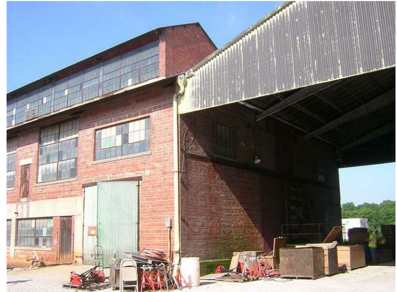
Building 81 – 5A – Nitrate House: Water flows from the attached shed towards the north wall.
