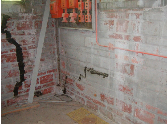
2009 Photo #13: Previously repaired cracks in wall at Northwest corner
