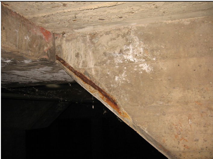
2009 Photo #18: Spalled concrete at basement structure
