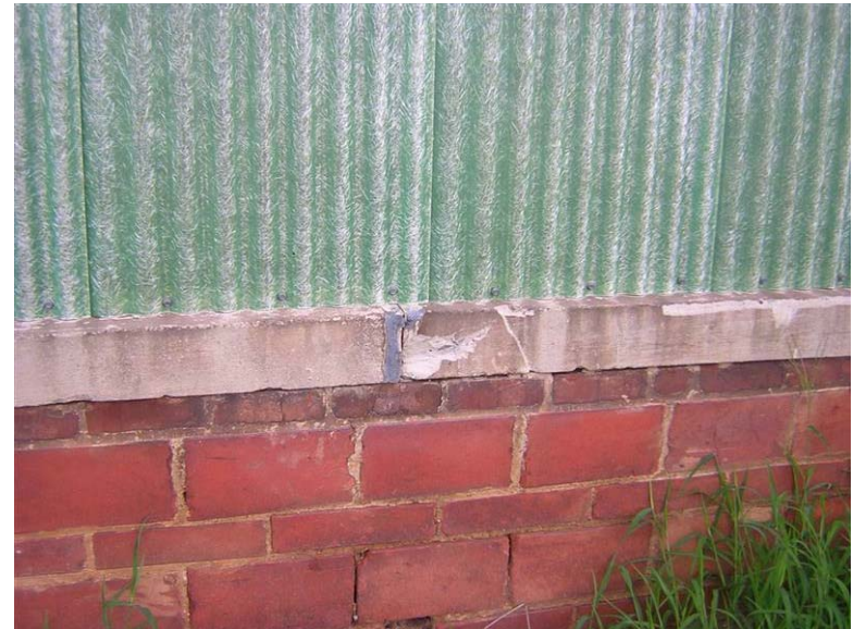
Building 79 – 3A – Nitrate House: Localized cracking and chipping is prevalent in the concrete sills.
