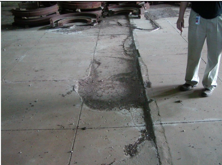
2009 Photo #10: Defective area of elevated slab above basement
