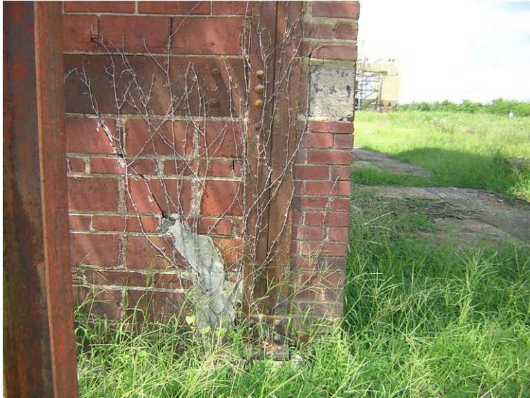
Building 72 – Catalyzer Building No. 4: The crack at the south wall has been partially parged with concrete.
