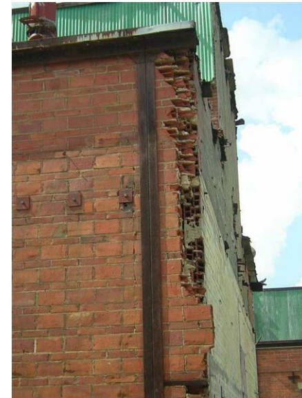
Building 70 – Catalyzer Building No. 2: The hollow clay tile is broken at the corner where the adjacent portion of the building has been demolished.
