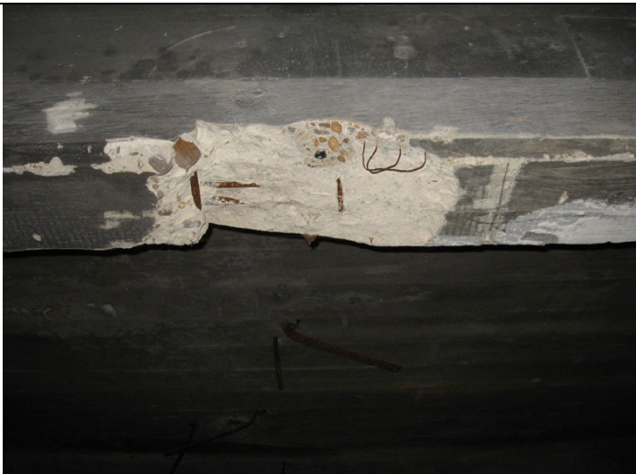
2009 Photo #24: Heavily damaged mezzanine concrete beam
