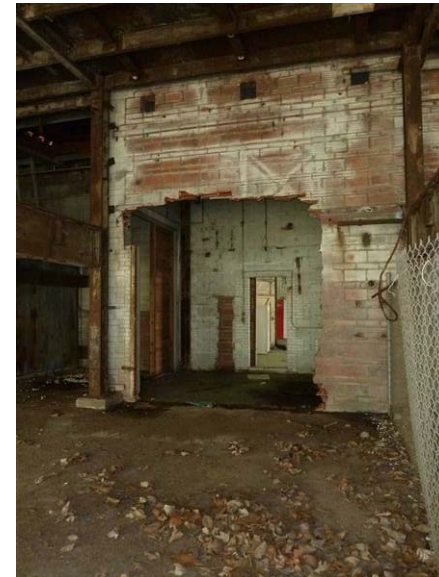
Building 39 – Engineering Lab: The lintel is missing where an opening was made in the hollow clay tile wall adjacent to the south addition.
