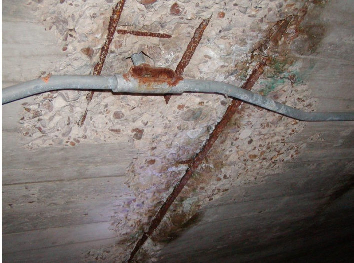
2009 Photo #17: Severely spalled concrete at basement ceiling
