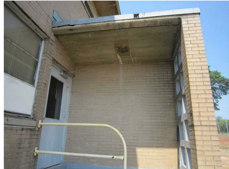
Building 01A - Chemical Feed House: Water has stained the concrete adjacent to the light fixture.
