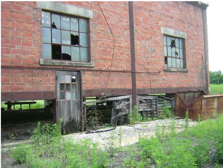
Building 73 – Catalyzer Building No. 5: The wood door is damaged from moisture and the steel windows have several broken panes.
