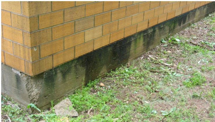
2009 Photo #6: Spalled foundation wall and exterior evidence of interior water intrusion
