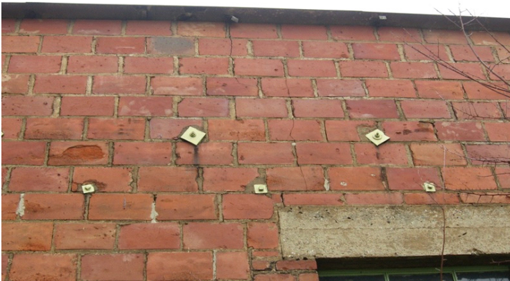
2009 Photo #4: Vertical cracks in masonry – West side
