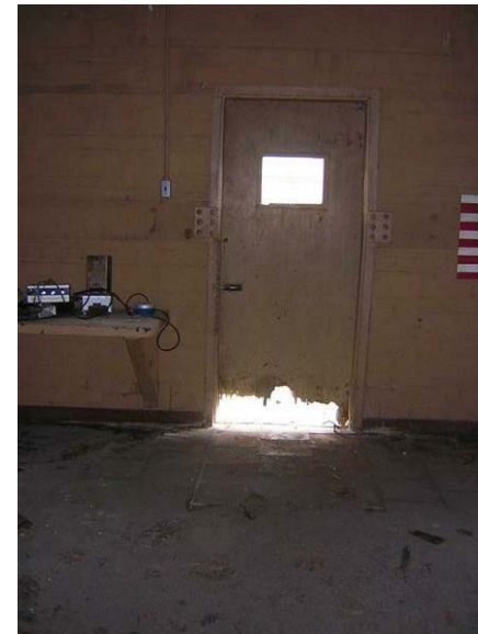
Building 70 – Catalyzer Building No. 2: This door leading to the exterior has worsened in condition.
