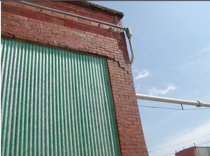
2009 Photo #4: Crack and partially dislodged masonry at Southeast corner
