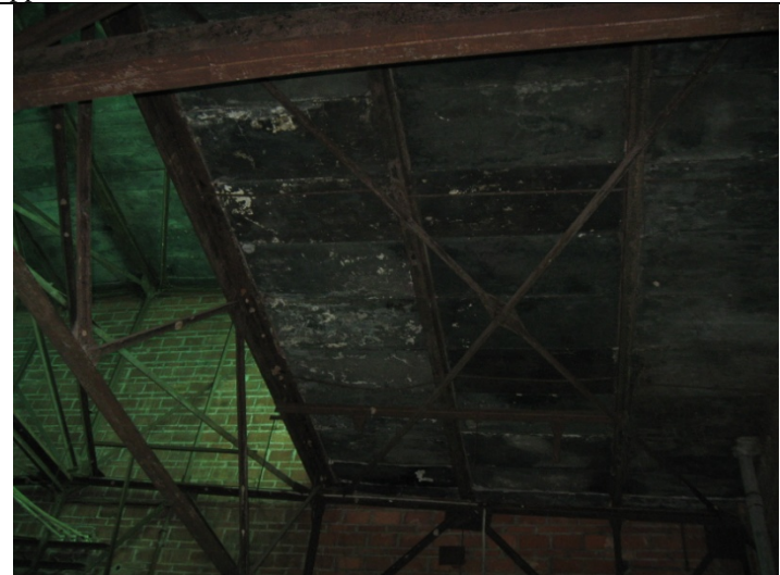
2013 Photo #8: Progressive deterioration of roof framing and deck appears to be evident
