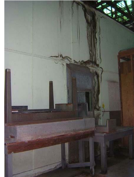
Building 70 – Catalyzer Building No. 2: Water infiltration has stained this interior partition.
