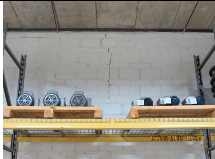
2013 Photo #35: Interior crack in South masonry wall near East end. Daylight seen through crack due to continued settlement.
