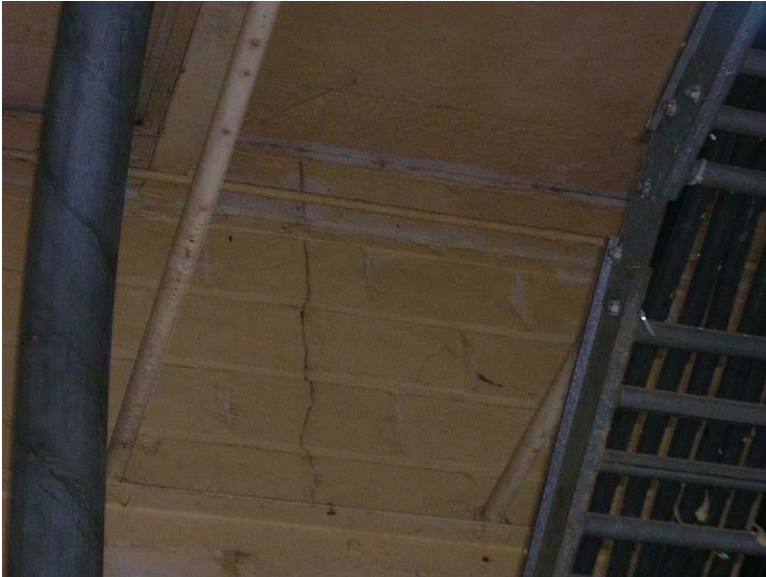
Building 57 – Substation No. 2: Horizontal cracking was visible in the upper wall.
