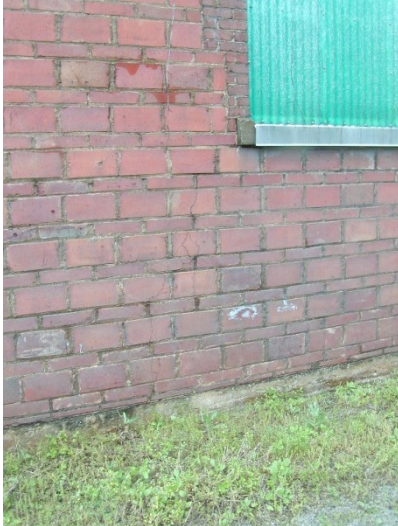
2009 Photo #5: Crack in South exterior wall
