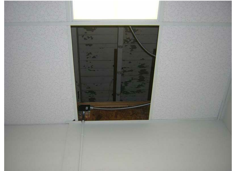
Building 44 – Project Operations Bath House: Wood roof decking and plywood is visible above the acoustical ceiling tiles.
