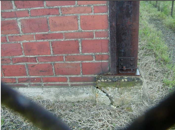
2009 Photo #4: Cracked concrete pier and masonry at Northwest corner
