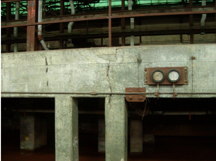
2009 Photo #17: Cracks at edge of elevated slab above basement
