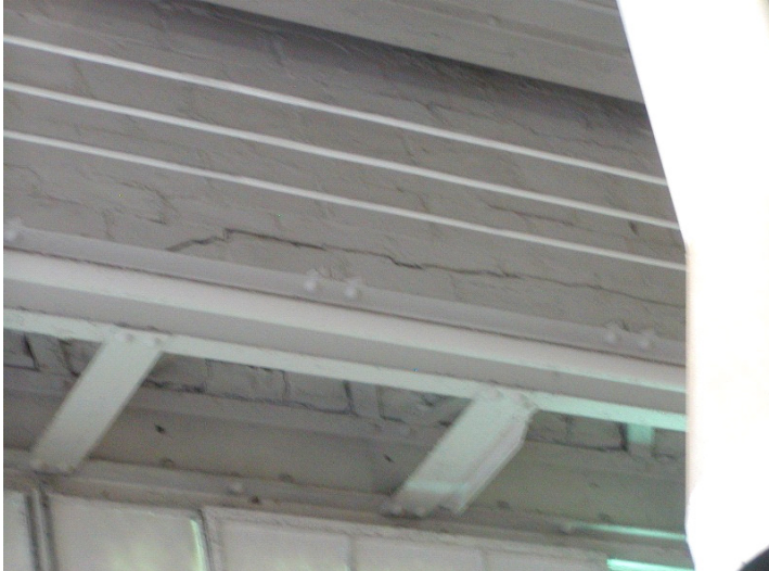
2009 Photo #25: Horizontal crack in masonry at South wall
