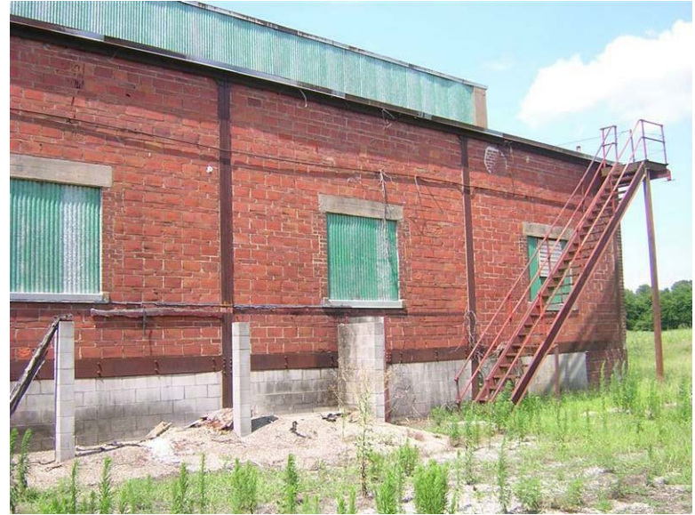
Building 72 – Catalyzer Building No. 4: The exterior metal stair is rusted and in poor condition.
