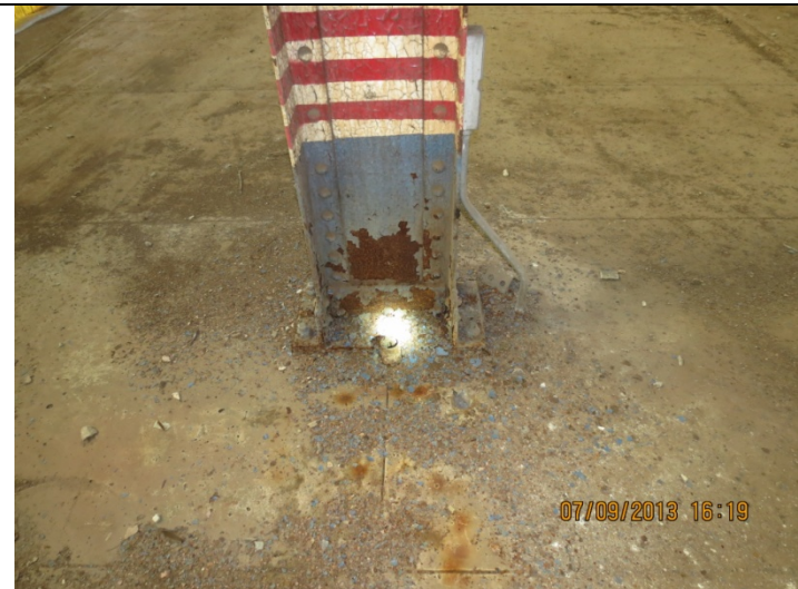
2013 Photo #14: Corroded steel column. Paint flakes have fallen from above as corrosion has worsened. Different location than 2009.
