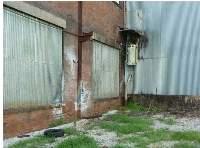
Building 26 – L / N Building Grounds Maintenance Shop: Efflorescence, spalling masonry and eroded mortar joints where water is flowing down the face of the building.
