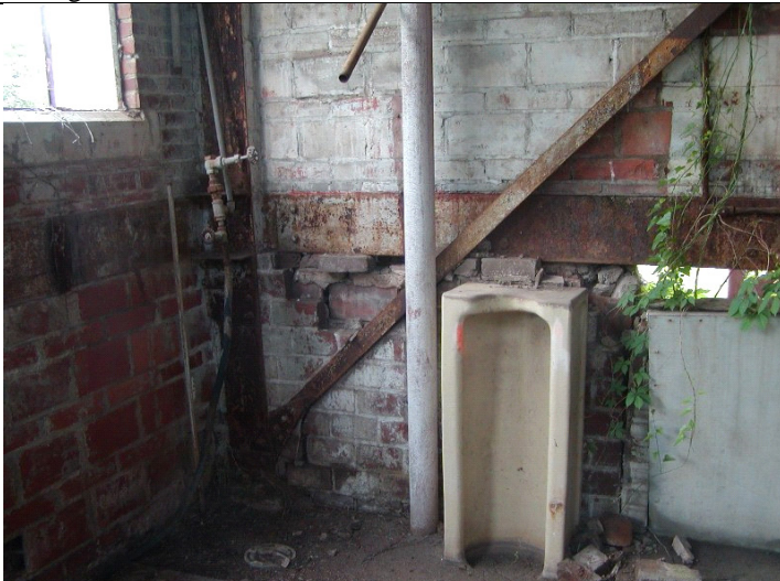
2009 Photo #10: Damaged masonry infill at Southeast corner
