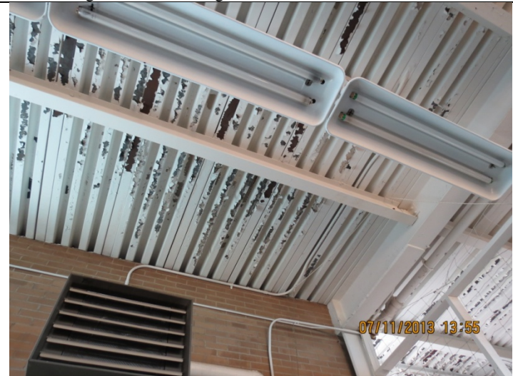
2013 Photo #4: Increased amount of flaking paint and corroded steel decking at vehicle storage area.
