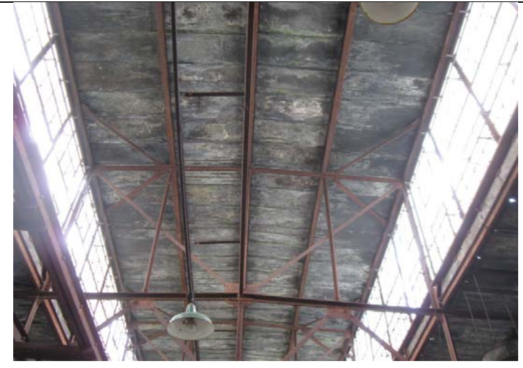
2013 Photo #8: Progressive deterioration of concrete plank roof deck indicates change in condition from (4) "Deteriorated" to (5) "Critical"
