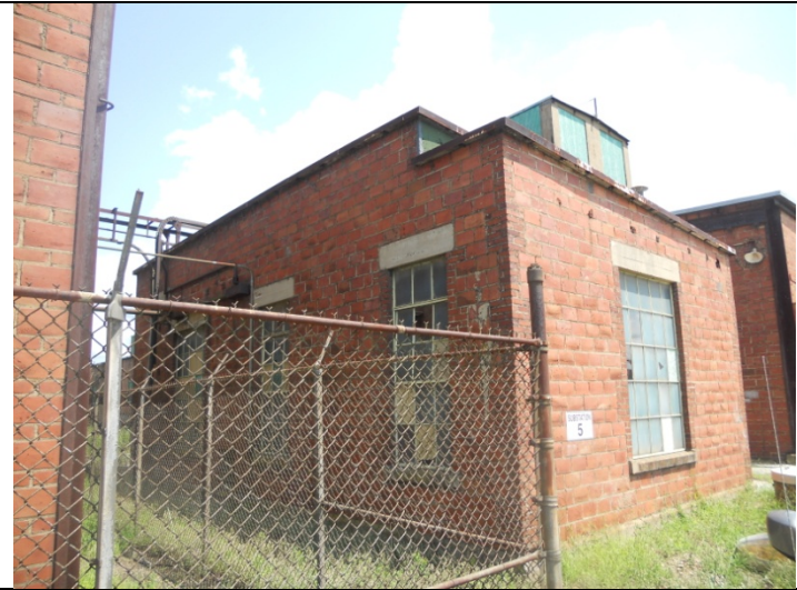
2013 Photo #1: West wall of substation in generally good condition
