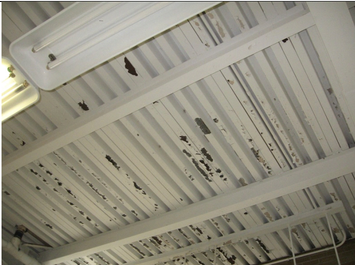
2009 Photo #4: Flaking paint at metal roof deck in vehicle storage area
