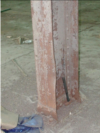
2009 Photo #9: Moderately corroded steel column with impact damage
