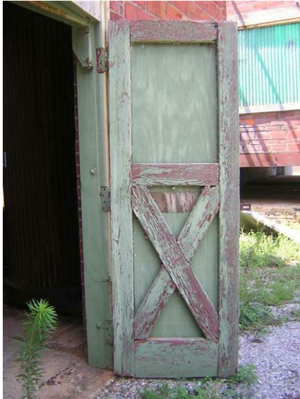
Building 68a – Substation No. 5: Paint is flaking from the wood doors on the east facade.
