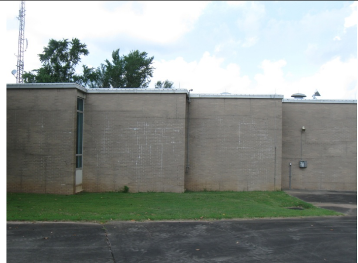
2013 Photo #12: Efflorescence not previously documented at the exterior south masonry wall was observed.
