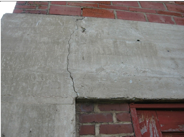
2009 Photo #10: Substantial crack in exterior mezzanine concrete frame
