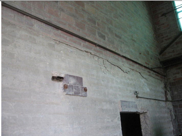
2009 Photo #18: Cracked and spalled concrete at interior wall
