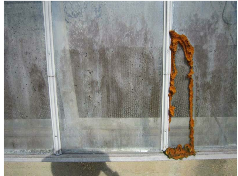
Building 118 – Greenhouse B-D: The broken pane has been sealed with an orange substance.
