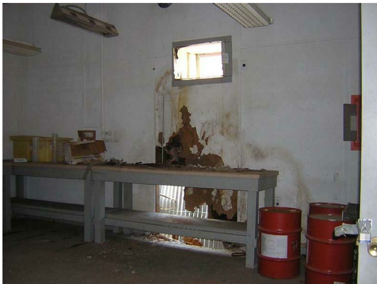
Building 71 – Catalyzer Building No. 3: Water infiltration has severely damaged the wood stud wall.
