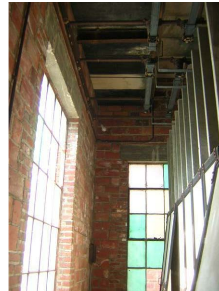
Building 68 – Substation No. 4: A row of concrete panels along the west wall are blackened from moisture
