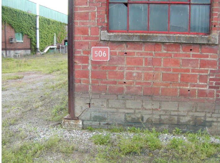
2009 Photo #13: Settlement cracks in masonry at Northwest corner
