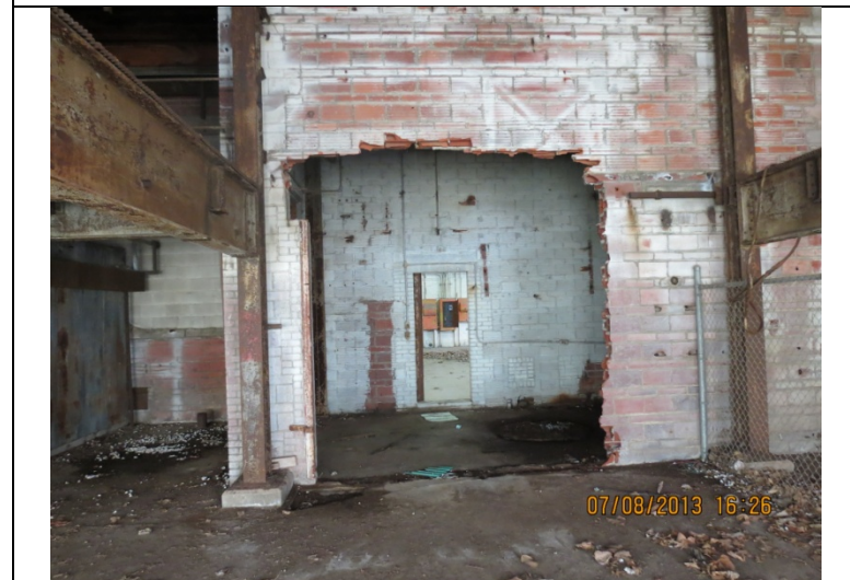
2013 Photo #24: Hole in masonry wall of main section of Building 39. Steel framing has been cut as well.
