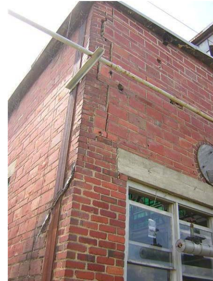
Building 71 – Catalyzer Building No. 3: The quoins are cracked at the rear corners.
