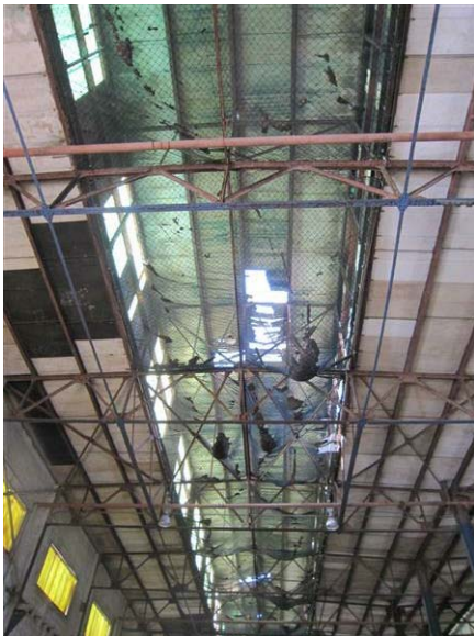
Building 22, 23 – L / N Building: Ceiling panels have deteriorated since the previous assessment.
