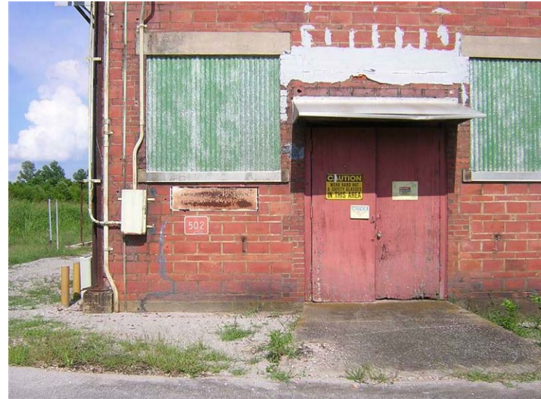
Building 69 – Catalyzer Building No. 1: The historic awning has been replaced and the flush wood doors are damaged.
