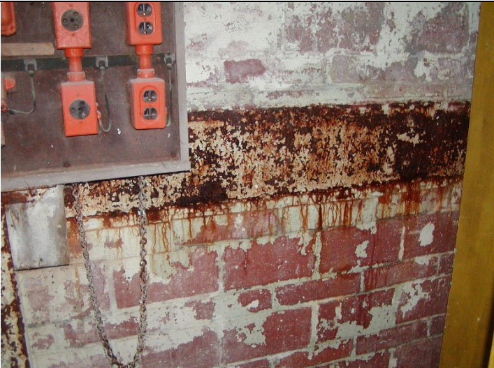
2009 Photo #12: Heavily corroded steel framing at North wall
