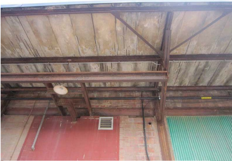
Building 33, 34, 35, 36 – Chemical Plant Warehouse: Concrete panels are spalling exposing the rebar at the north canopy.
