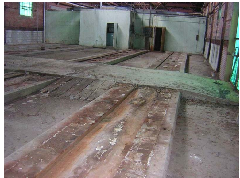
Building 74 – Catalyzer Building No. 6: The bricks in the raised floor have visible efflorescence.
