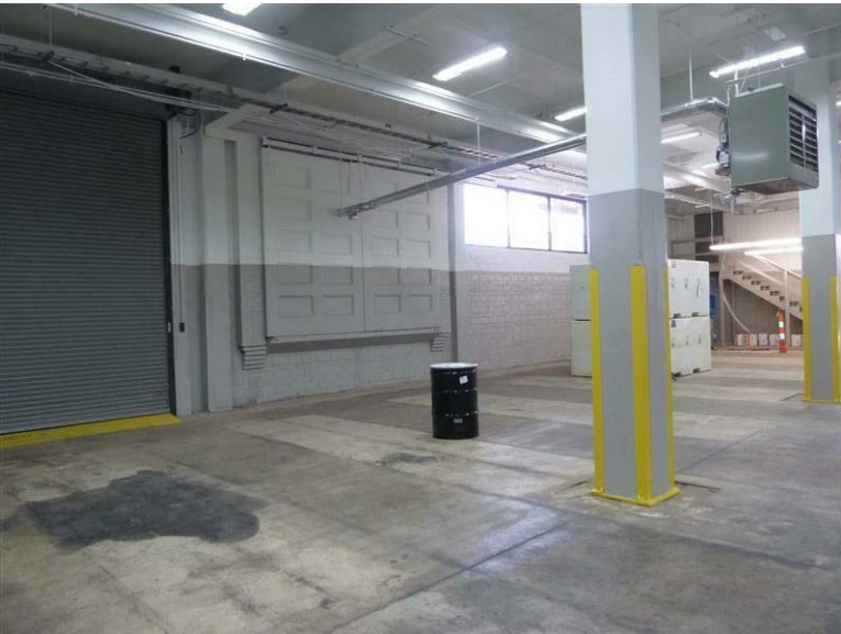
Building 35 – Chemical Plant Warehouse: Recent modifications have been made to this space. A pipe penetrates the historic door.
