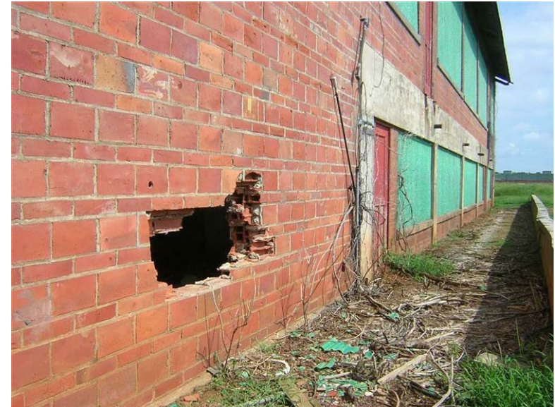
Building 79 – 3A – Nitrate House: There is a hole in the hollow clay tile on the east wall.
