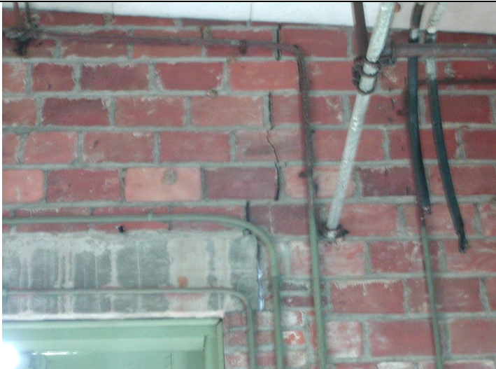
2009 Photo #4: Cracked masonry at substation lintel
