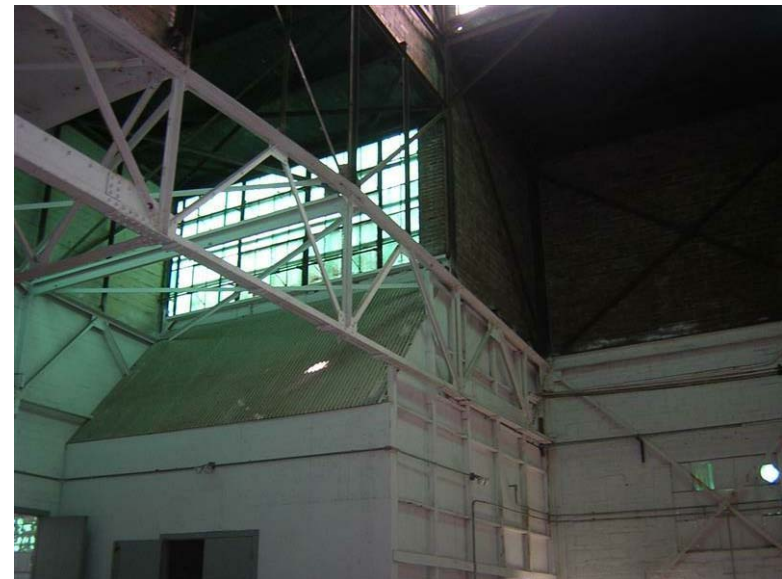
Building 71 – Catalyzer Building No. 3: Metal decking has been placed over this interior infill.
