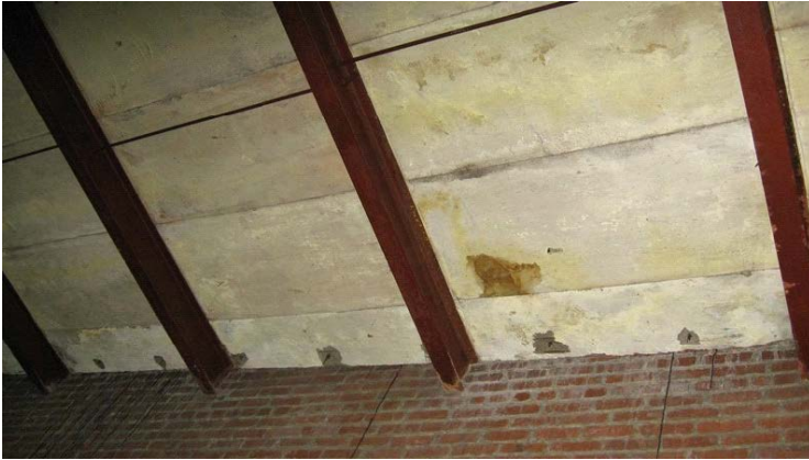
2009 Photo #43: Spalls and surface deterioration at concrete roof planks at interior walls.
