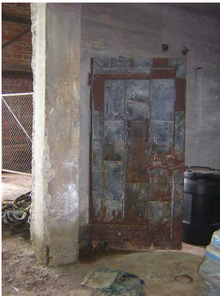
Building 79 – 3A – Nitrate House: The metal door is rusted.
