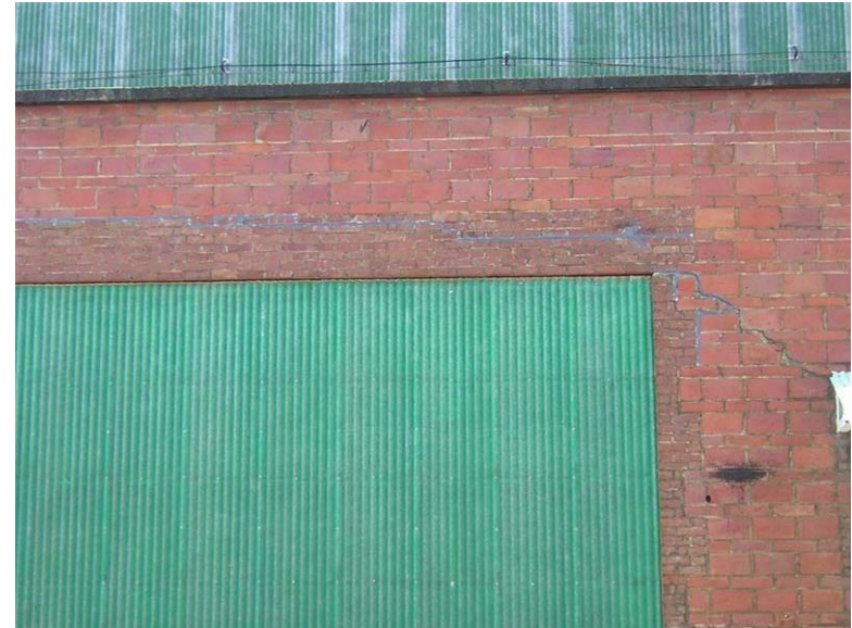
Building 42 – Pipe Shop: This horizontal crack continues across much of the south facade.
