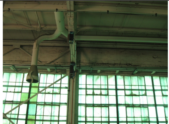
2013 Photo #7: Minor progressive deterioration of masonry above windows was observed
