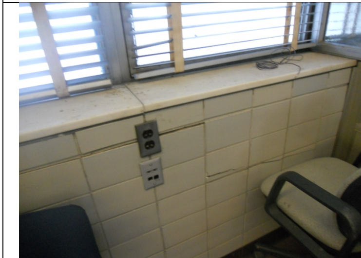
2013 Photo #19: Unoccupied: Stair step cracking in wall finish below marble window sill.
