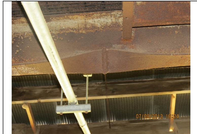
2013 Photo #22: Damaged steel beam due to impact or other unforeseen use of member.
