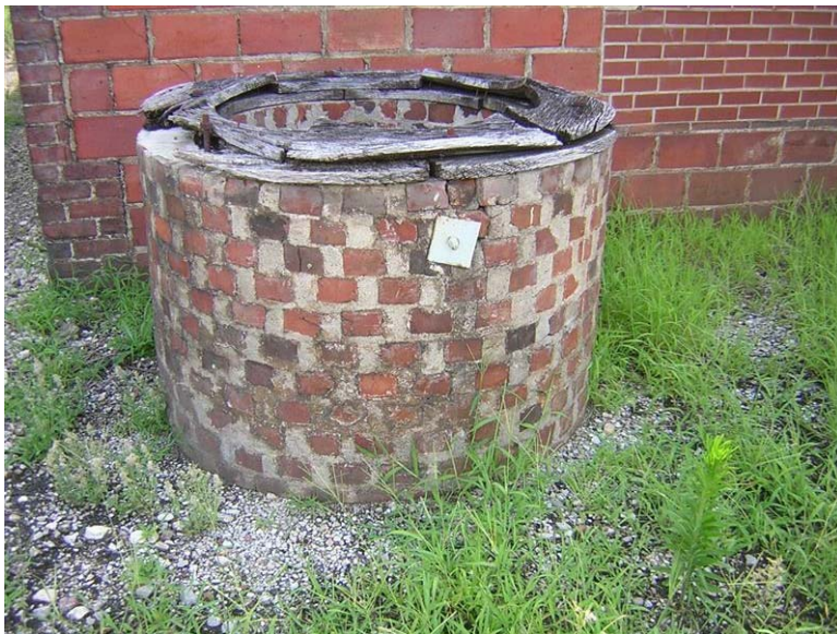
Building 74 – Catalyzer Building No. 6: The wood on top of the brick well / structure is warped and damaged.
