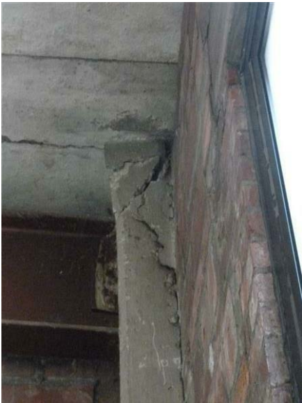
Building 33 – Chemical Plant Warehouse - Shipping and Receiving Office: The concrete columns are severely damaged.
