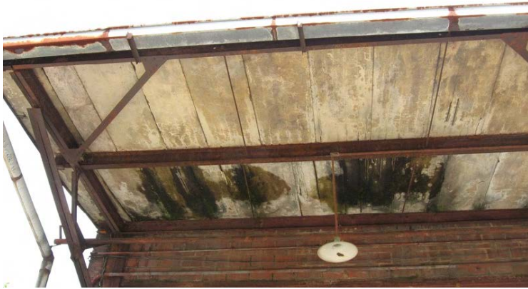
2009 Photo #15: Deteriorated concrete roof planks at West end of South canopy.
