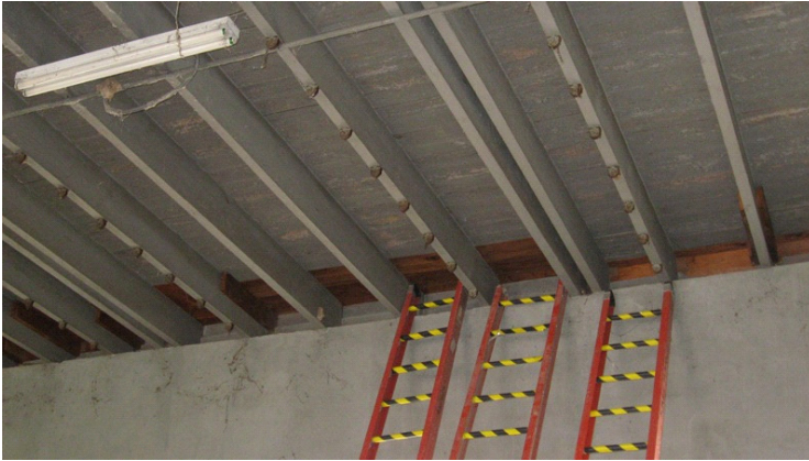
2009 Photo #9: Partially replaced wood roof deck
