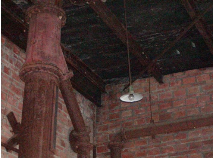
2009 Photo #9: Severely deteriorated roof structure at West end of building
