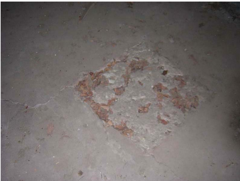
Building 72 – Catalyzer Building No. 4: The concrete floor is cracked and damaged in several areas.
