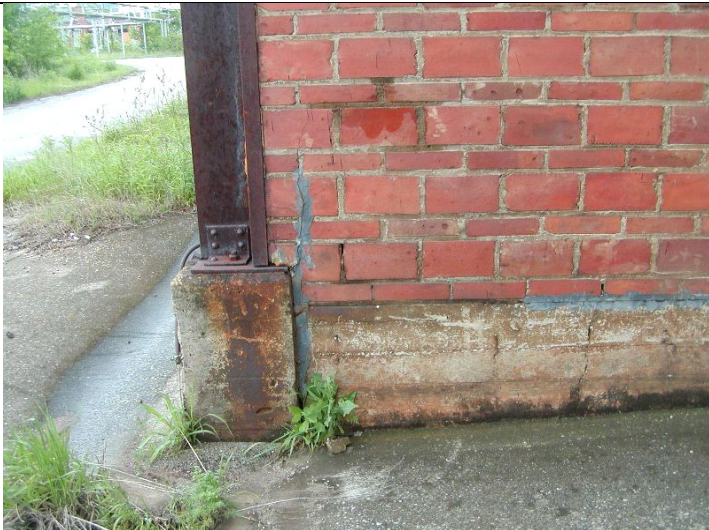
2009 Photo #14: Cracks in masonry and foundation wall at Southwest corner
