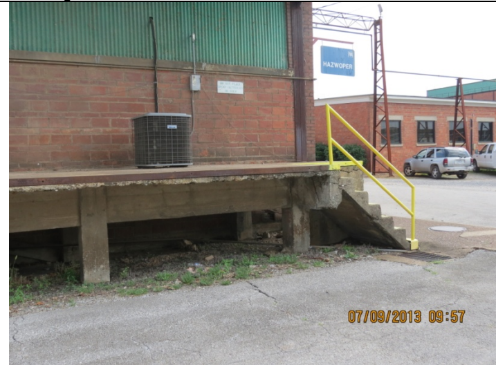
2013 Photo #23: Deteriorated concrete steps and support at East and South loading dock. Elevated slab deterioration evident.
