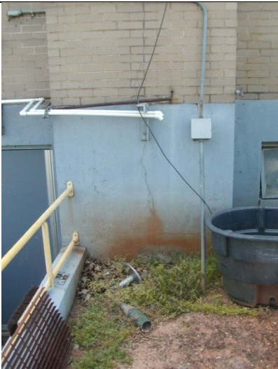
2009 Photo #4: Cracks in masonry and foundation wall on East side
