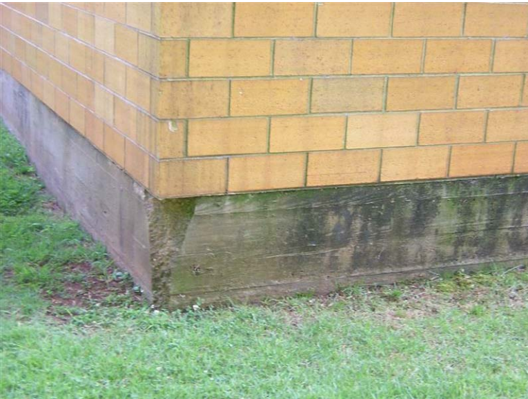
Building 118 – Greenhouse A: Localized damage is visible at the corner of the concrete foundation.
