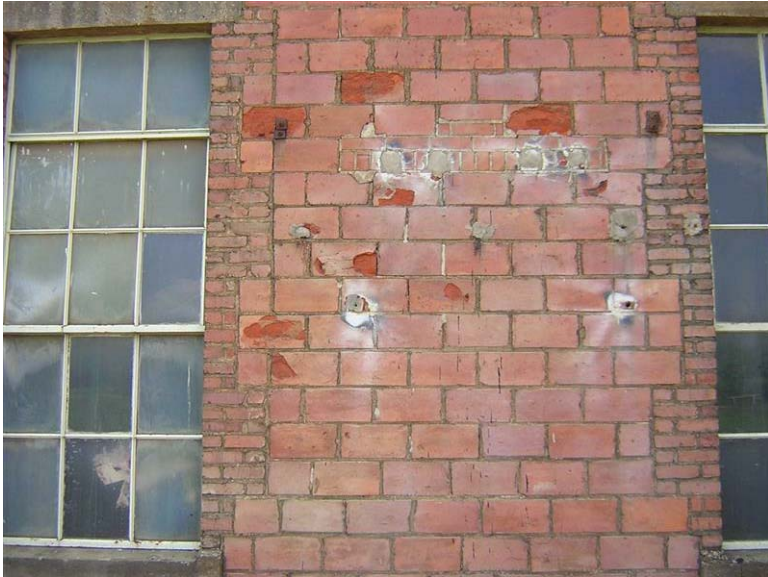
Building 57 – Substation No. 2: Some of the holes in the hollow clay tile have been parged with concrete.
