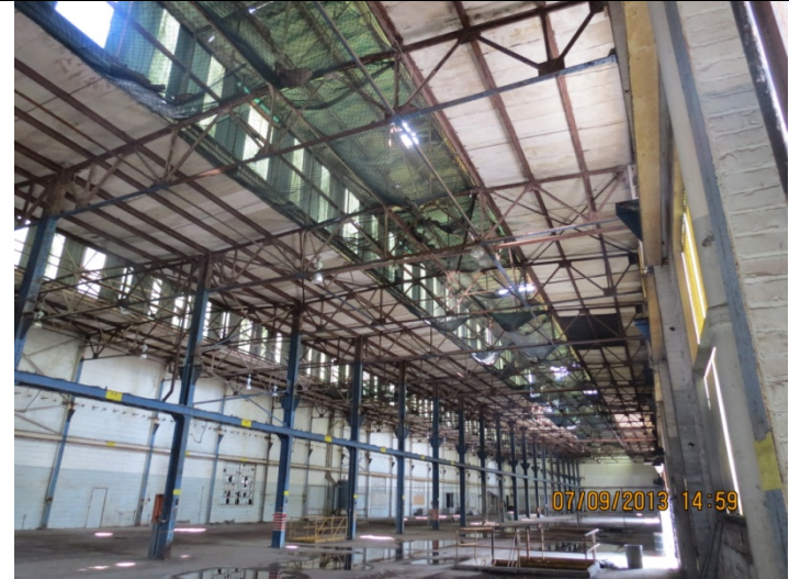
2013 Photo #3: Interior building looking South. Continued concrete roof plank deterioration evident.
