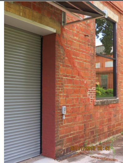
2013 Photo #4: Repairs to cracks in masonry South end of West wall observed.
