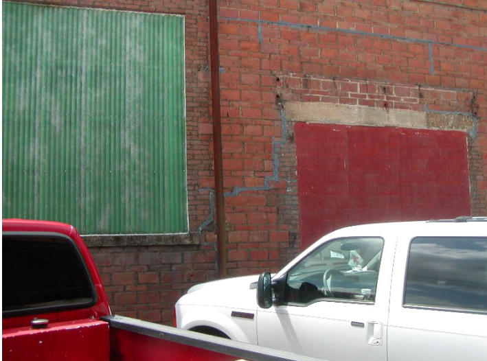
2009 Photo #11: Cracks in masonry at North wall
