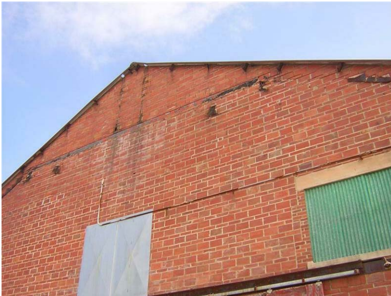
Building 79 – 3A – Nitrate House: There is a large horizontal crack across the gable end.
