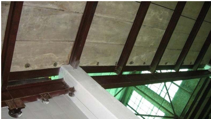
2009 Photo #40: Spalls at concrete roof planks adjacent to clerestory monitor.
