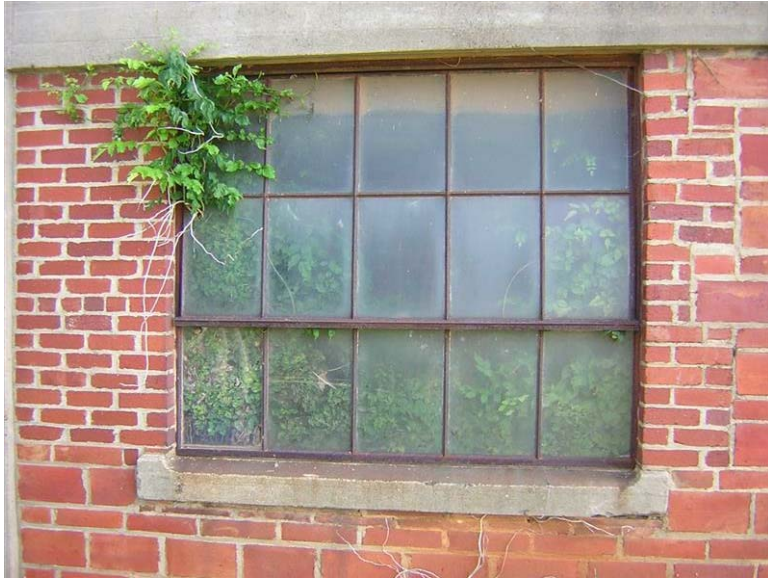
Building 81 – 5A – Nitrate House: Localized plant growth is located in the building.
