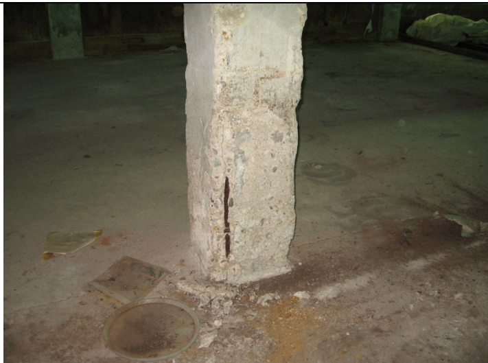
2009 Photo #22: Severely spalled mezzanine concrete column
