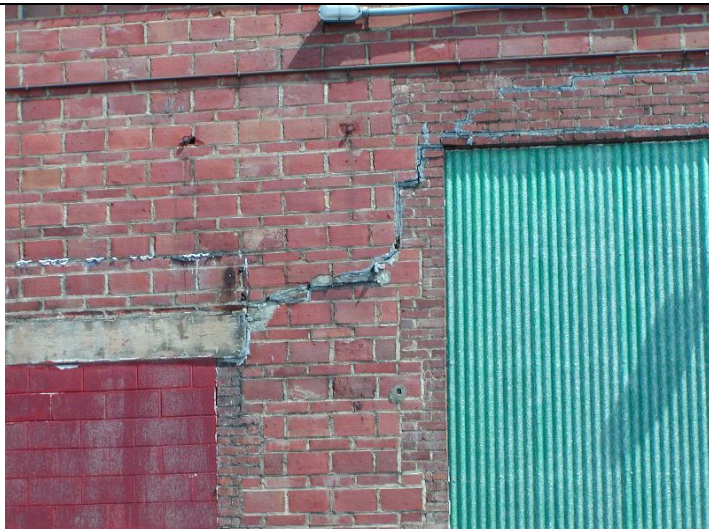
2009 Photo #6: Cracks in masonry on South side
