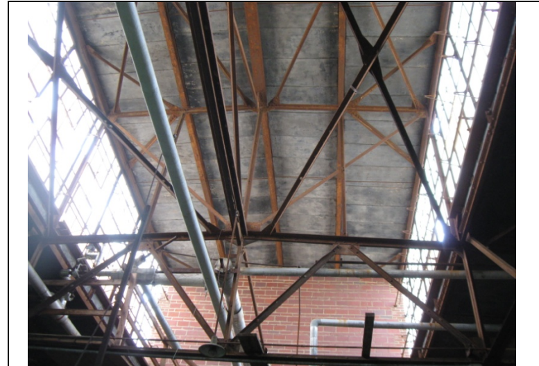
2013 Photo #9: Minor progressive deterioration of steel framing and concrete plank roof deck appears to be evident
