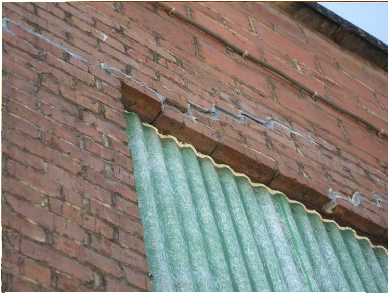
Building 37, 38 – Machine Shop: Several cracks occur in the brick surround, which has begun to shift above the window.
