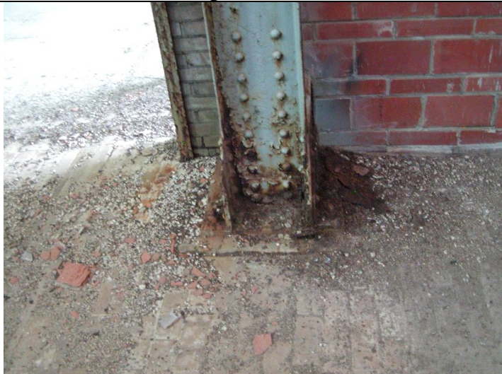
2009 Photo #9: Severe corrosion at column base plate attachment
