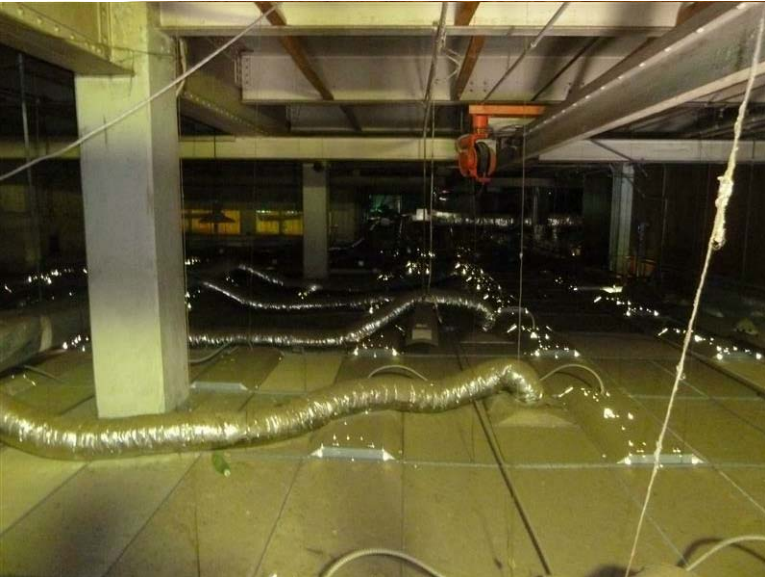
Building 34 – Chemical Plant Warehouse - Instrumentation / Electric Shop: Acoustical ceiling tiles have installed, lowering the ceiling height.
