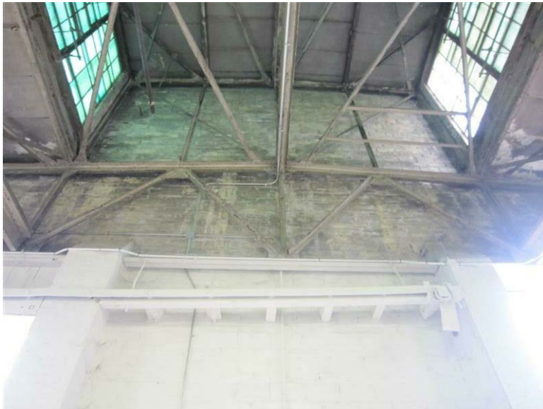
Building 38 – Machine Shop - Gas and Diesel Repair Shop: The hollow clay tile walls leading to the clerestory are stained.
