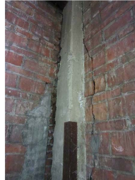
Building 33 – Chemical Plant Warehouse - Shipping and Receiving Office: Severe cracking is visible along exterior corners.
