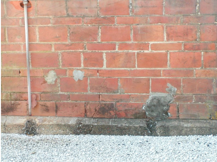
2009 Photo #9: Cracks in masonry and exposed slab edge on North side
