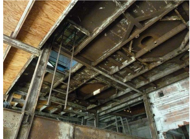
Building 39 – Engineering Lab: Portions of the wood decking have been replaced with plywood.
