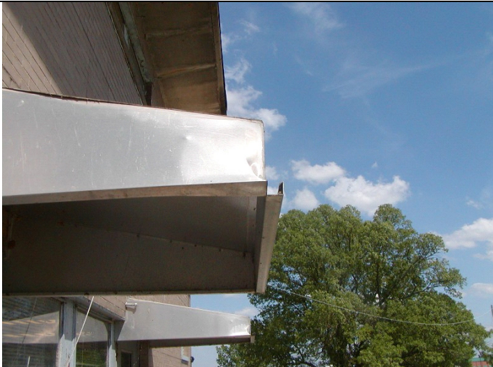
2009 Photo #6: Dented metal awning on South side.
