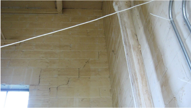
2009 Photo #5: Cracks in masonry – West wall
