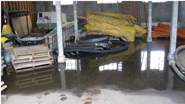
2009 Photo #8: Standing water on floor in one area of uncovered roof deck
