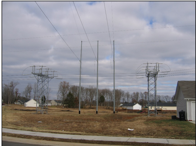
Photo 2-3. Example of switch structures and associated 3-pole transmission structure at a transmission line tap point
