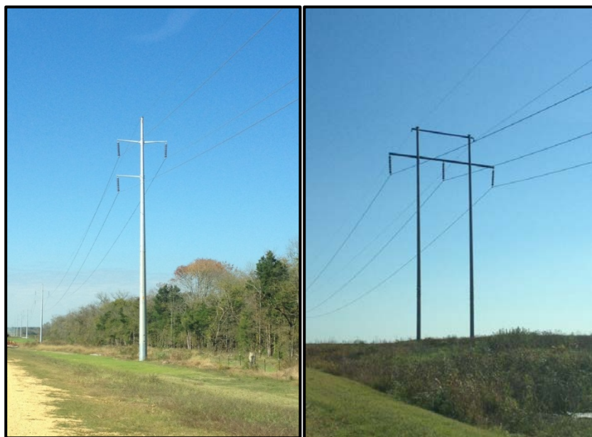
Figure 2-3. Typical Single and Double Steel-Pole Structures
