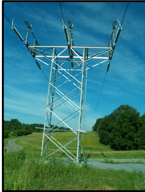
Figure 2-4. Typical Transmission Line Switch Structure
