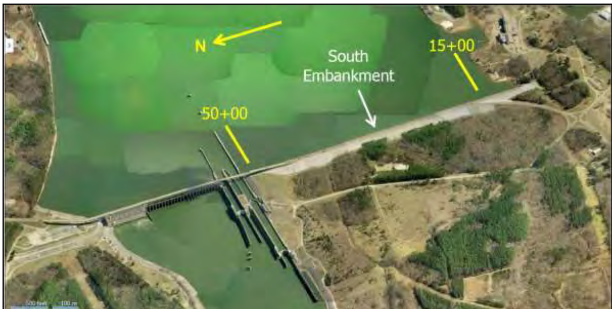
Exhibit 1 Pickwick Landing Dam, South Embankment
