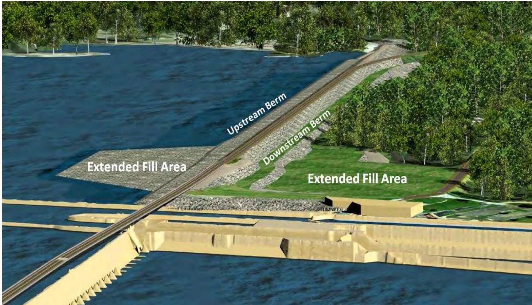
Exhibit 2 Proposed Action Alternative - Berms and Extended Fill Areas (Pickwick Landing Dam South Embankment)
