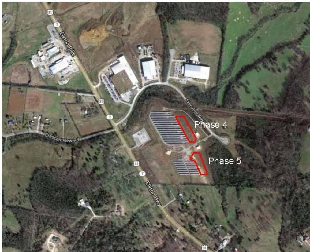
Figure 1. Proposed Phase 4 and Phase 5 expansions of Pulaski Energy Park solar generating facility.
