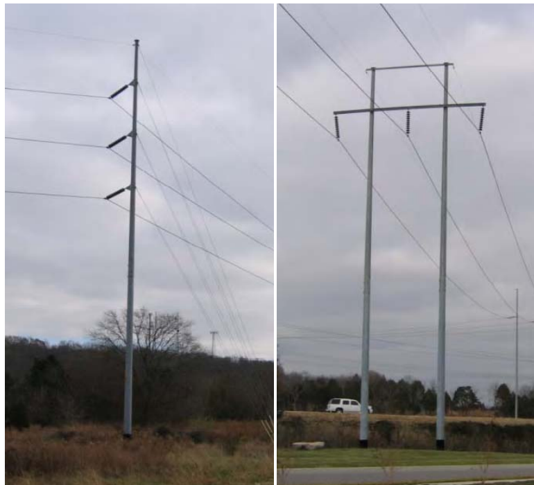
Figure 2-2. Examples of 161-kV Transmission Structures
