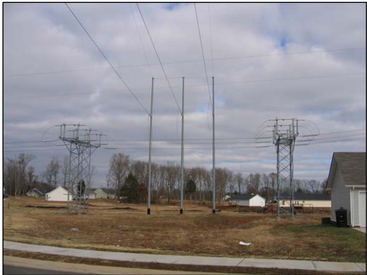
Photo 2.2-3. Example of switch structures and associated 3-pole transmission structure at a transmission line tap point
