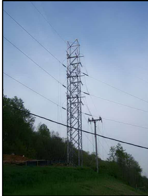
Figure 2-2 Transmission Line Switch Structure
