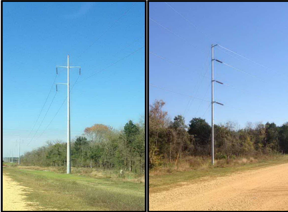
Figure 2-1 Typical Single Steel-Pole Structures
