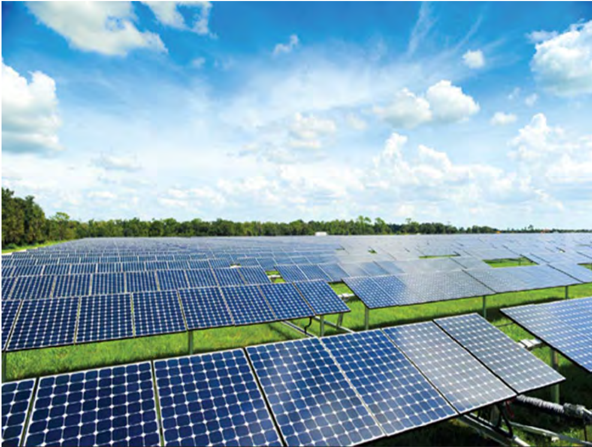
Photo 3.5-7. Single-axis, tracking photovoltaic system with panels close to maximum tilt as viewed from the east or west.
