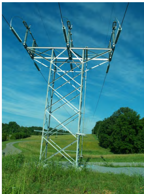
Figure 2-2. Example of a 161-kV Transmission Line Switch Structure
