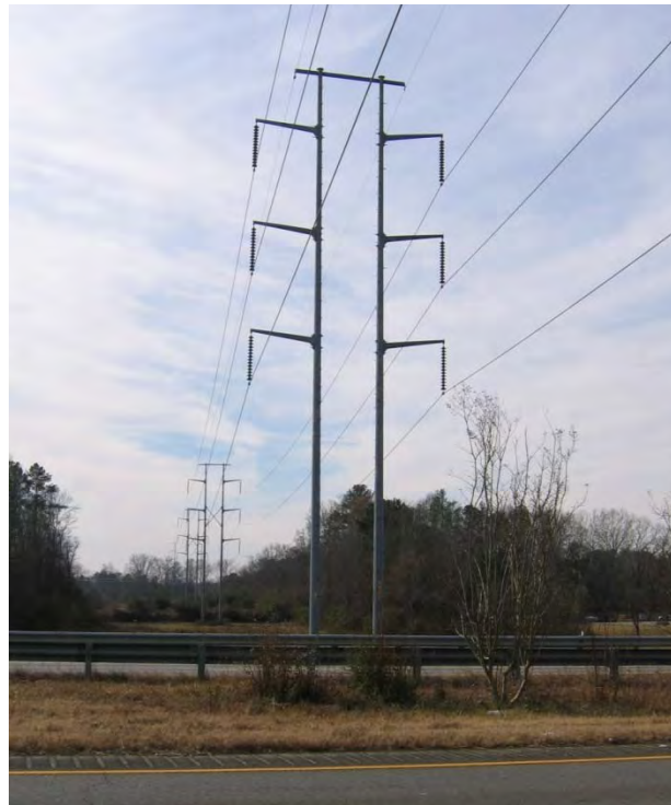
Figure 2-1. Example of Double Steel-Pole 161-kV Transmission Structures
