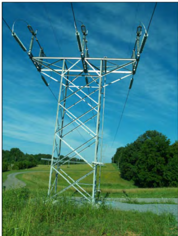
Figure 5. Switch structure similar to those proposed for the current project.
