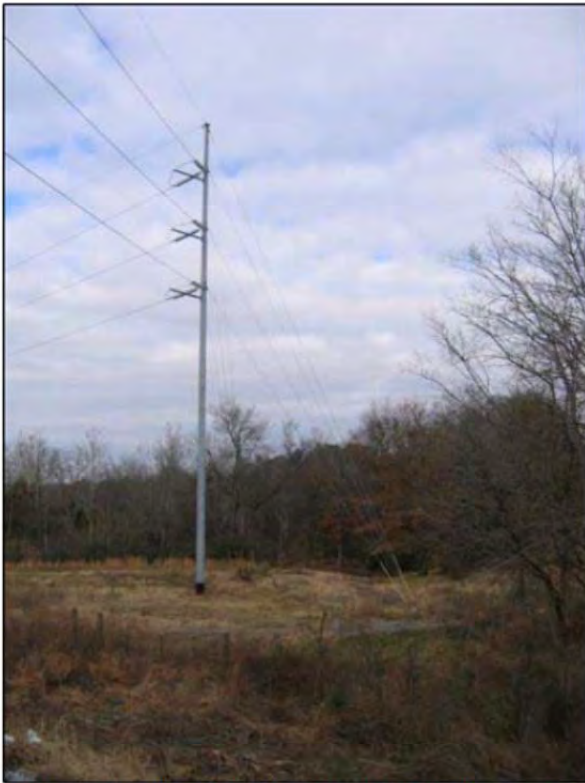
Figure 3. Single pole structure similar to those proposed for the current project.
