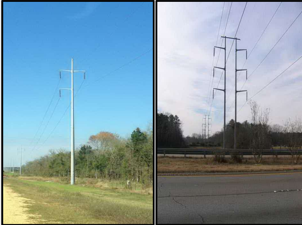
Figure 2-1 Typical Single Steel-Pole and Double Steel-Pole Structures
