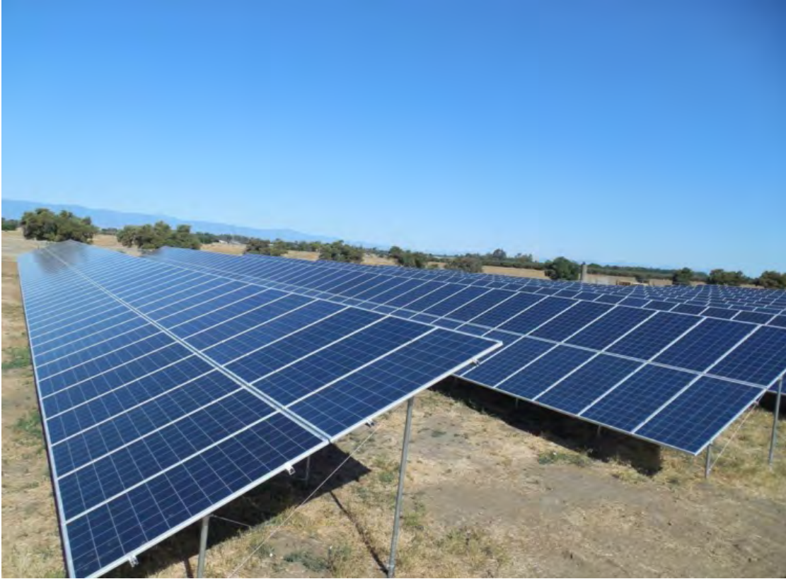
Figure 2-6. Photovoltaic array – Option 2, fixed-tilt example.
