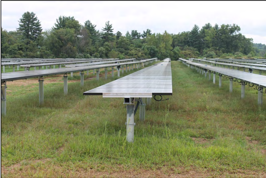
Figure 2-5. Photovoltaic array – Option 1, single-axis tracking example.
