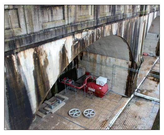
**Concrete Arch Showing Spalling and Efflorescence**
