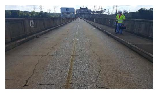
Figure 7: Typical Deck Cracking
