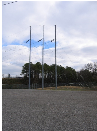
Photo 2.2-2. Example of three-pole structure
