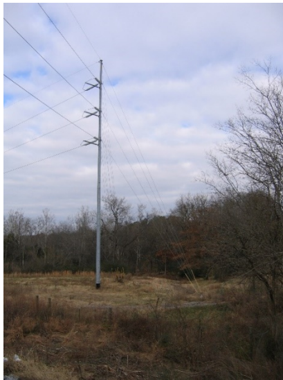
Photo 2.2-1. Typical single-pole structure
