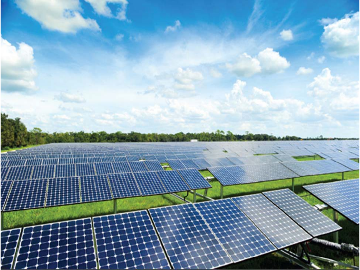
Photo 3.5-9. Single-axis, tracking photovoltaic system with panels showing some tilt as viewed from the east or west
