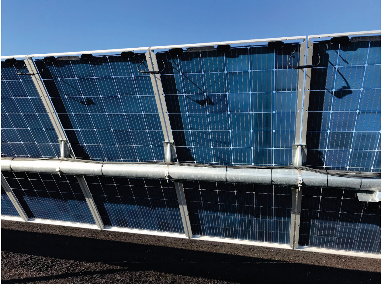
Photo 3.5-10. The backside of the single-axis tracking photovoltaic solar panels.
