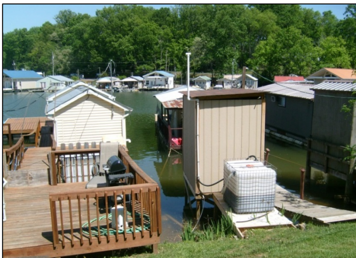
Figure 1.3-12. Shore-based sewage holding tank
