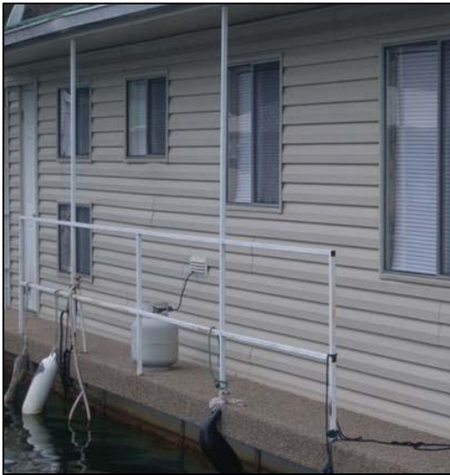
Figure 1.3-11. Propane tanks as floating house fuel source
