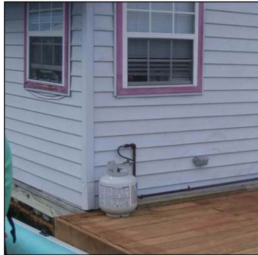
Figure 1.3-11. Propane tanks as floating house fuel source
