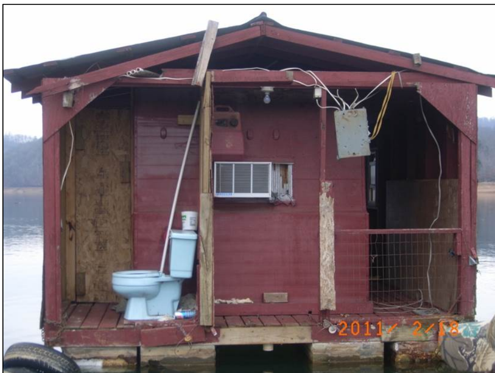
Figure 1.3-19. Derelict floating house with unknown wastewater disposal
