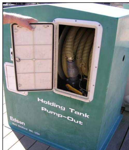
Figure 1.3-14. Holding tank pump-out system
