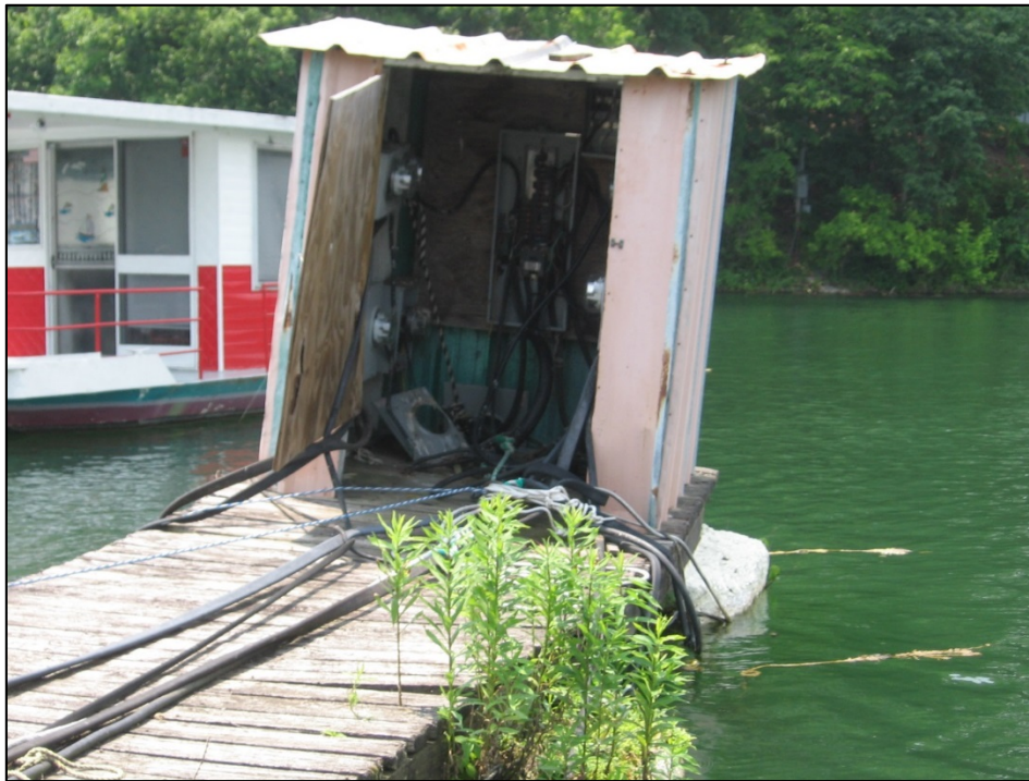
Figure 3.4-5. Unsafe electrical system
