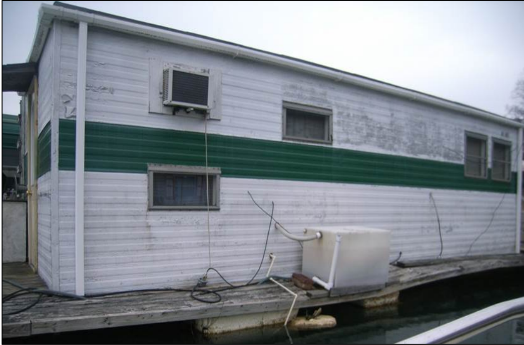
Figure 1.3-16. Sewage capture at floating house and grey water discharge pipe
