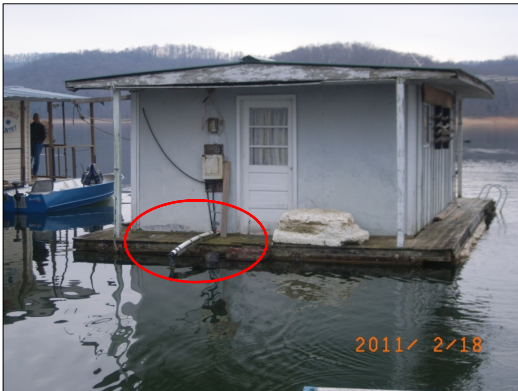
Figure 1.3-17. Wastewater discharge pipe in red circle
