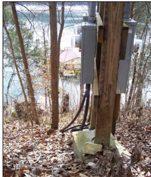
Figure 1.3-5. Onshore electrical junction for underwater lines to floating houses
