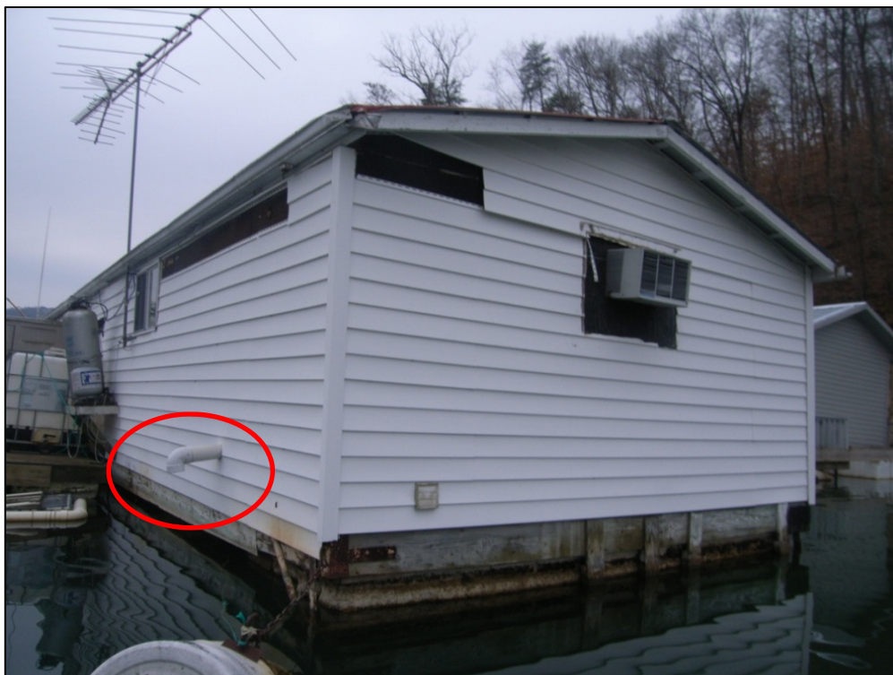
Figure 1.3-18. Wastewater discharge pipe in red circle
