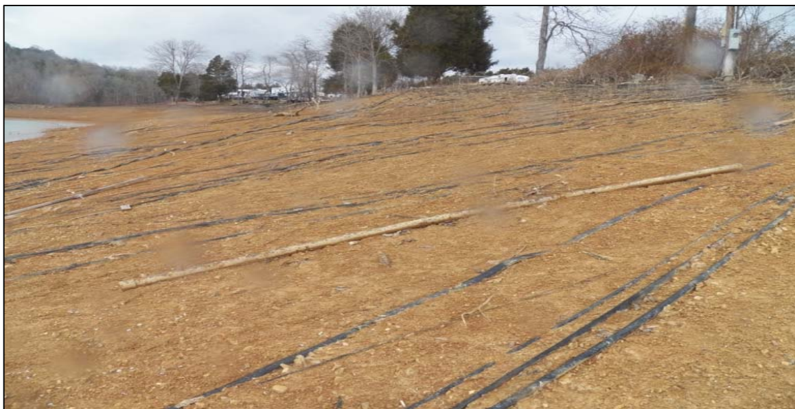
Figure 1.3-6. Electrical underwater lines to floating houses, exposed due to low water levels during winter drawdown
