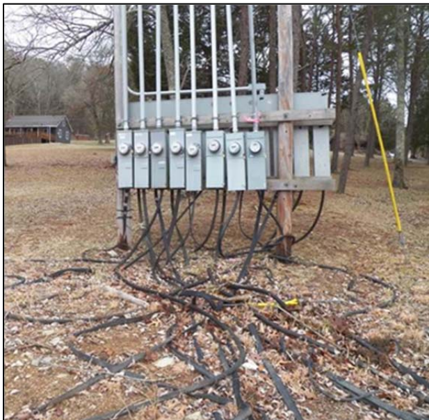
Figure 1.3-4. Onshore electrical junction for underwater lines to floating houses
