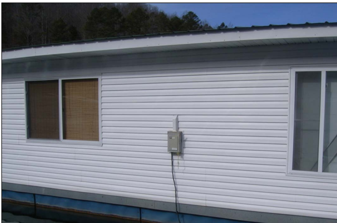
Figure 1.3-7. Electrical connection to floating house from underwater electrical line
