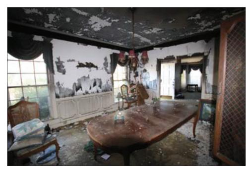
Figure 4.14. Example of MD-IP-2 interior fire damage within the central block dining room (view to the southeast).
