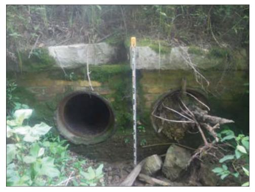
Figure 5.24. Culvert 2 in 40MD267, constructed of ferrous metal pipes, brick, and limestone (view to the southwest).
