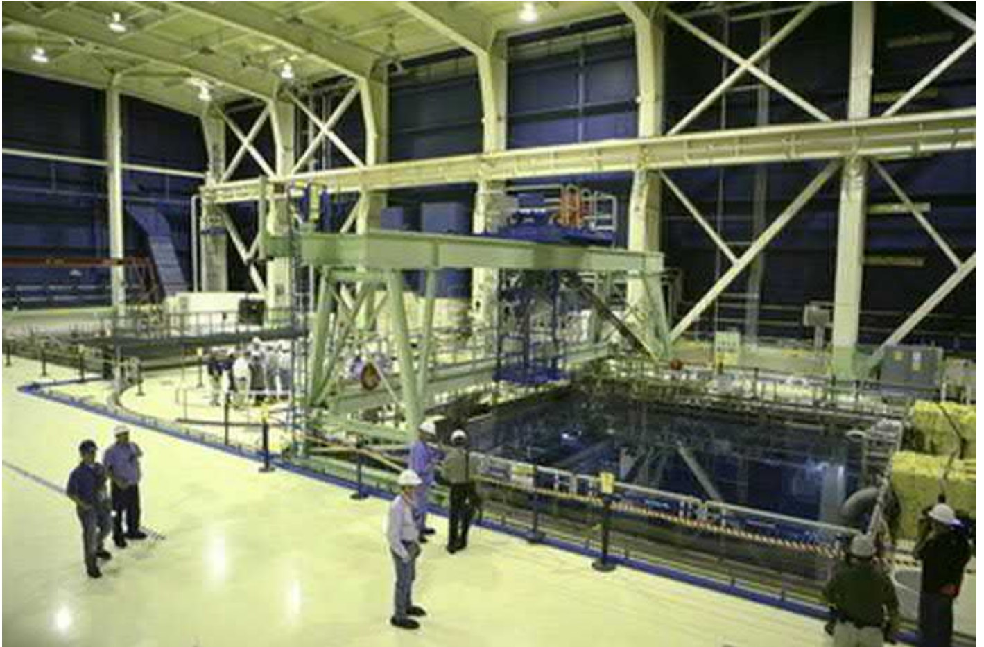
The top floor of the reactor building at Browns Ferry Nuclear Plant shows the cover of Unit 1 and the spent fuel storage tank where 29 feet of water covers the rods. (Michael Mercier/ The Huntsville Times)
