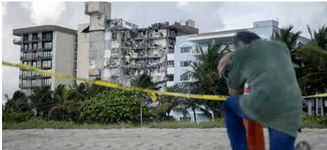
A man prays Friday near where search and rescue operations are ongoing at the partially collapsed 12-story Champlain Towers South condo building in Surfside, Fla. (photo: Joe Raedle/Getty Images)
