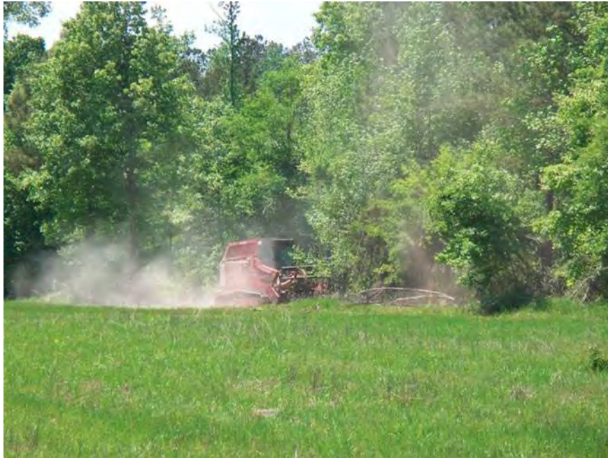
Removal and mulching of trees along an existing TL ROW that are encroaching on the easement
