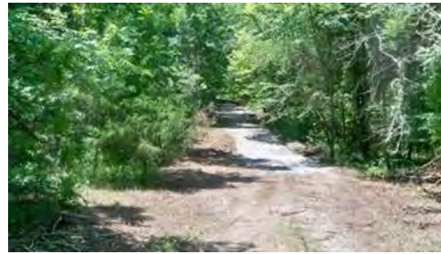
Re-graveling/re-grading along access road
