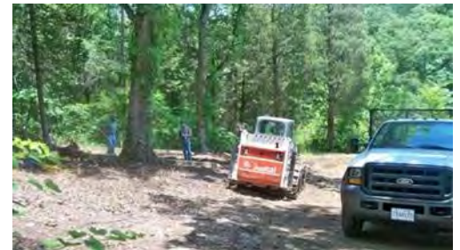
Re-graveling/re-grading along access road
