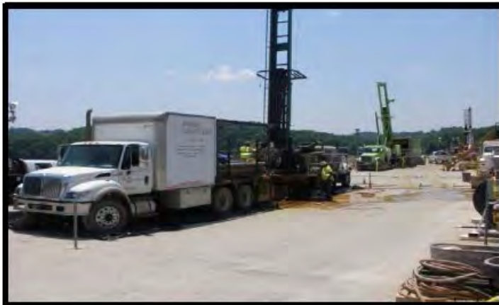
Crest Drilling and Grouting Looking West
