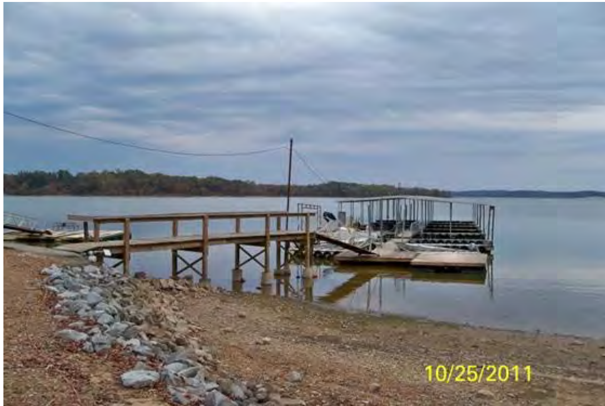
Marina boat slips with riprap in foreground
