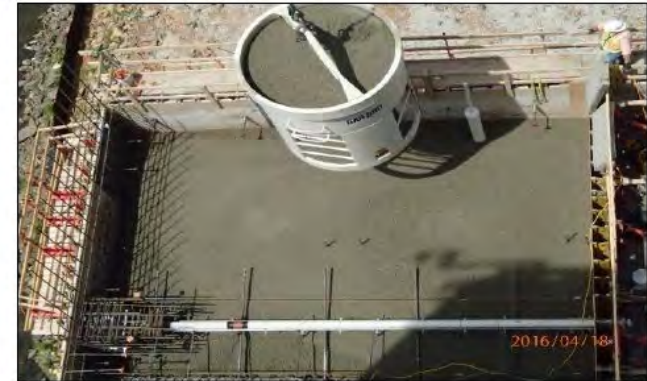
L17C Lift 5 mid-placement
