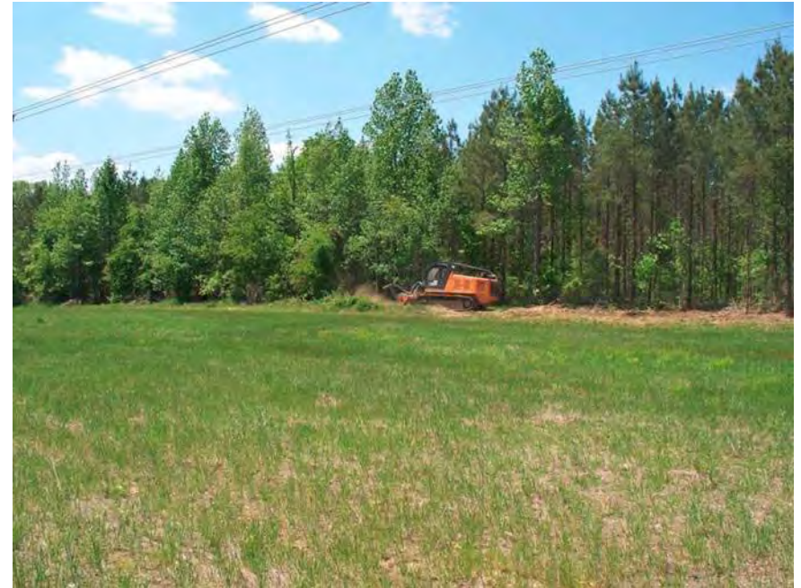
Removal and mulching of trees along an existing TL ROW that are encroaching on the easement
