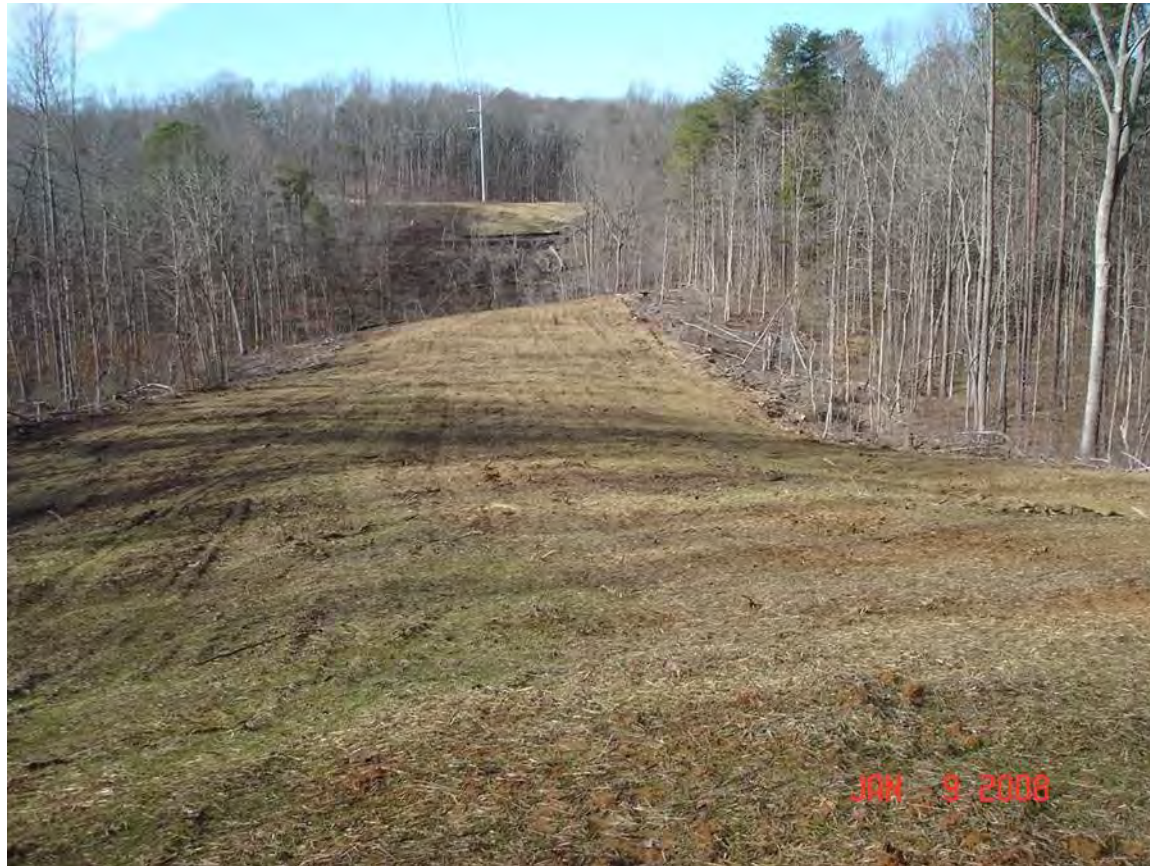
Tree removal spanning ravine - BMP
