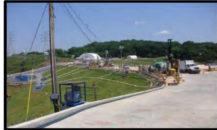
Crest Drilling and Grouting Looking East
