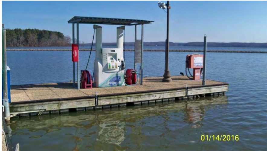
Marina fuel station
