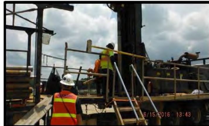
BSC 1379 - Sonic rig 3 completed sonic drilling down to 117.3'.
