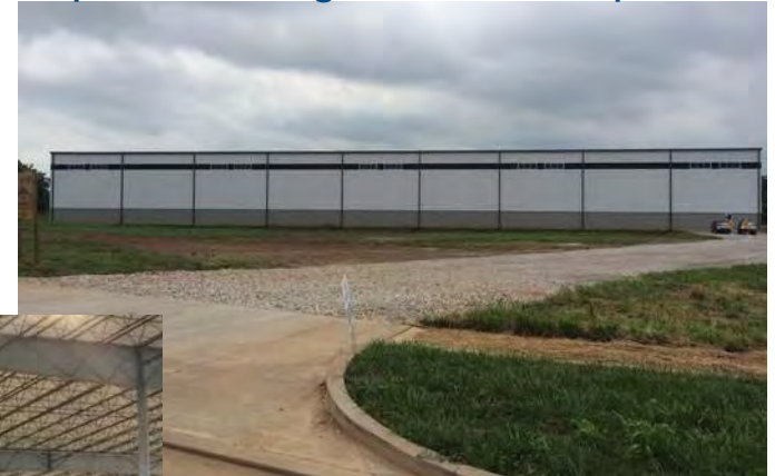
Spec. building on concrete pad
