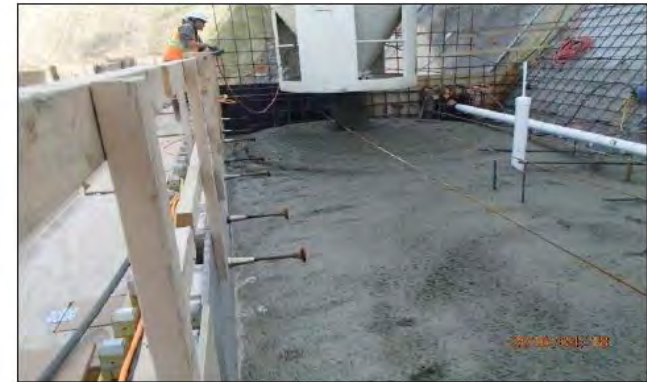
L17A Lift 5 mid-placement.
