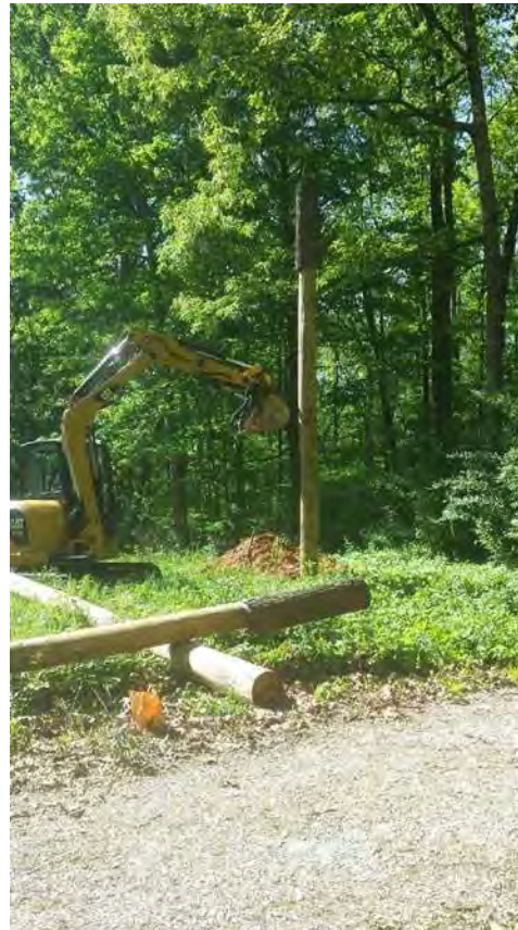
Installation of artificial bat roosts
