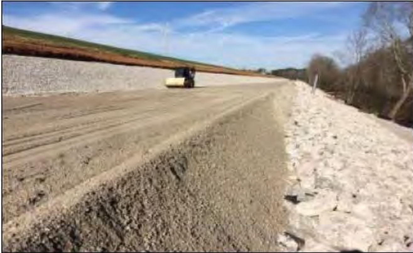
Temp slope protection, work platform, bank restoration
