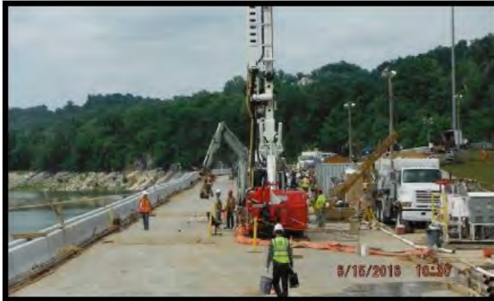
BTR 1651.5 - LMG grouting rig B setup and started LMG grouting.
