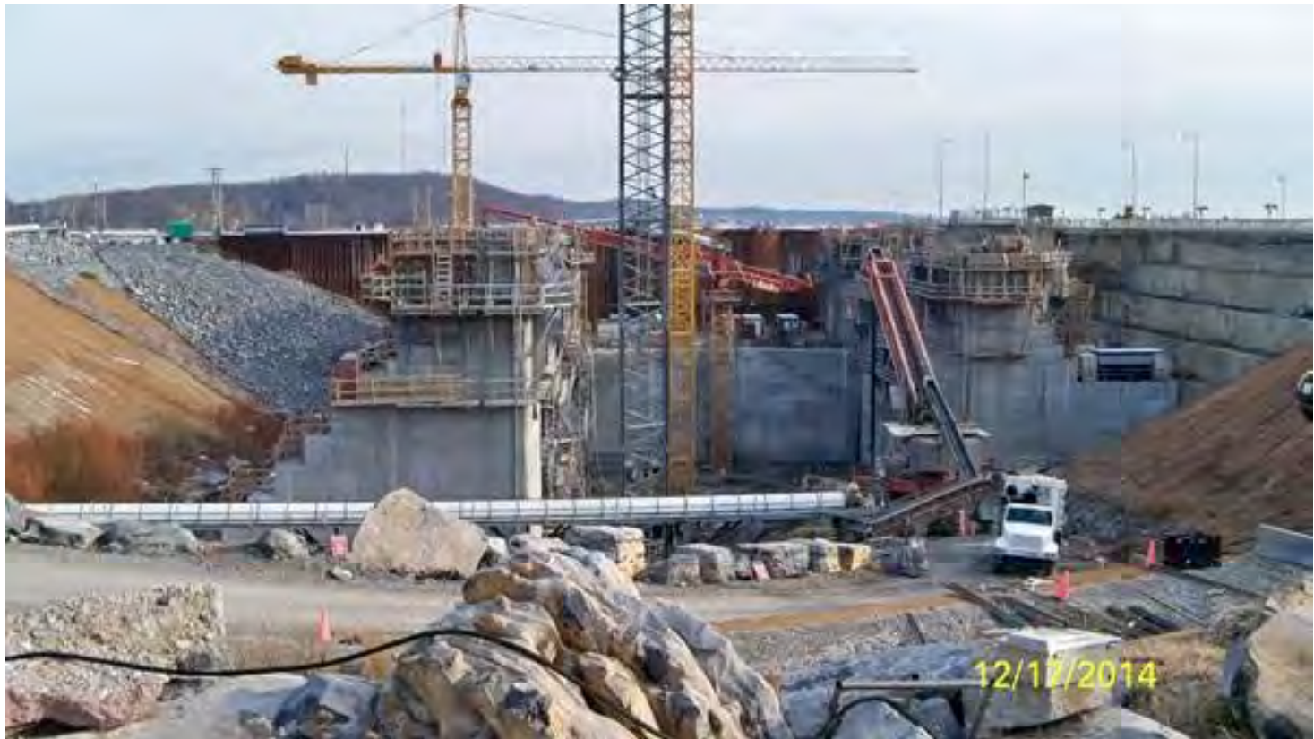
Construction – Lock at Kentucky Dam
