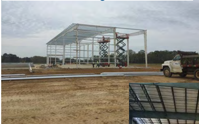
Industrial building construction
