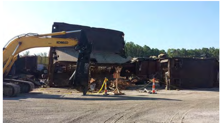
Gallatin FP – ductwork demolition
