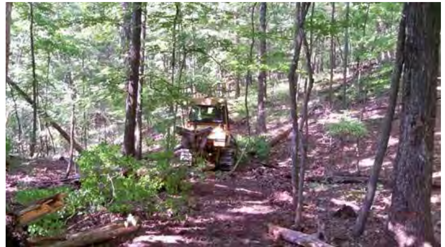
Constructing fire lines for planned burn
