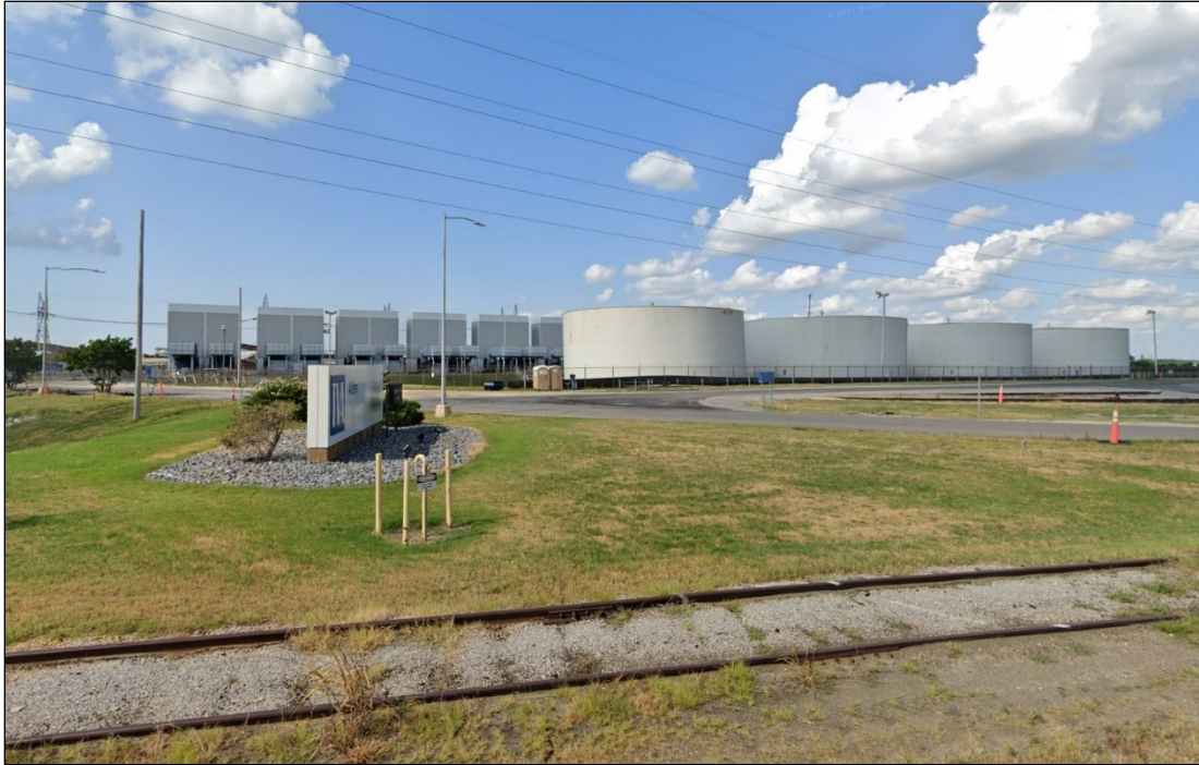
Figure 5. ACT, as seen from Plant Road. Google Street View; image dated July 2021.
