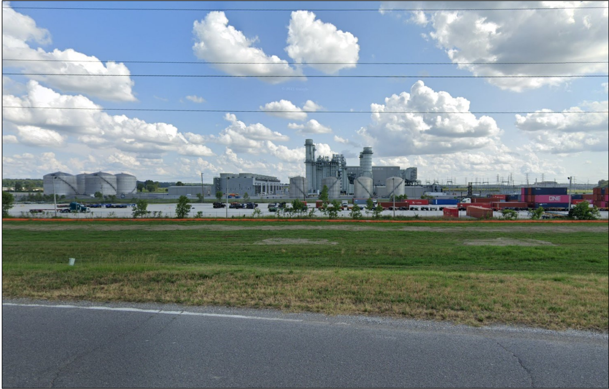
Figure 6. ACC, as seen from Plant Road. Google Street View; image dated July 2021. Note CMC Container Maintenance facility in middle ground.
